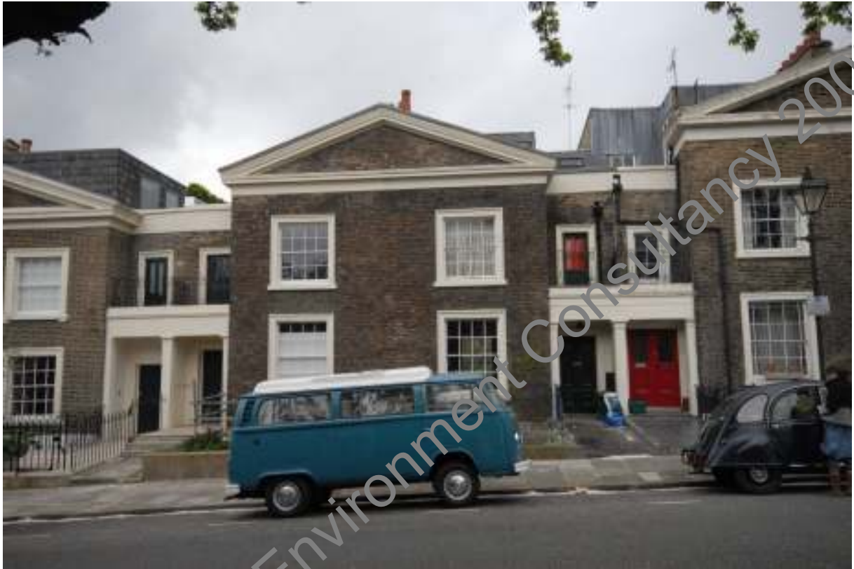
Plate 10: Wharton Street Roof Garden
