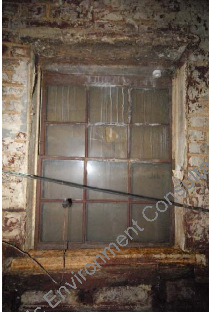
Plate19 Original Basement Window
