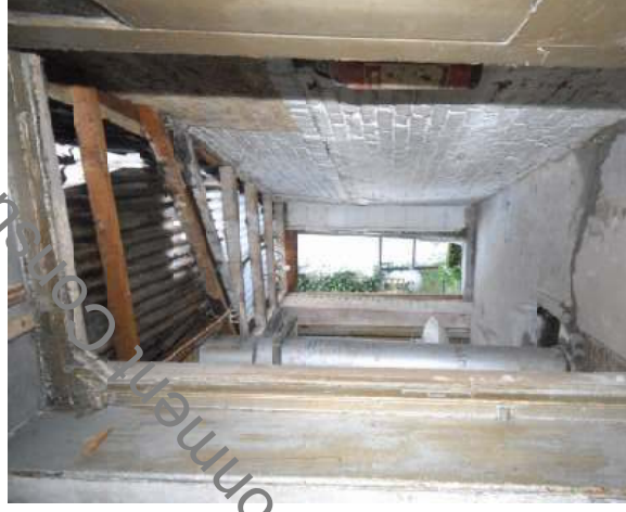
The Lean To Extension
