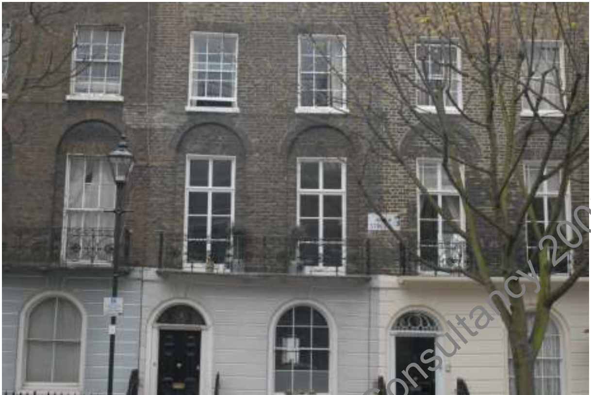
Plate35 Doors to Balcony River Street.
