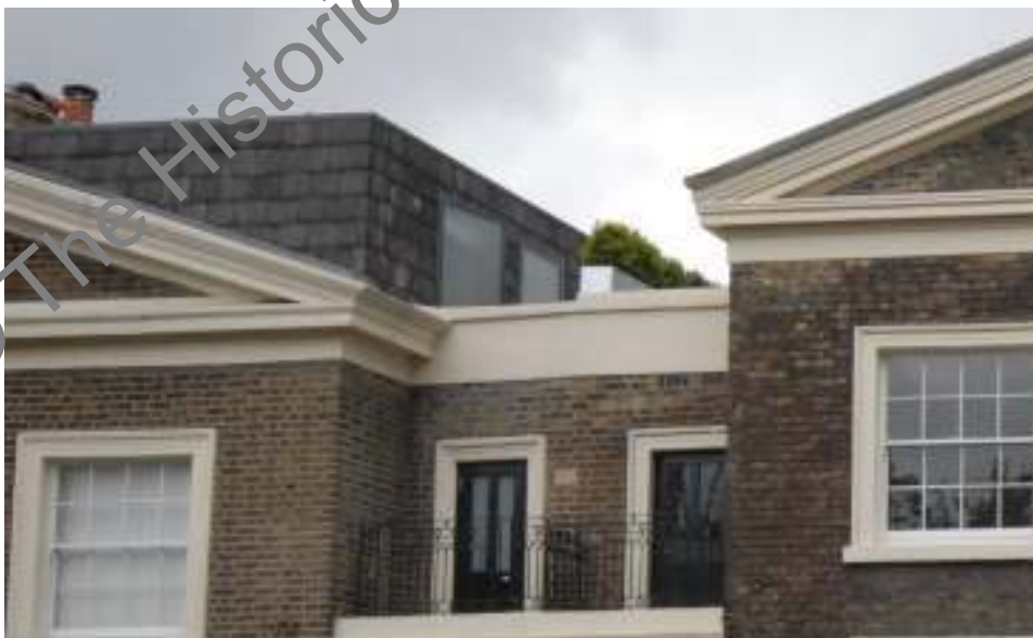
Plate 11: A hedge has been used as a boundary at third floor level Wharton Street
