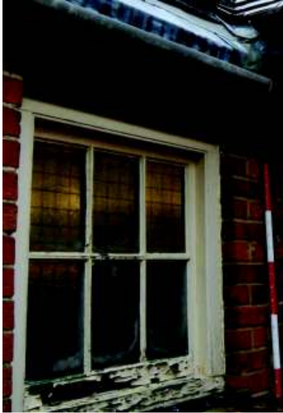
Plate 14: Eastern window, unit 2, south elevation, showing different lintel
