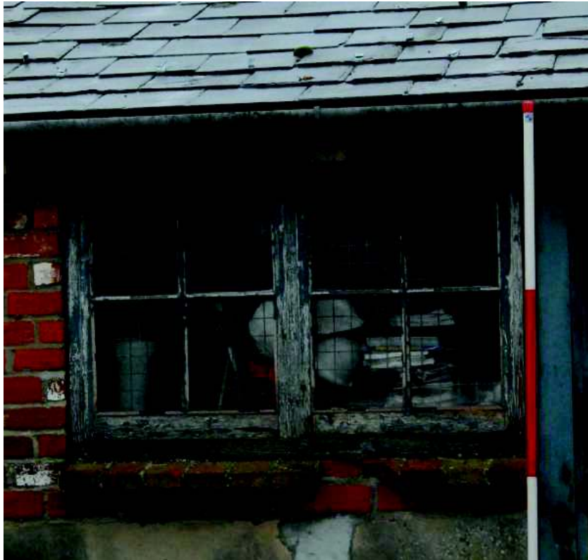
Plate 24: Detail of window, unit 6
