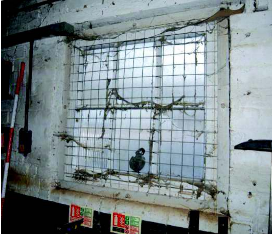
Plate 6: Interior of window, unit 1
