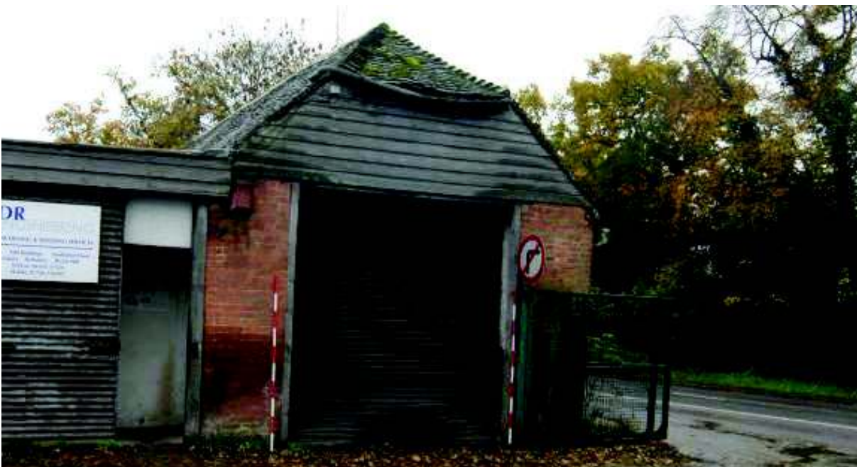
Plate 18: Unit 4 north elevation
