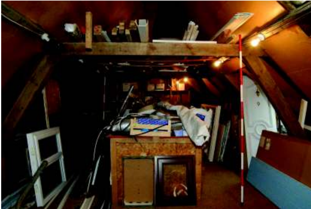
Plate 35: Roofing timbers of unit 7
