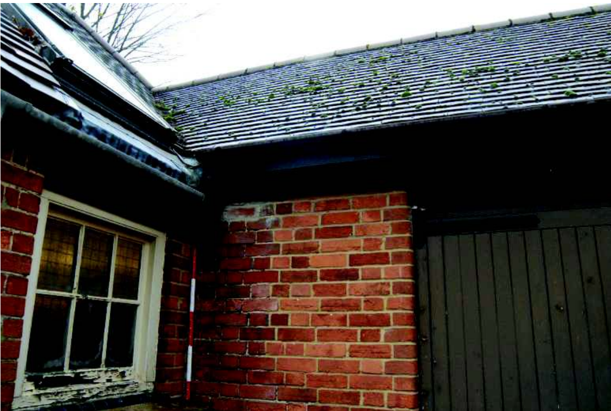
Figure 10: Corner of units 2 and 3, showing original brickwork in wall of unit 3
