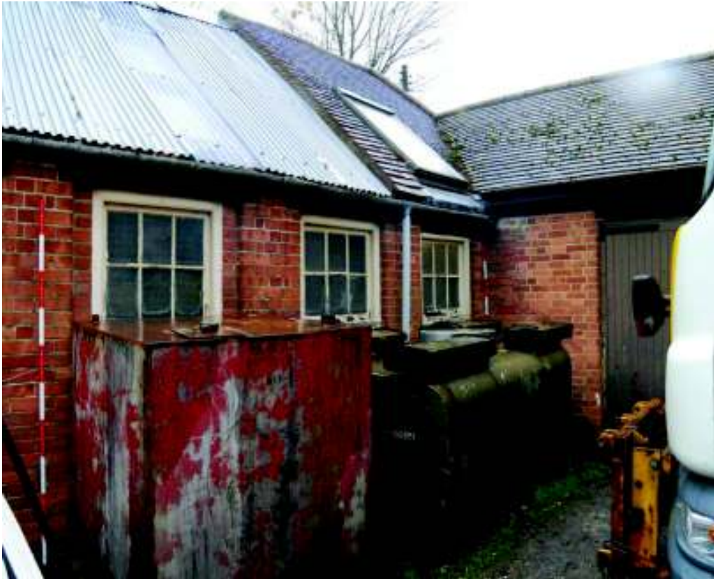
Plate 12: Unit 2 south elevation, east end
