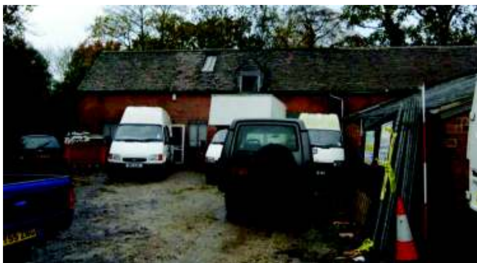
Plate 26: Unit 7 east elevation partially obscured
