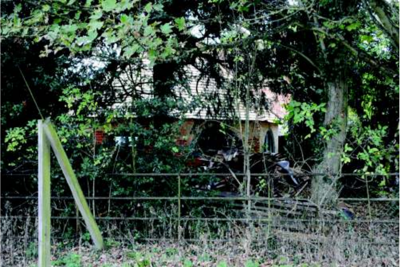
Plate 45 View of The Dairy from The East
