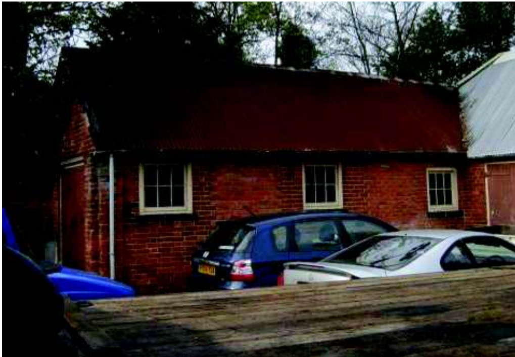
Plate 3 East elevation, unit 1
