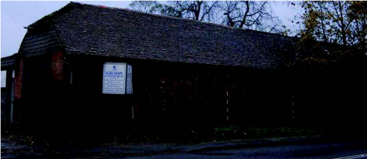
Plate 19: Western elevation, unit 4
