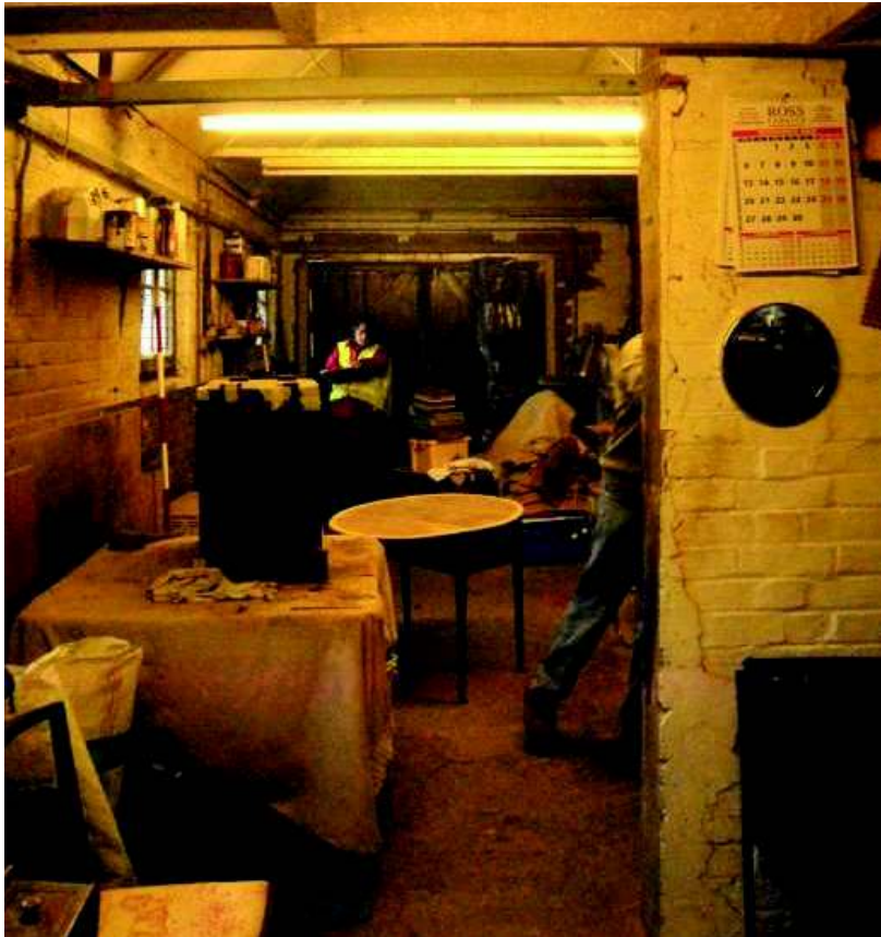
Plate 7: Unit 1 from north, viewed through partially demolished wall
