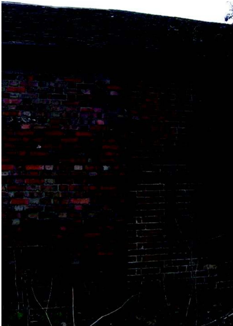
Plate 20: Join between unit 4 (left) and unit 7 (right) is clear from the western elevation
