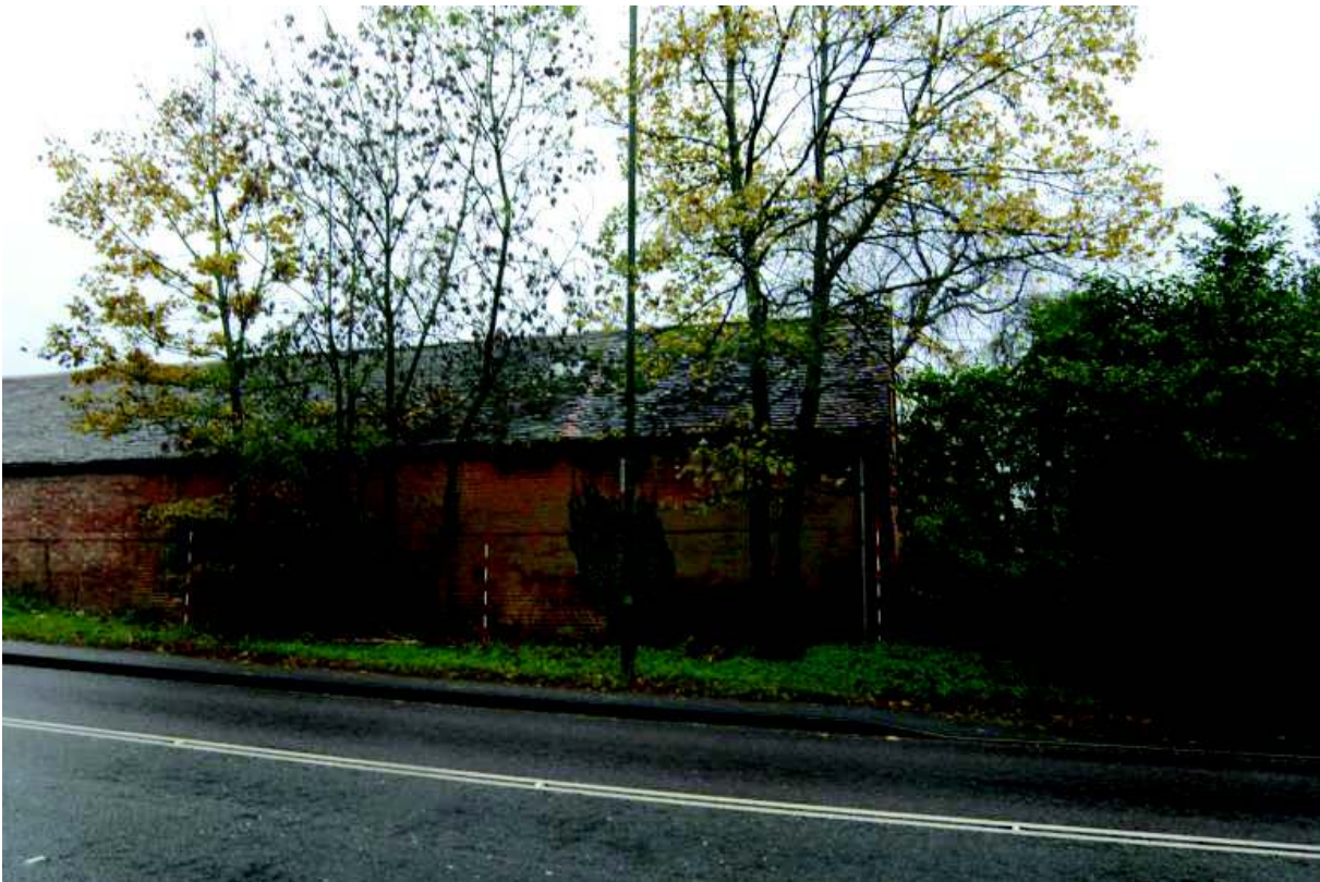
Plate 30: West elevation, unit 7
