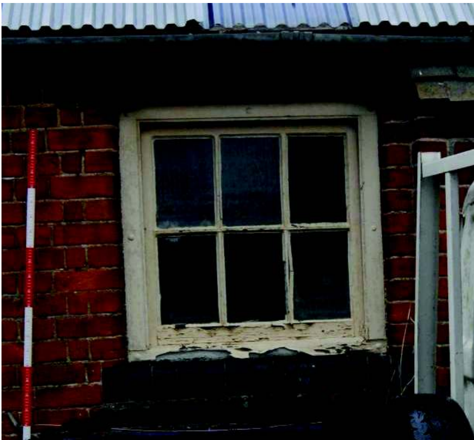
Plate 13: Window, unit 2, showing lintel
