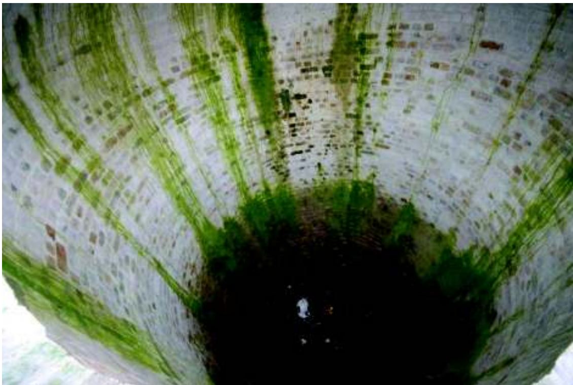
Plate 39: The internal structure of the ice house (Avoncroft Museum of Buildings)
