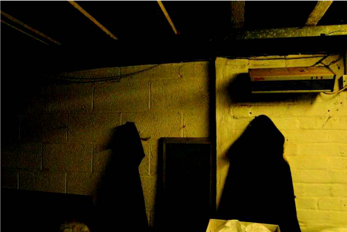
Plate 8: Unit 1, modern partition wall to unit 2 (left), original wall (right)
