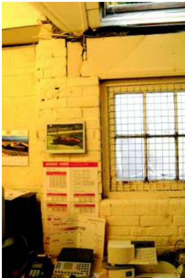
Plate 15: Unit 2 internal, showing original wall of north-south range
