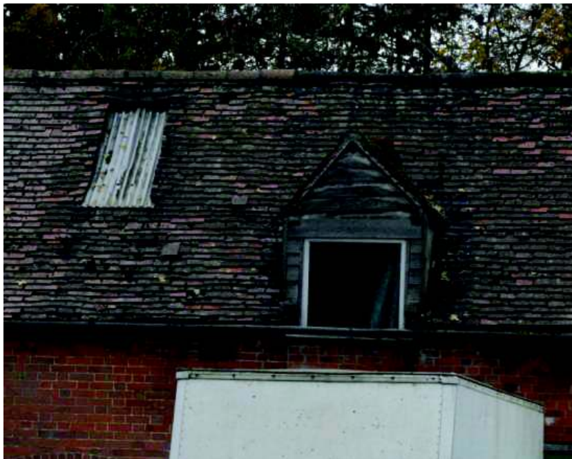
Plate 28: Detail of roof, east side, showing dormer and roof window
