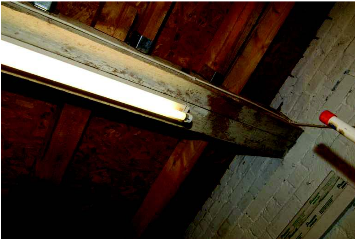
Plate 34: Modern north-south timbers and original east-west timbers supporting upper floor
