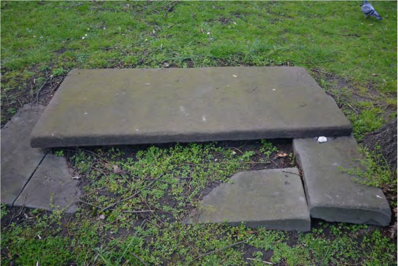
Plate 53 Damaged Grave Markers
