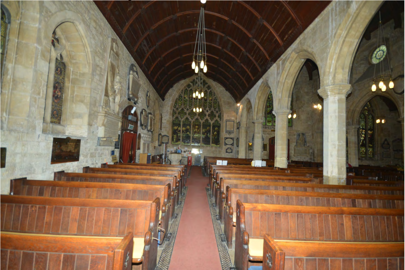
Plate 15 The South Aisle
