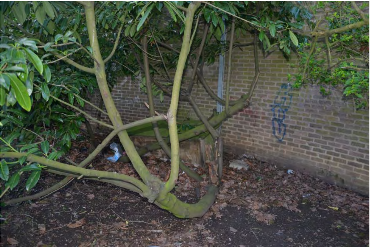
Plate 54 Damage to a Table Tomb
