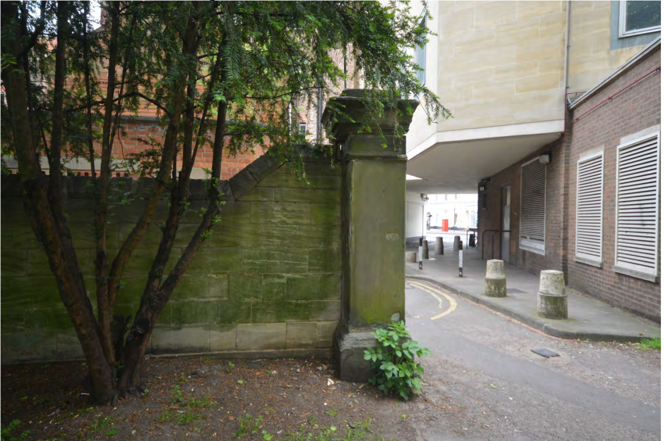
Plate 29 Gate Pier Church St South
