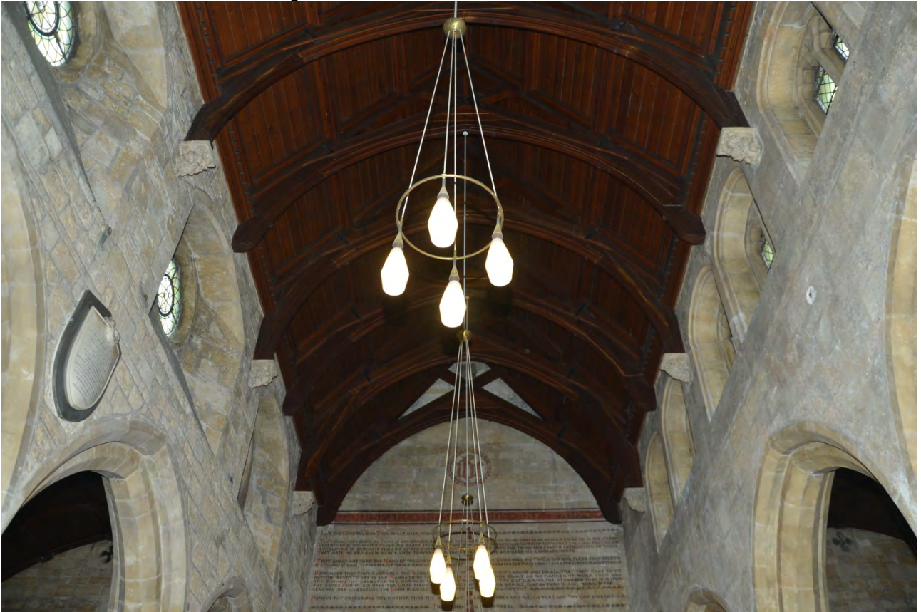
Plate 19 The Nave Roof
