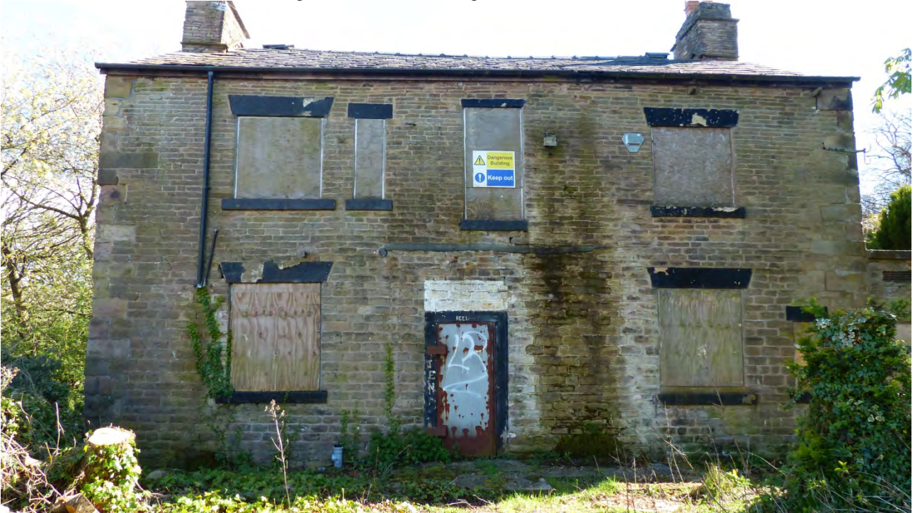
Plate 6: North elevation, building 3
