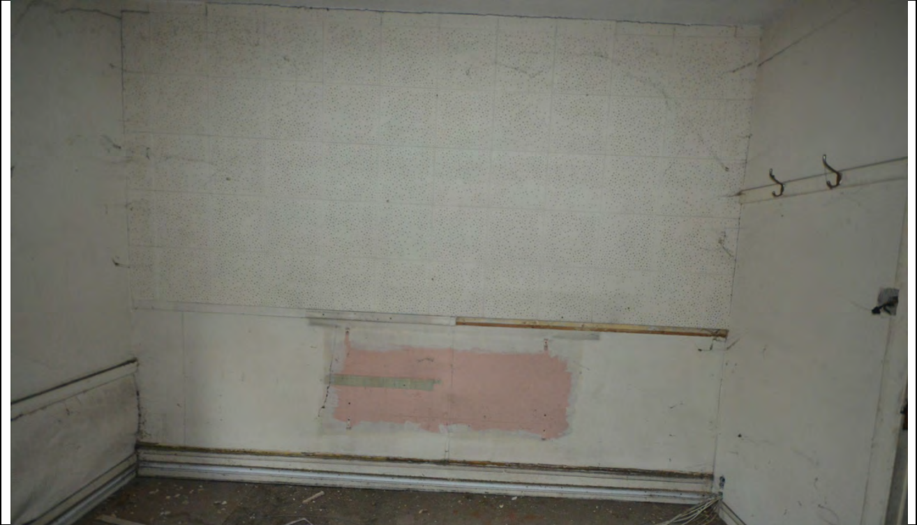
Plate 18: First Floor Room 2 Looking North
