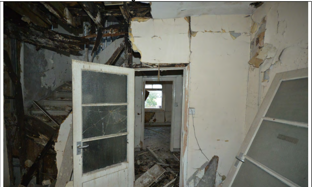
Plate 25: First Floor Room 3 Looking West
