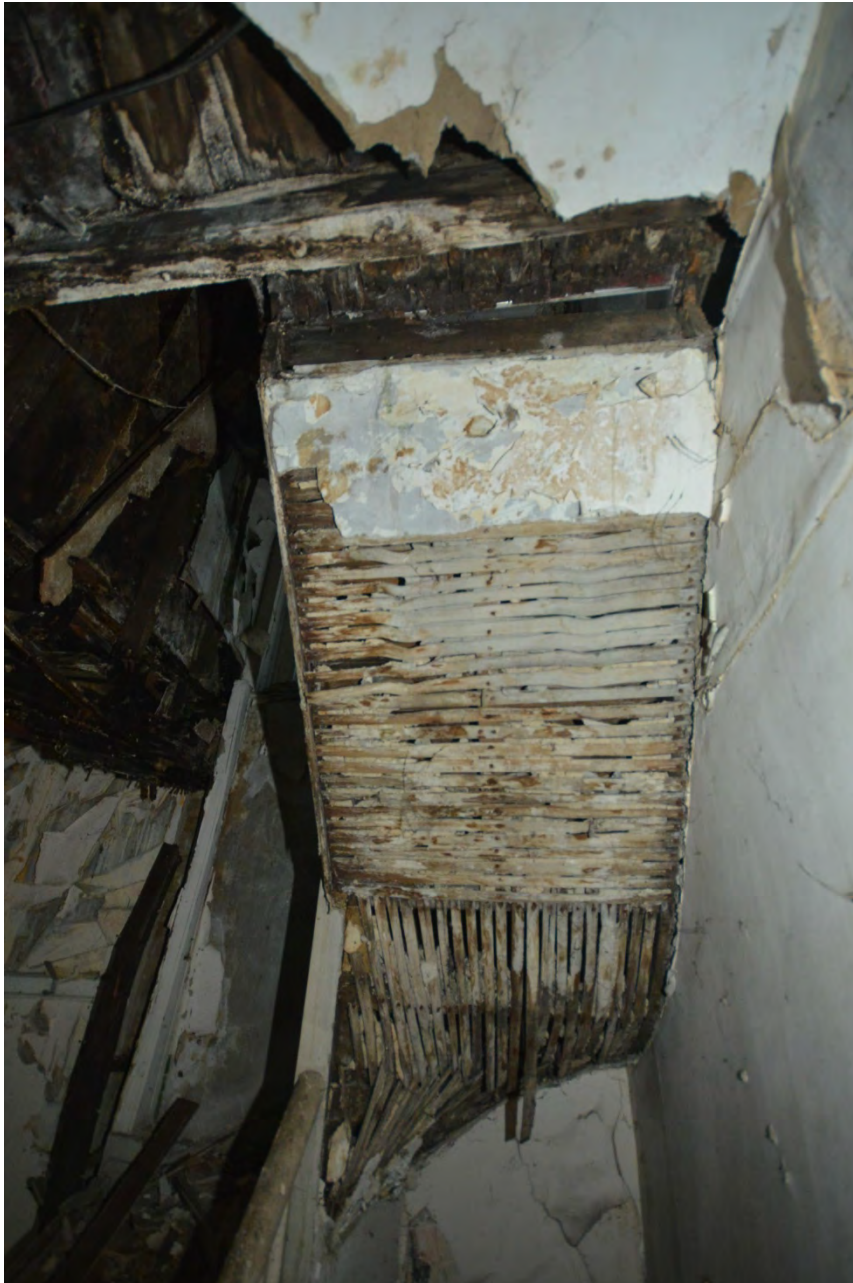
Plate 26: Underside of staircase to second floor
