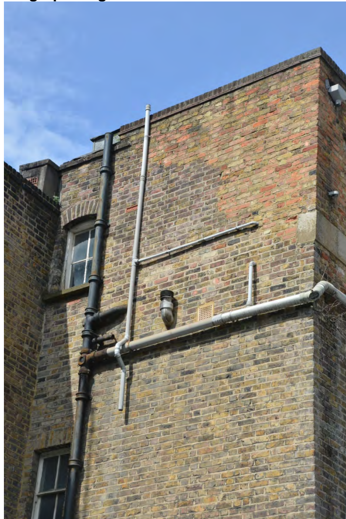
Plate 10: Detail of south elevation
