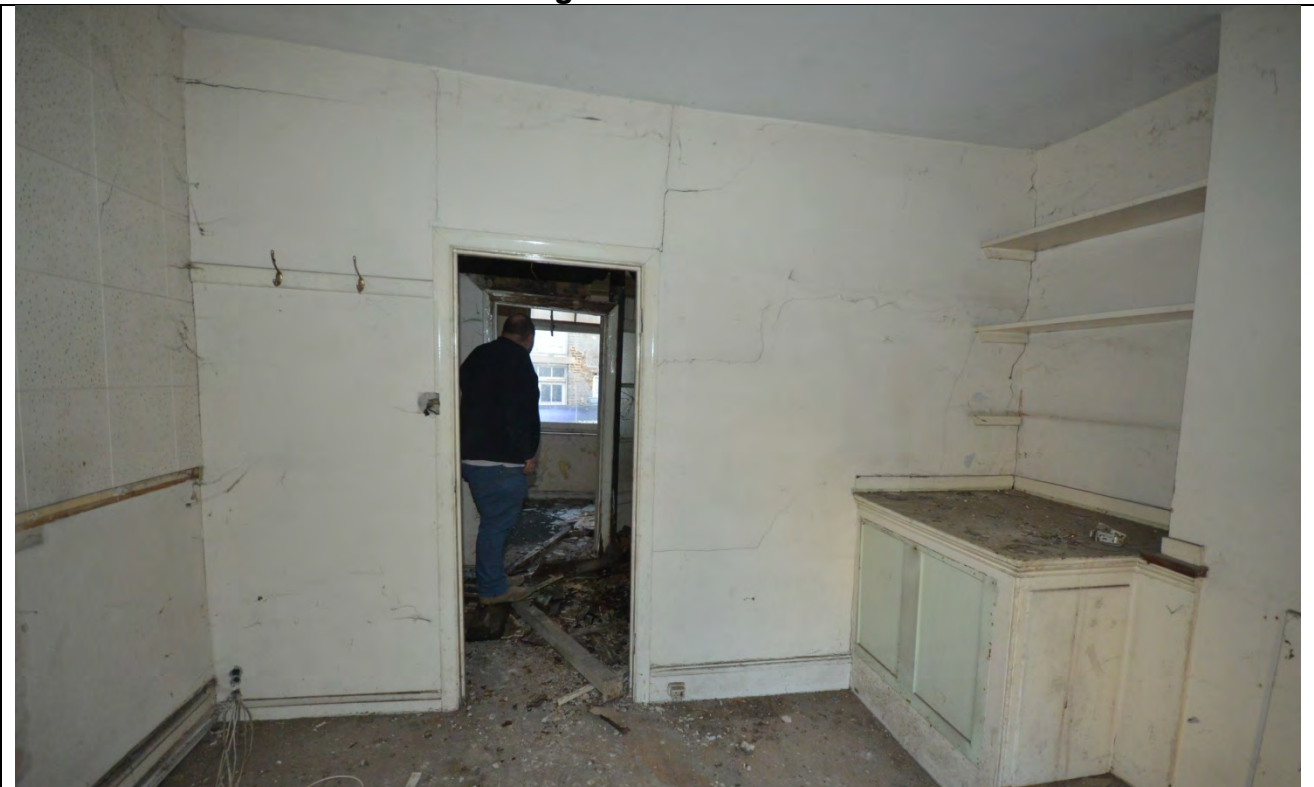
Plate 19: First Floor Room 2 Looking East
