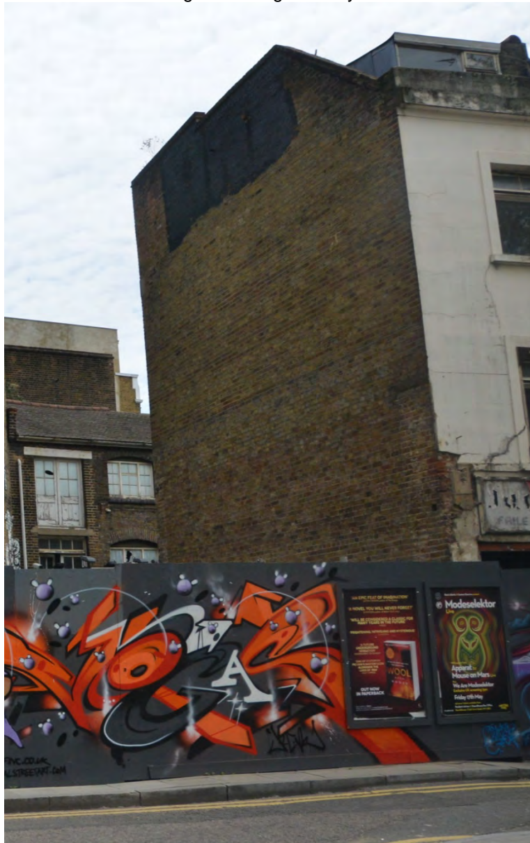
Plate 7: North aspect The northern wall is plain yellow/red brick.
