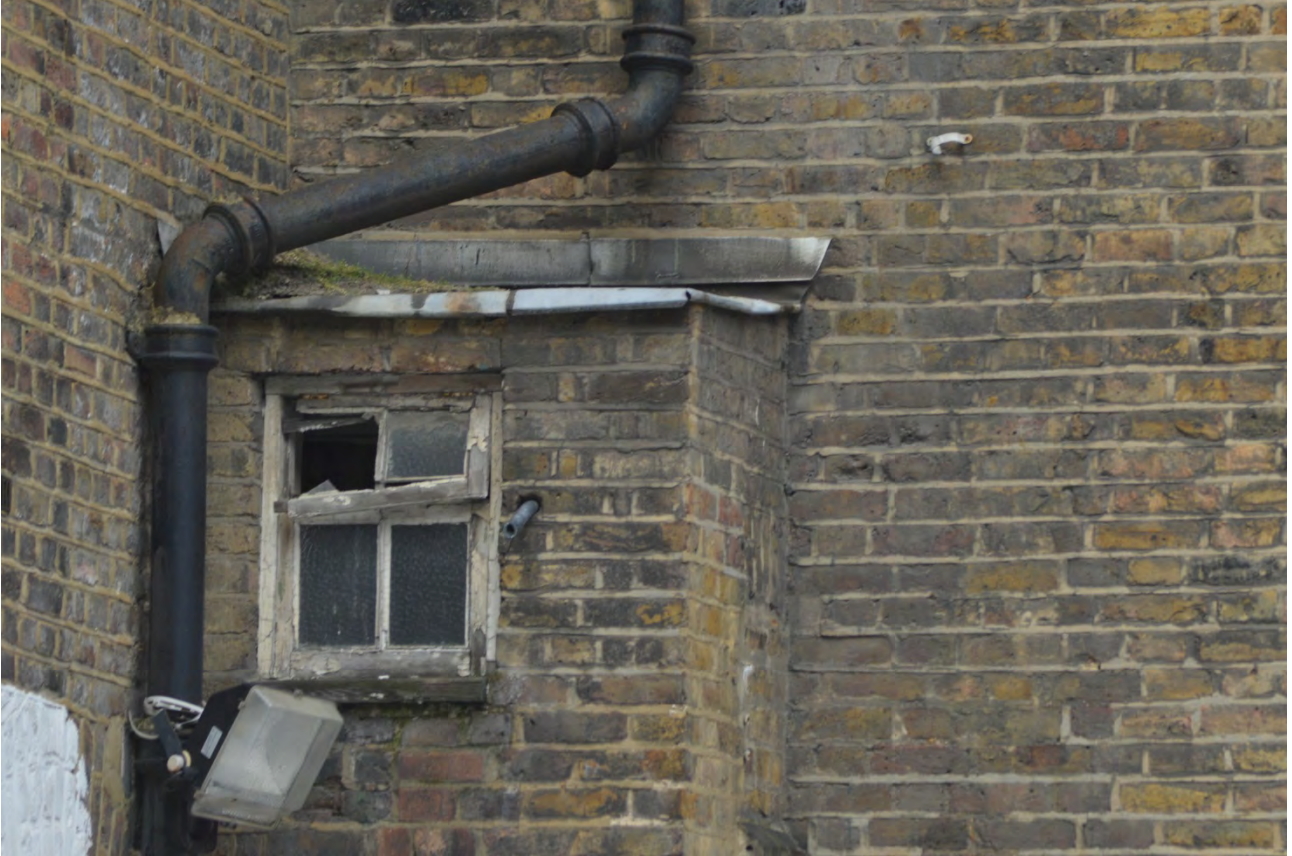
Plate 11: Detail of projecting lavatory section
