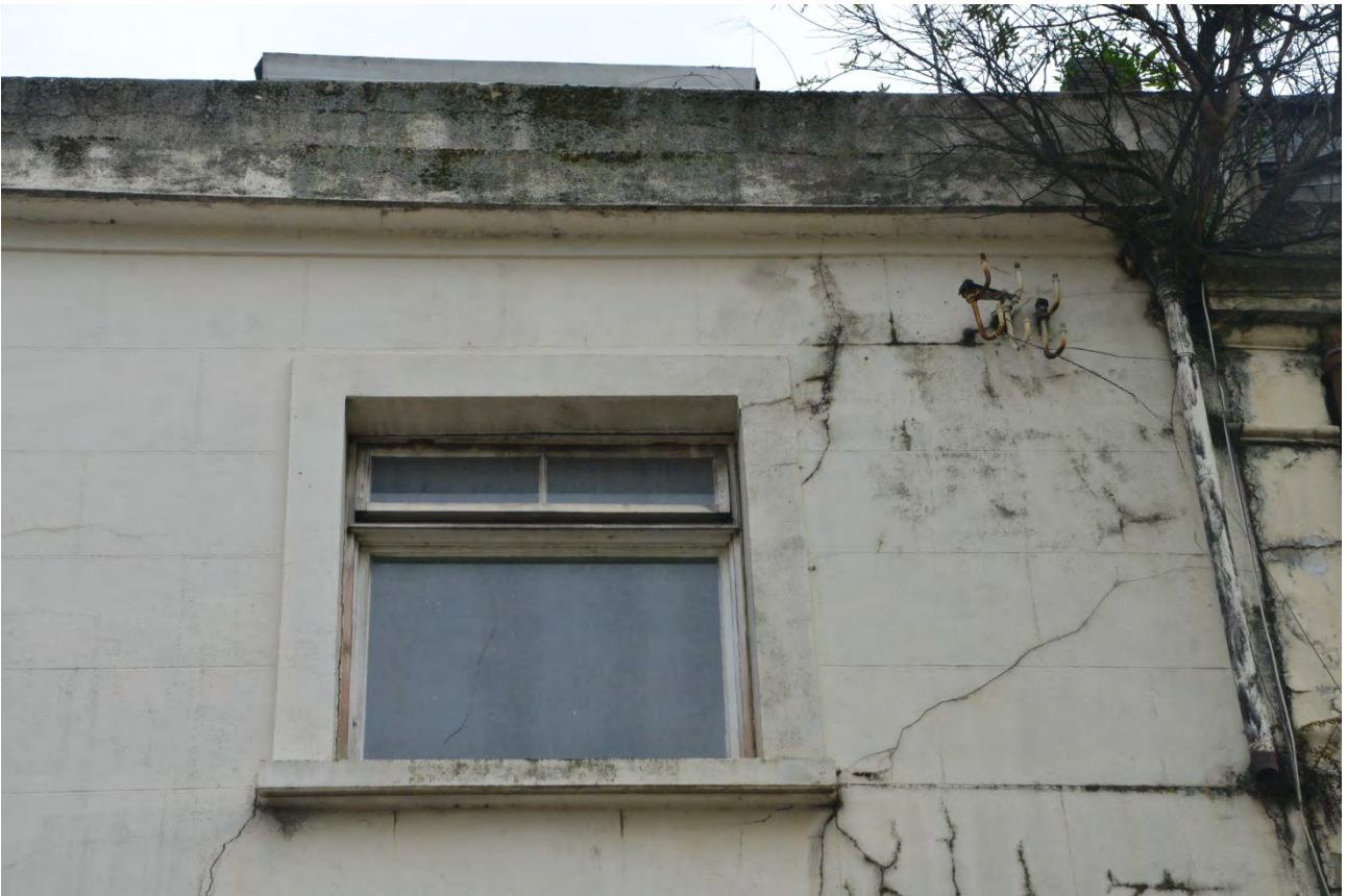
Plate 6: Detail of parapet and first floor window
