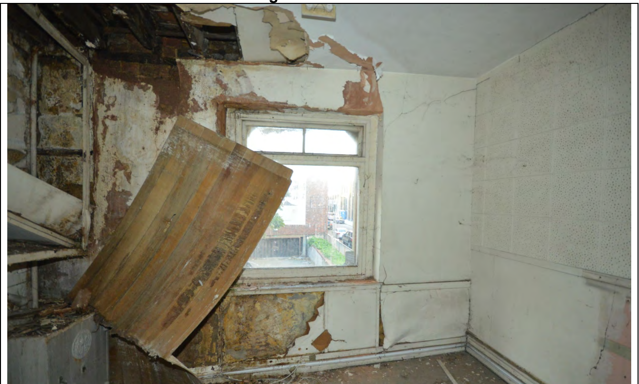
Plate 21: First Floor Room 2 Looking West
