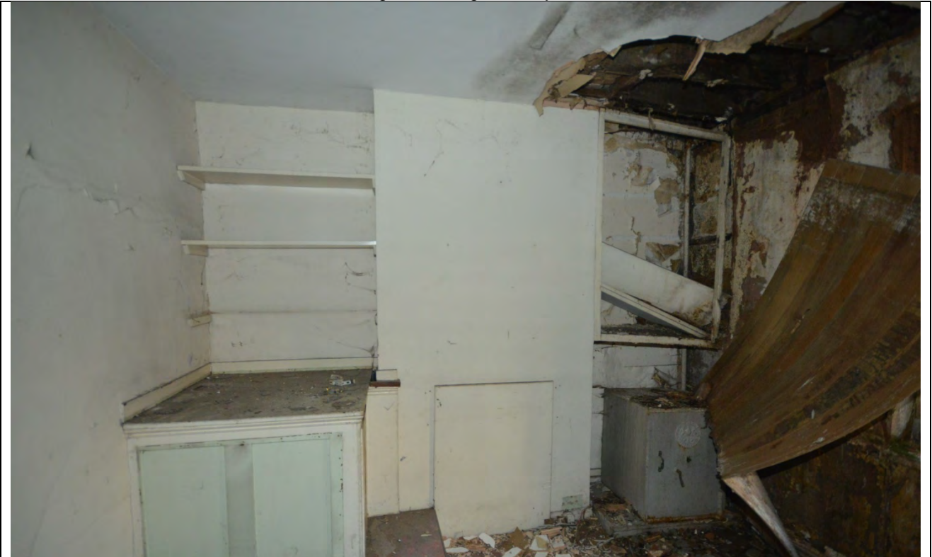
Plate 20: First Floor Room 2 Looking South
