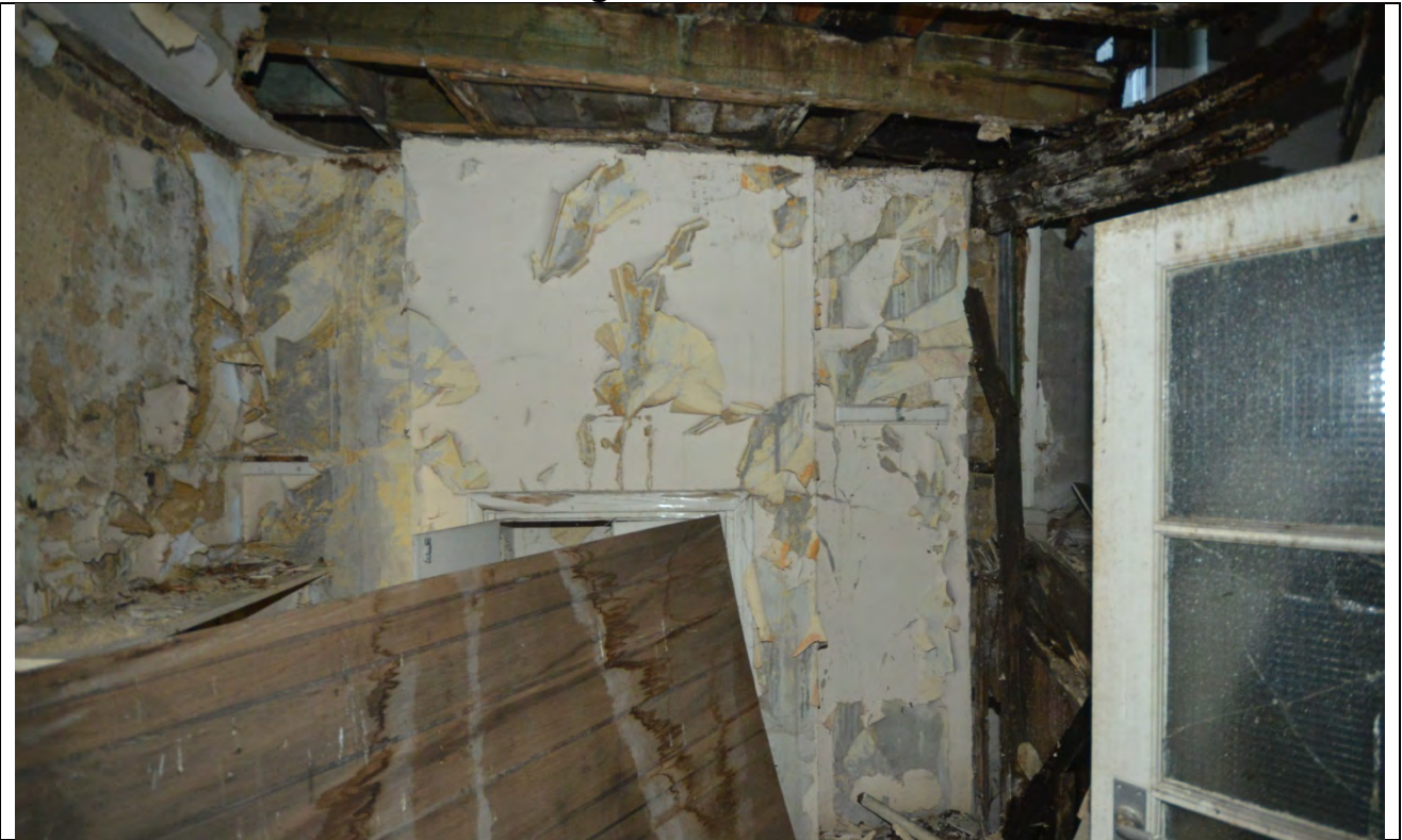
Plate 24: First Floor Room 3 Looking South
