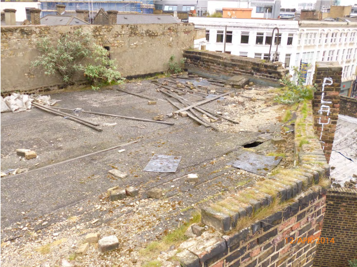
Plate 21: Roof over 63 Great Eastern Street
