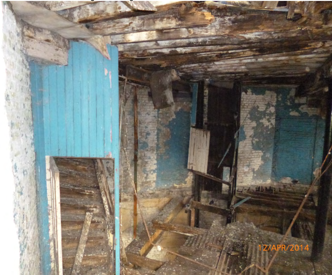
Plate 35: First floor, showing staircase
