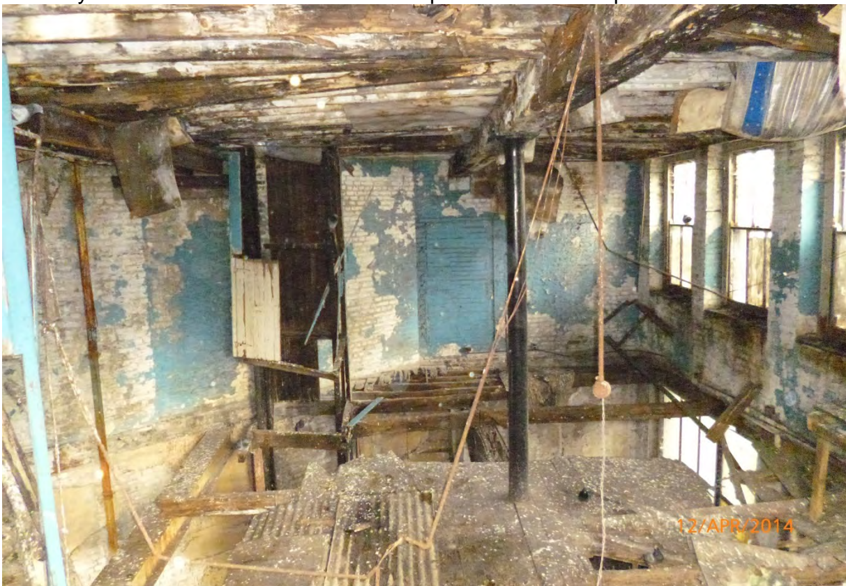
Plate 34: West view, first floor
