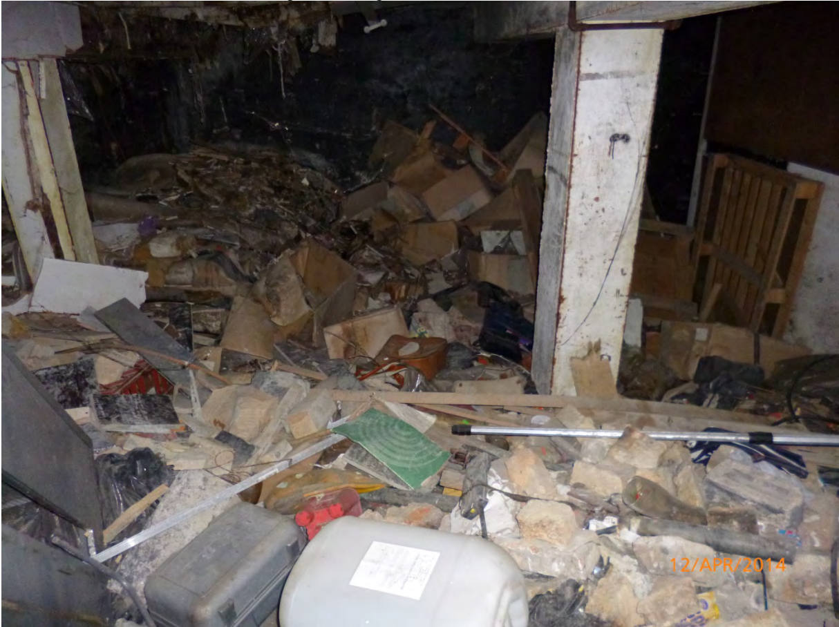
Plate 60: Ground floor, northern part of building
