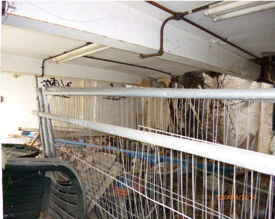
Plate 64: Northern room, first floor
