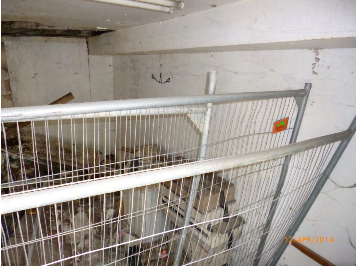
Plate 63: Northern room, first floor
