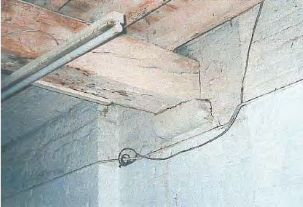
Plate 54: Detail of main beam and corbel, 2nd floor (Shaya 2000)
