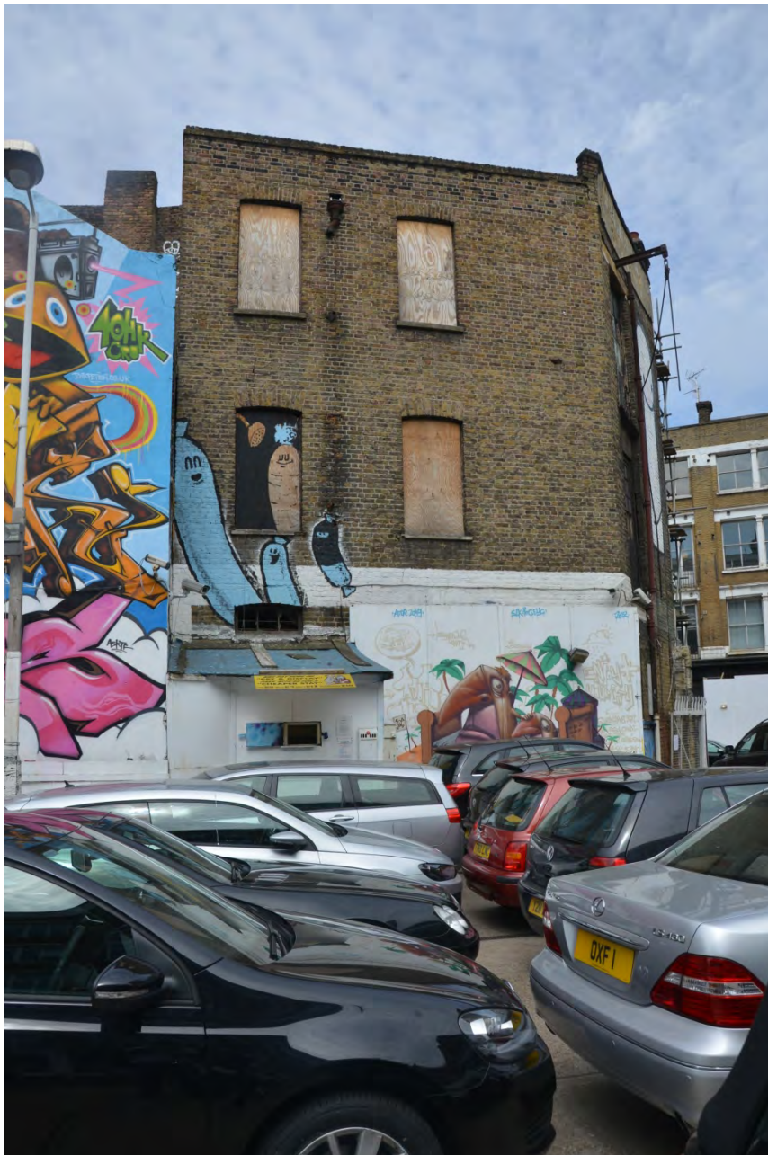
Plate 18: Rear elevation, east of gable
