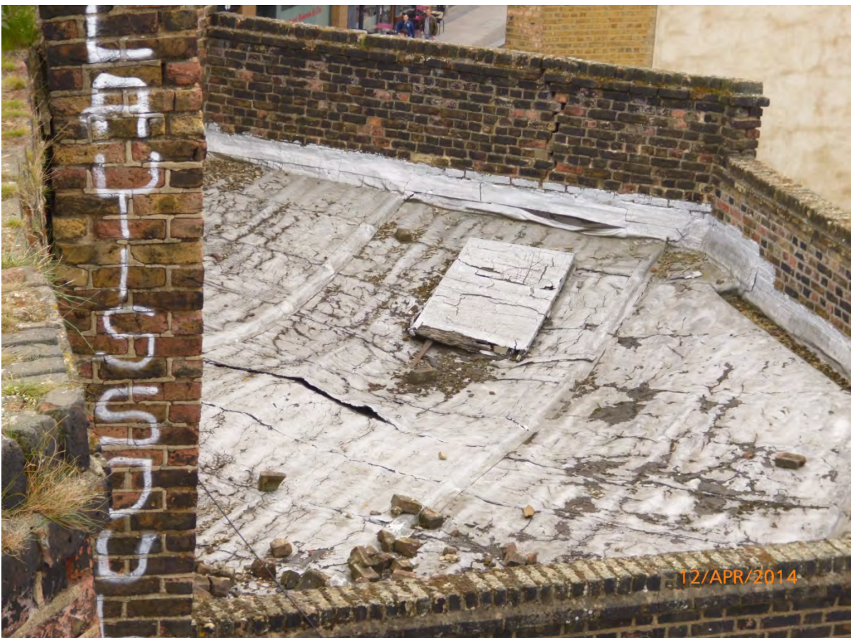
Plate 22: Detail of roof hatch, 61 Great Eastern Street
