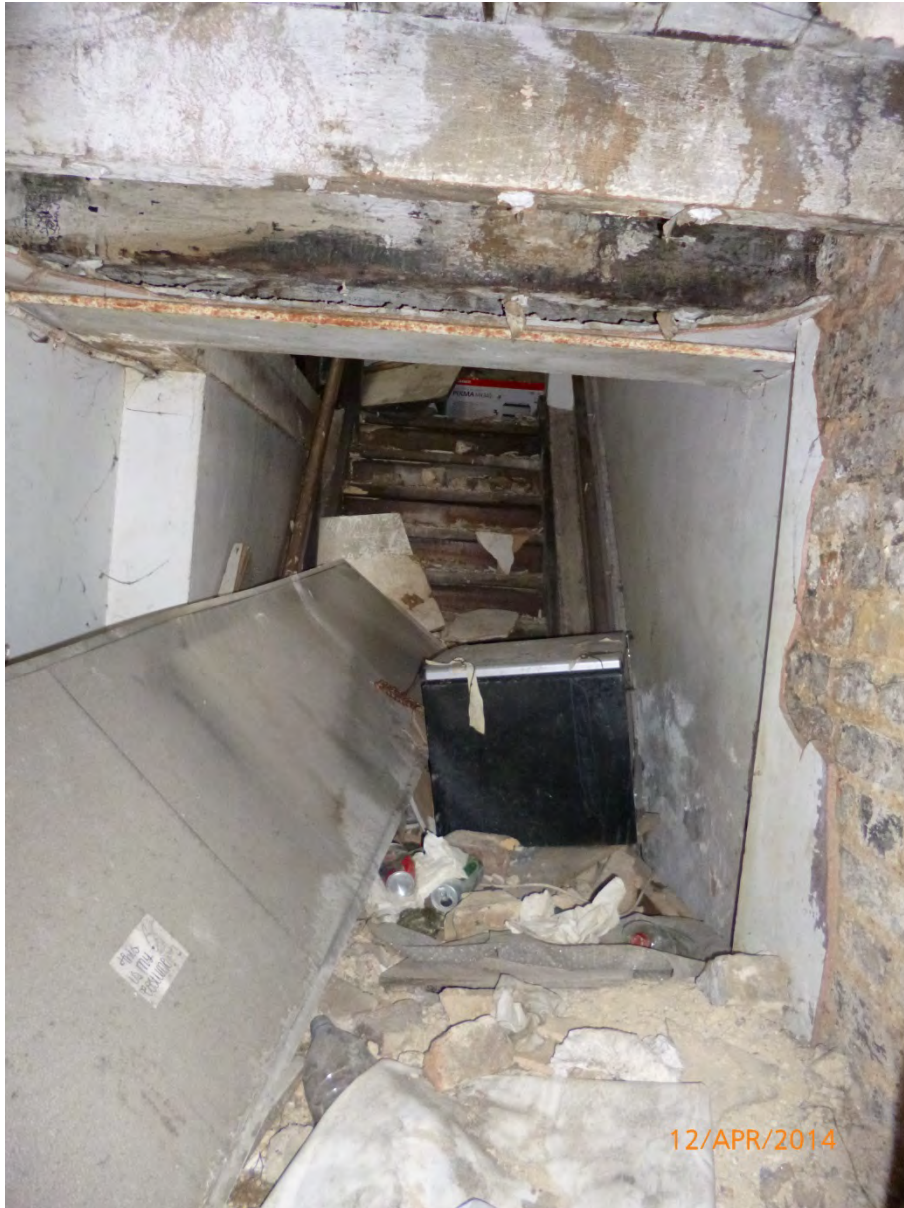
Plate 59: Staircase to first floor
