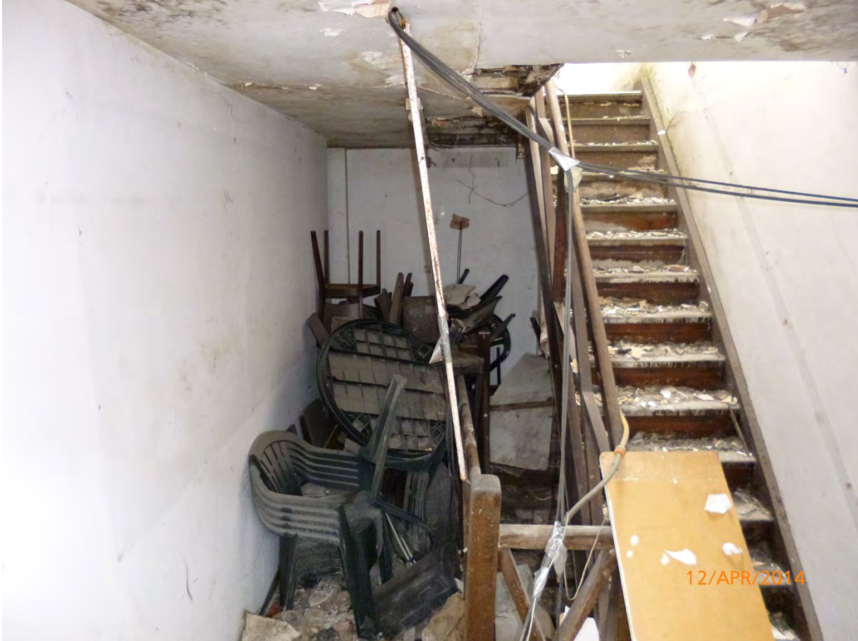
Plate 62: Staircases between floors, southern room
