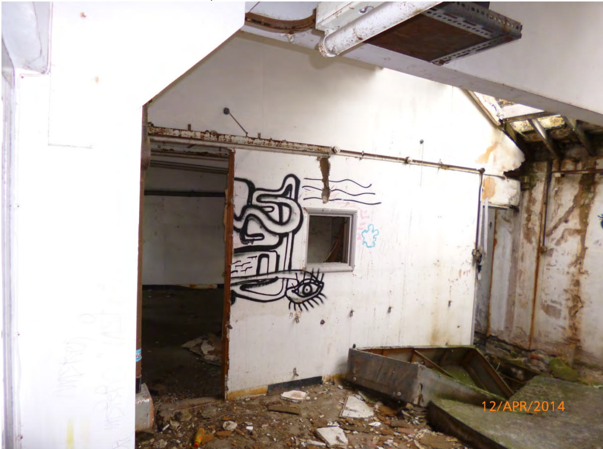
Plate 68: Detail of dividing wall, second floor
