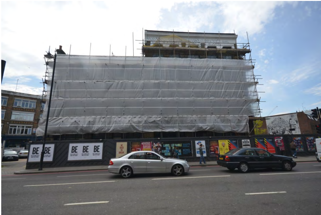
Plate 1: The facade of the building, concealed by scaffolding and hoarding
