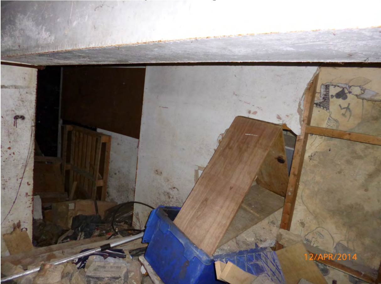
Plate 61: Ground floor, northern part of building
