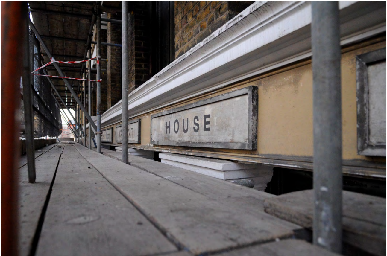
Plate 24: Detail of mouldings, facade of 63 (2011 photograph)
