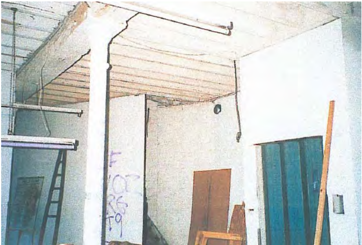
Plate 51: Southern aspect, second floor (Shaya 2000)
