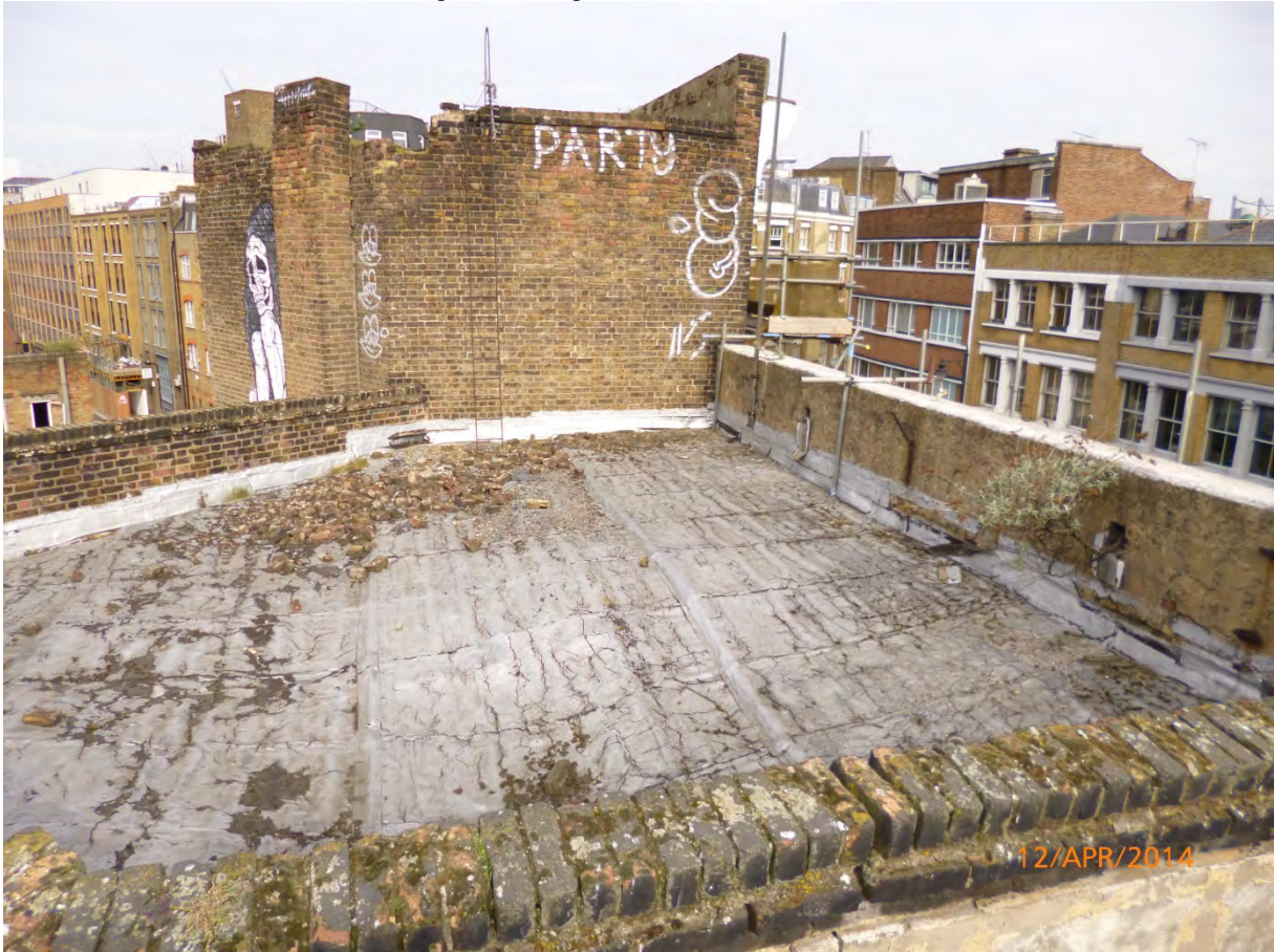
Plate 19: Roof over 61 Great Eastern Street
