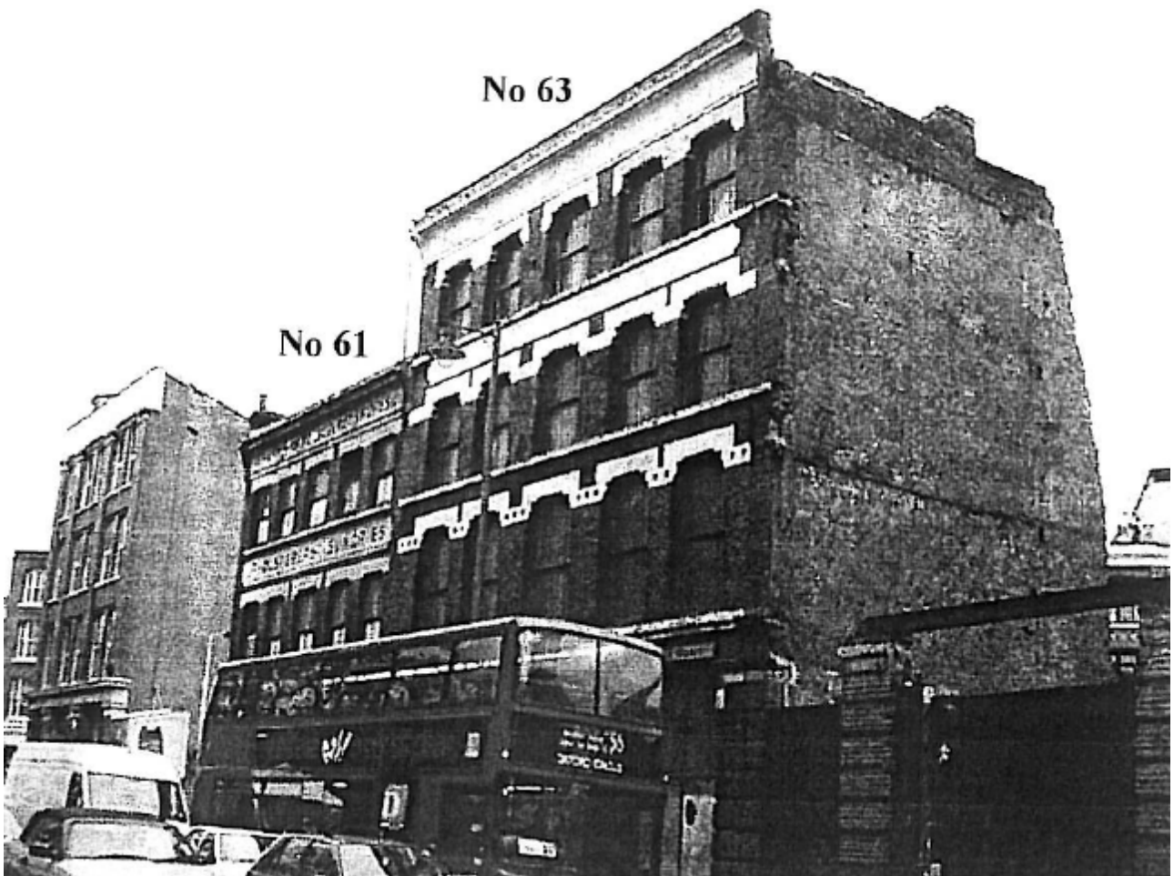
Plate 4: The building in 2000 (Shaya 2000)
