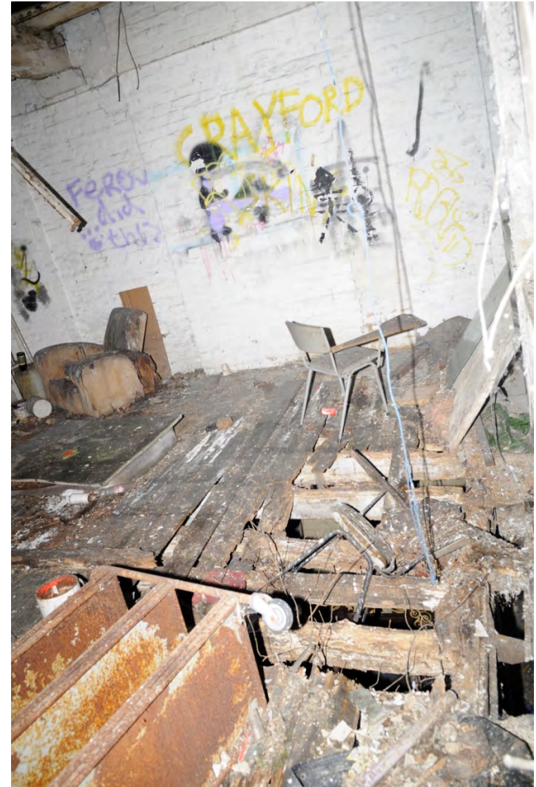
Plate 53: Detail of floor
