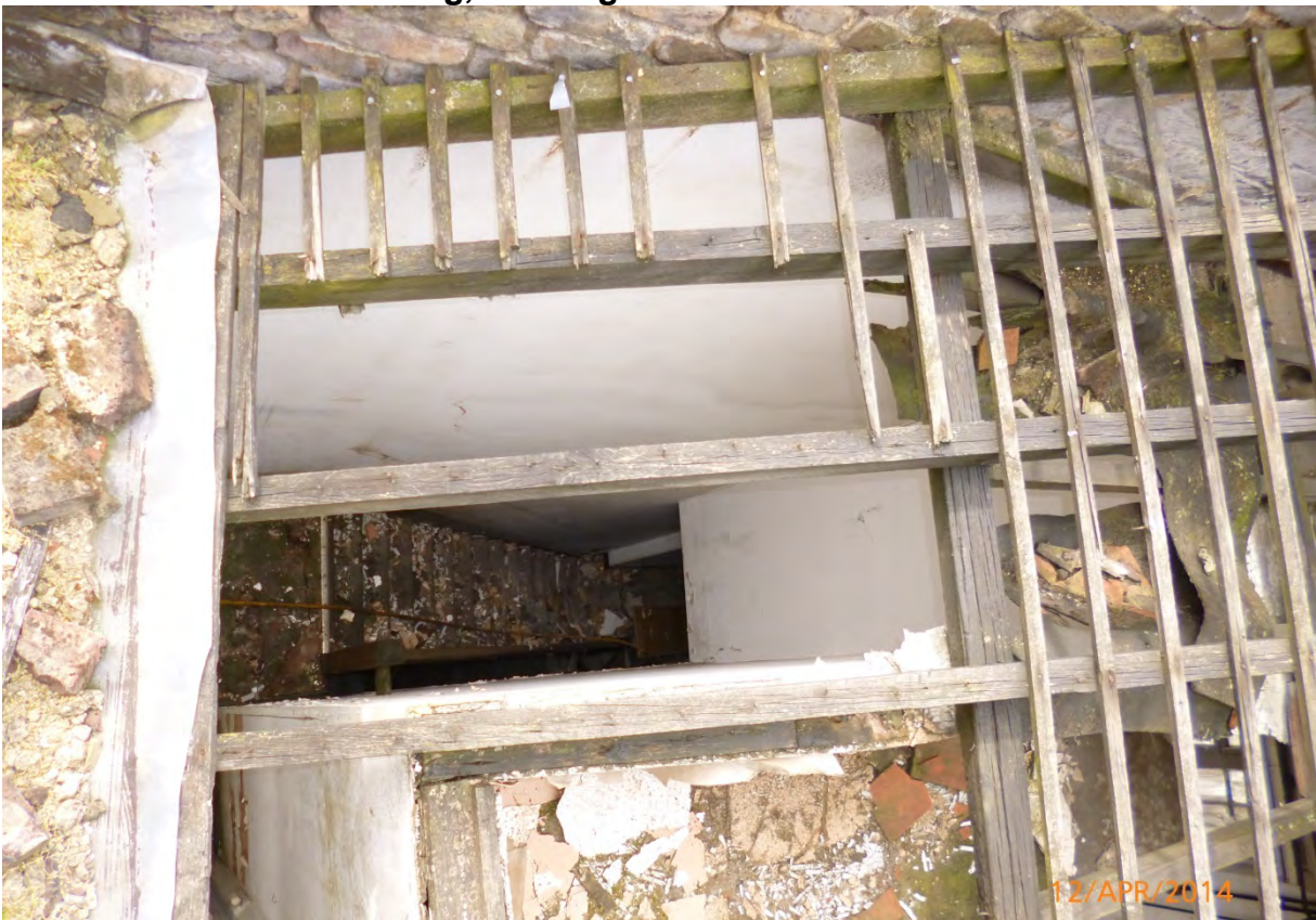
Plate 66: View of staircase from roof area
