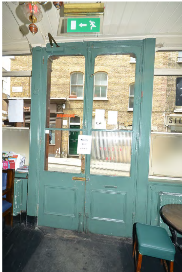
Plate 15: Double door, west wall
