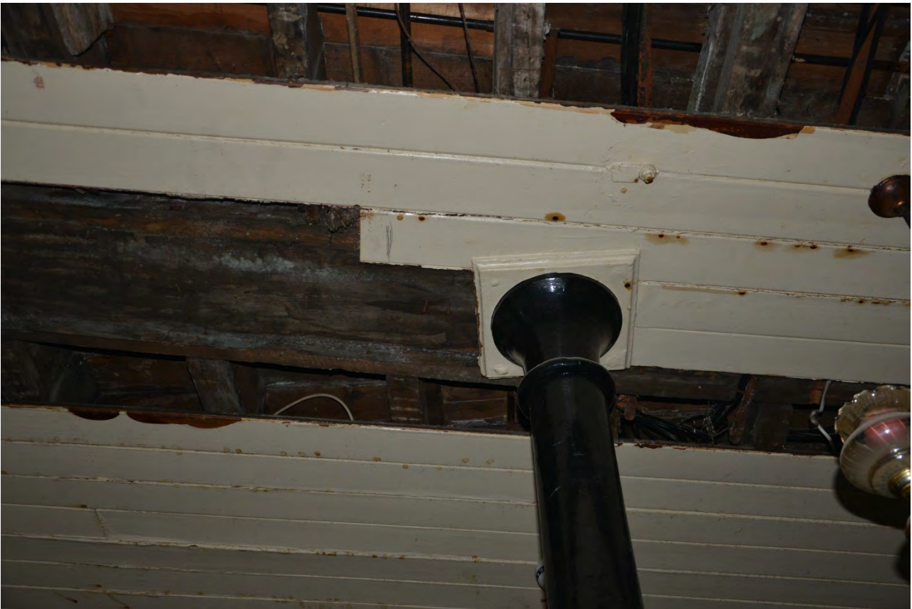
Plate 61: Exposed ceiling / first floor timbers, area B
