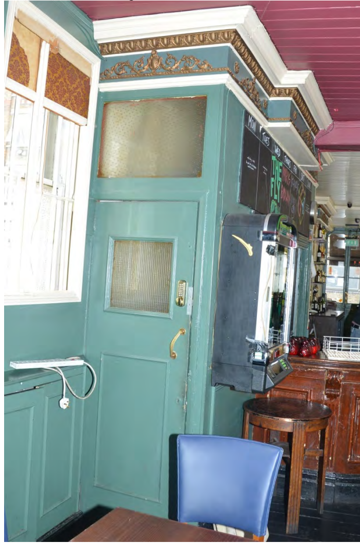
Plate 33: This door opening is to be blocked
