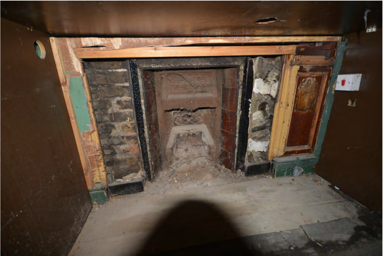
Plate 50: Fireplace revealed during strip of back bar area
