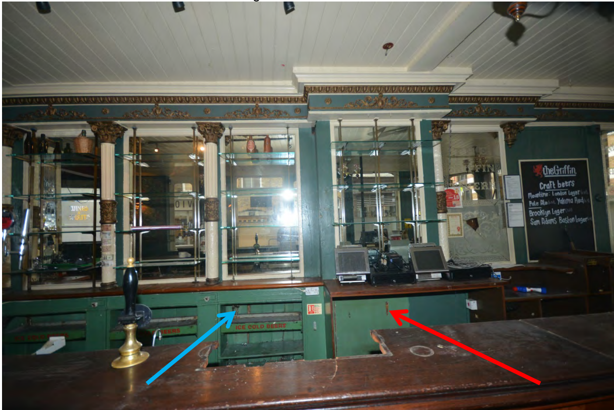
Plate 55: Location of fireplace (arrowed red) and wallpaper (arrowed blue) The above photograph clearly shows the chimneybreast leading up from the fireplace.
