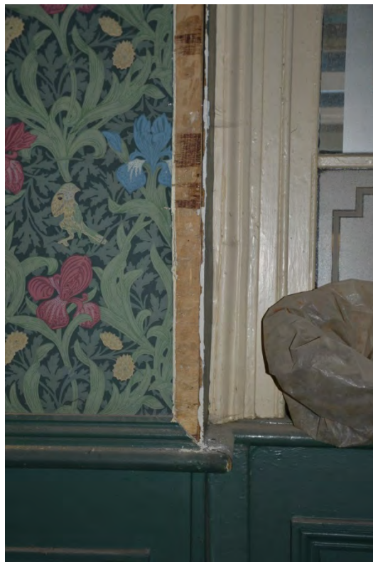
Plate 21: Modern plywood revealed during recent works
