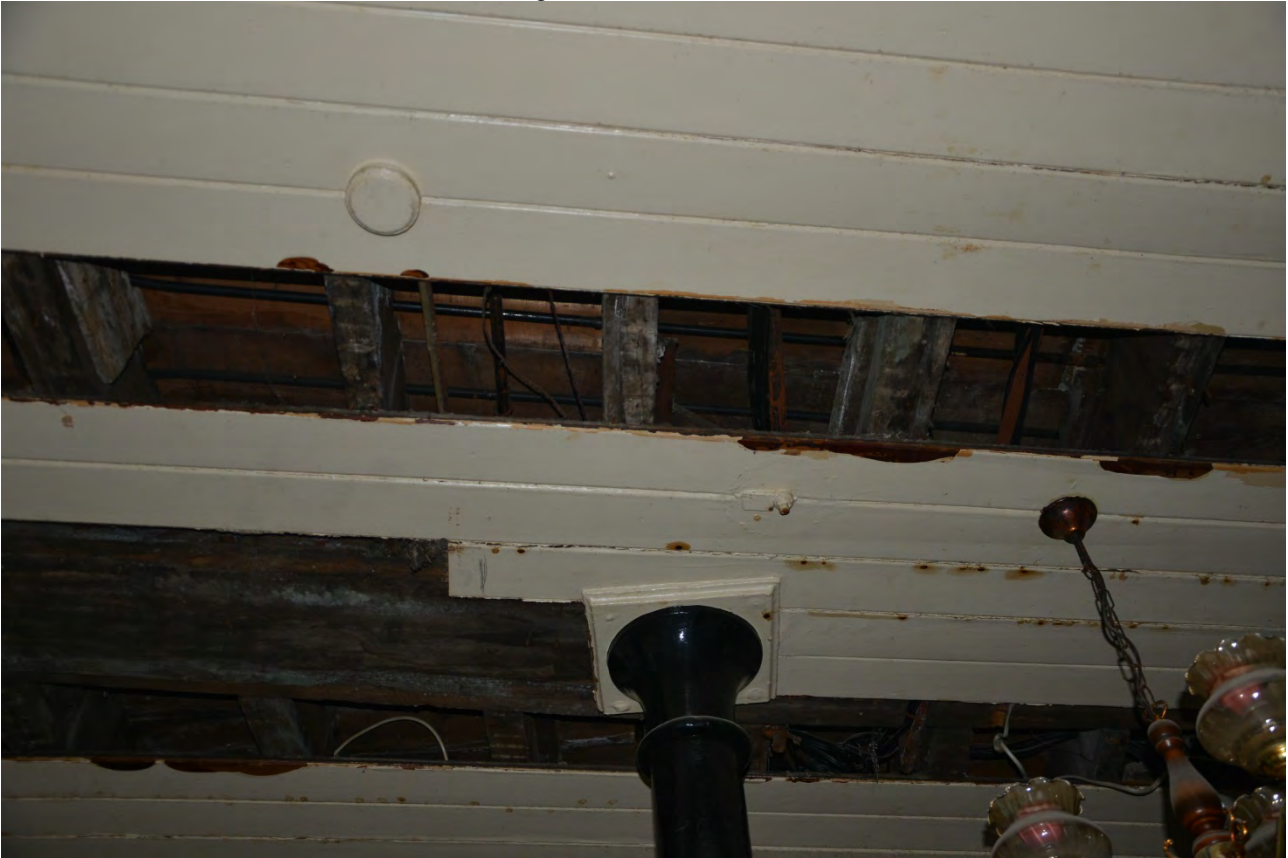
Plate 60: Exposed ceiling / first floor timbers, area B
