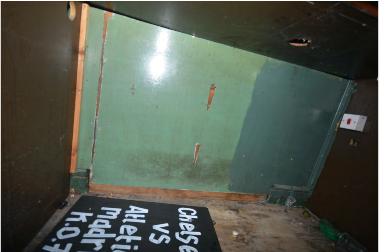
Plate 52: Former refrigerator recess showing board blocking fireplace
