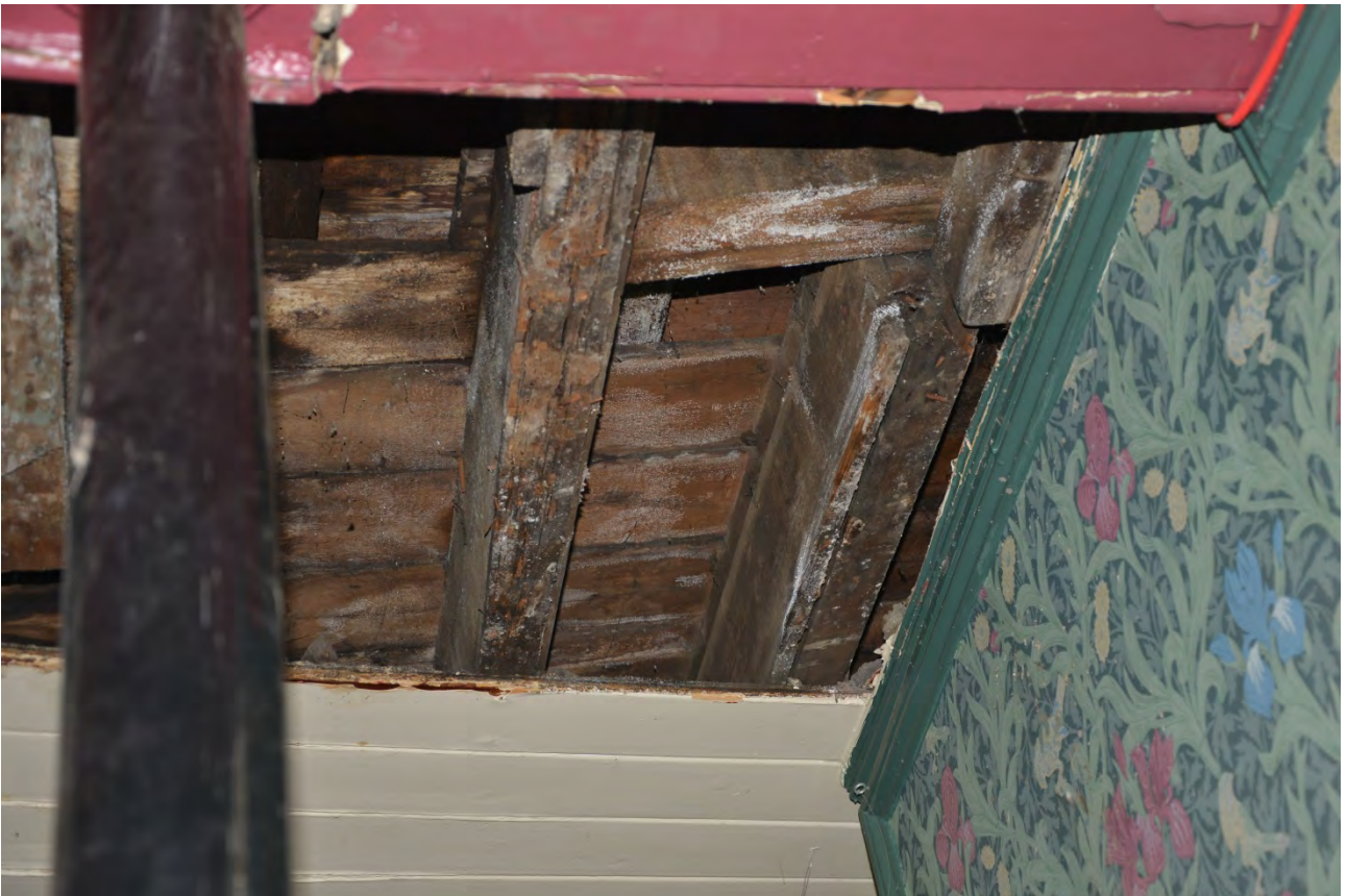
Plate 59: Exposed ceiling / first floor timbers, area A
