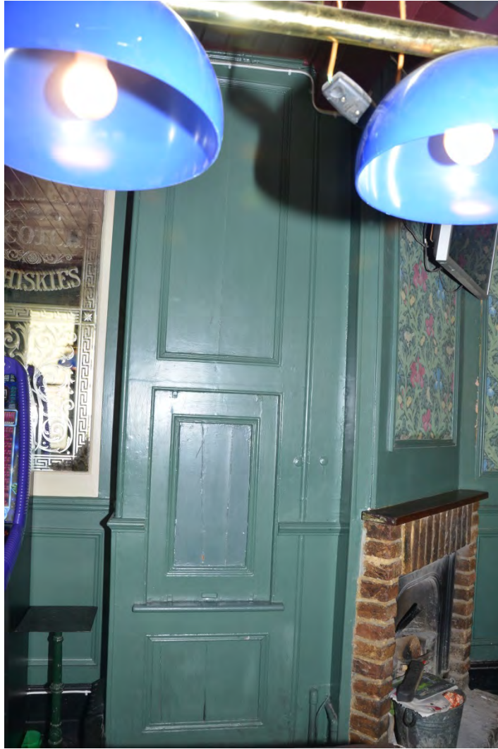
Plate 22: Panelled enclosure for the dumb waiter
