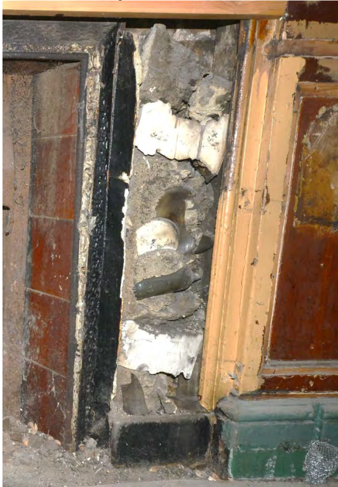
Plate 51: Detail of bottles and refuse forming right hand wall of fireplace
