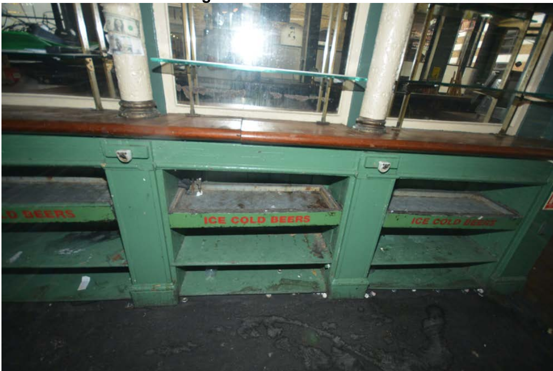
Plate 36: Detail of back bar fittings to be removed
