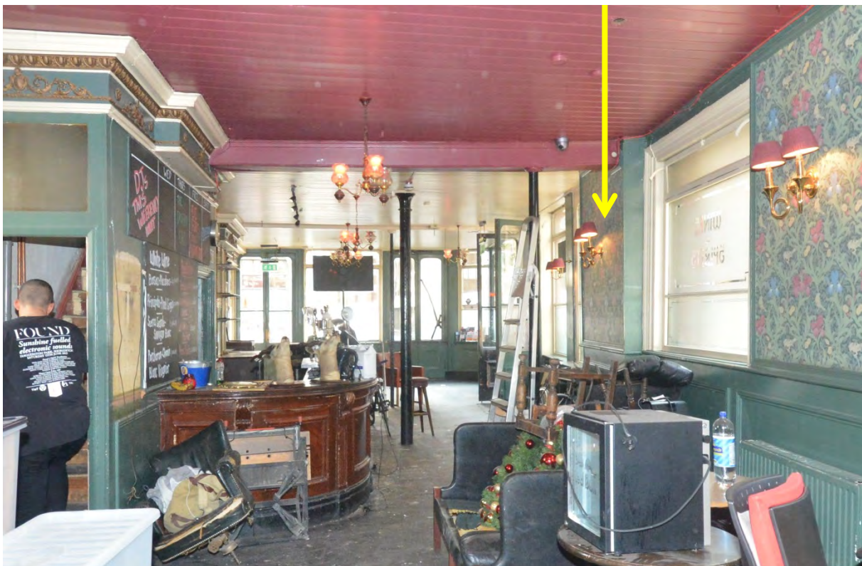
Plate 56: Location of plywood boxing (arrowed)
