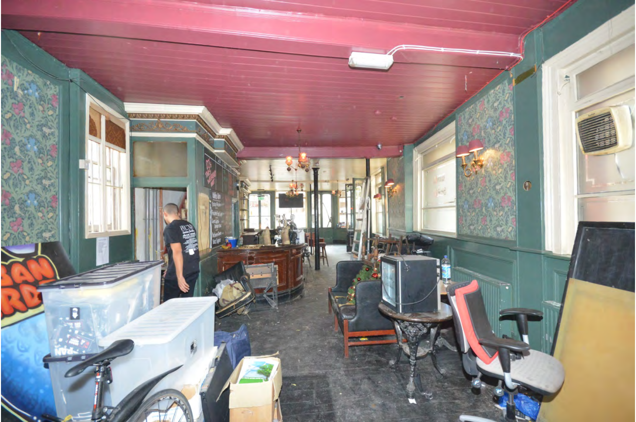
Plate 34: Timber panelled ceiling
