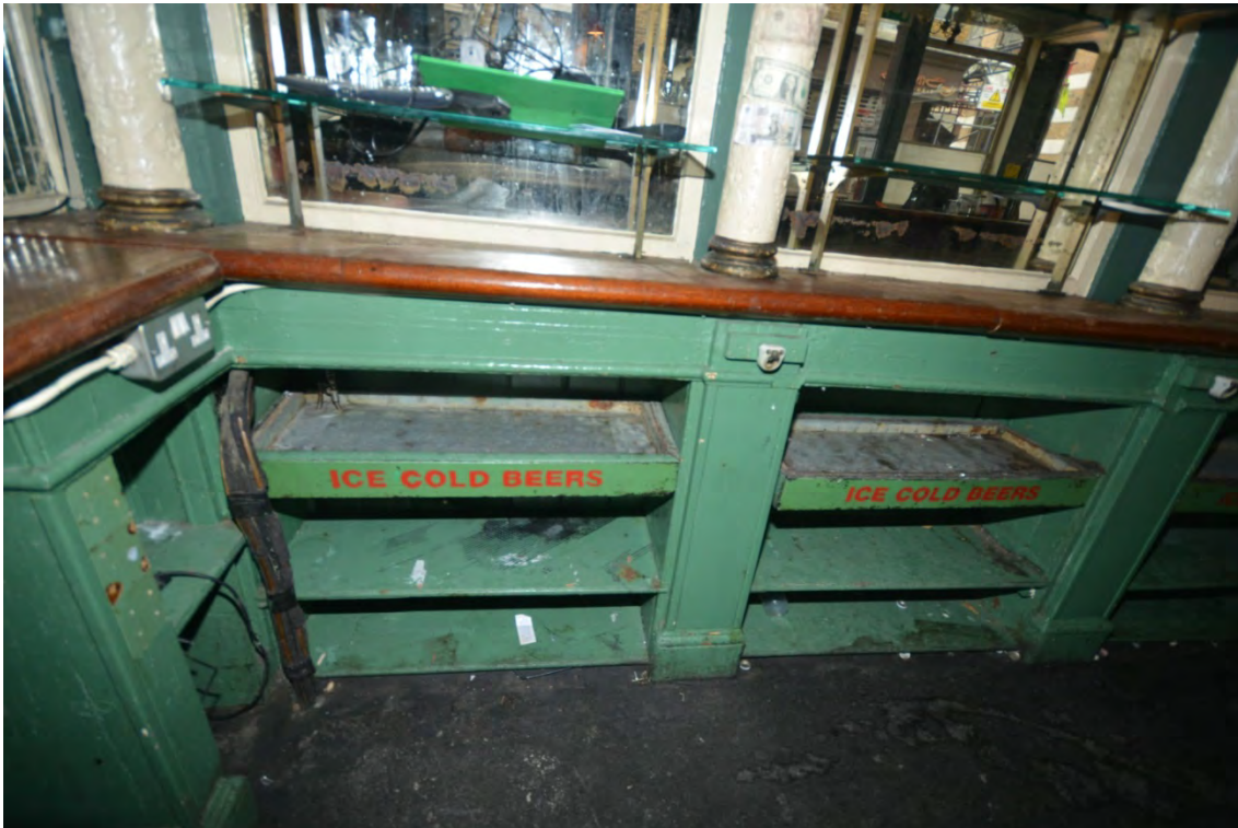
Plate 35: Detail of back bar fittings to be removed
