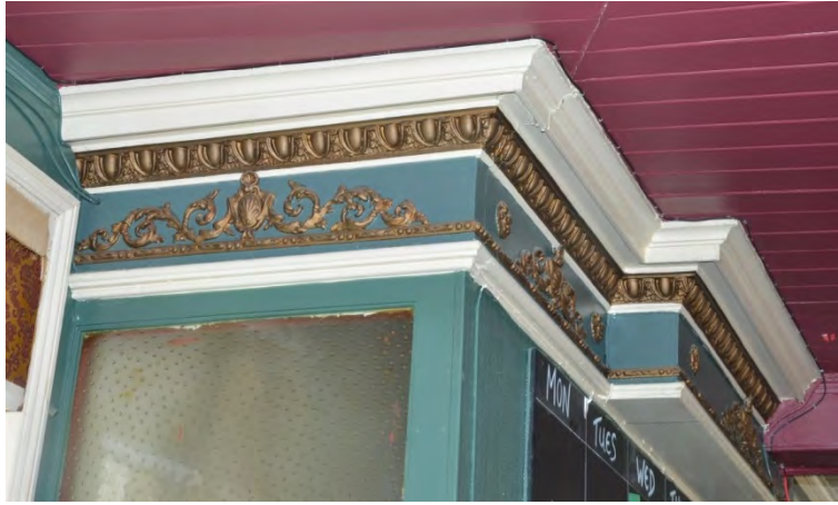
Plate 6: Cornice and moulding, east wall
