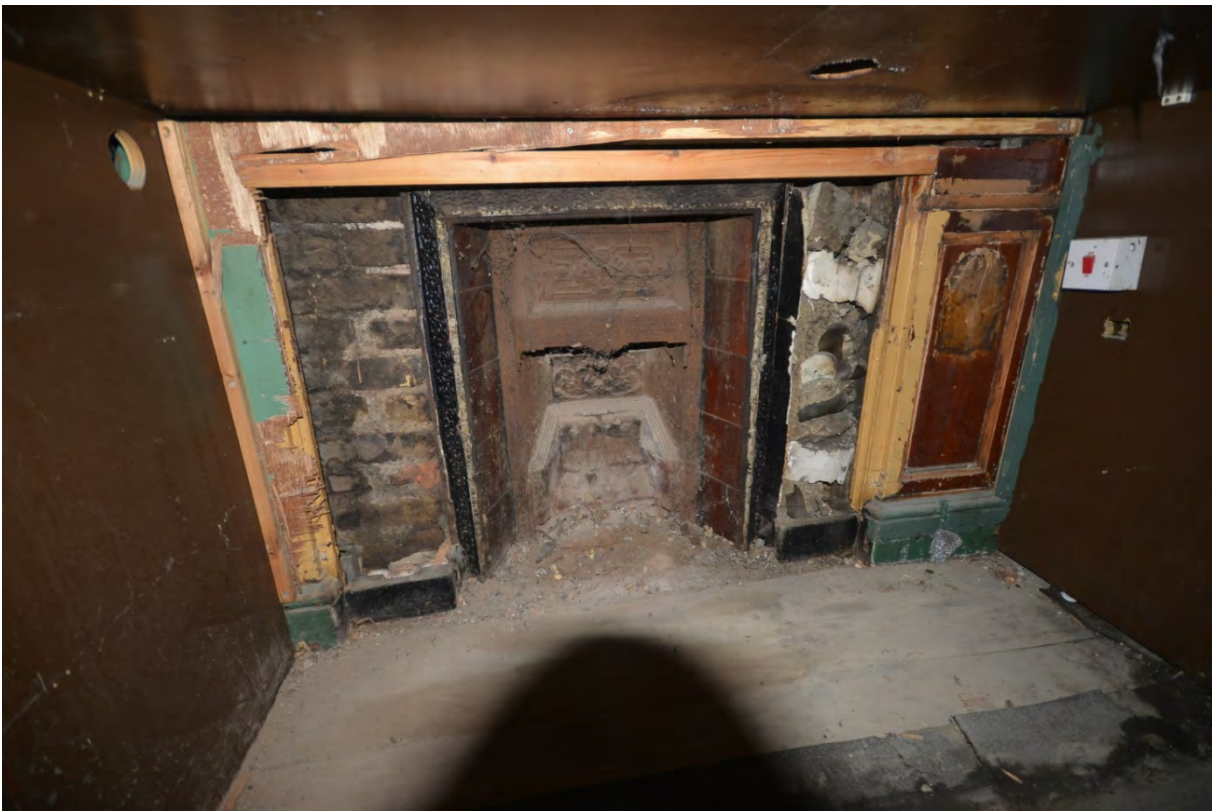
Plate 30: Fireplace revealed during strip of back bar area
