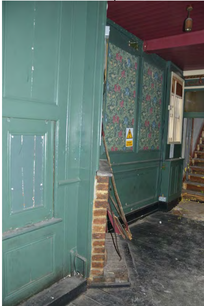
Plate 49: Panelling and walls to be refurbished
