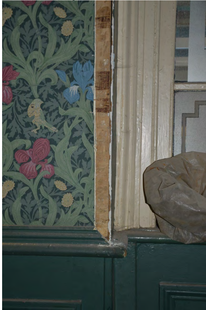
Plate 57: Plywood boxing in of soil pipe
