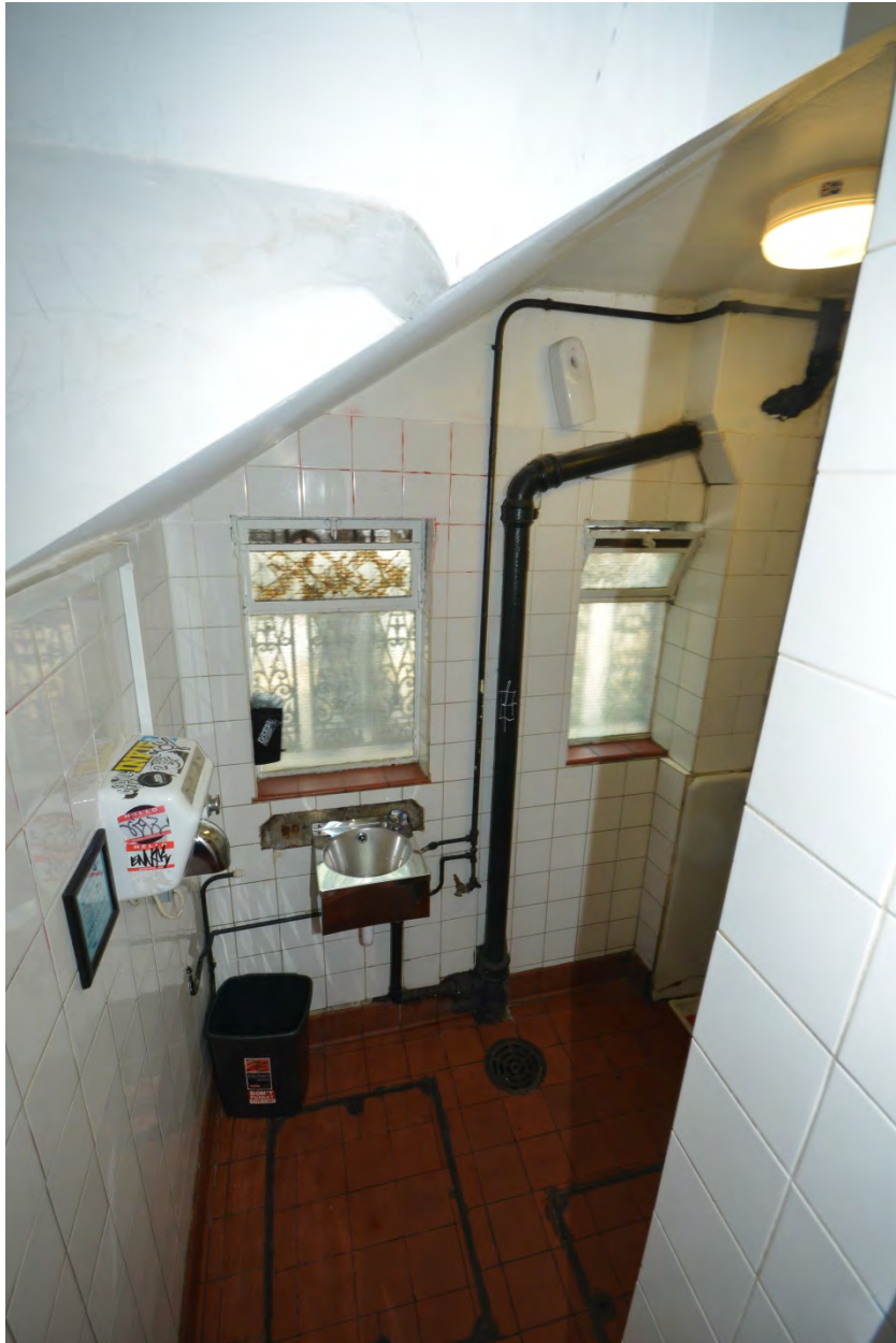
Plate 43: View into gents' lavatory
