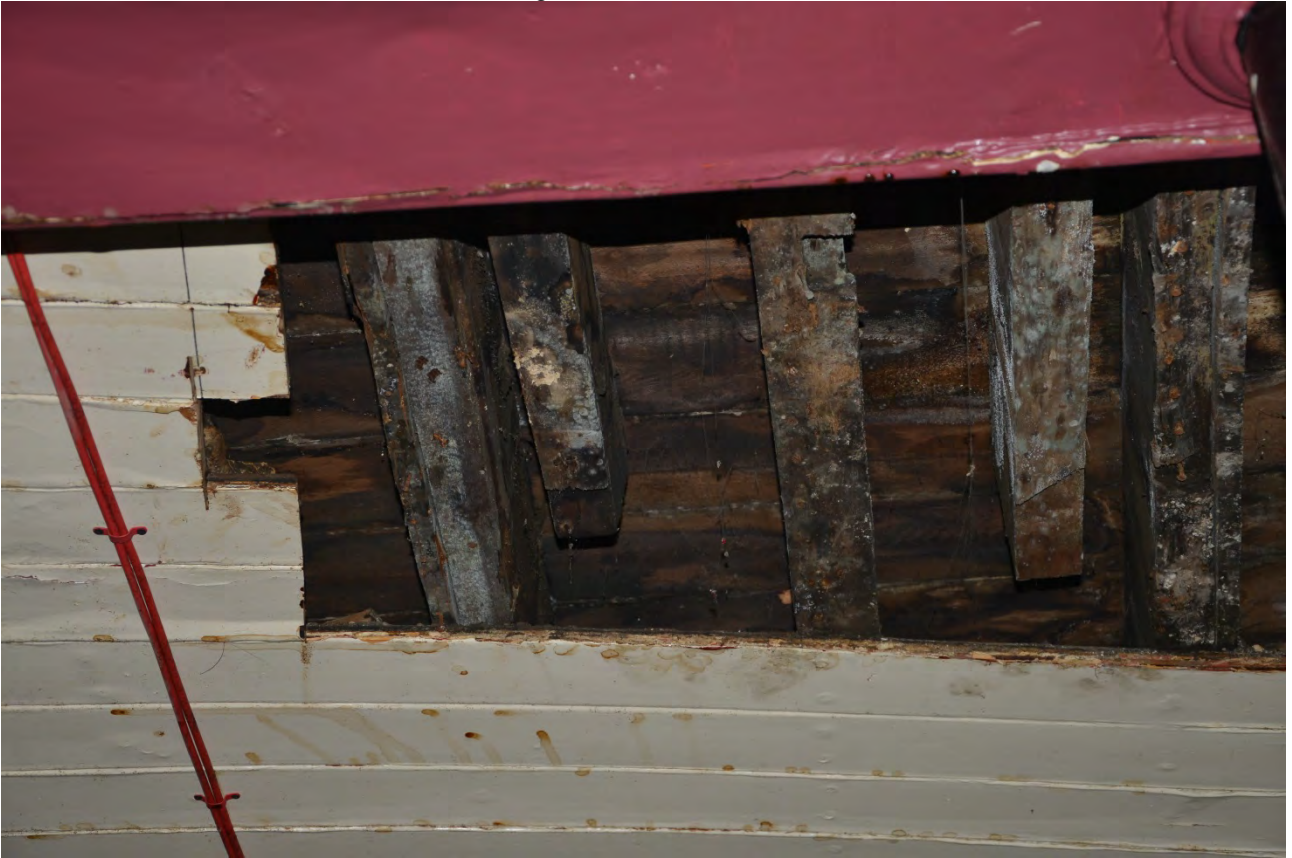
Plate 58: Exposed ceiling / first floor timbers, area A
