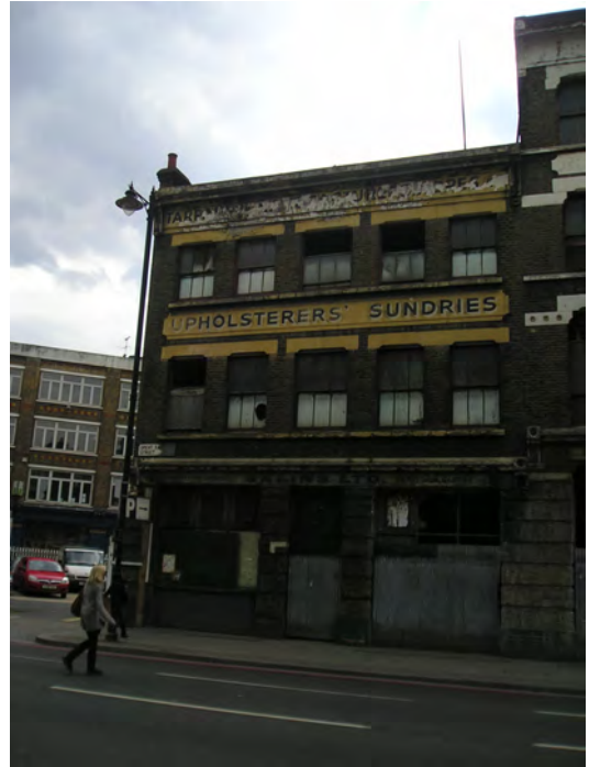
DP 2- 61 Great Eastern Street, looking south-west.
