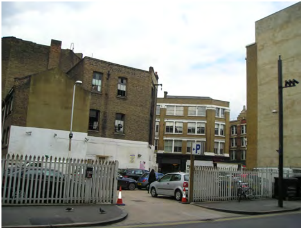
DP 7- View of 95 Leonard Street looking north
