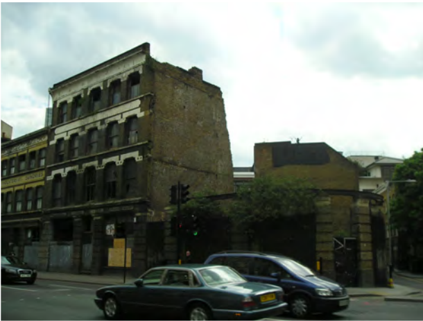
DP 3- 61-65 Great Eastern Street looking south-east
