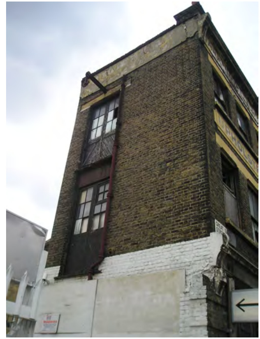
DP 6- Gable end of 61 Great Eastern Street showing hoist. Looking north-west
