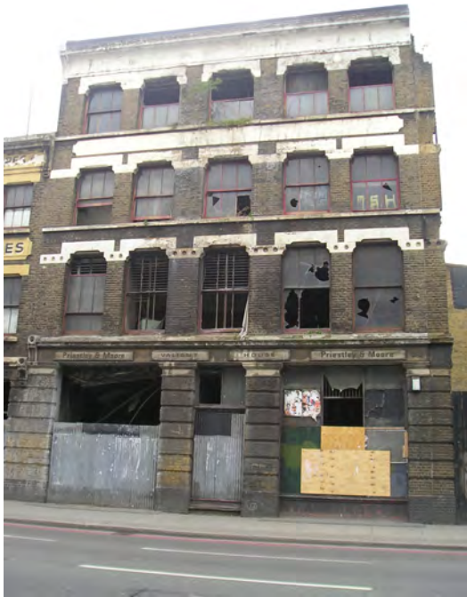
DP 1- 63 Great Eastern Street, looking south-west.
