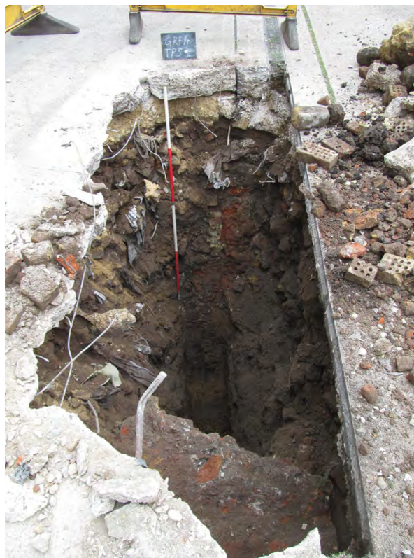
Plate 10: TP.5 – general overview, looking east
