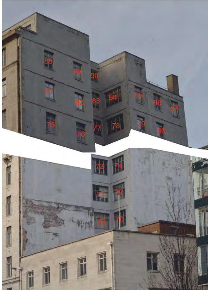
Figure 7: Window locations, south face
