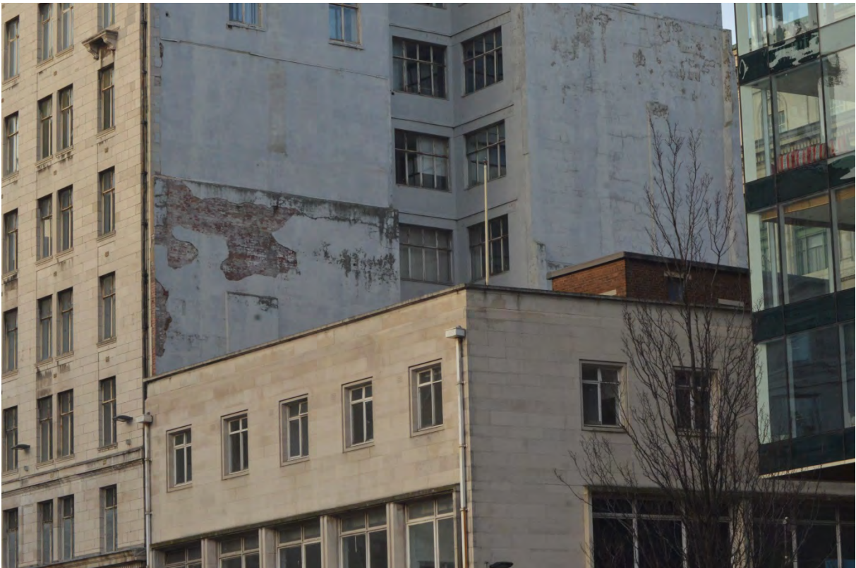
Plate 17: Lower part, southern elevation
