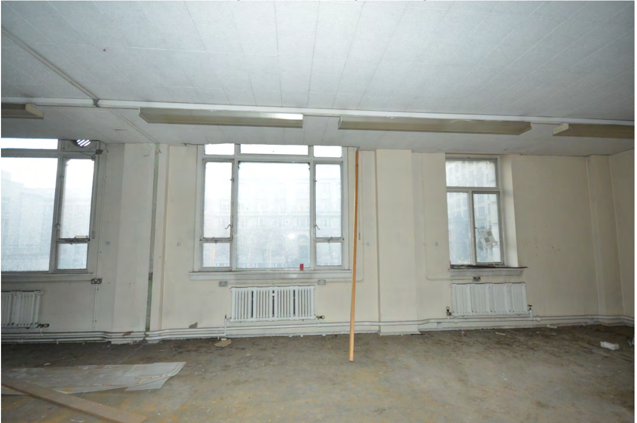
Plate 26: Detail of first floor windows
