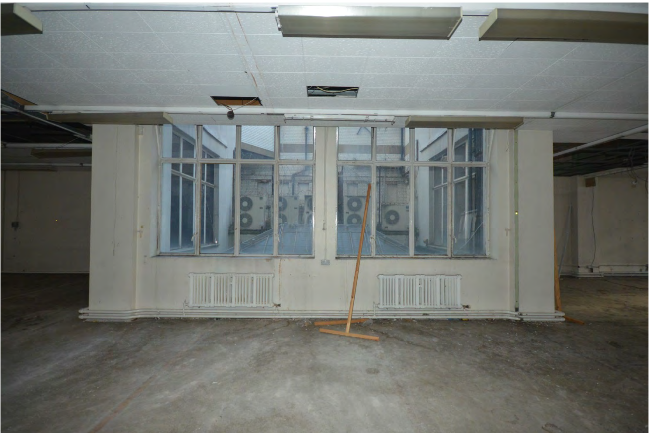
Plate 25: View into light well
