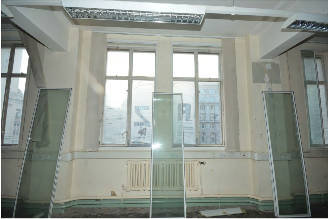
Plate 30: Detail of second floor windows
