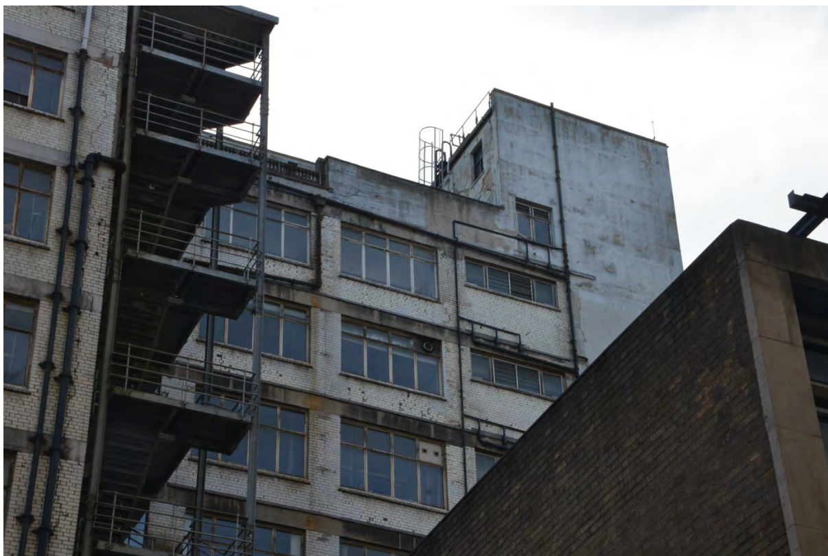
Plate 21: North end, east elevation
