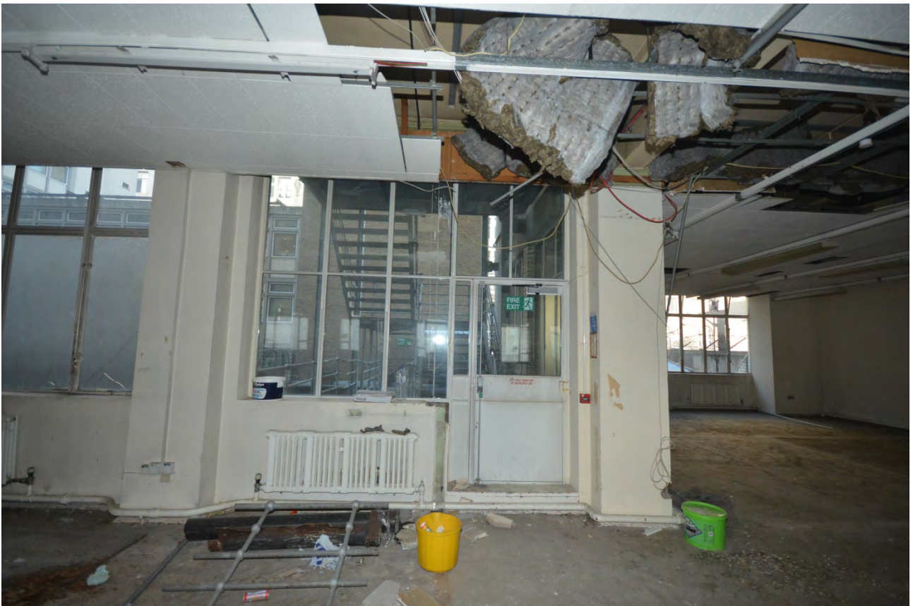
Plate 27: Detail of fire escape to rear of building
