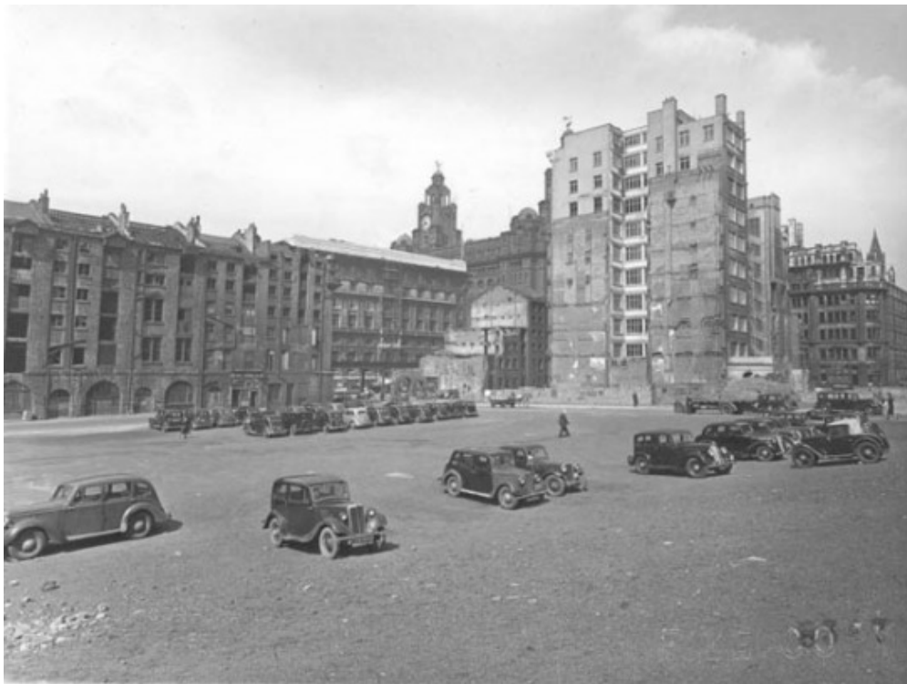
Plate 5: 1946 View of the building looking west from the car park situated on Brunswick Street
