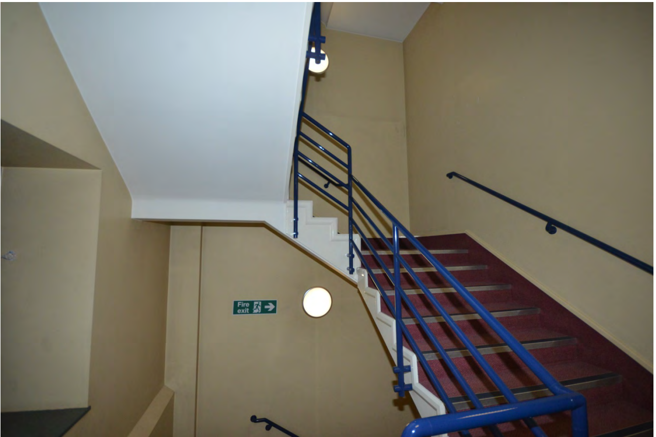
Plate 33: Detail of staircase
