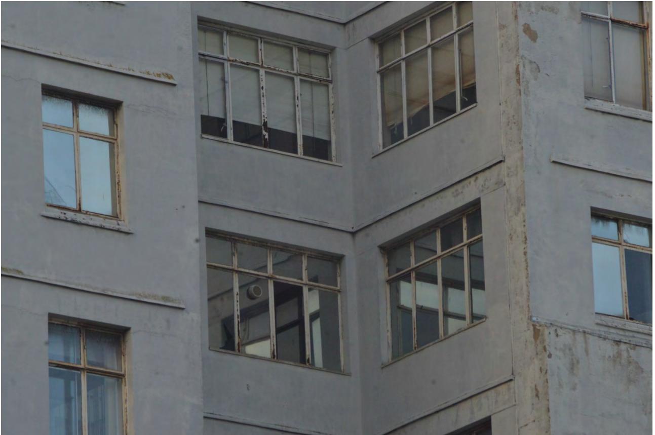
Plate 18: Detail of windows, southern elevation
