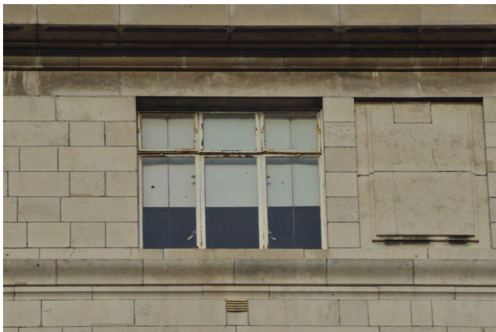
Plate 12: Window and sunken panel
