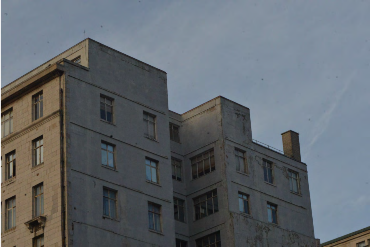
Plate 16: Upper part, southern elevation
