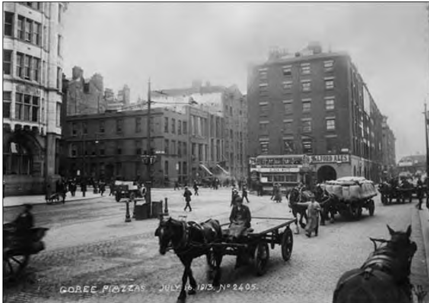
Plate 2: View towards the position of Wellington Buildings, 1913
