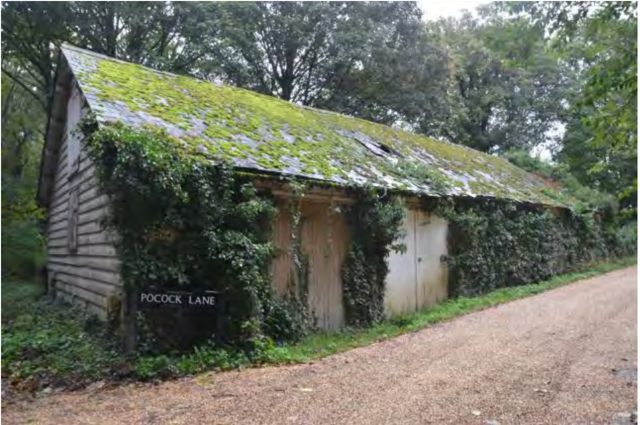
Plate 10 Recent Building Pocock Lane
