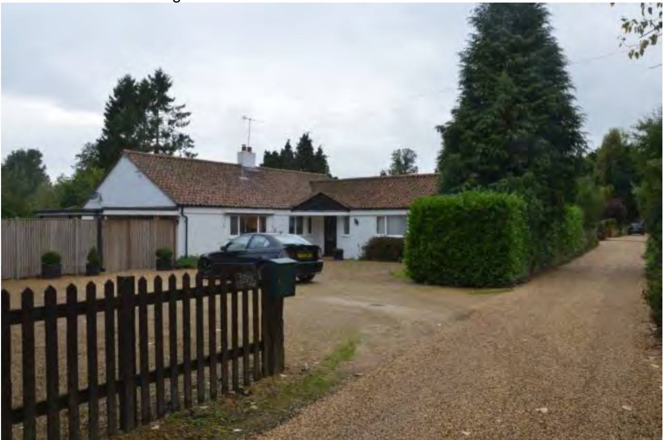
Plate 11 Recent Building Pocock Lane
