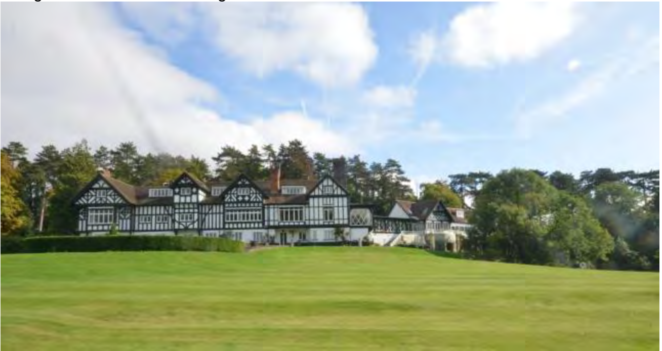
Plate 14 The Springs Hotel rear elevation
