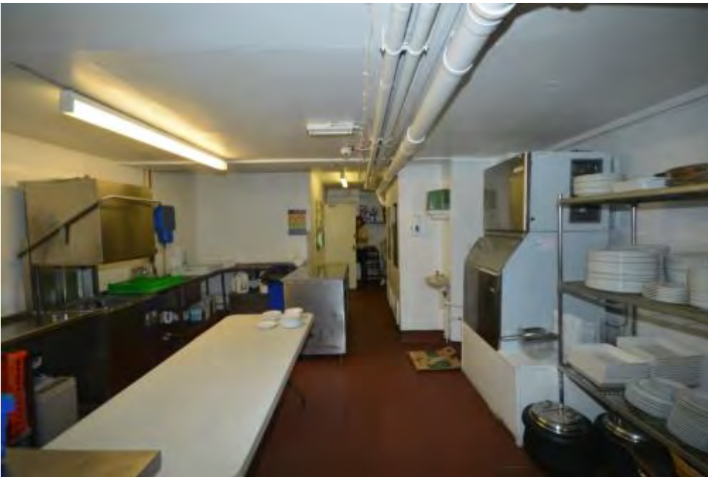
Plate 27: General view, kitchen wing
