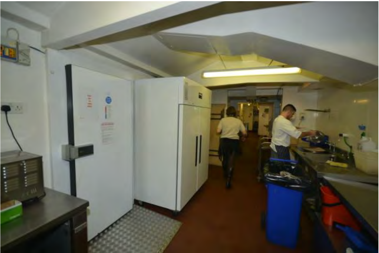
Plate 25: General view, kitchen wing
