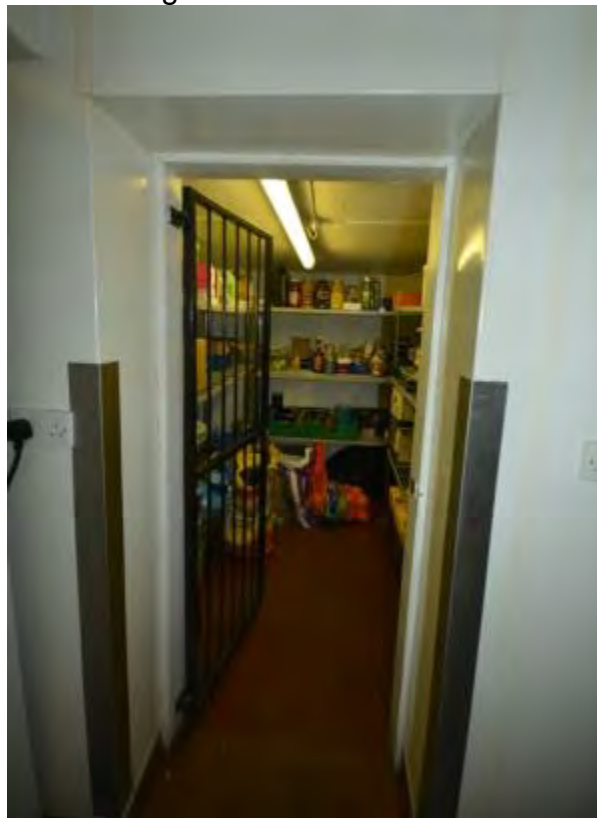
Plate 26: General view, kitchen wing
