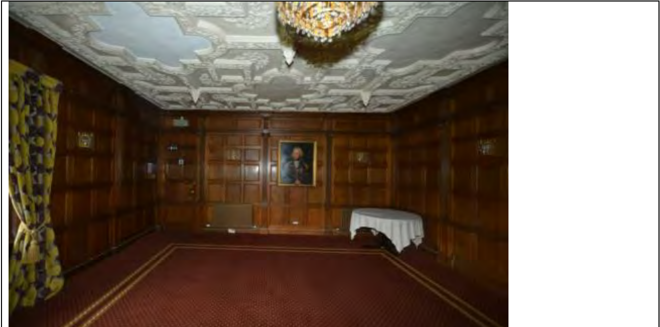
Plate 74: Ground Floor Room 3 Looking North
