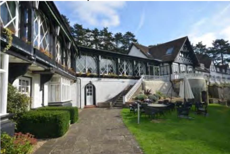
Plate 13: West elevation where north wing (left) joins Lakeside wing (right)
