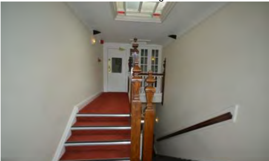
Plate 114: First Floor Room 1 Looking West
