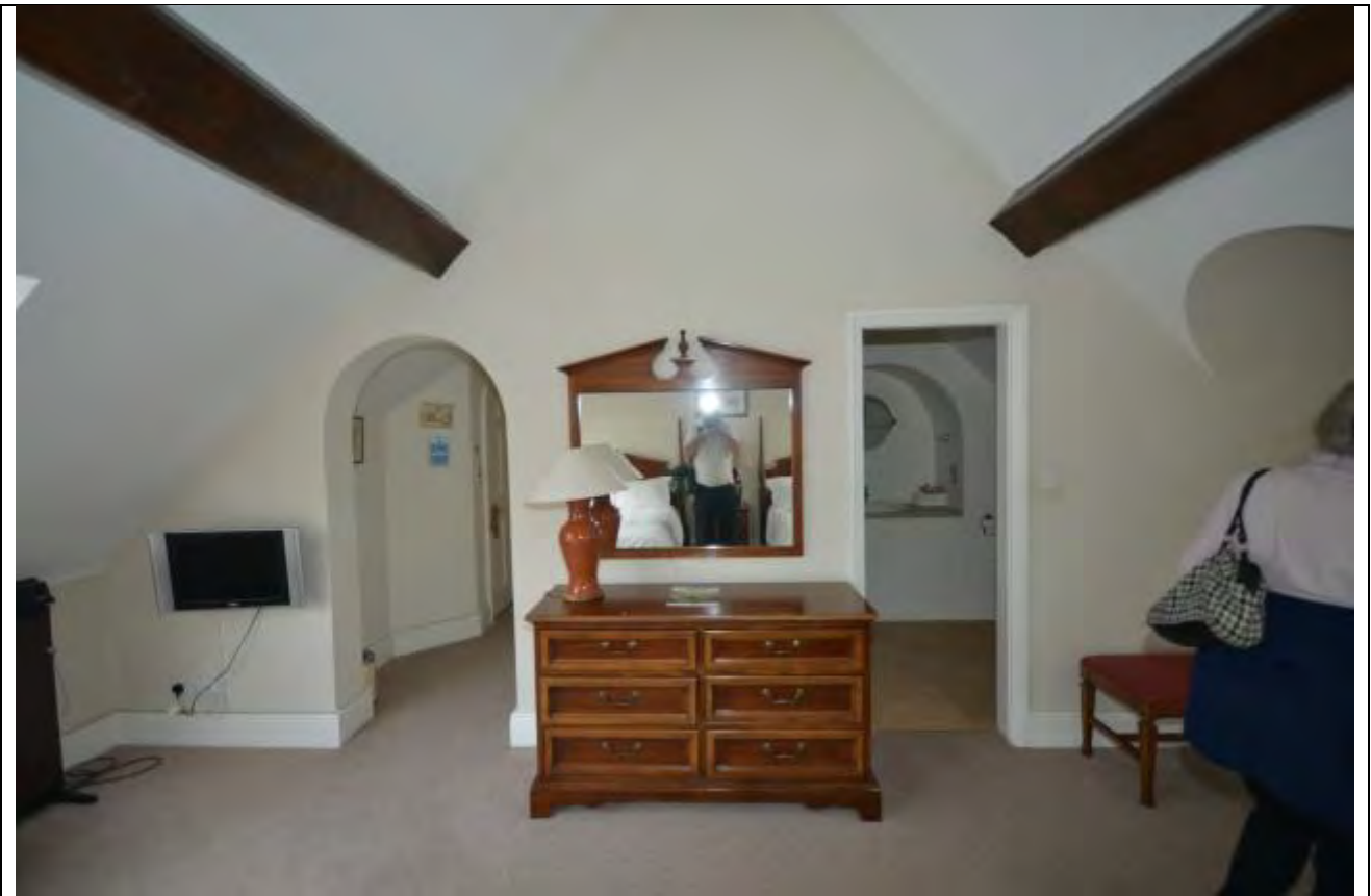
Plate 208: First Floor Room 6 Looking South
