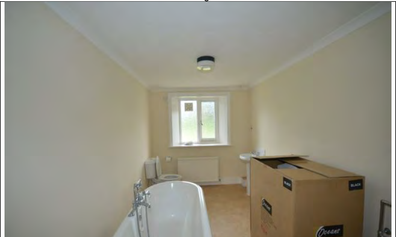
Plate 64: Lower Ground Floor Room 12 Looking West
