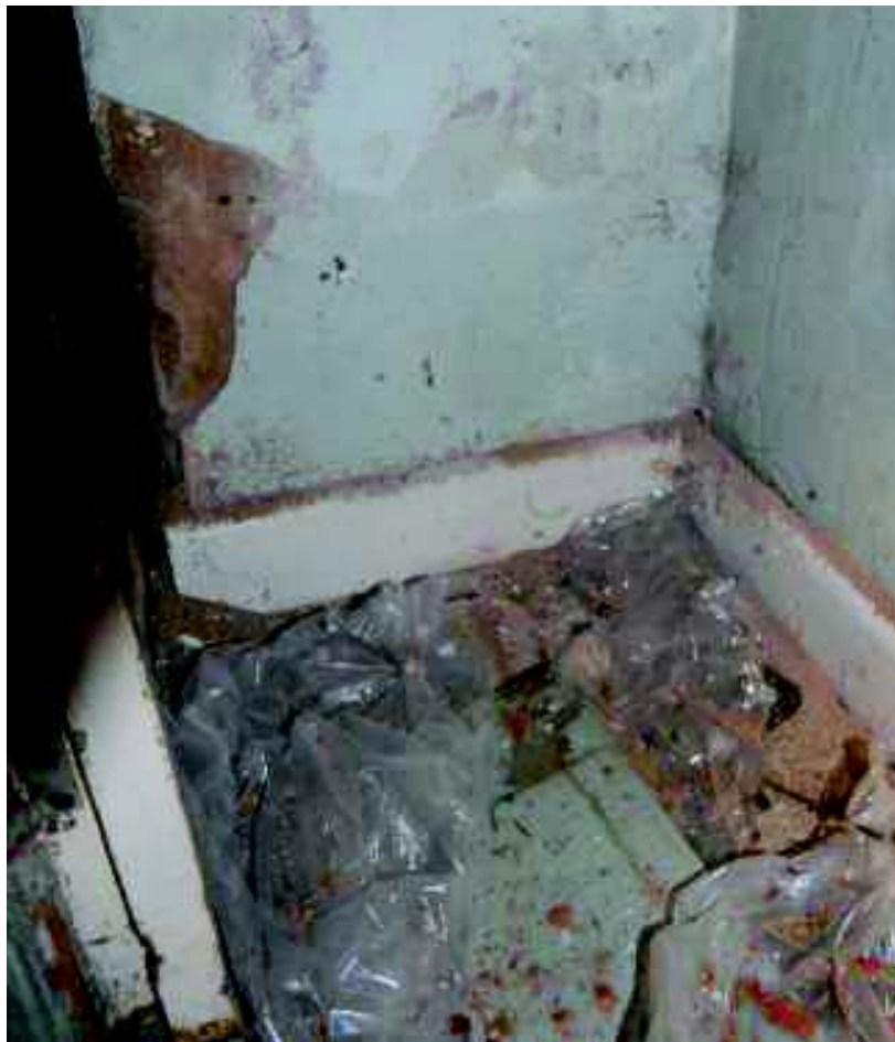
Plate 13: Detail of skirting, cupboard
