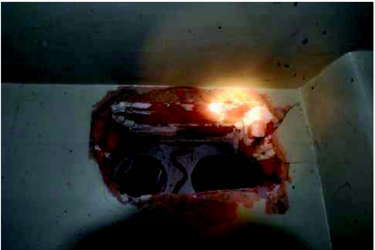
Plate 11: Detail of air vents, cupboard
