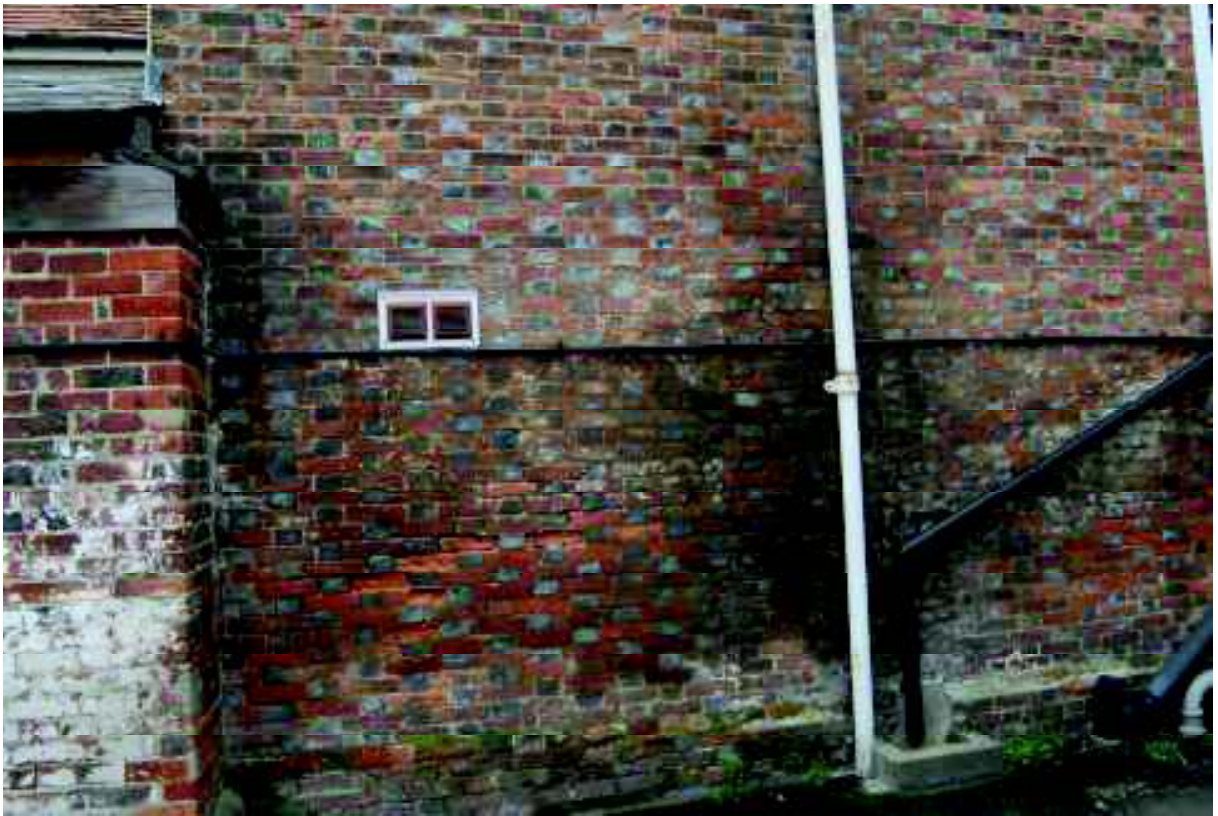
Plate 12: Reverse of wall showing area of blocked window (surrounding air vents)
