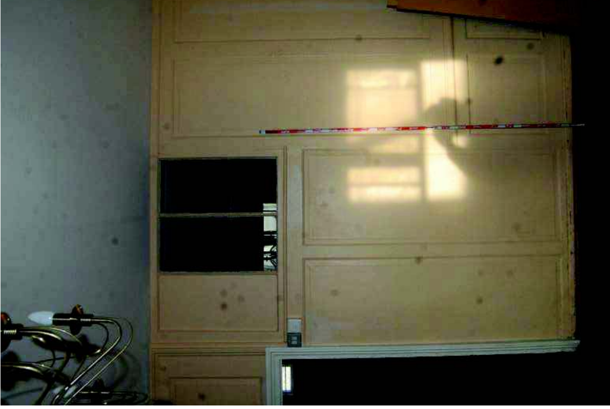
Plate 7: 'Secondary panelling' east of doorway
