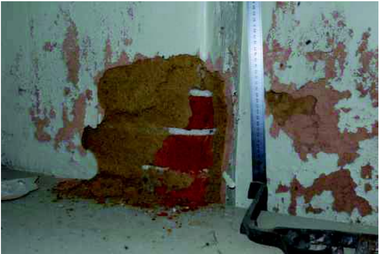
Plate 10: Detail of exposed brickwork, cupboard
