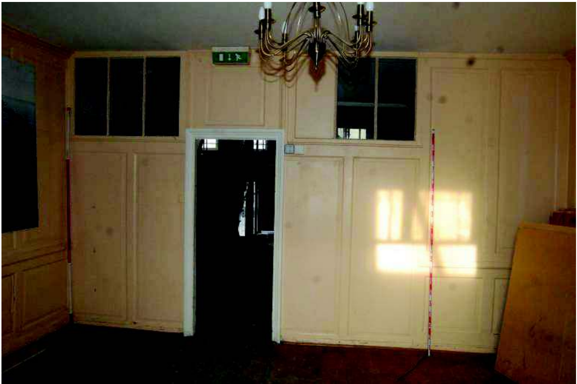
Plate 2: Northern elevation, panellled room
