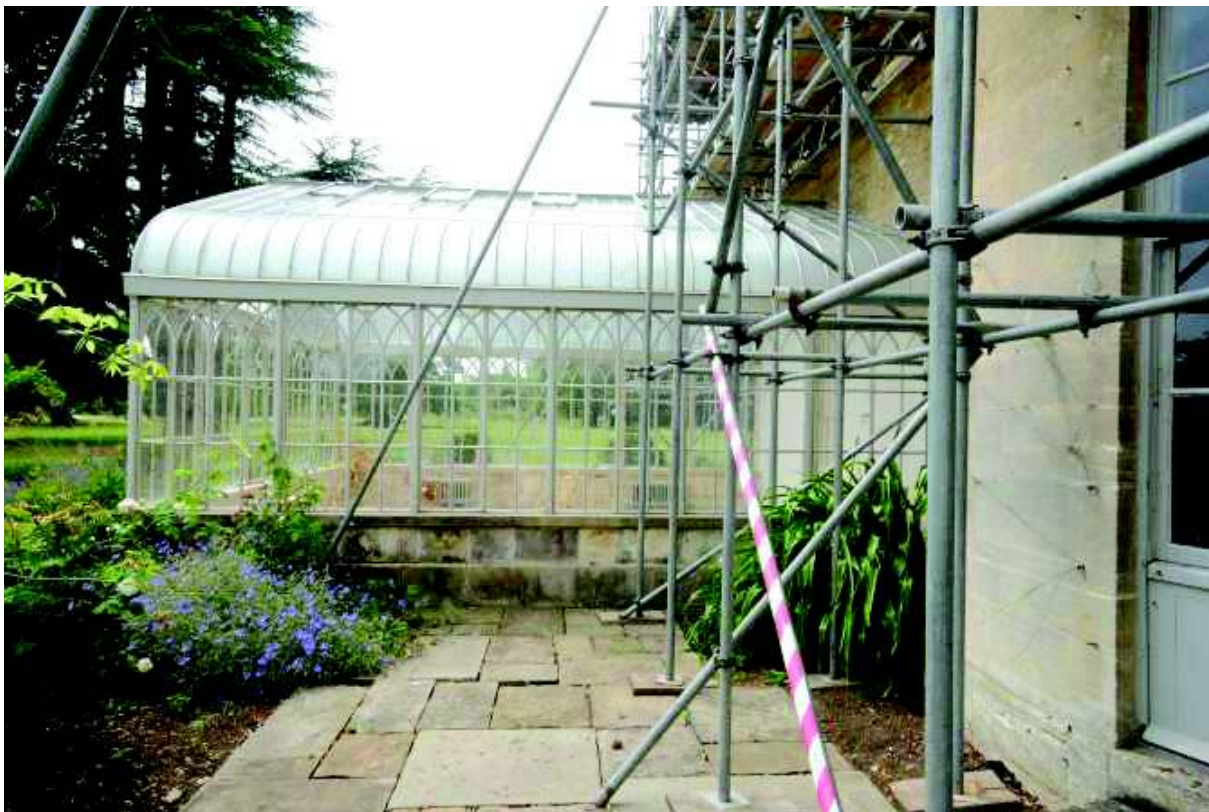
Plate 13: Conservatory viewed from the northeast
