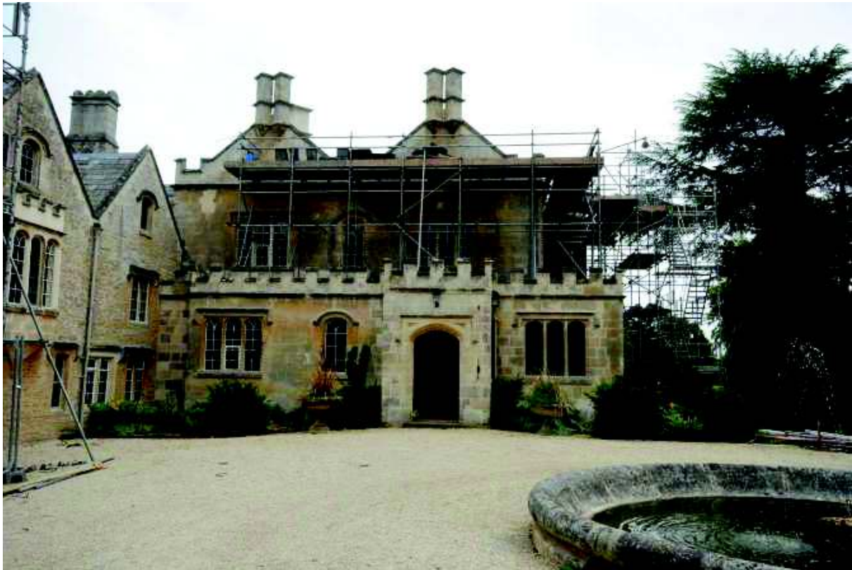
Plate 8: Northwest elevation, southwest wing
