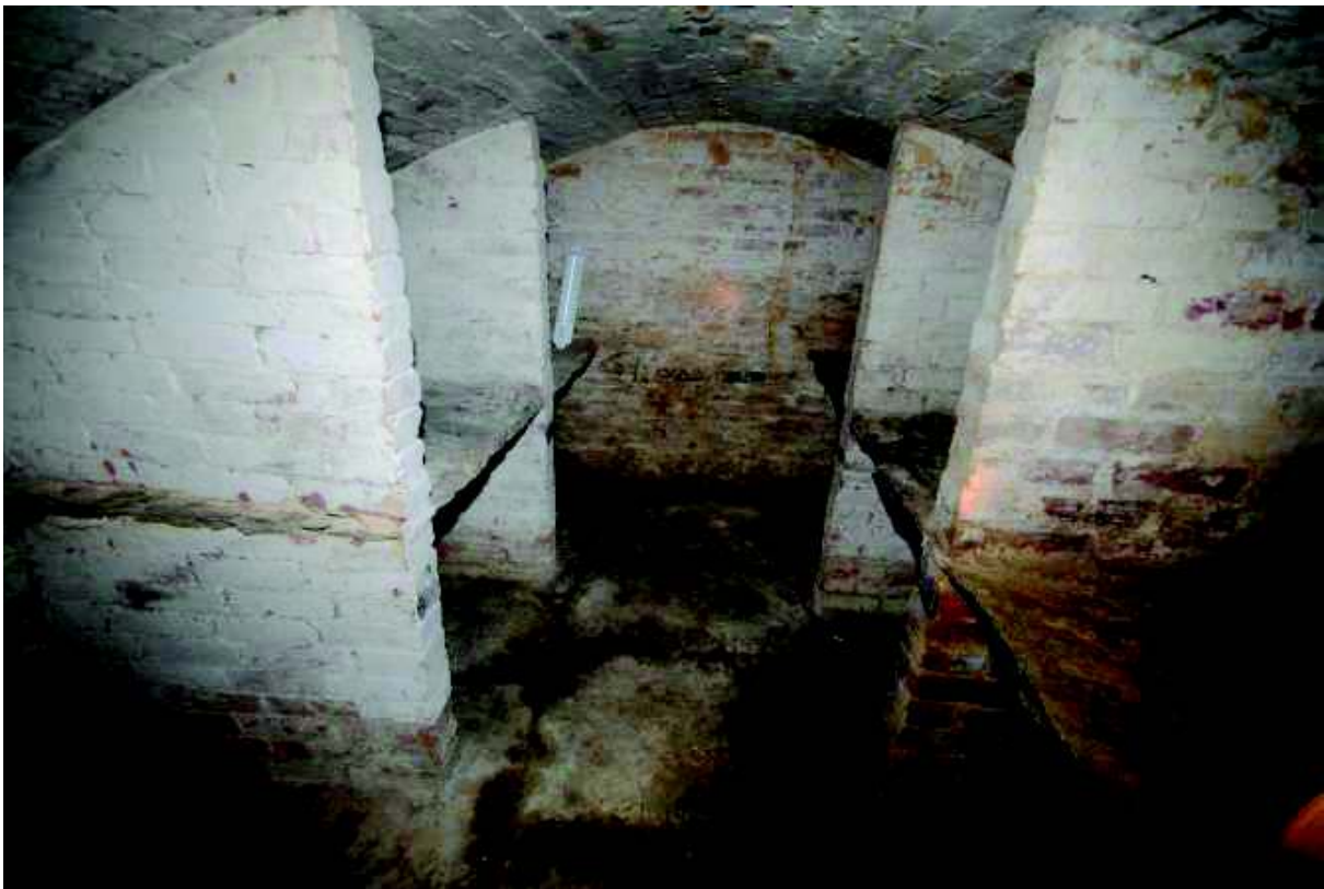
Figure 7: Northwest room viewed from northeast
