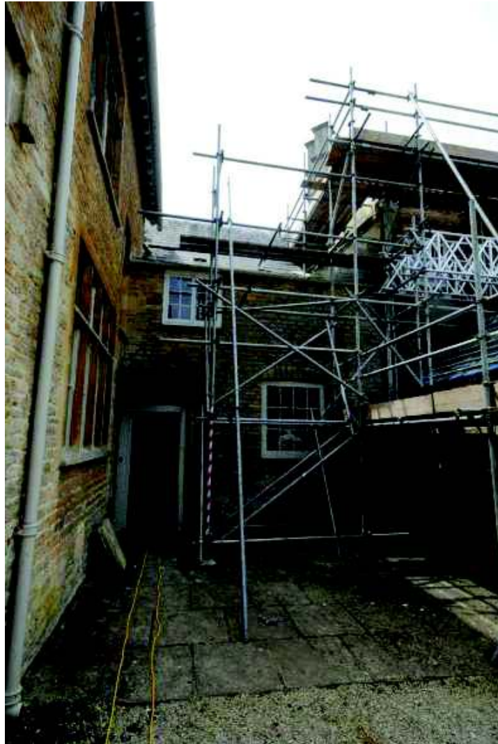
Plate 2: Recessed area to southeast of northeast elevation, northwest wing
