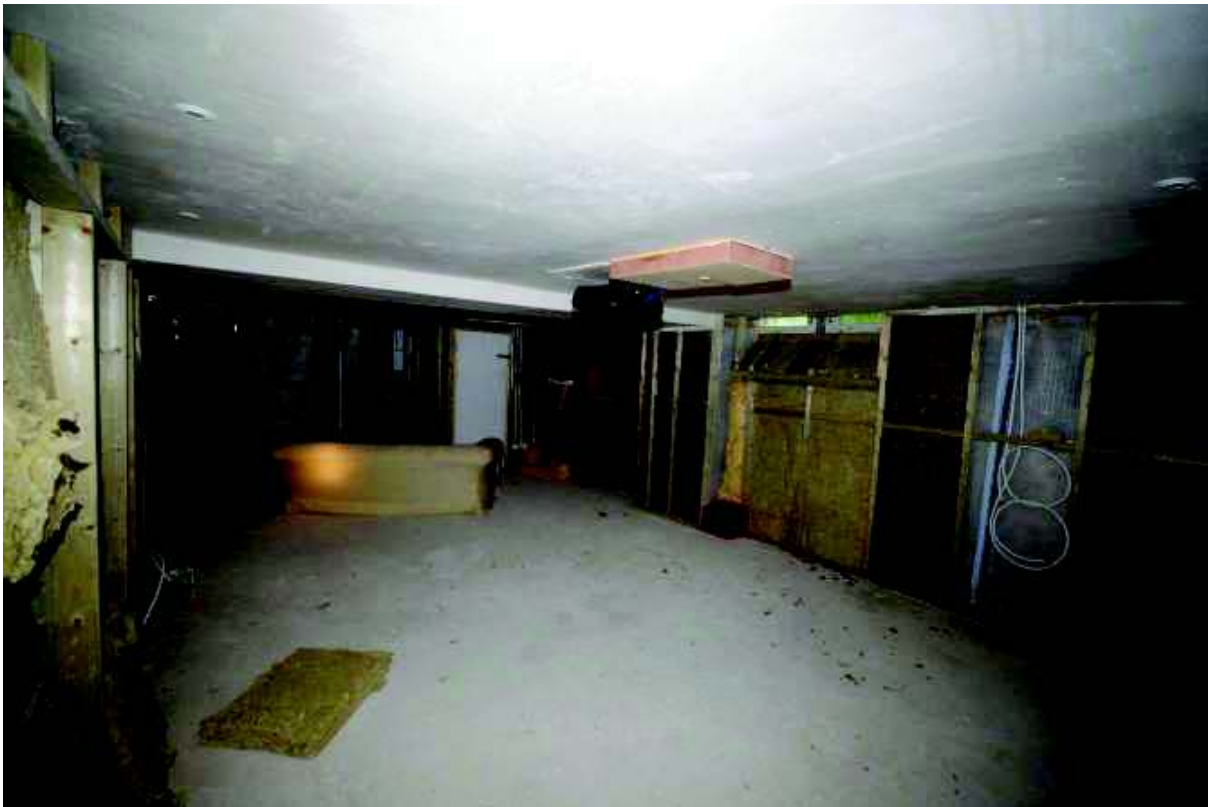
Plate 15: Eastern aspect, southeast cellar room
