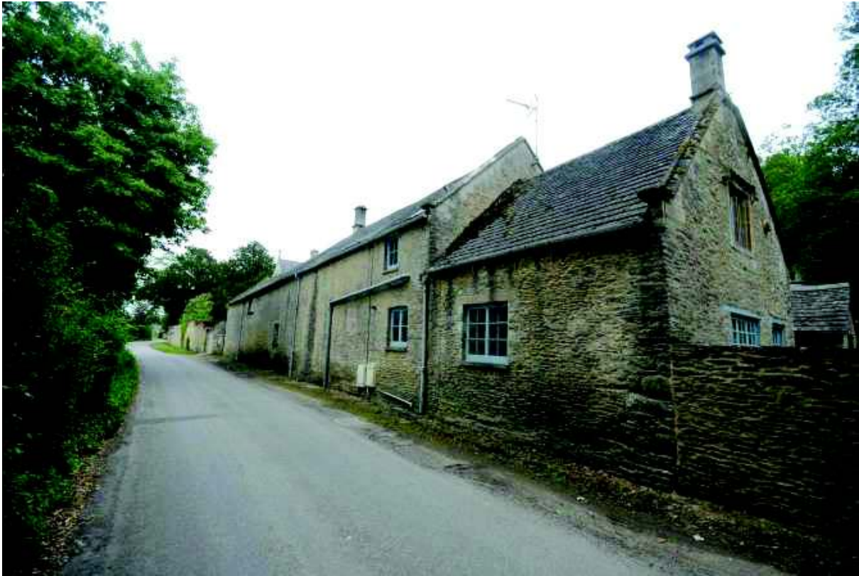
Plate 104: Northeast elevation viewed from north
