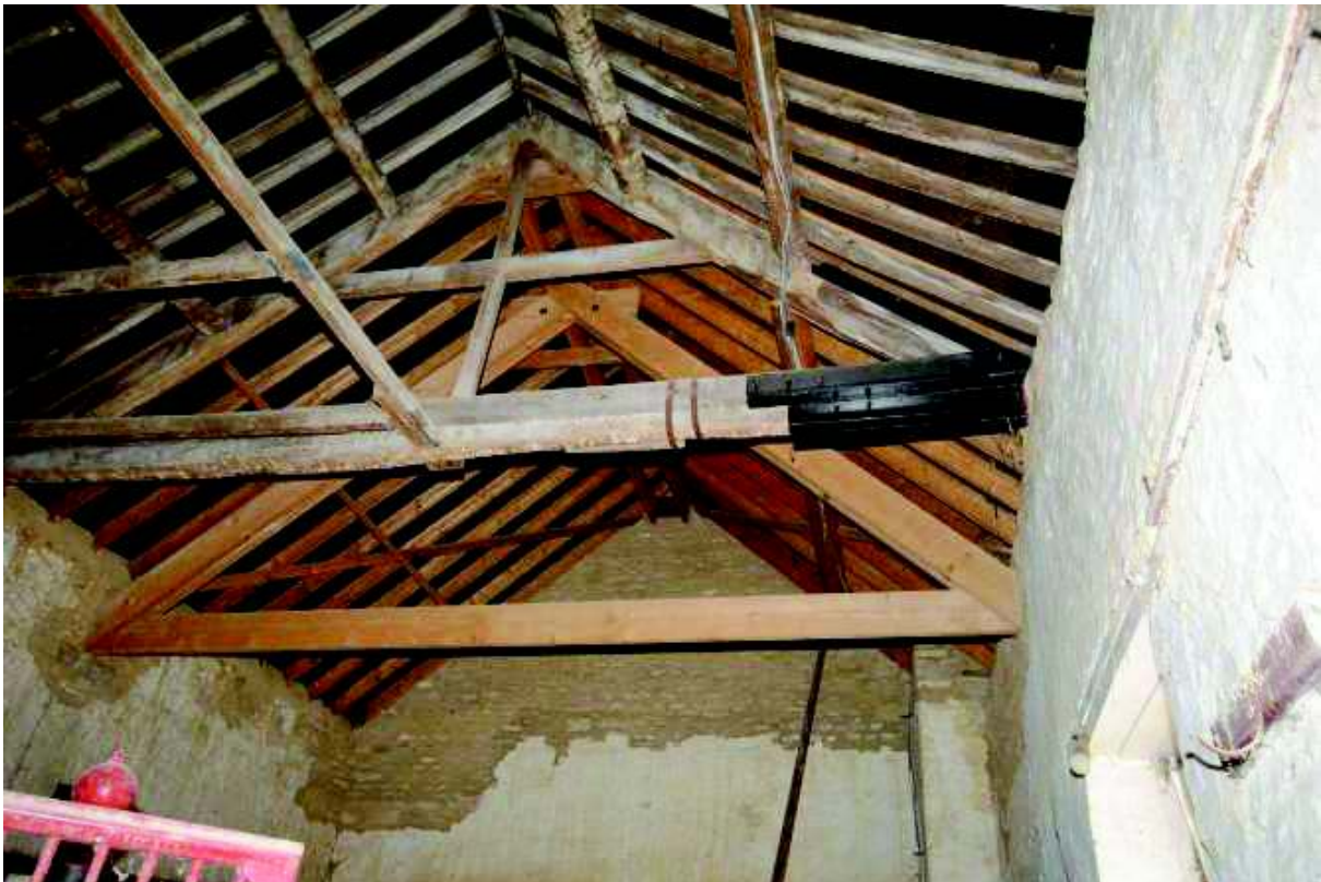
Plate 120: Detail of roof structure
