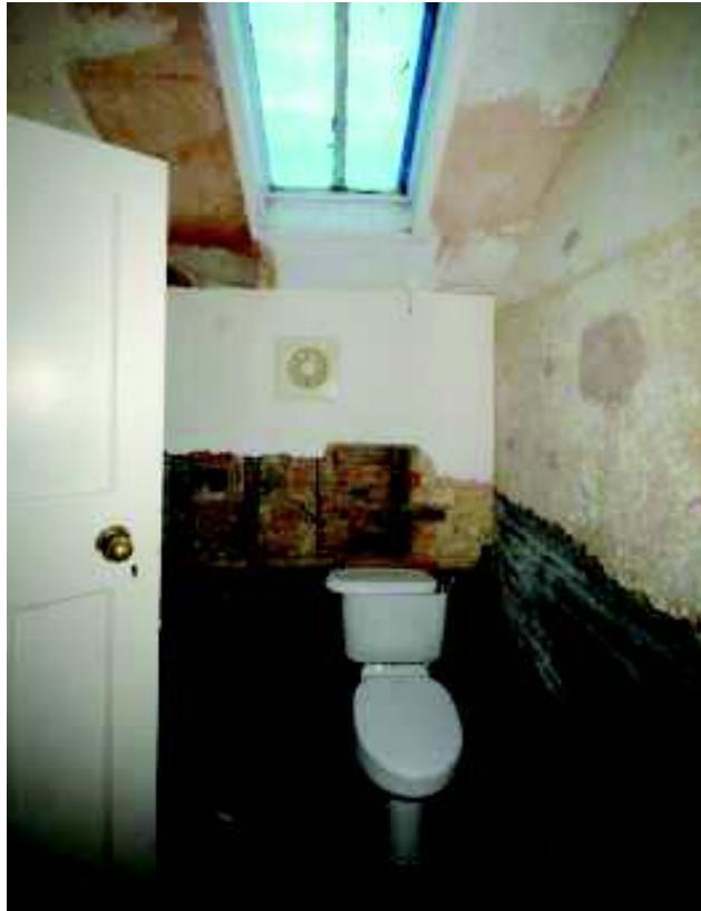
Plate 61: Northeast aspect, lavatory
