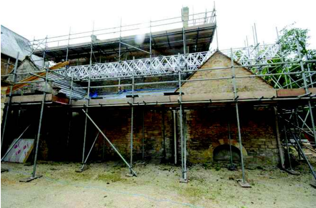
Plate 1: Northwest part of northeast elevation, northwest wing
