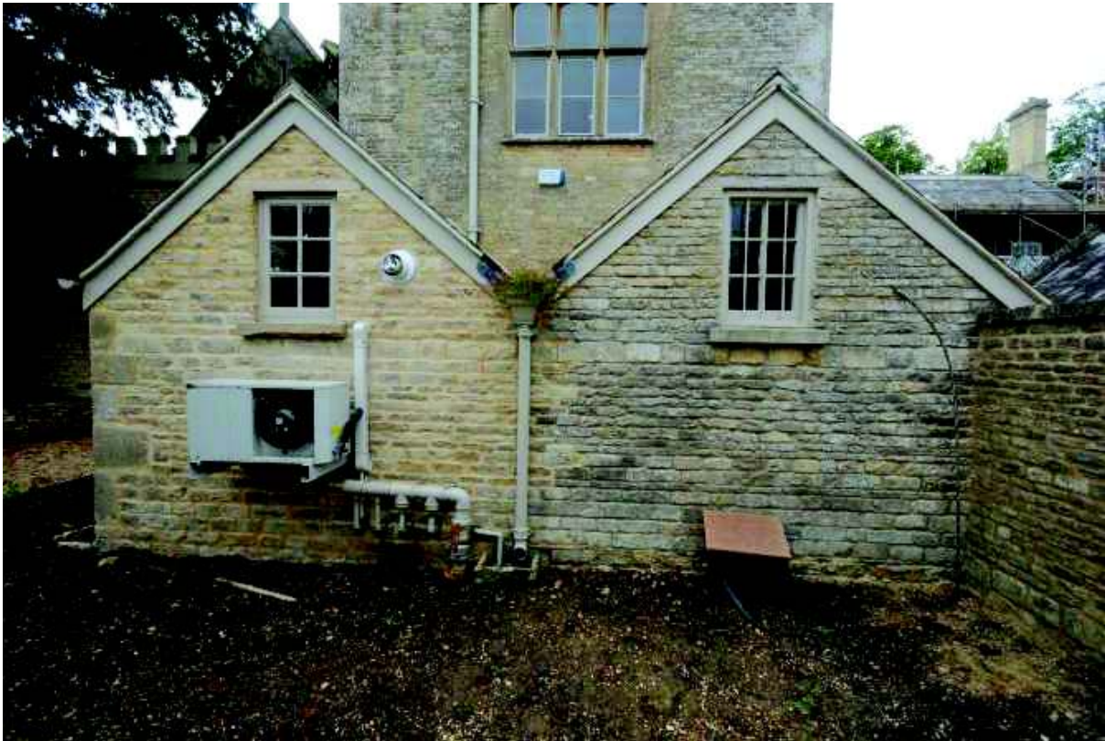
Plate 5: Northeast elevation, northeast extensions
