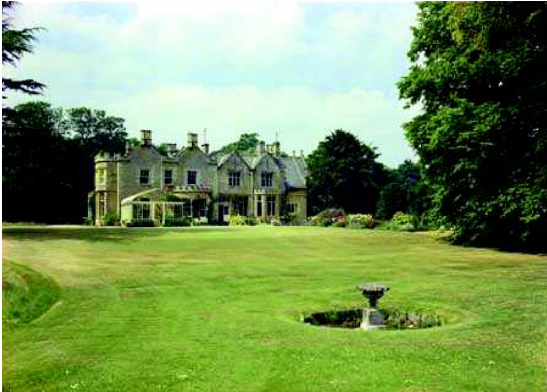
Plate 127: View of rear from across gardens, 1974
