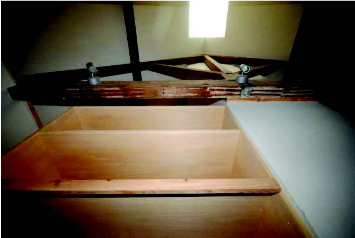
Plate 79: Roof structure over storage area
