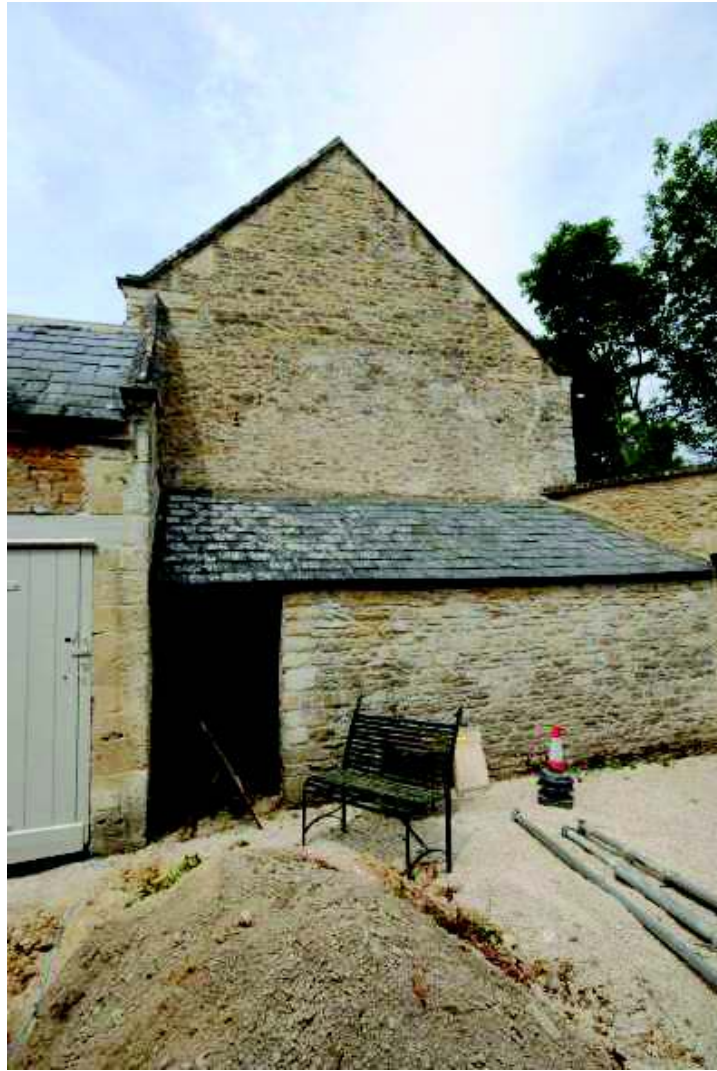
Plate 103: Detail of lean-to structure and southeast wall of main range
