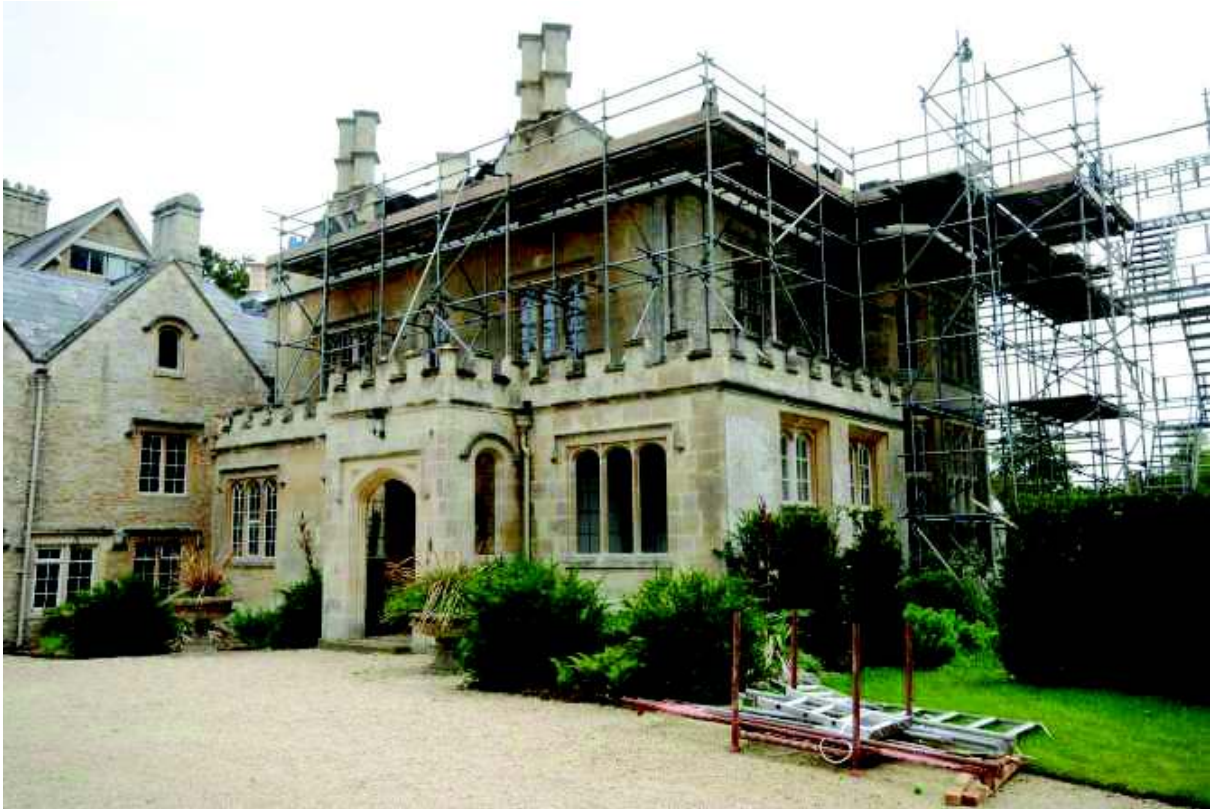
Plate 9: Southwest wing viewed from west
