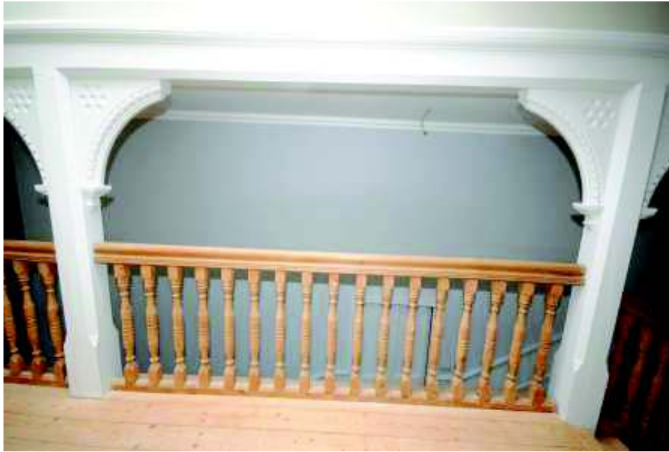
Plate 75: Detail of brackets and balusters
