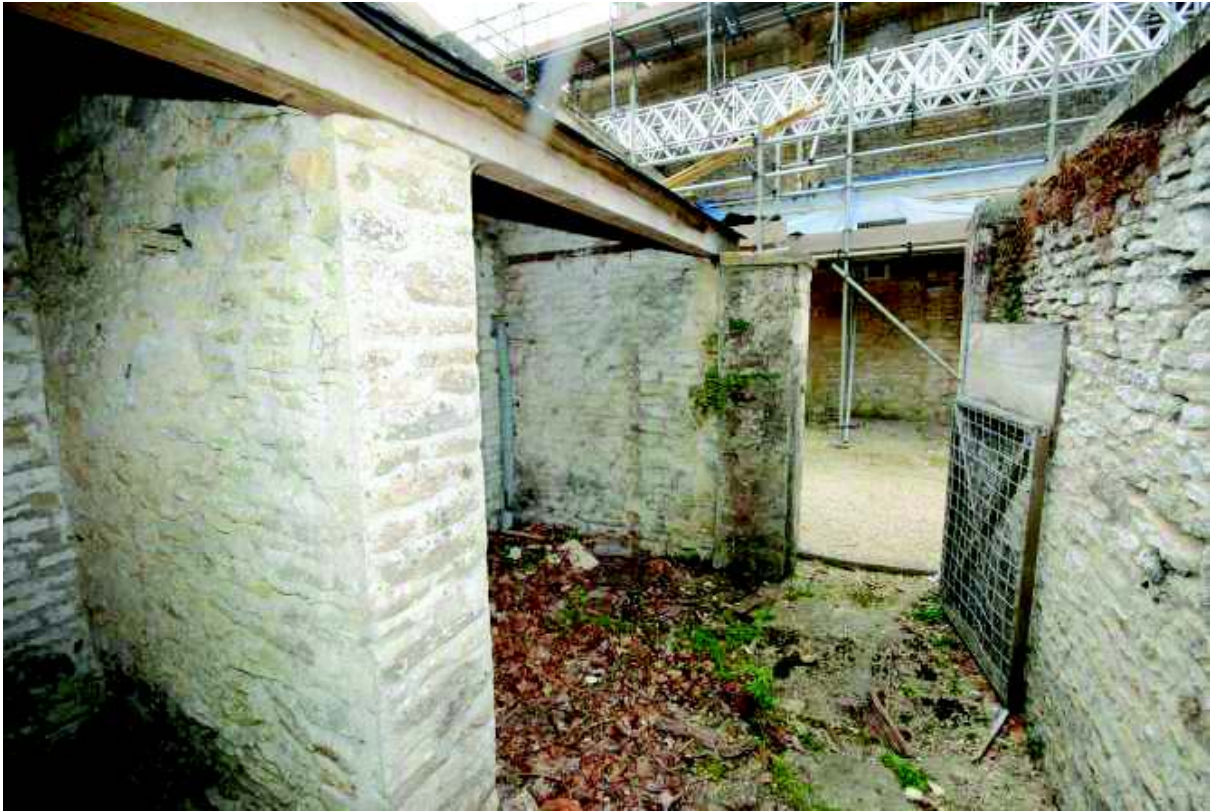
Plate 102: View southwest from coal / wood store
