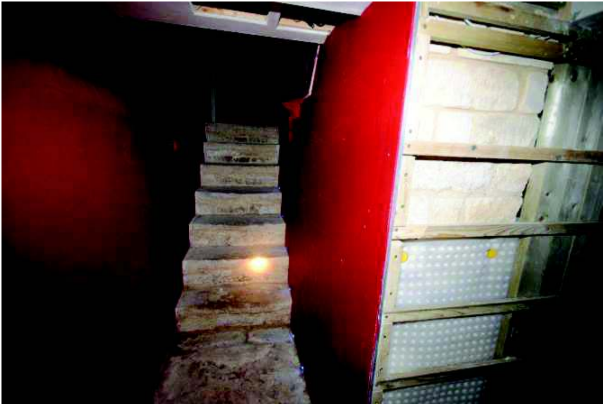
Plate 16: Internal staircase from ground floor
