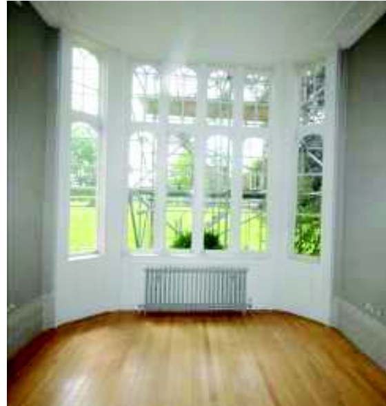
Plate 21: Detail of windows in bays
