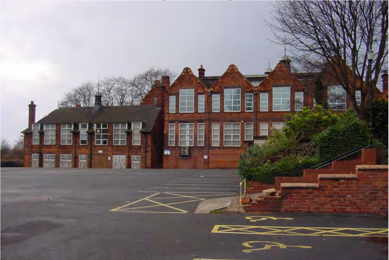
Plate 3: The rear of the building in 2003/4
