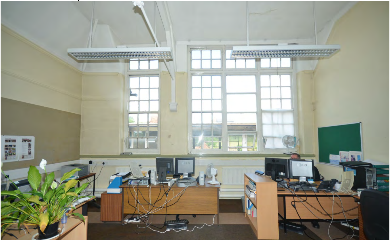
Plate 143: First Floor Room 8 Looking North
