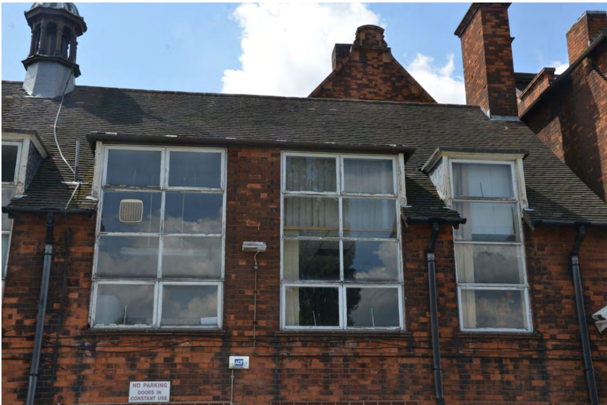
Plate 39: Detail of first floor windows, east wall, southern wing
