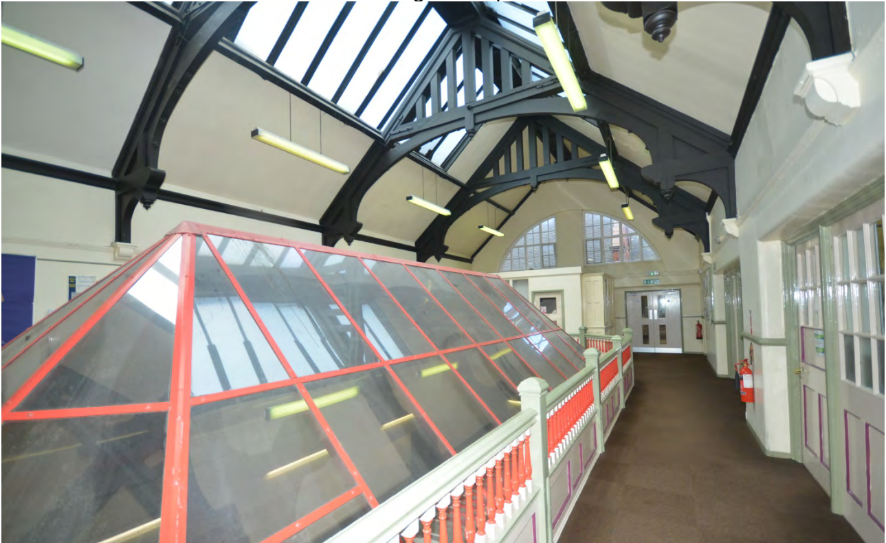
Plate 152: First Floor Room 12 Looking North
