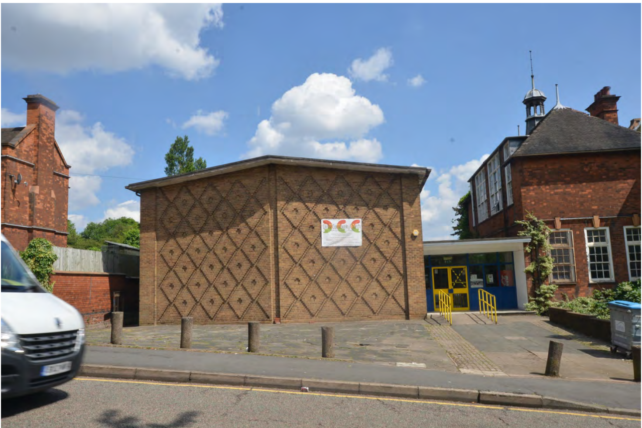
Plate 49 Extension to north
