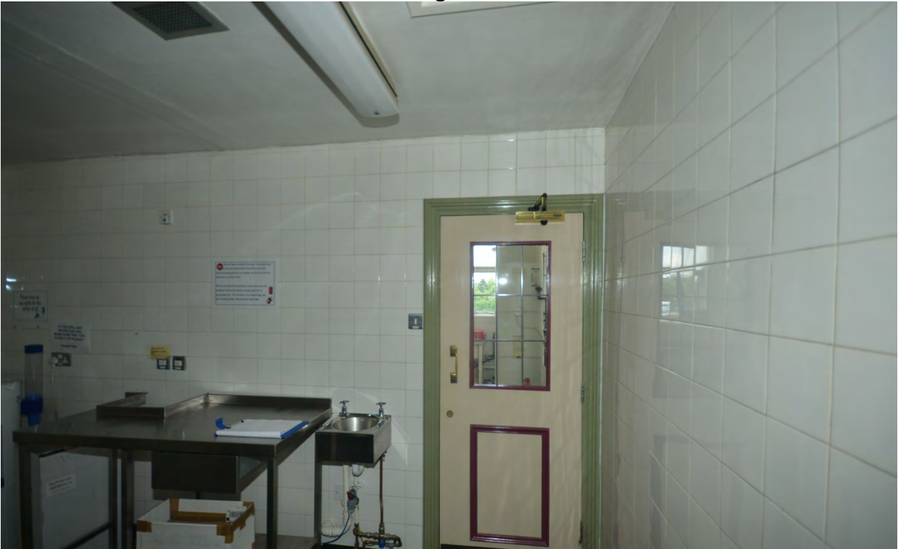
Plate 113: Ground Floor Room 23 Looking East
