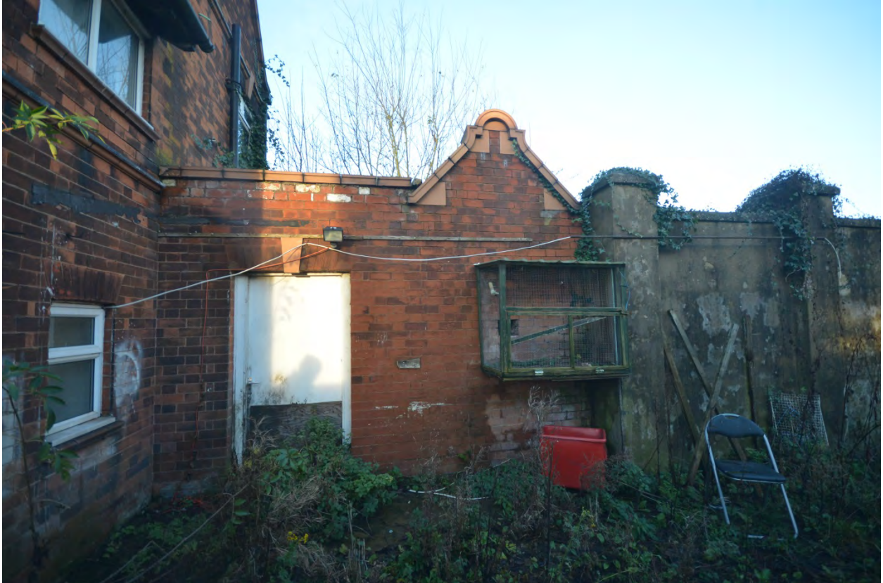
Plate 204: South elevation, outbuilding to rear of house
