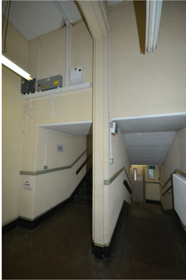
Plate 98: Ground Floor Room 17 Looking West
