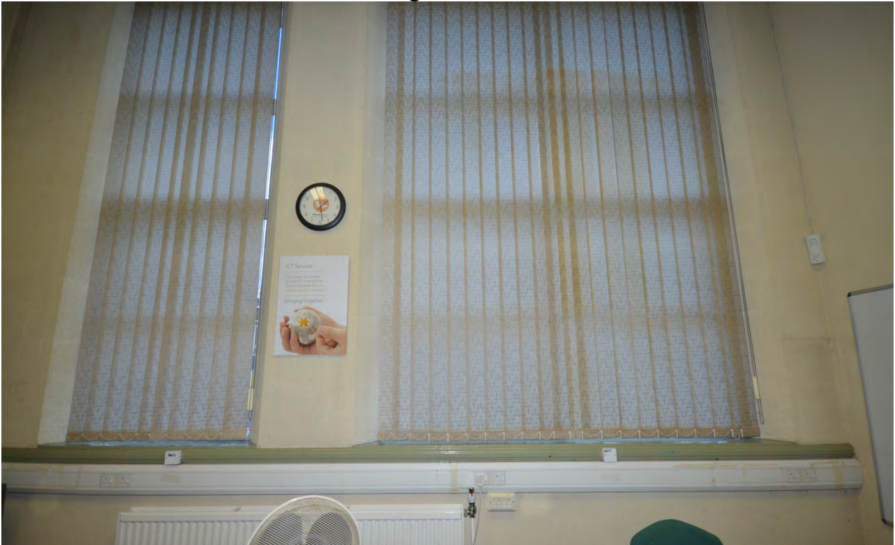
Plate 63: Ground Floor Room 5 Looking East
