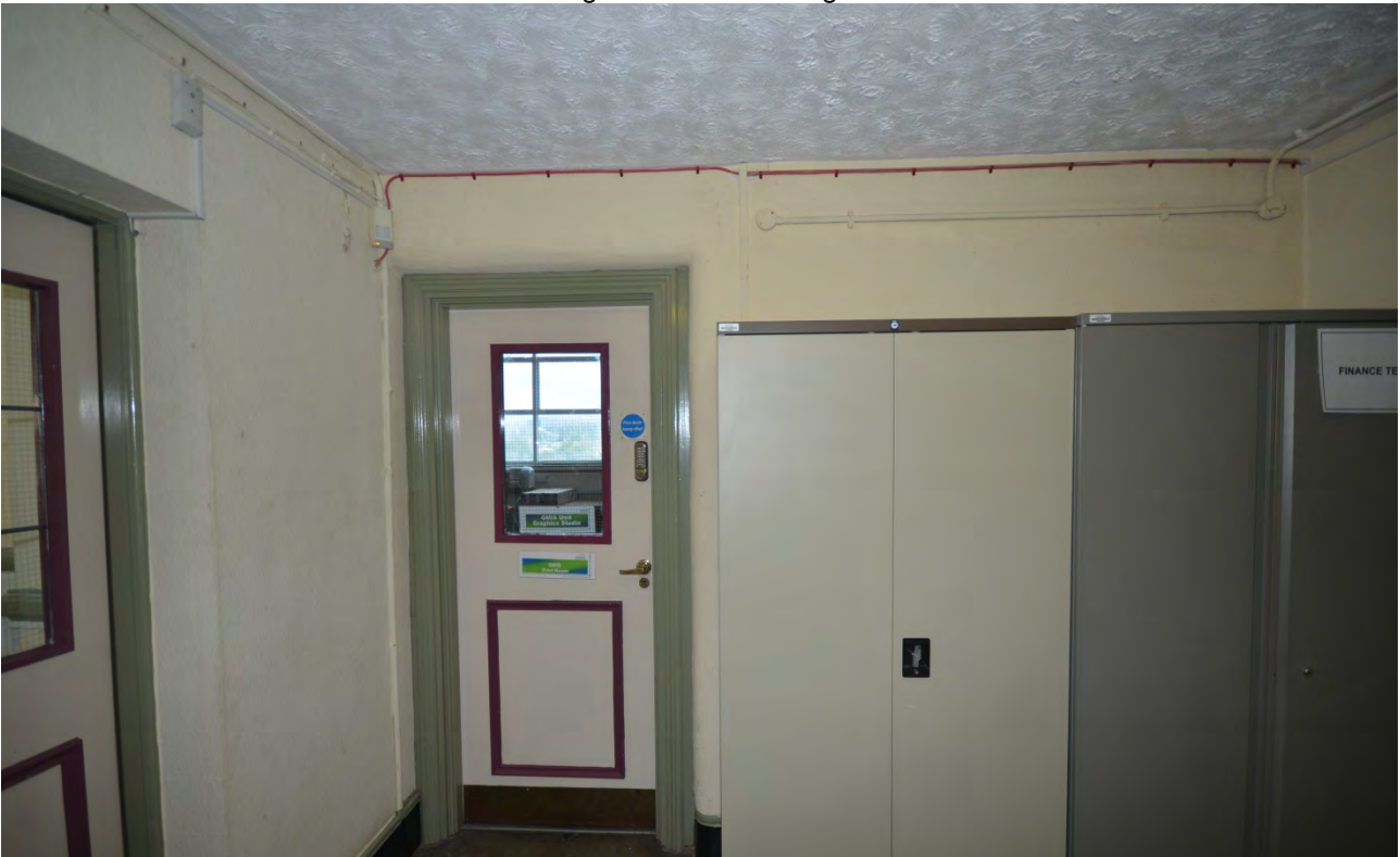
Plate 169: First Floor Room 18 Looking East
