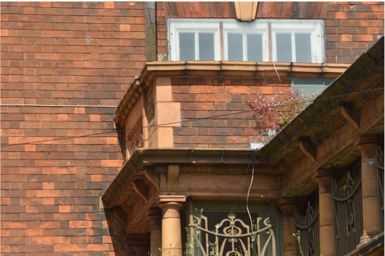
Plate 27: Detail of parapet and pilasters over girls' entrance
