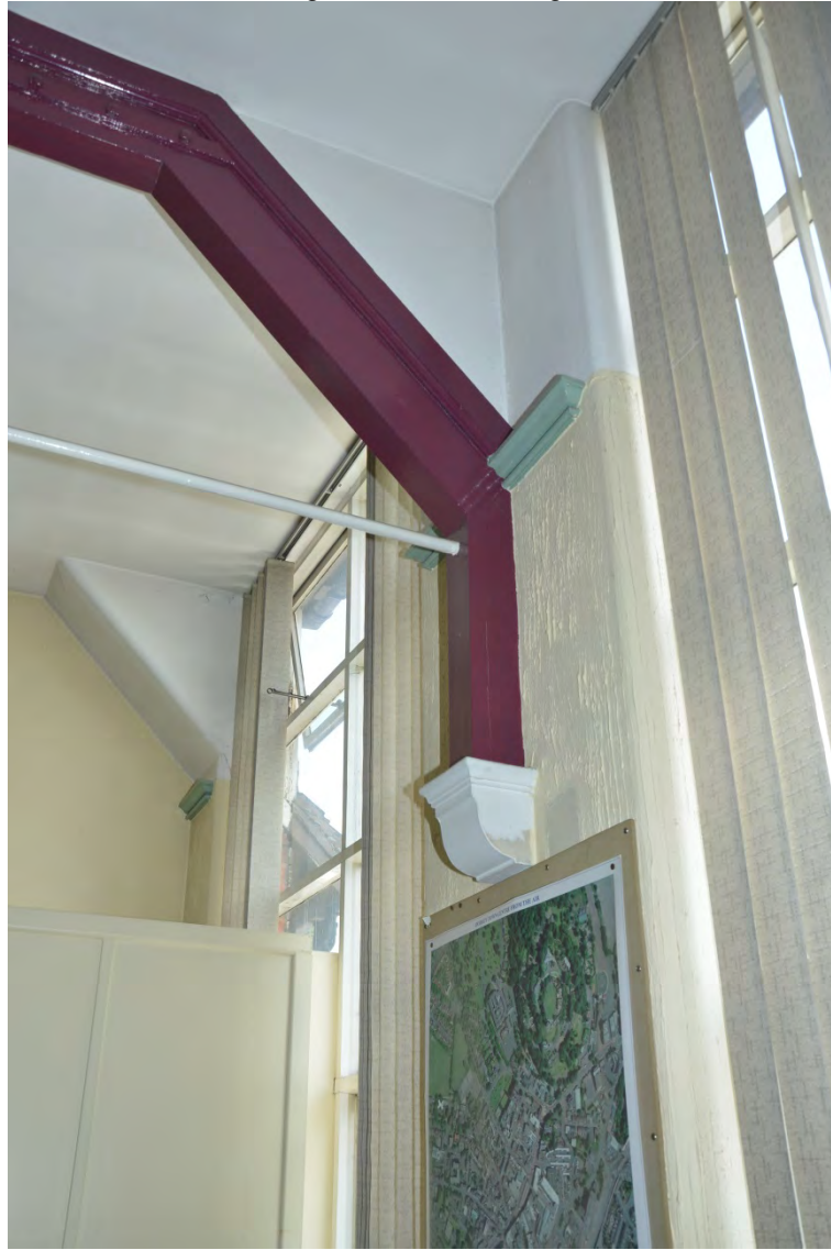
Plate 122: Detail of roof truss and corbel
