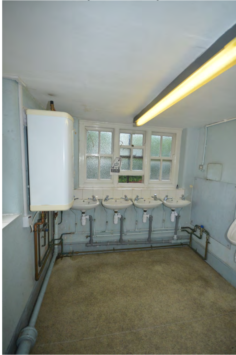
Plate 104: Ground Floor Room 19 Looking West
