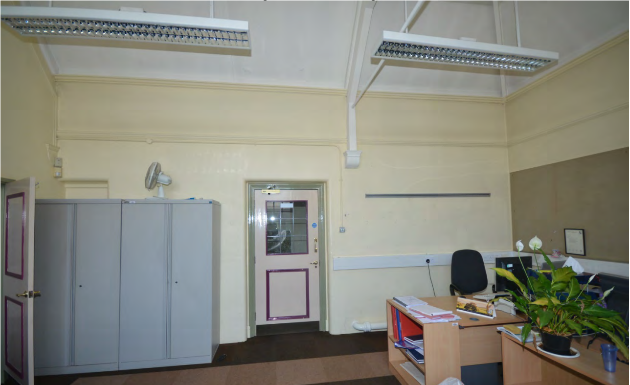
Plate 145: First Floor Room 8 Looking South
