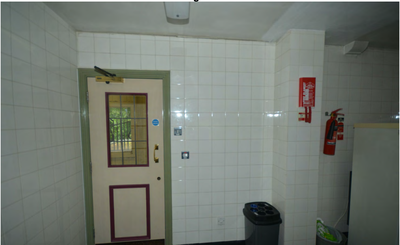
Plate 115: Ground Floor Room 23 Looking West
