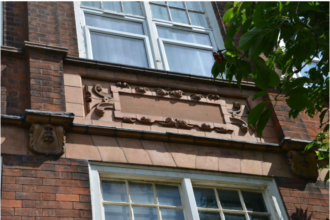
Plate 21: Detail of ceramic mouldings, central gables
