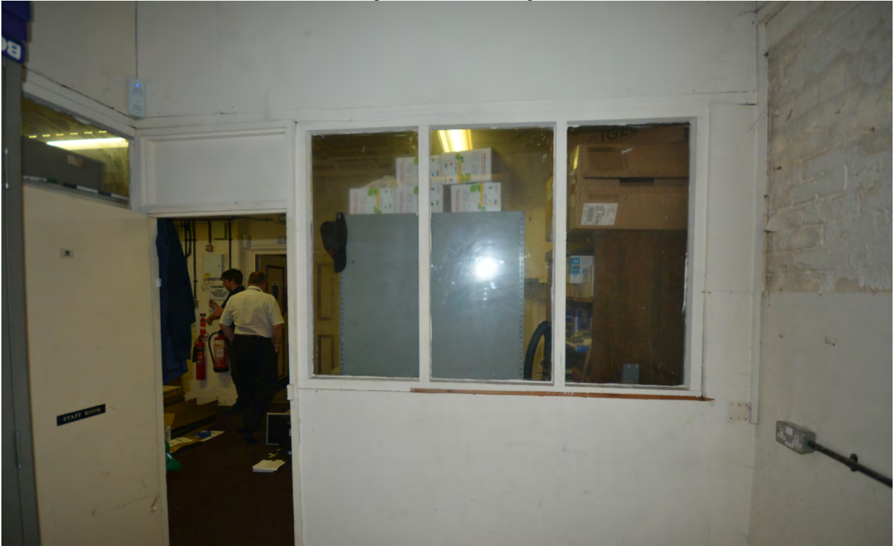
Plate 196: Lower Ground Floor Room 3 Looking West
