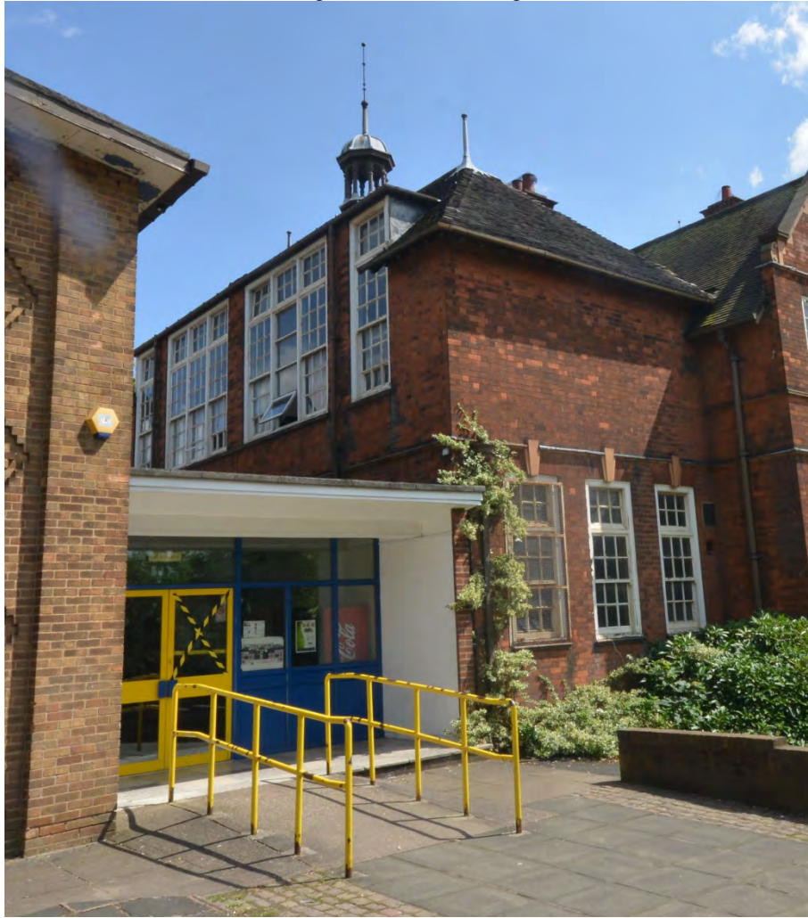
Plate 16: Detail of northern end, west elevation
