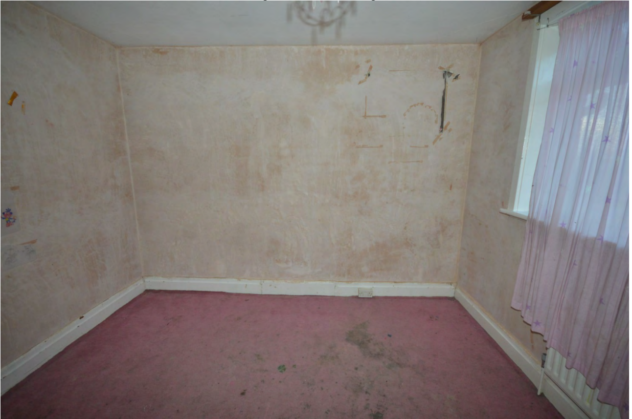
Plate 222: Southern aspect, southwest bedroom
