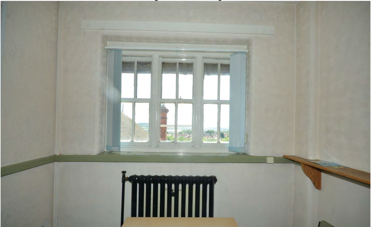
Plate 178: First Floor Room 21 Looking South
