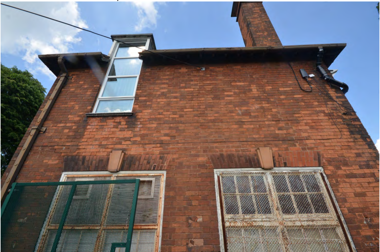
Plate 34: South elevation, southern wing
