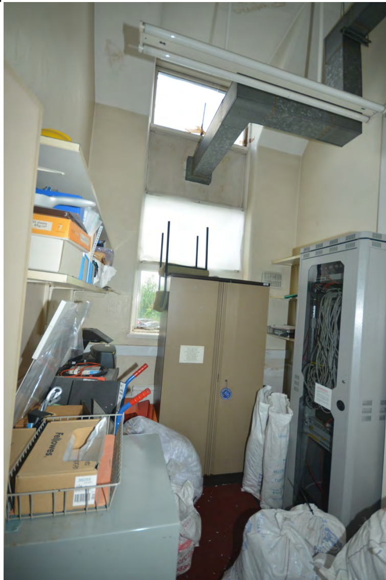
Plate 117: Ground Floor Room 25 Looking East
