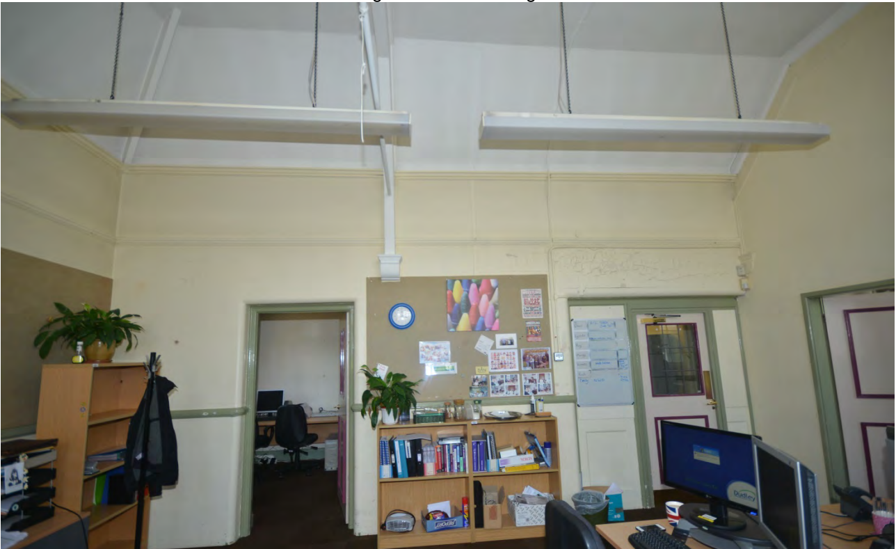
Plate 125: First Floor Room 1 Looking South
