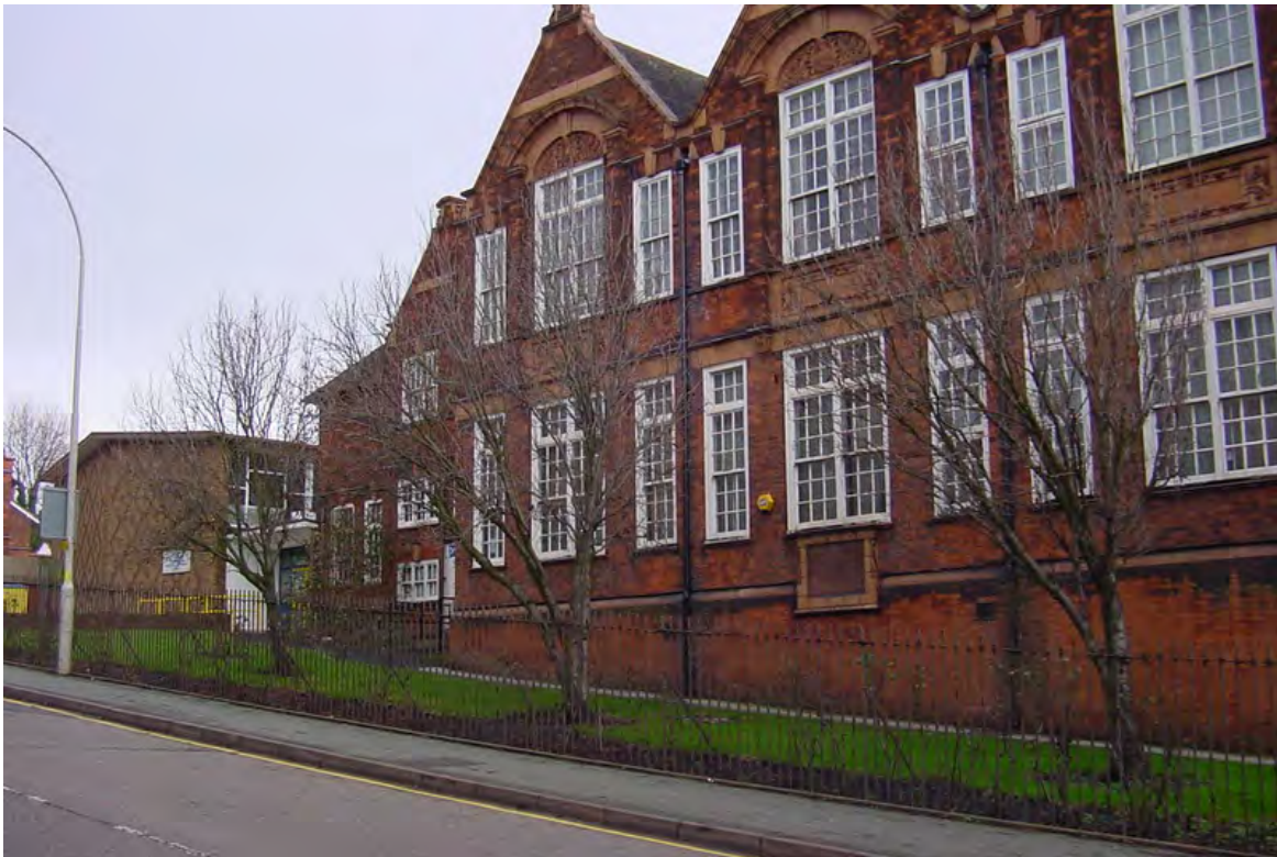
Plate 2: The facade in 2003/4
