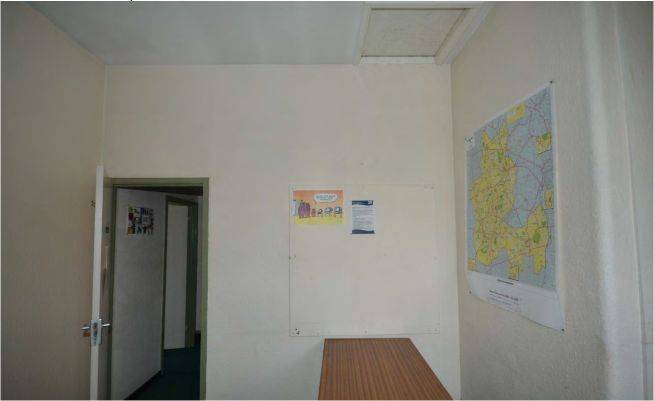
Plate 180: First Floor Room 22 Looking North
