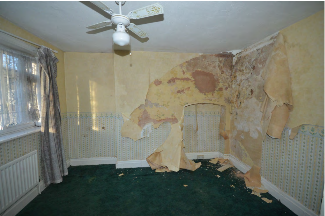
Plate 219: North aspect, northwest bedroom
