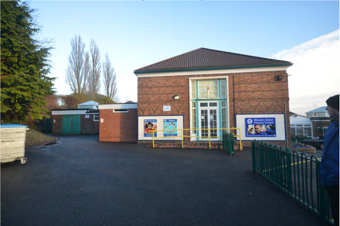
Plate 12 Blowers Green Primary School
