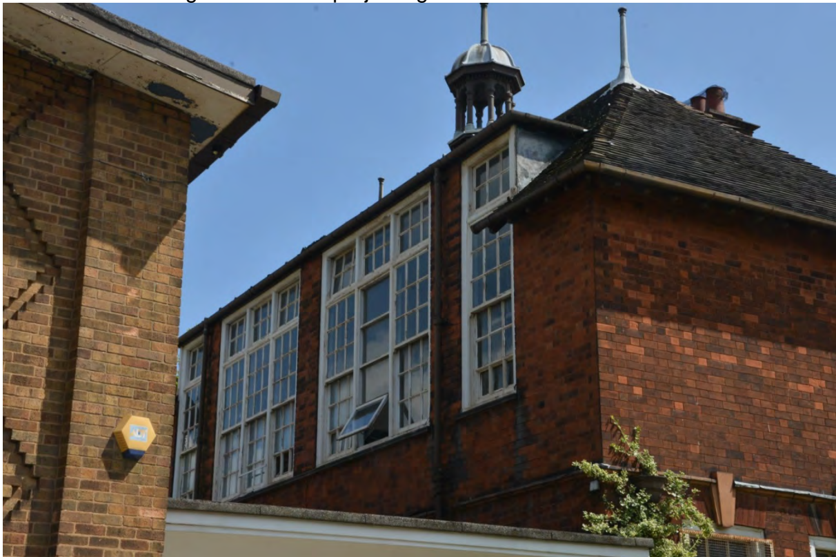
Plate 45: Detail of first floor windows, north elevation
