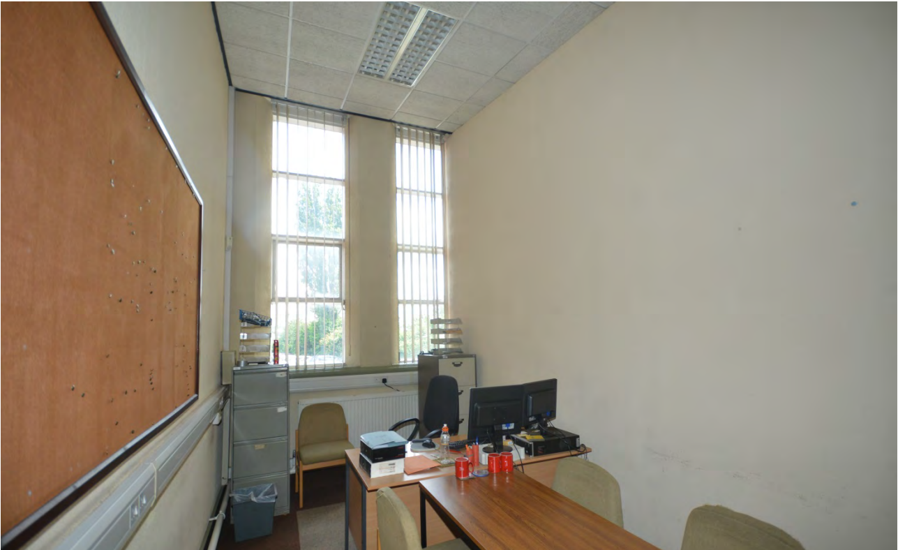
Plate 78: Ground Floor Room 11 Looking East
