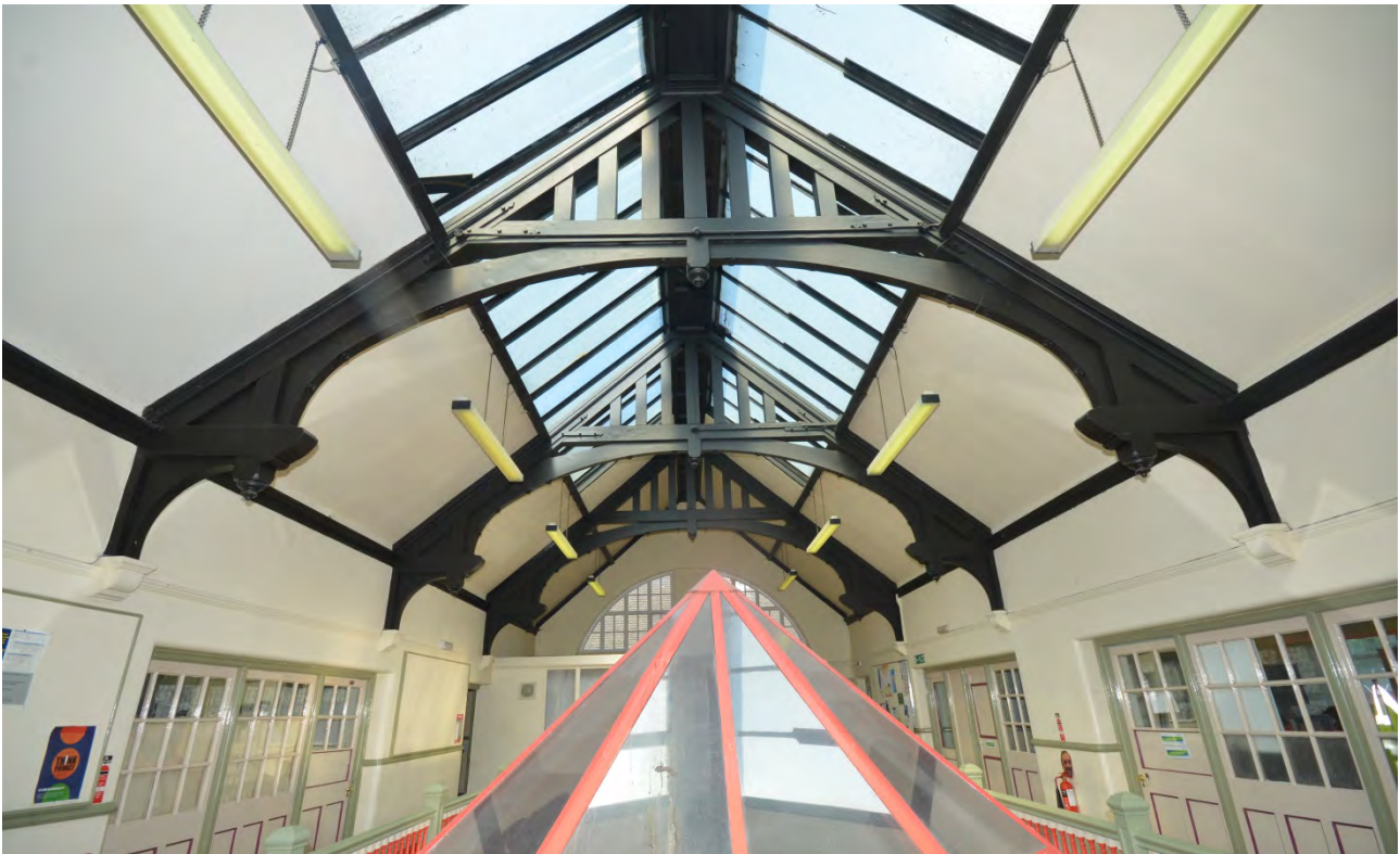
Plate 153: First Floor Room 12 Looking South
