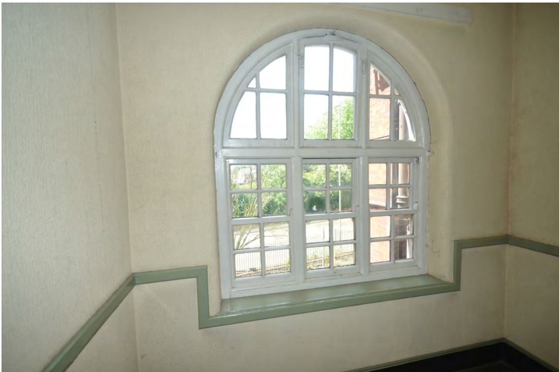
Plate 151: Arched window, staircase
