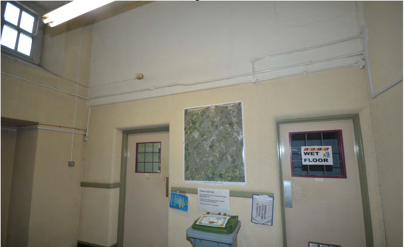
Plate 101: Ground Floor Room 18 Looking West
