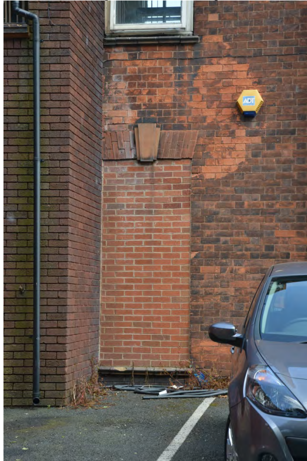
Plate 31: Detail of blocked window, west elevation, southern wing
