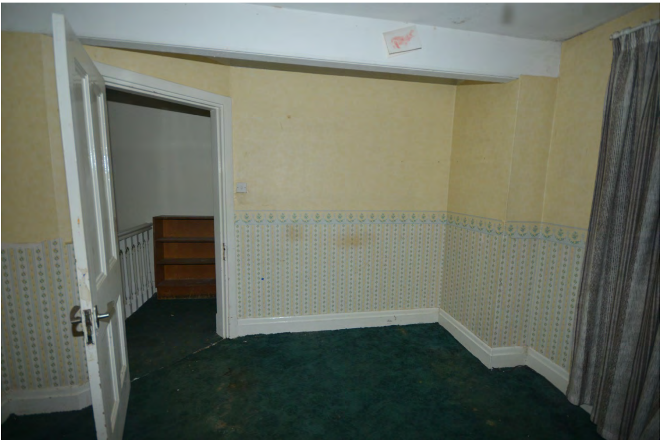
Plate 220: South aspect, northwest bedroom
