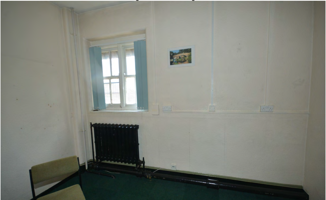
Plate 182: First Floor Room 22 Looking South
