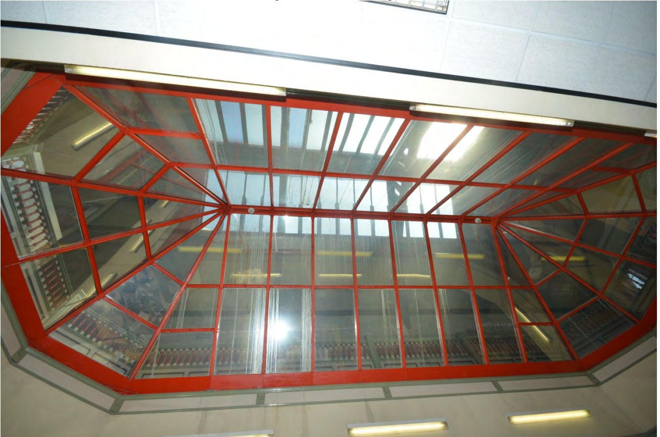
Plate 86: Detail of lantern
