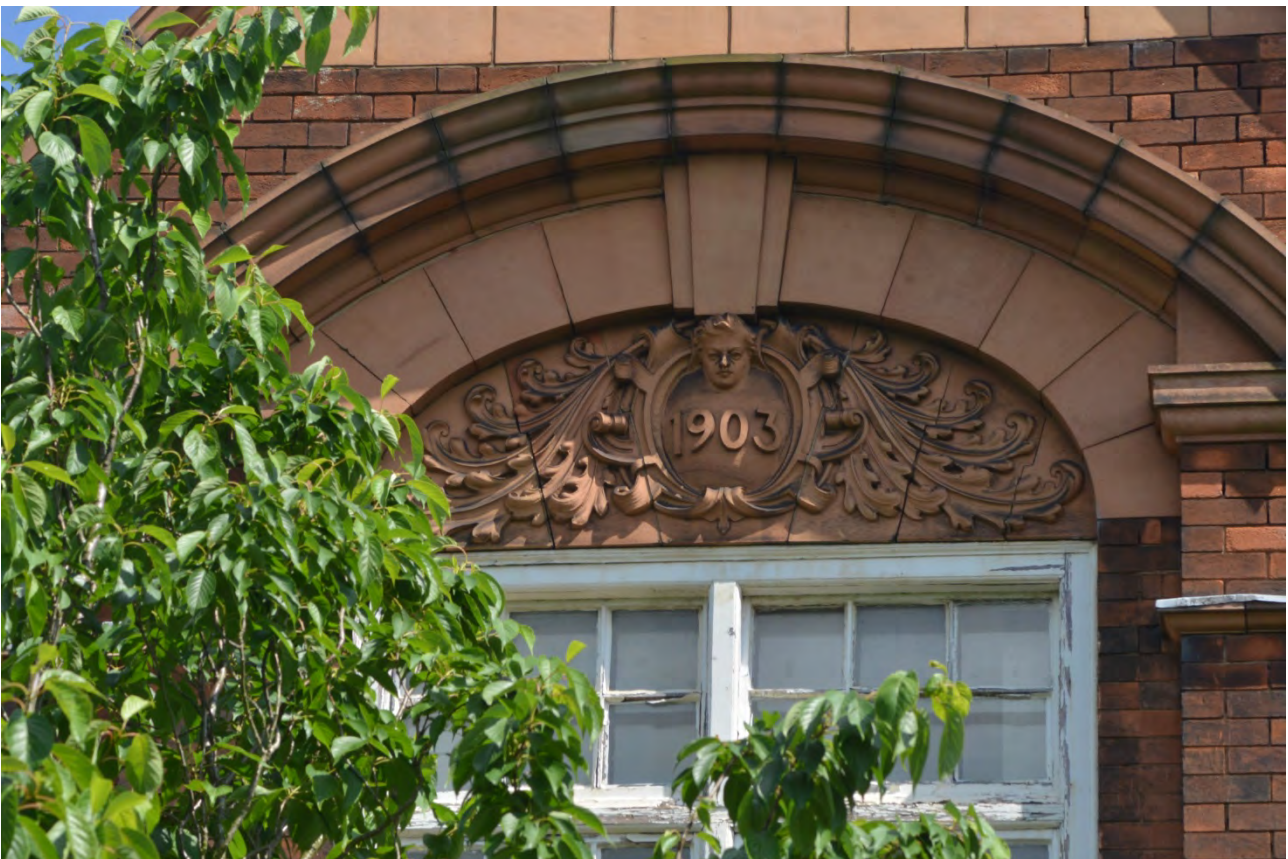
Plate 24: Detail of dated moulding at head of central gable
