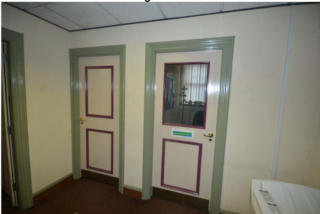
Plate 59: Ground Floor Room 4 Looking East
