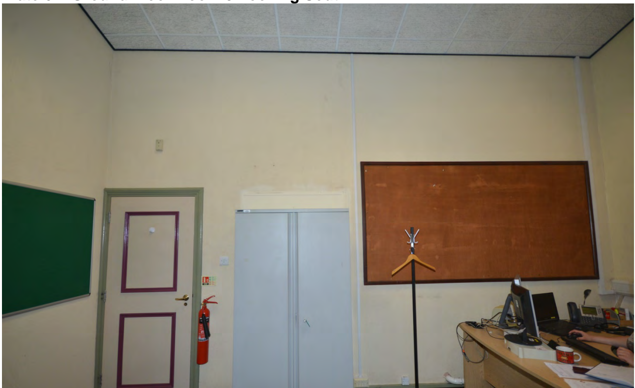
Plate 65: Ground Floor Room 5 Looking West
