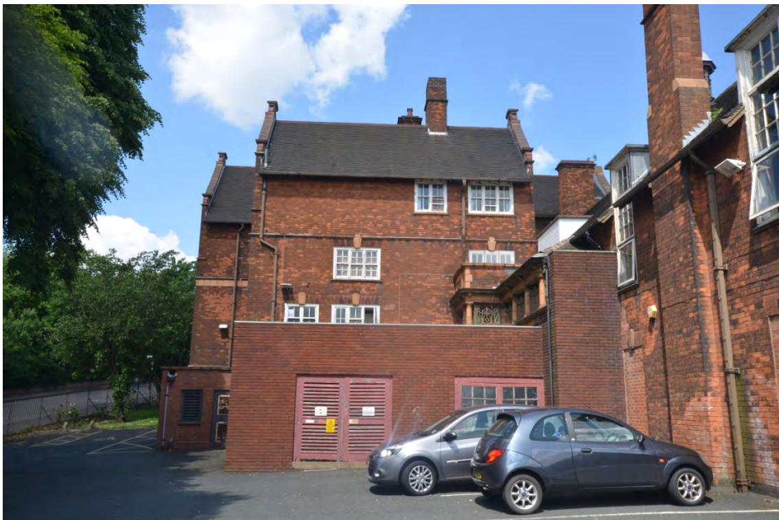
Plate 32: South elevation, western part of building
