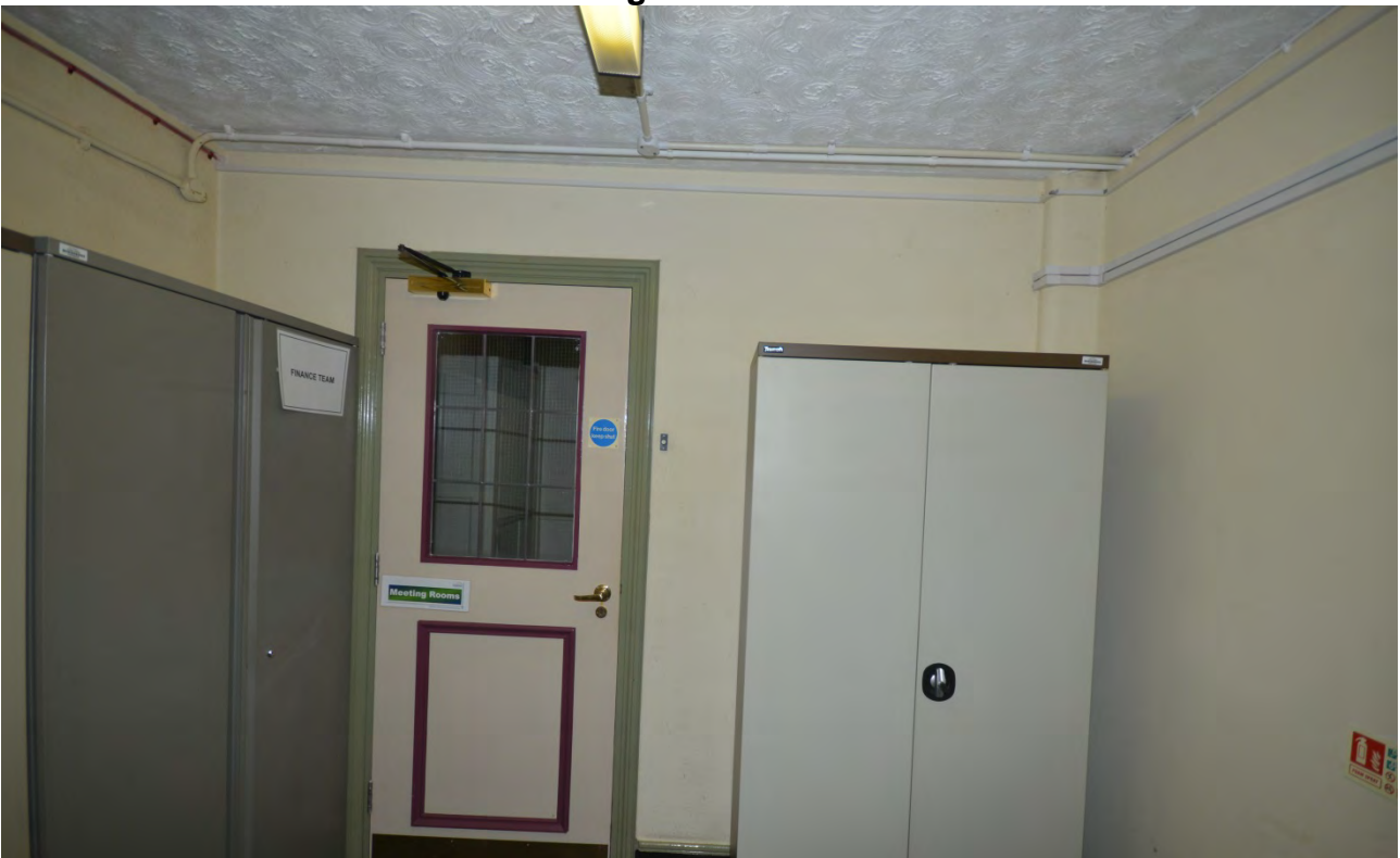
Plate 170: First Floor Room 18 Looking South
