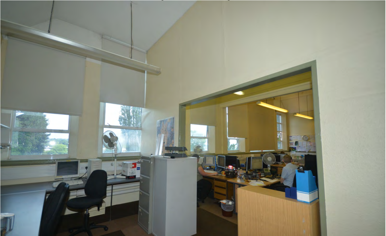
Plate 135: First Floor Room 4 Looking Southeast
