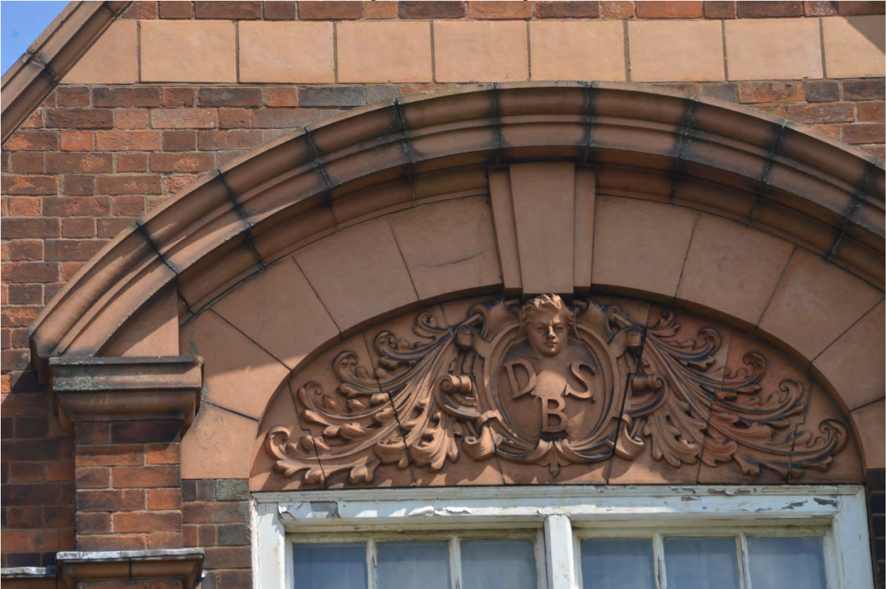
Plate 23: Detail of moulding at head of Coped gable
