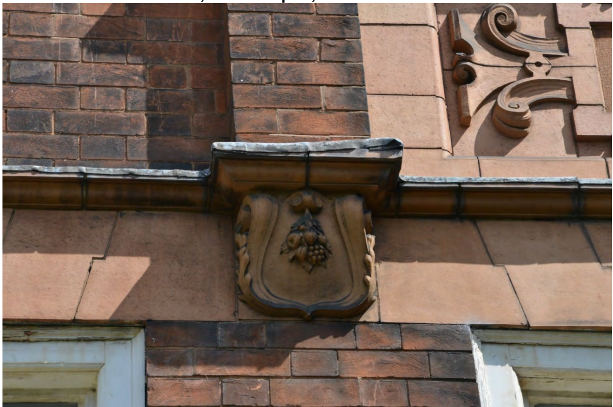
Plate 20: Detail of ceramic mouldings, central gables
