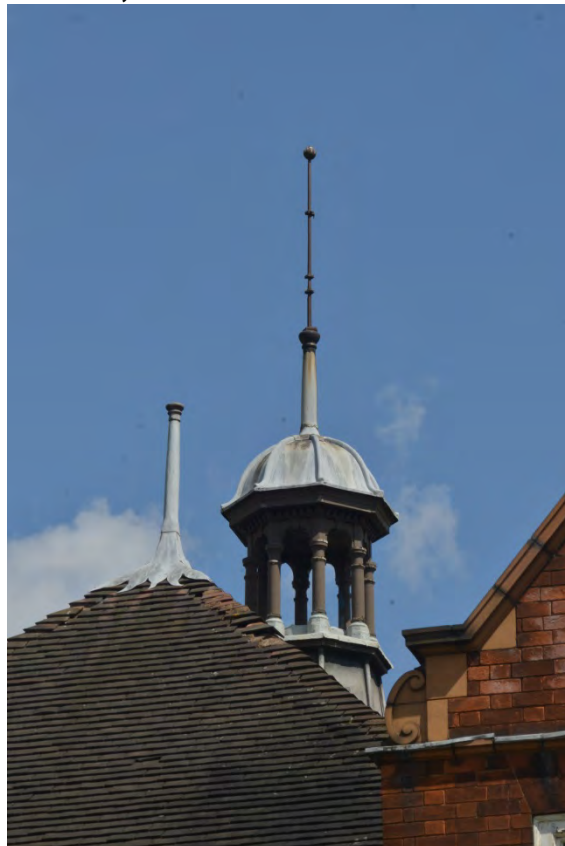
Plate 17: Detail of cupola vent and finial
