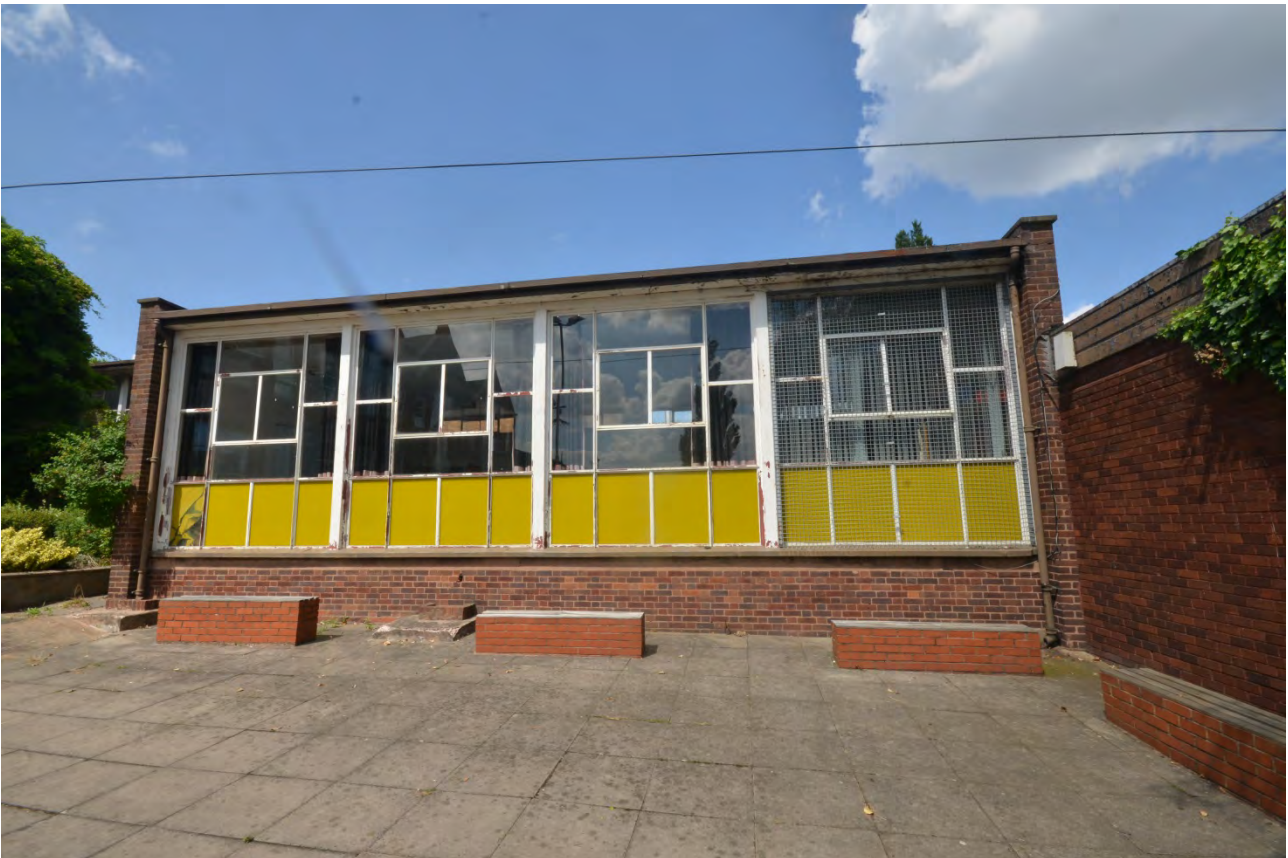
Plate 47 Extension to north
