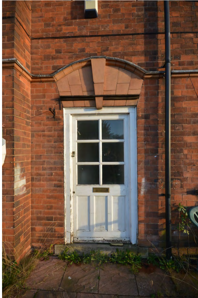
Plate 202: Detail of front door The front door is a modern timber replacement.
