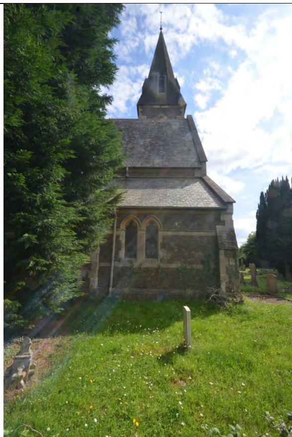
Plate 2 The Steeple North Elevation
