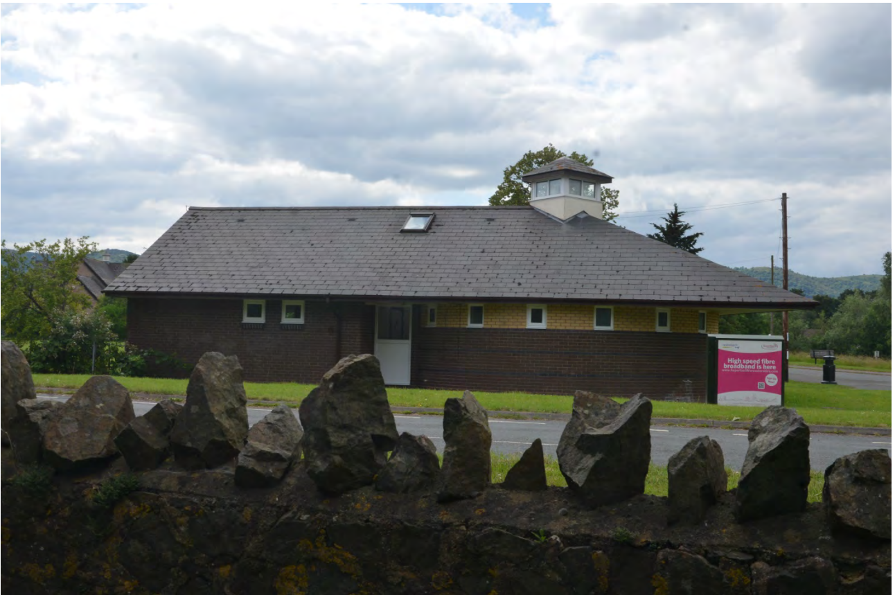
Plate 9 This recent building has totally removed views of the Malvern Hills. The BT advertising hoarding is an eyesore.
