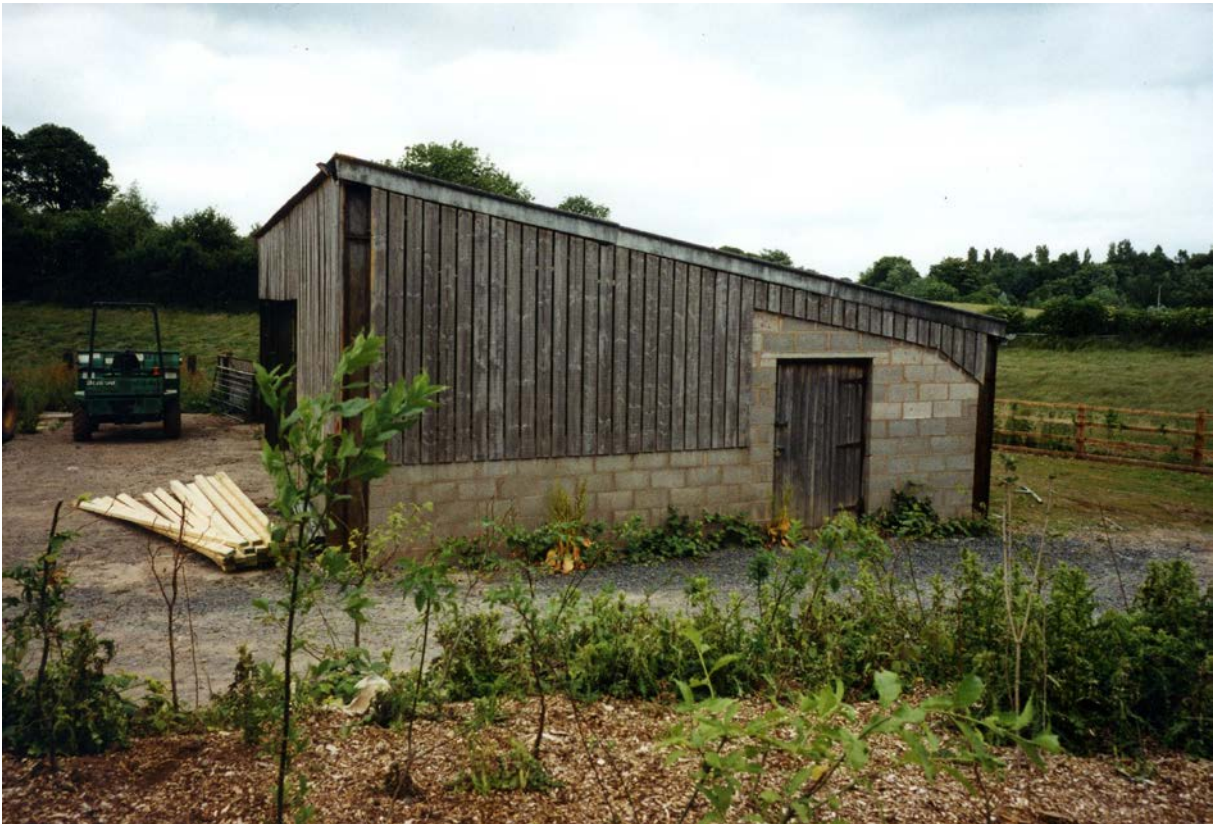
Plate 8: Southern elevation, shed / garage, prior to reordering
