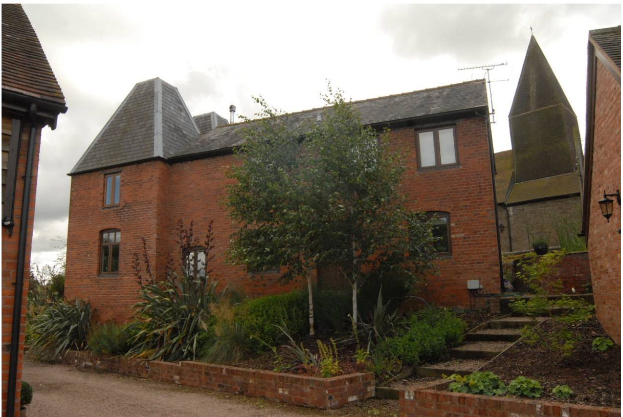
Plate 2: Northern elevation, The Hop Kiln
