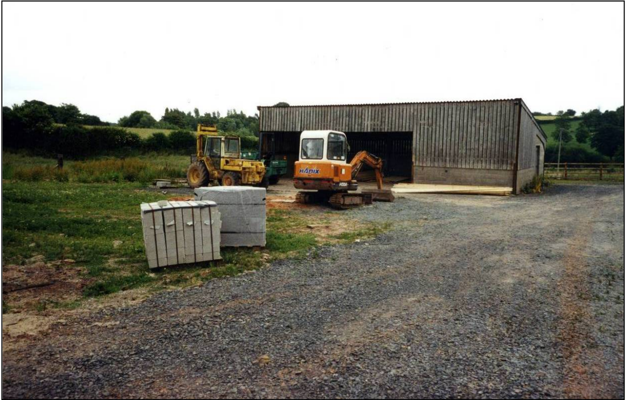
Plate 7: Western elevation, shed / garage, prior to reordering
