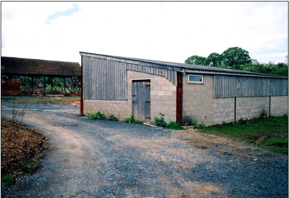
Plate 6: Shed / garage viewed from southeast, prior to reordering
