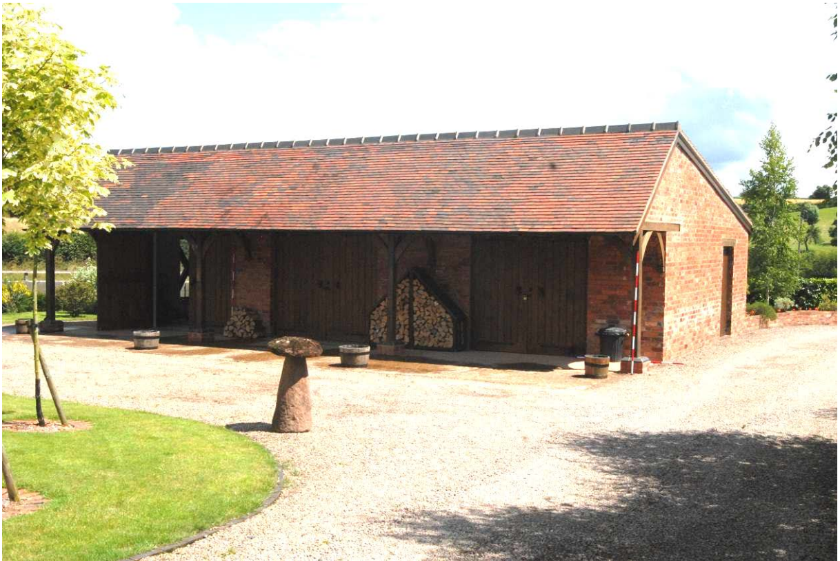
Plate 5: The Garage, western elevation
