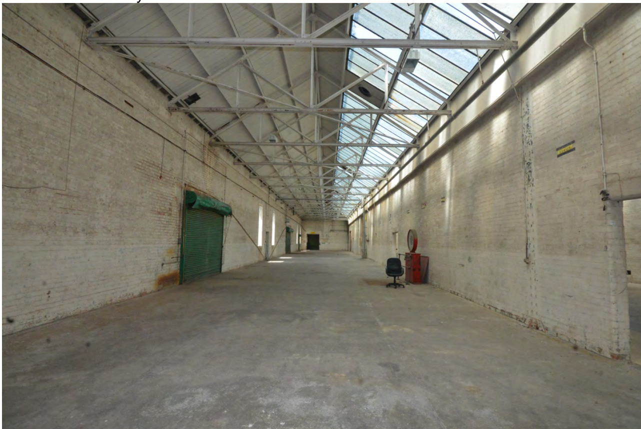
Plate 1: Section of factory without tiled walls
