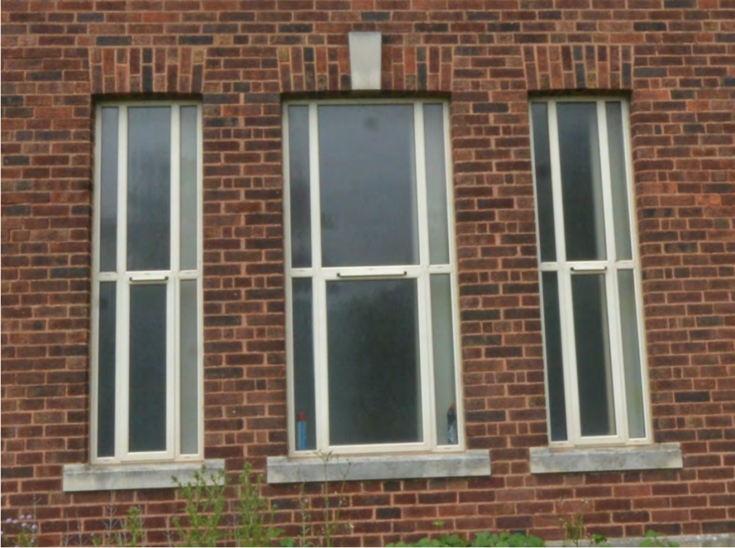
Plate 2: Powder coated Aluminium windows on "Admin" building
