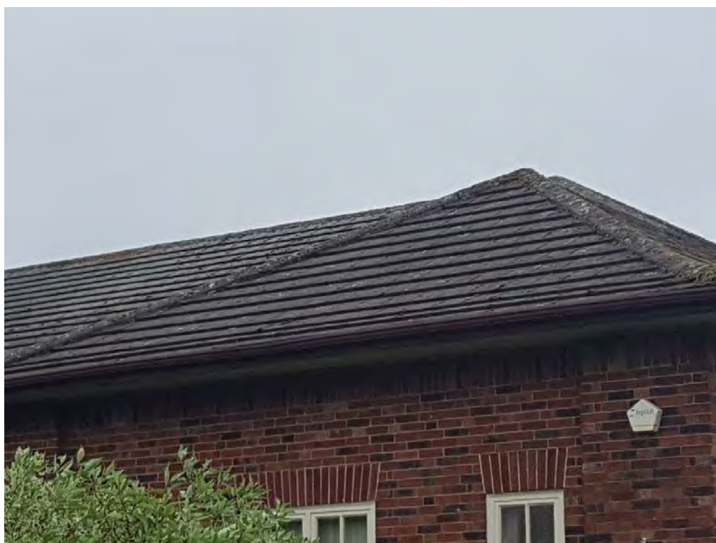
Plate 4: Concrete tiles on roof of “Welfare” building
