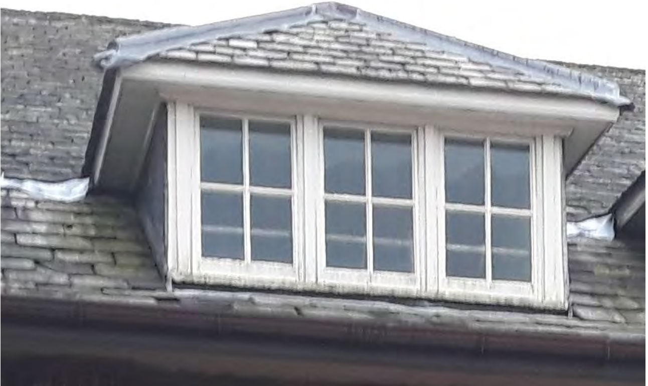
Plate 5 The slate roof of the rear of the welfare building
