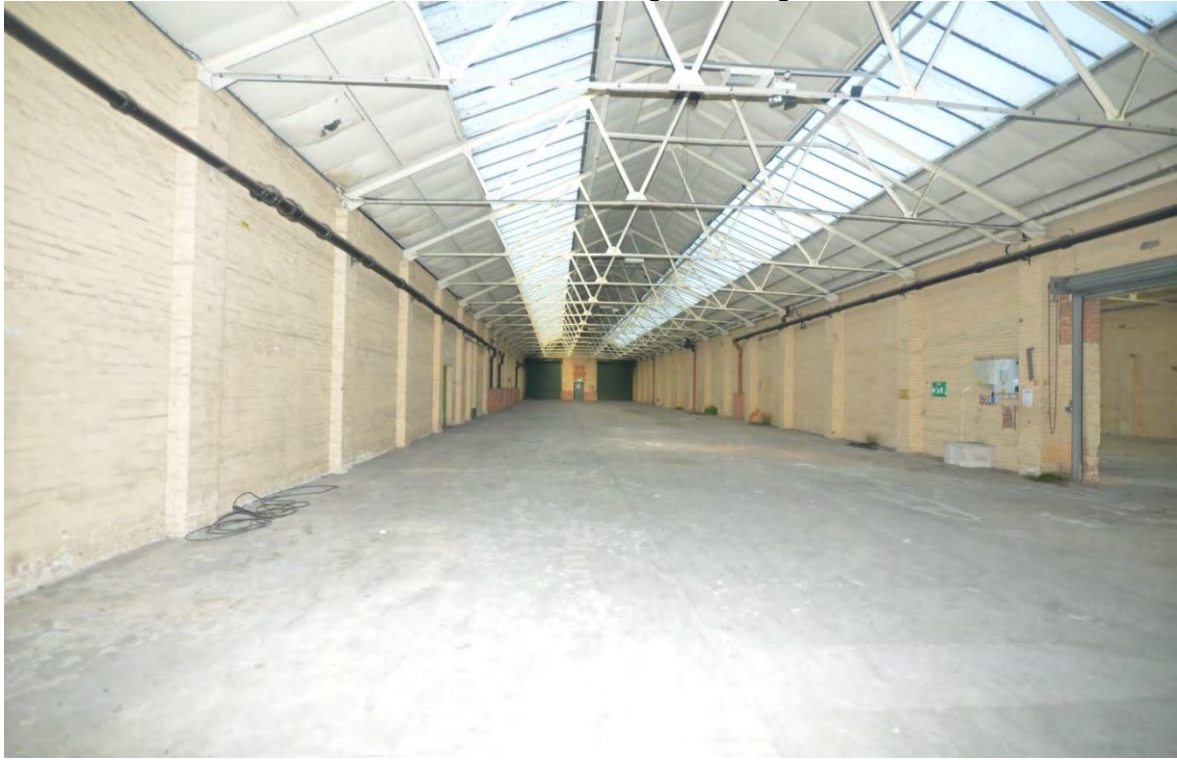
Plate 82: Warehouse Interior North-west bay looking North-east
