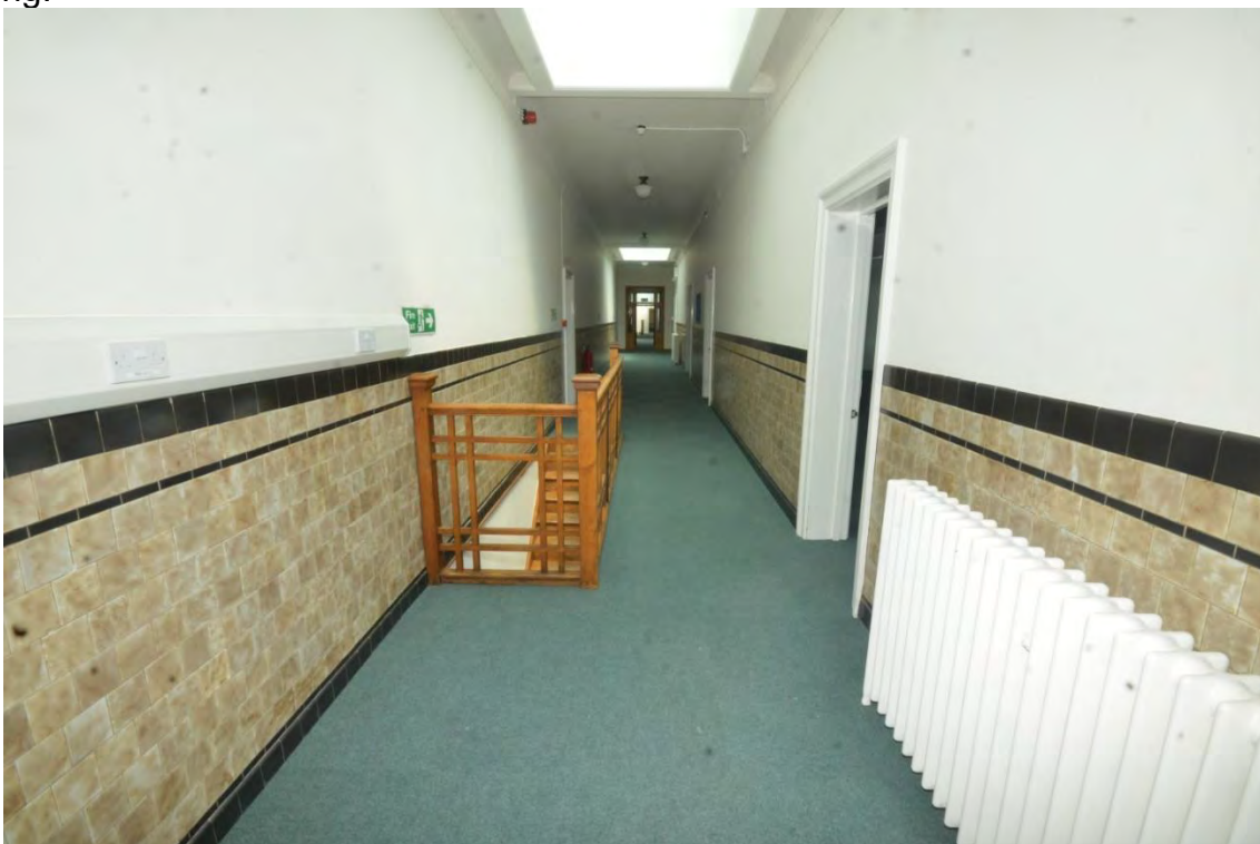
Plate 50: First floor corridor looking northeast
