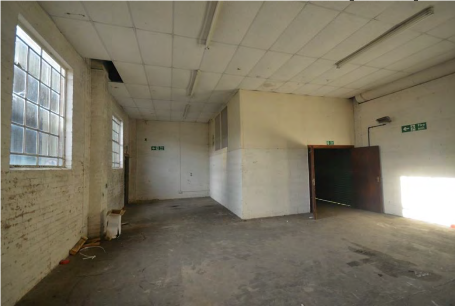
Plate 79: Transport Building room 9 looking North-west
