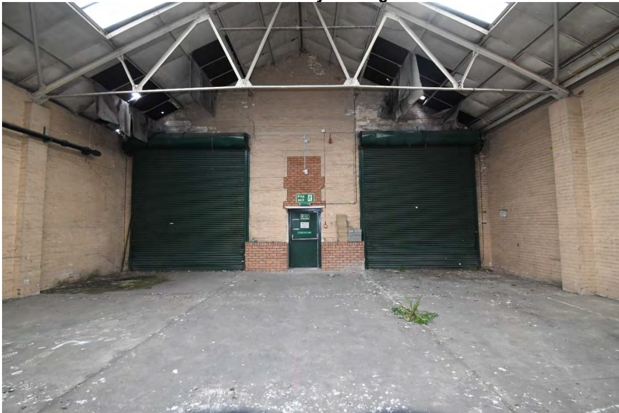
Plate 83: Detail of Warehouse interior northeast wall
