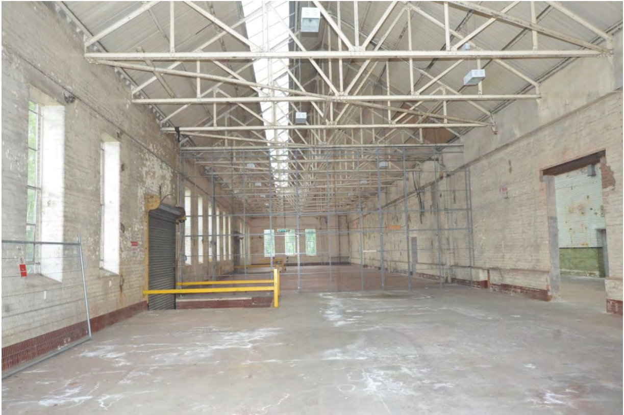
Plate 25: Room 6 goods in looking Southeast
