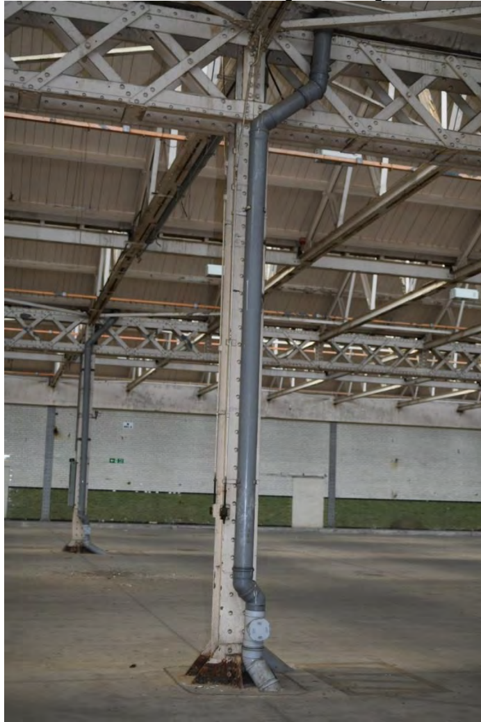
Plate 23: Supporting column, room 4, main manufactory area
