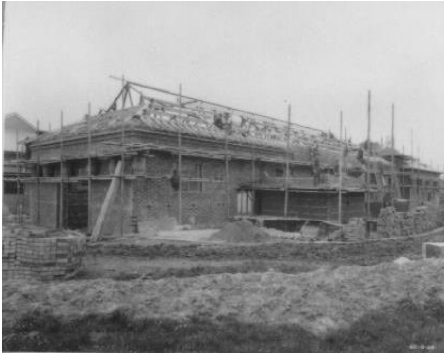
Plate 72: Boiler house and power house under construction, 1920s (Blue Bird Album)
