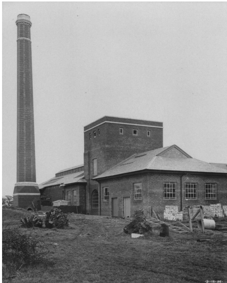
Plate 71: Boiler house and power house, 1926 (Blue Bird Album)
