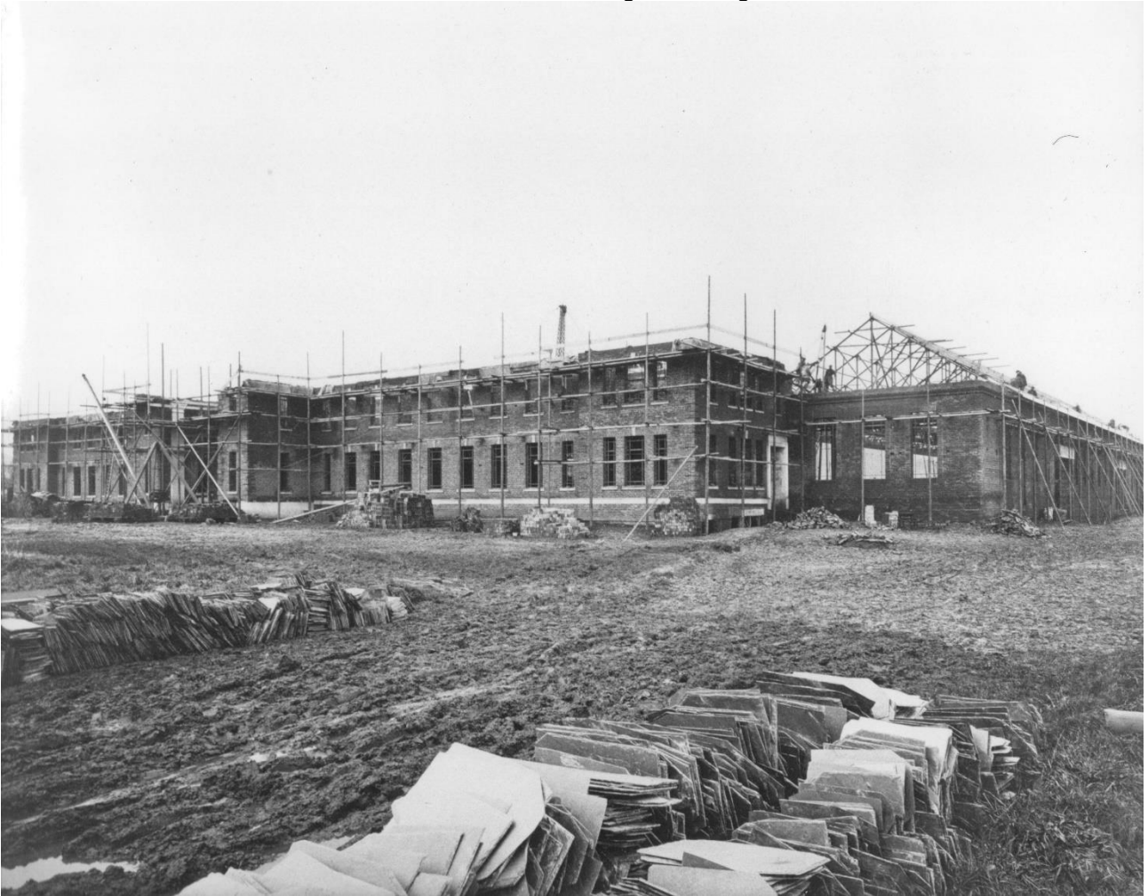
Plate 30: Admin & manufactory buildings under construction (Blue Bird Album)
