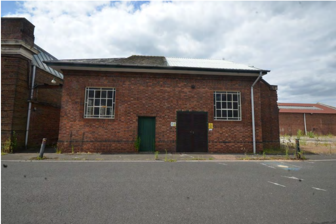
Plate 70: South-east elevation, power house
