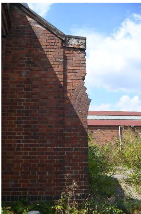
Plate 75: Stub of North-west wall of boiler house, showing start of arch
