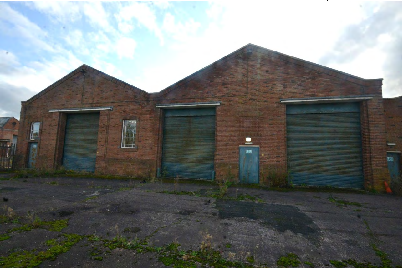
Plate 80: Building 9 Warehouse looking North-east
