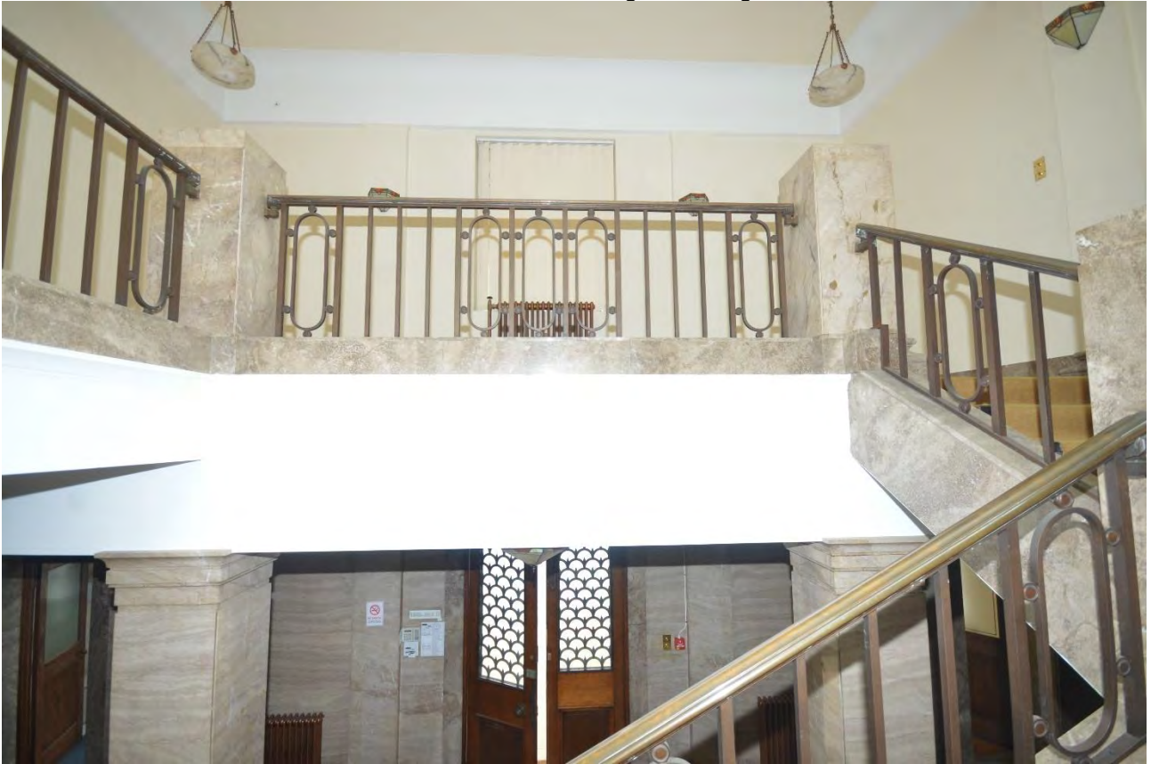
Plate 36: The central stairs at first floor level
