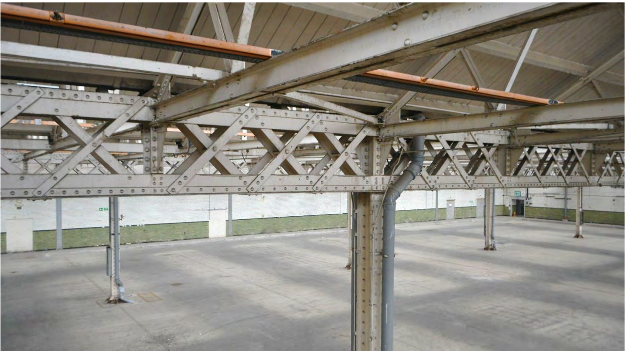
Plate 22: Elevated view of roof structure, room 4, main manufactory area
