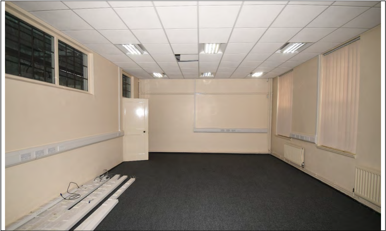
Plate 52: Ground Floor Room 7 Looking Northeast
