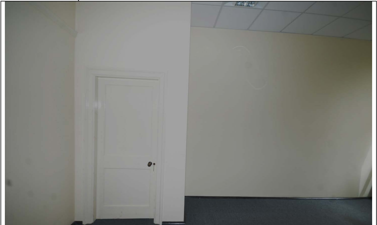
Plate 71: Ground Floor Room 12 Looking Northeast
