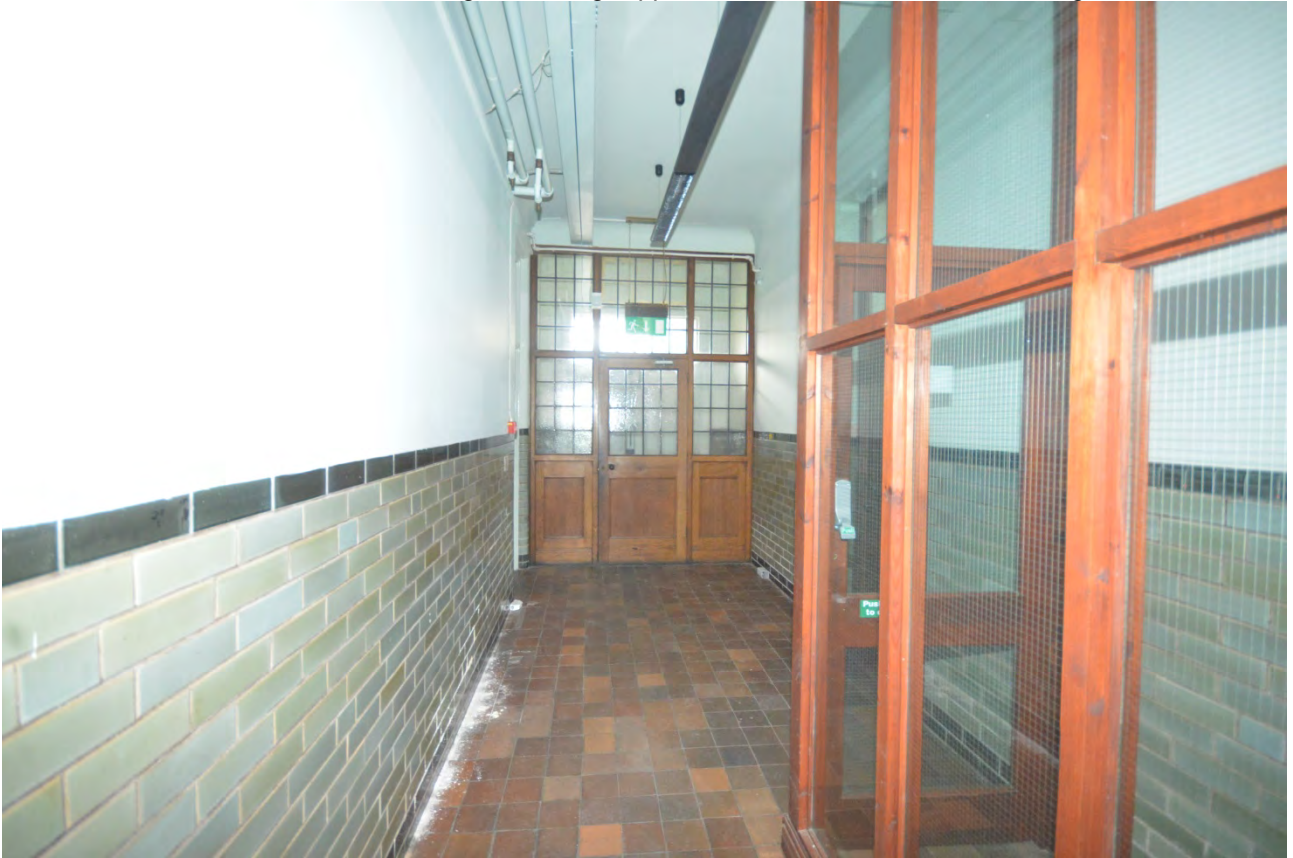
Plate 41: Partition at southwest end of corridor
