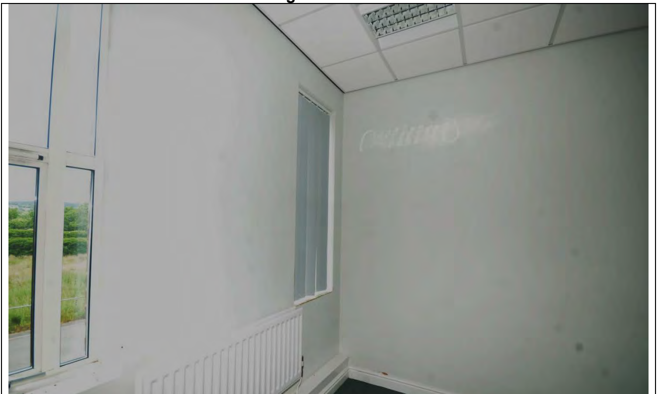
Plate 105: First Floor Room 5 Looking Northwest
