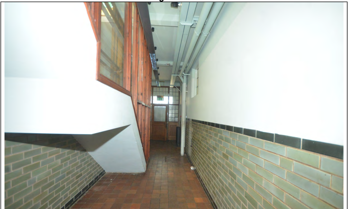
Plate 40: Staircase at northeast end of corridor
