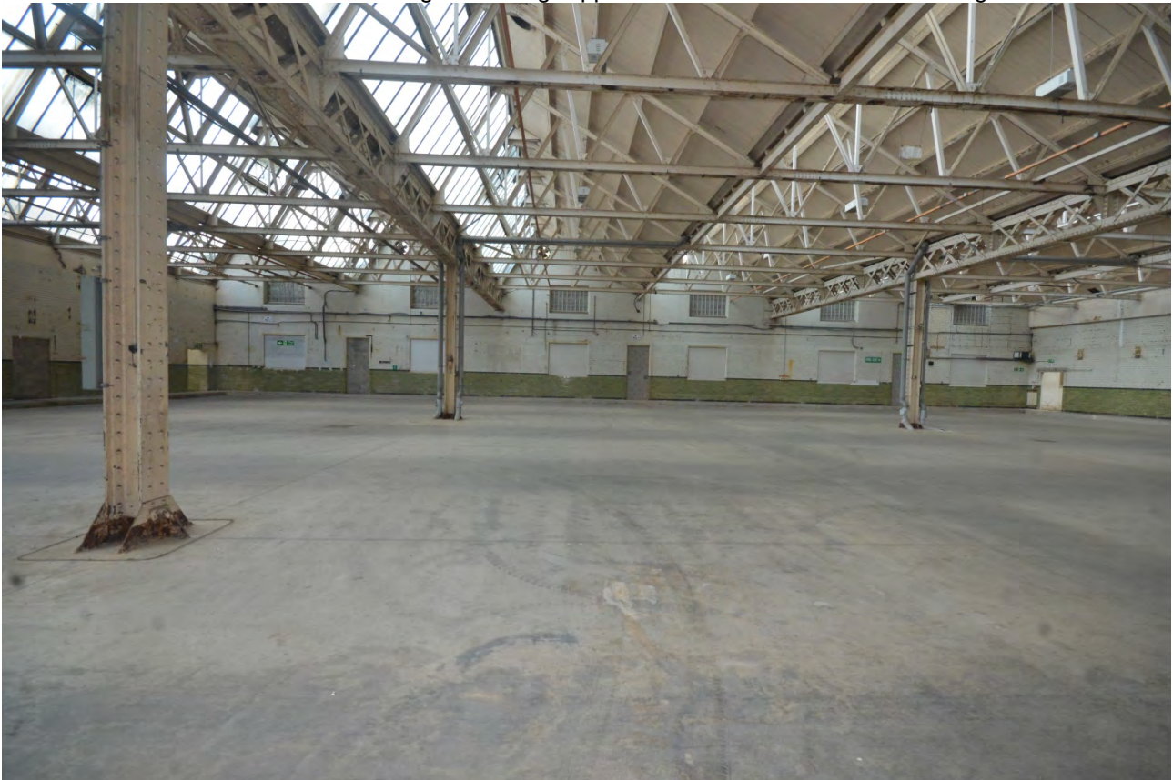
: Blocked windows and doorways to administration building in southeast wall of manufactory room 4
