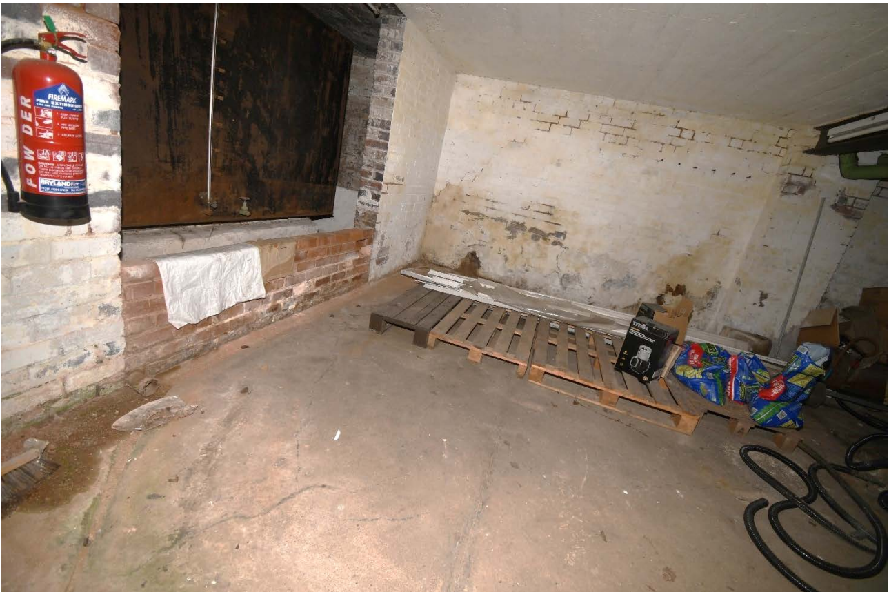
Plate 157: Plant Room Looking Southwest
