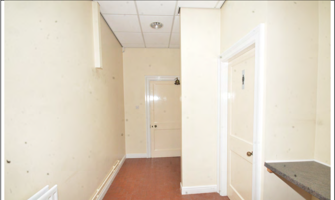
Plate 97: First Floor Room 4 Looking Northeast
