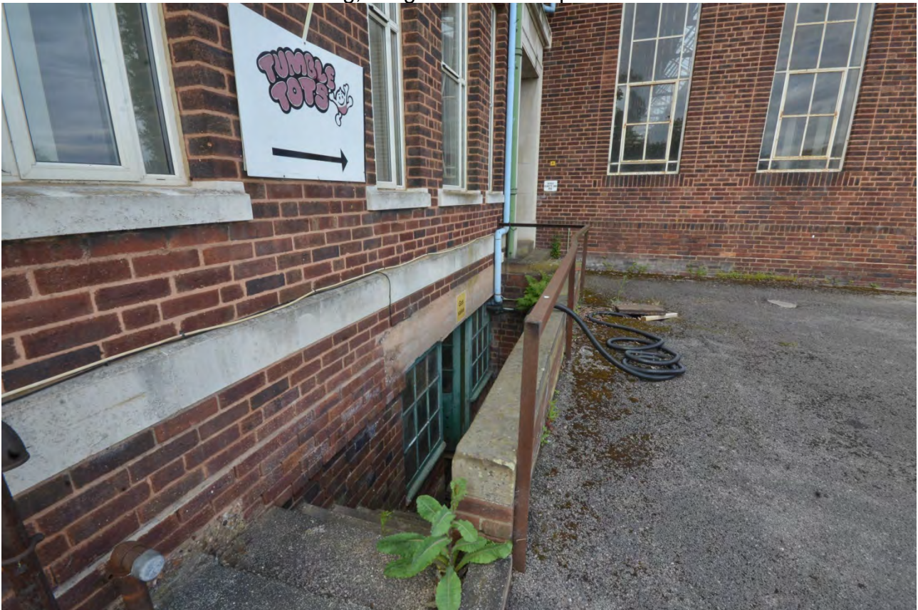
Plate 27: Staircase to basement / plant room
