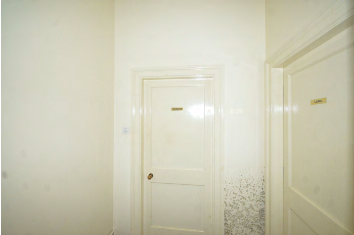
Plate 42: Ground Floor Room 3 Looking Southeast
