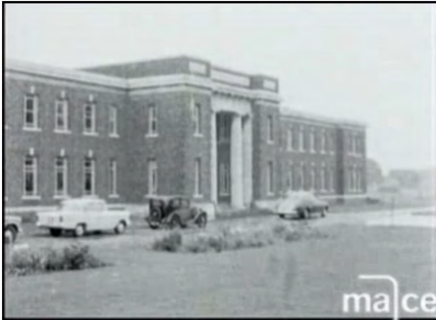
Plate 6: The administration building in 1958
