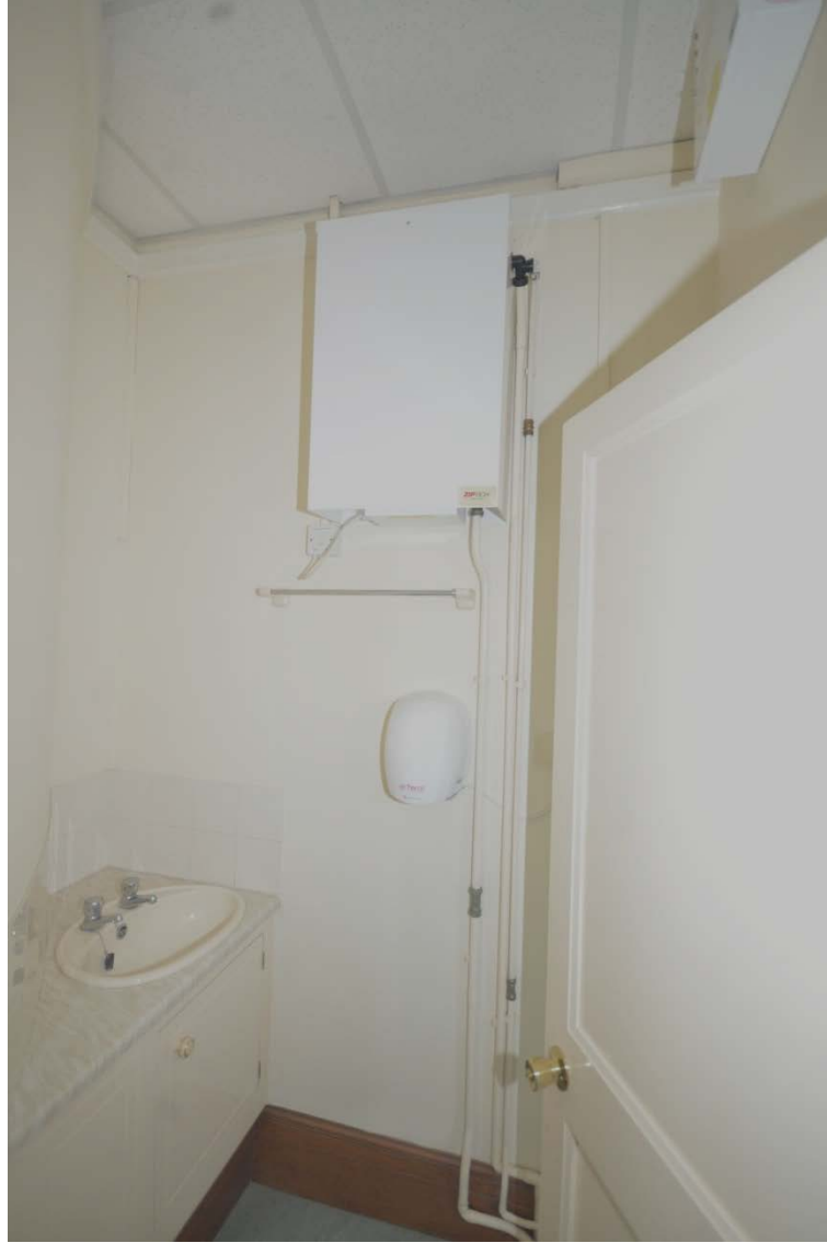
Plate 135: First Floor Room 14 Looking Northwest
