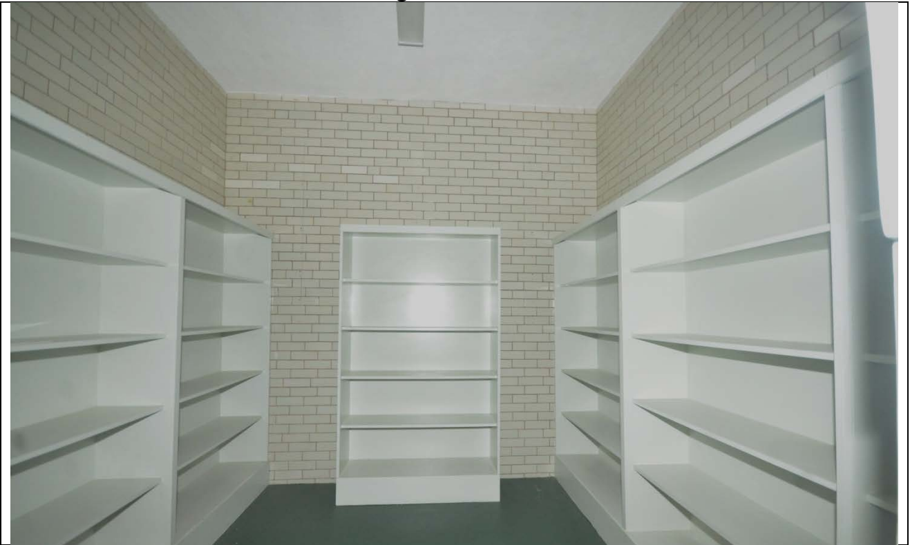
Plate 108: First Floor Room 6 Looking Southwest
