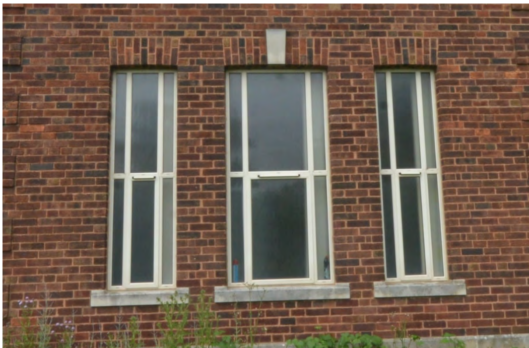
Plate 14: Detail of windows
