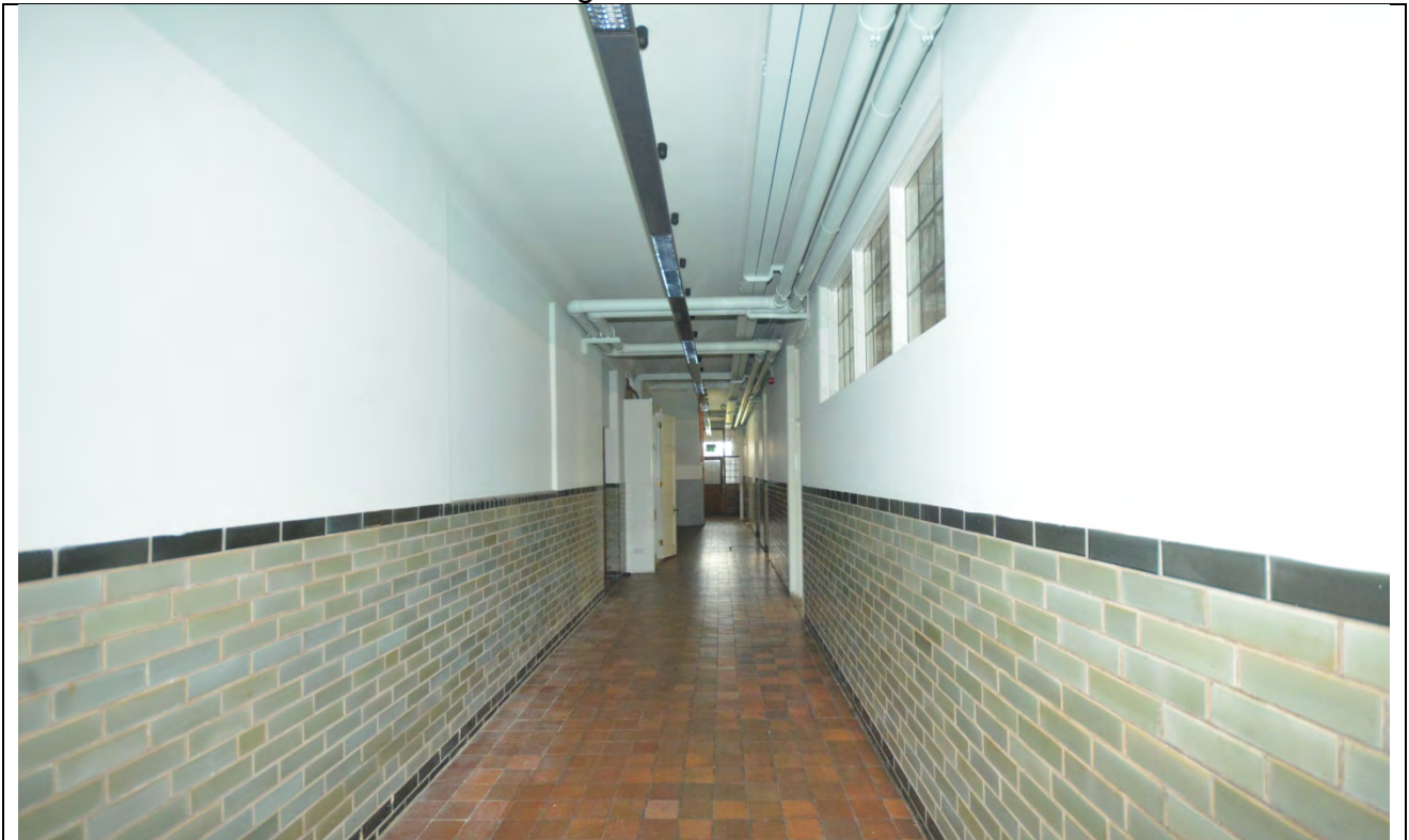
Plate 38: Ground Floor Room 2 Looking Northeast
