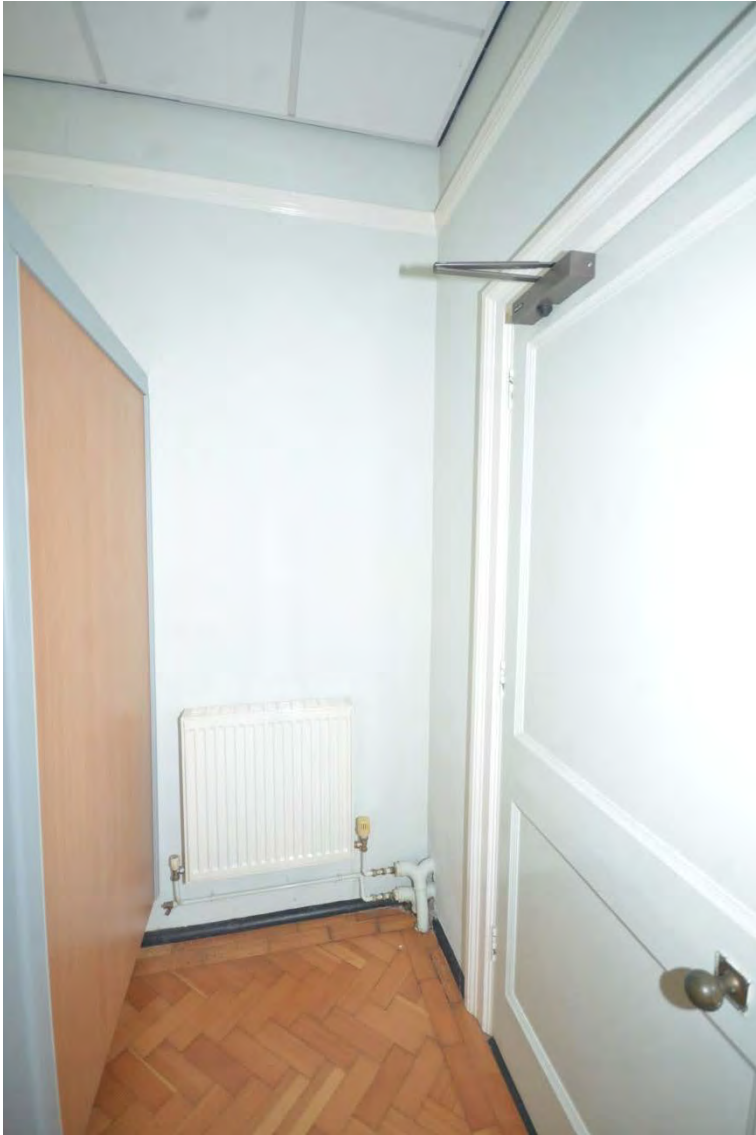
Plate 124: First Floor Room 11 Looking Southwest
