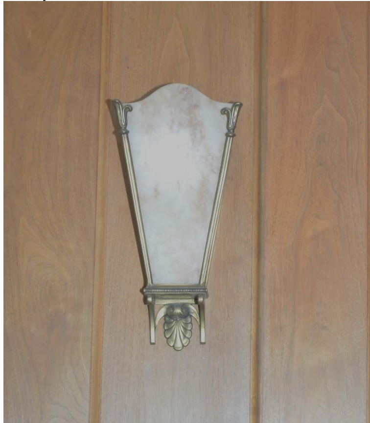
Plate 153: Detail of wall light
