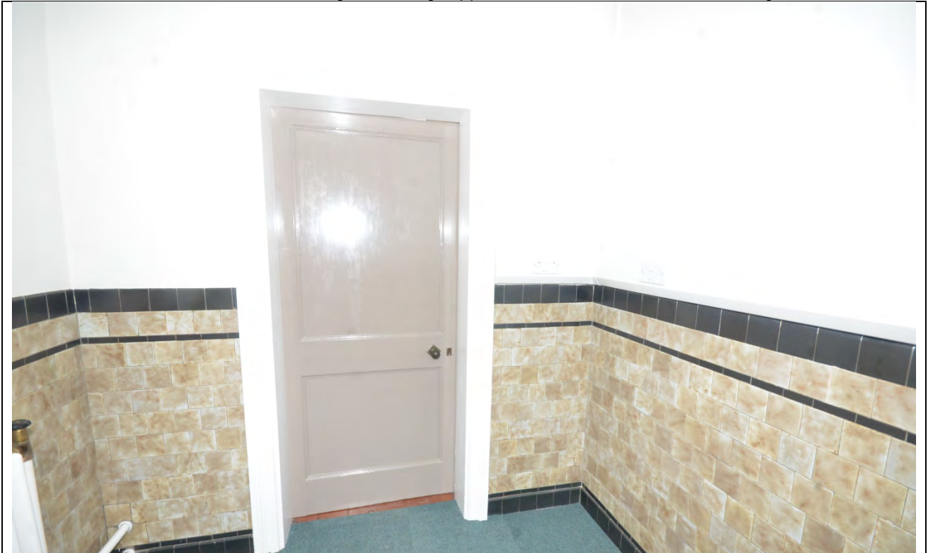
Plate 95: First Floor Room 3 Southwest Door
