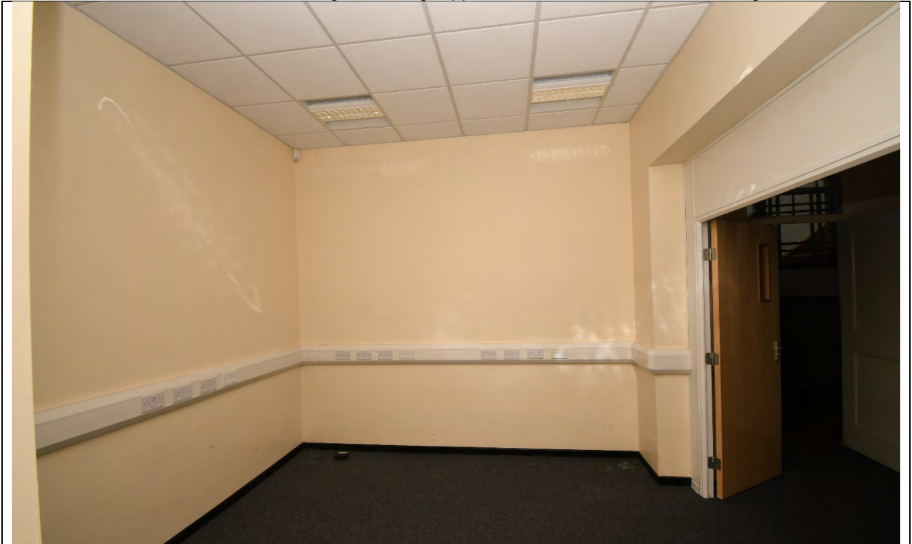
Plate 51: Ground Floor Room 6 Looking Northwest
