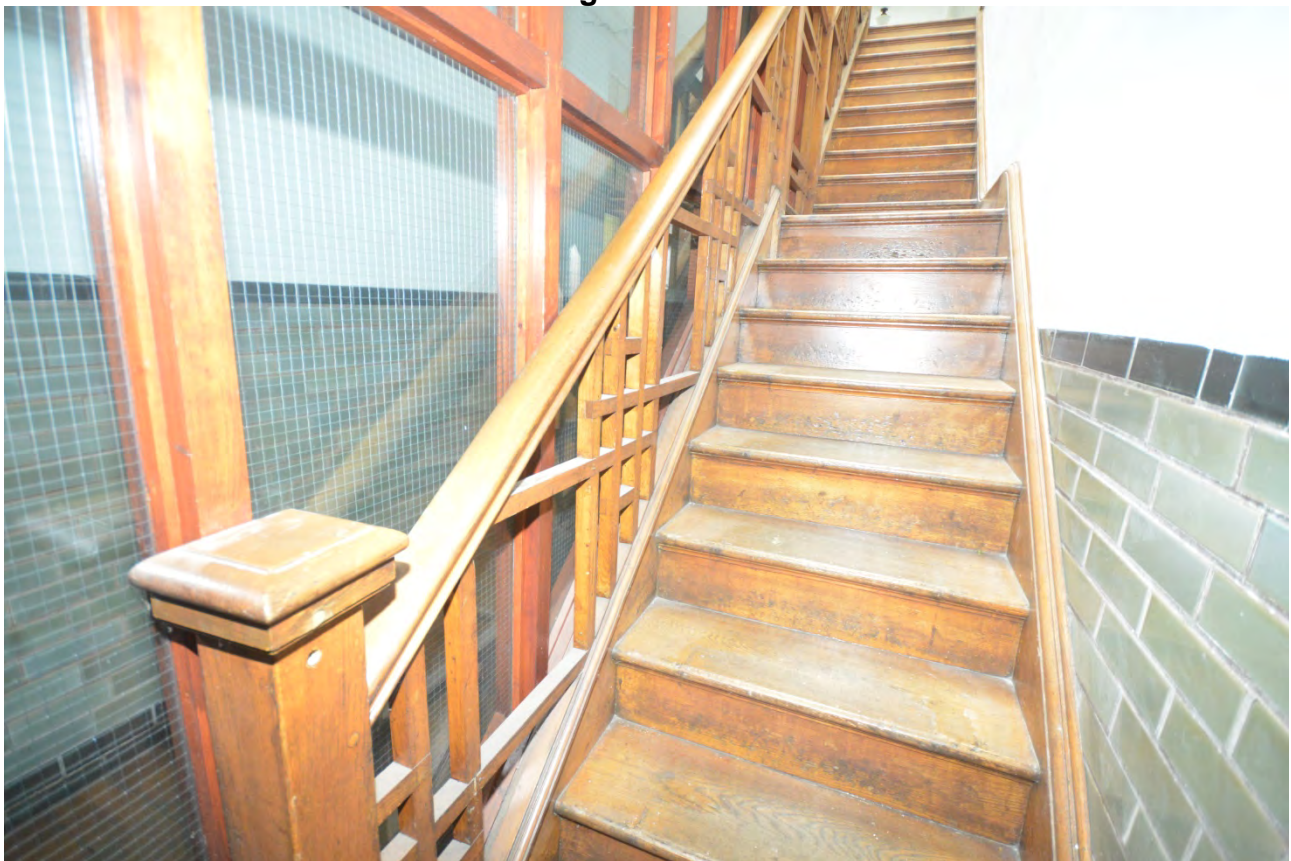
Plate 128: Detail of staircase
