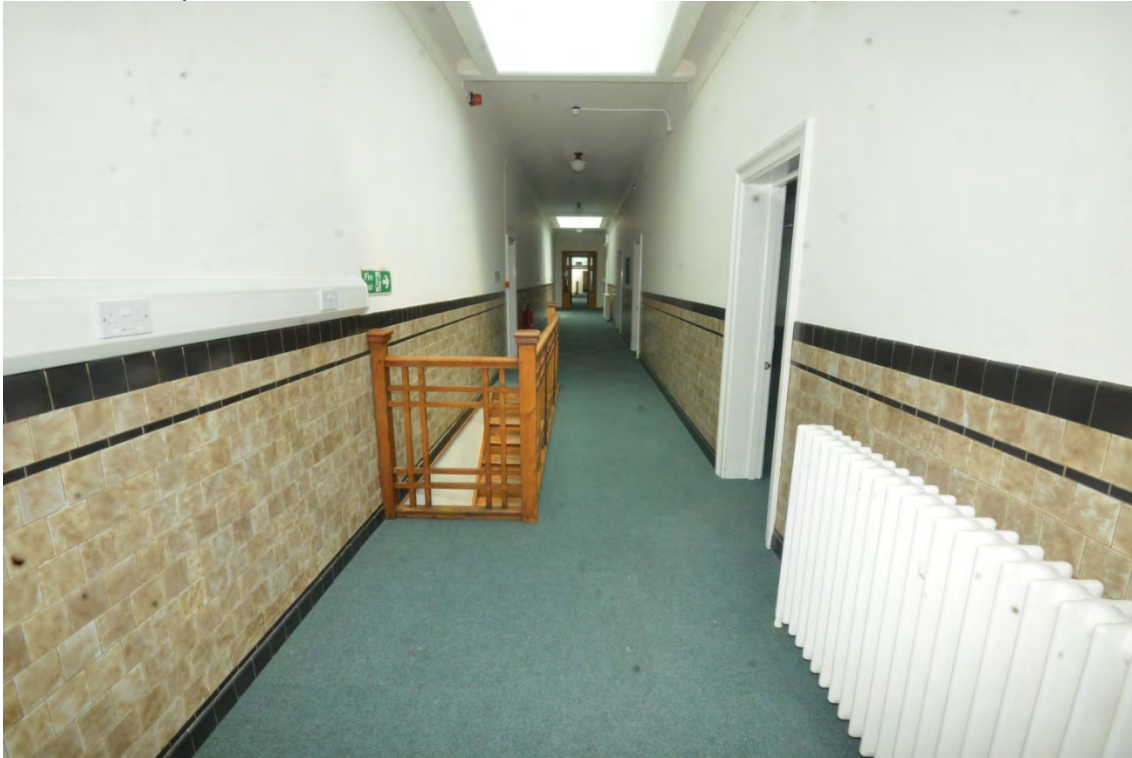
Plate 93: First Floor Room 3 Looking Northeast
