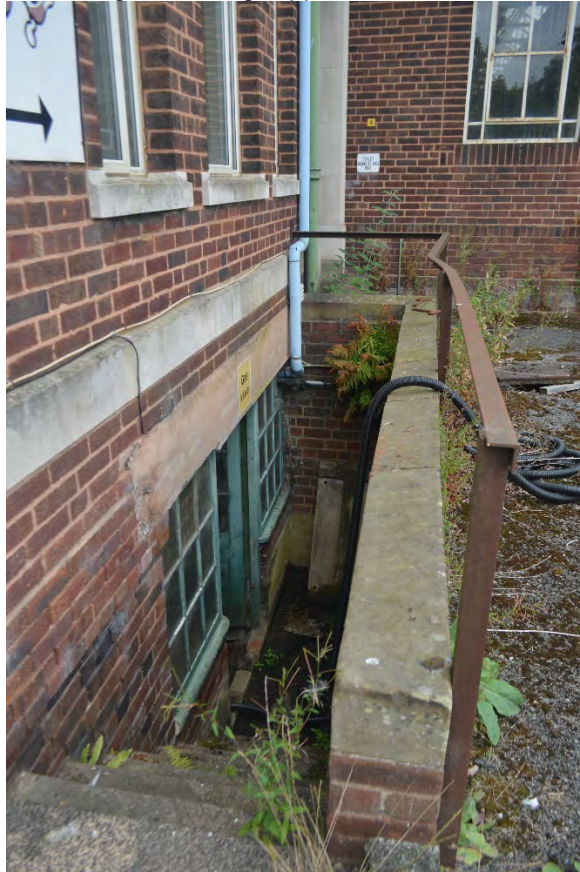
Plate 28: Staircase to basement / plant room
