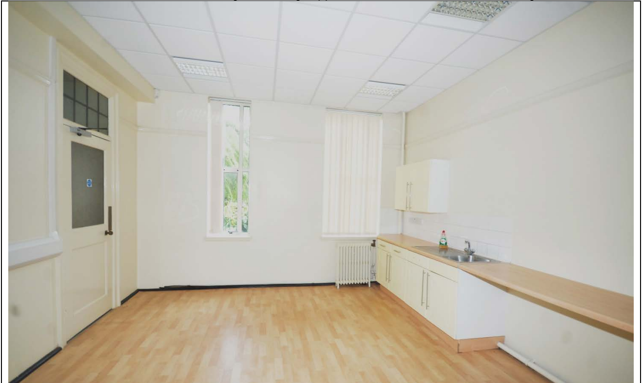
Plate 61: Ground Floor Room 9 Looking Southeast
