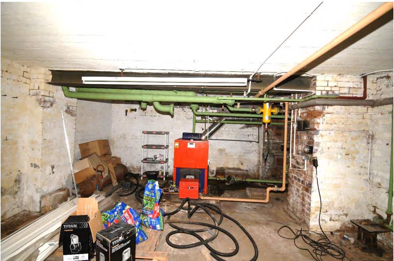
Plate 158: Plant Room Looking Northwest
