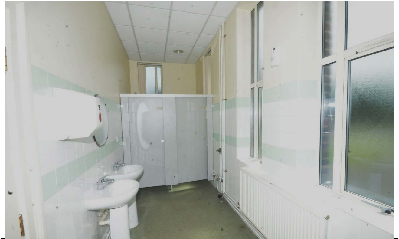
Plate 45: Ground Floor Room 4 Looking Southeast
