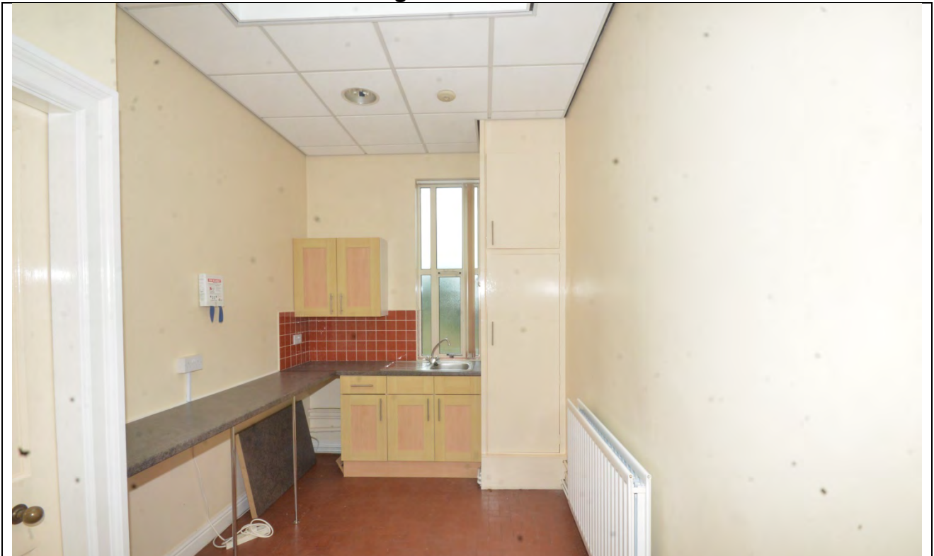
Plate 98: First Floor Room 4 Looking Southwest
