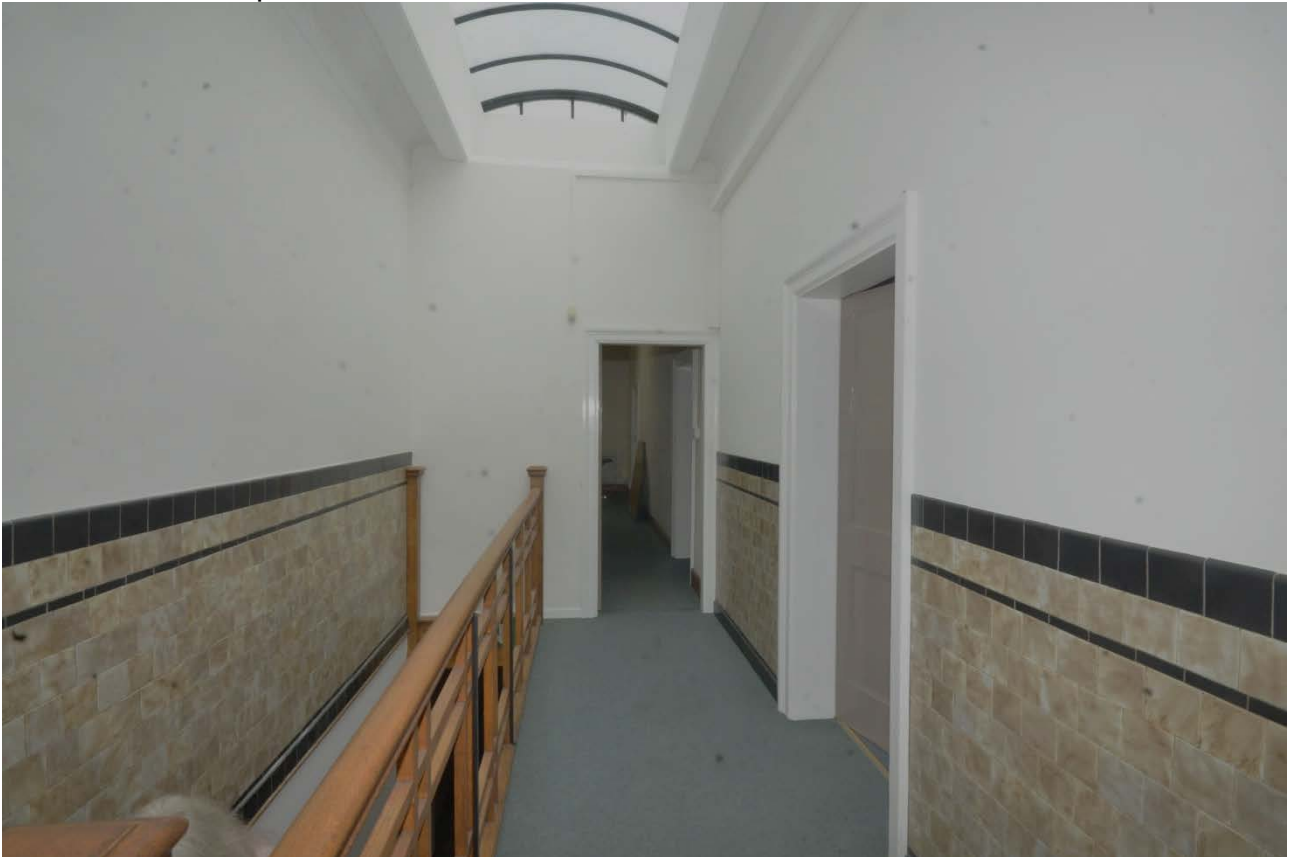
Plate 126: First Floor Room 12 Looking Northeast
