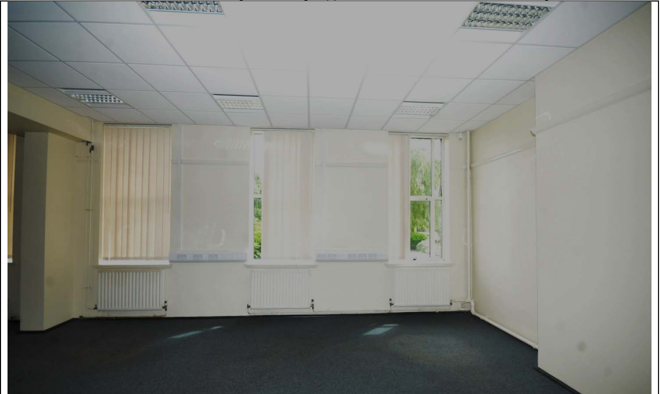
Plate 79: Ground Floor Room 14 Looking Southeast
