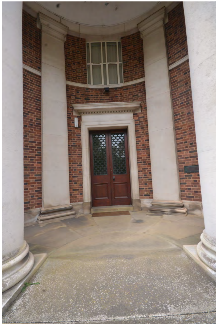
Plate 17: Detail of central entrance, southeast elevation
