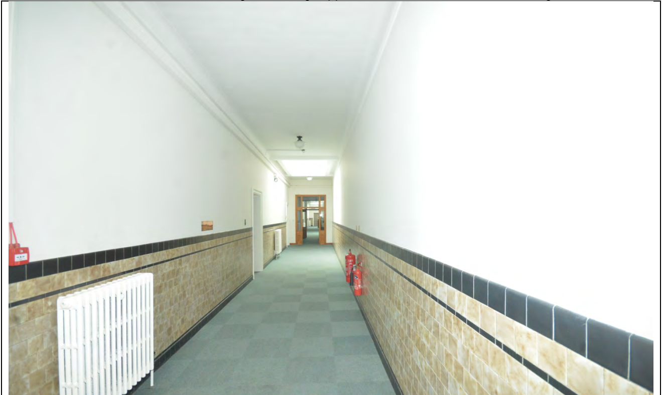
Plate 127: First Floor Room 12 Looking Southwest
