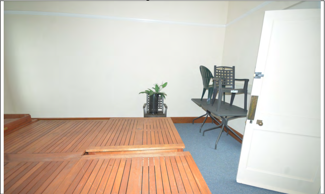
Plate 143: First Floor Room 16 Looking Southwest
