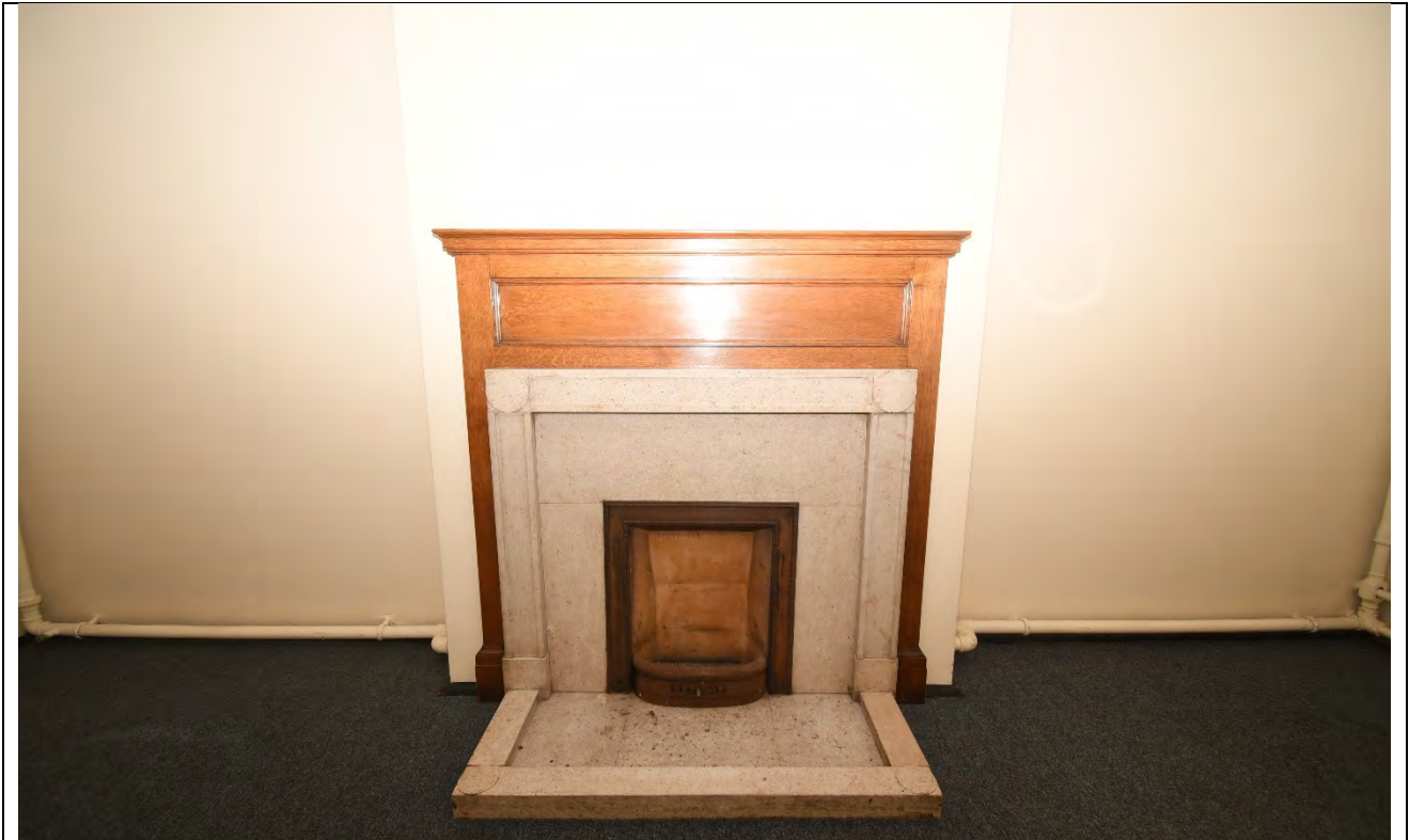
Plate 75: Ground Floor Room 13 Looking Northeast
