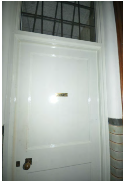
Plate 44: Ground Floor Room 3 Looking Northwest
