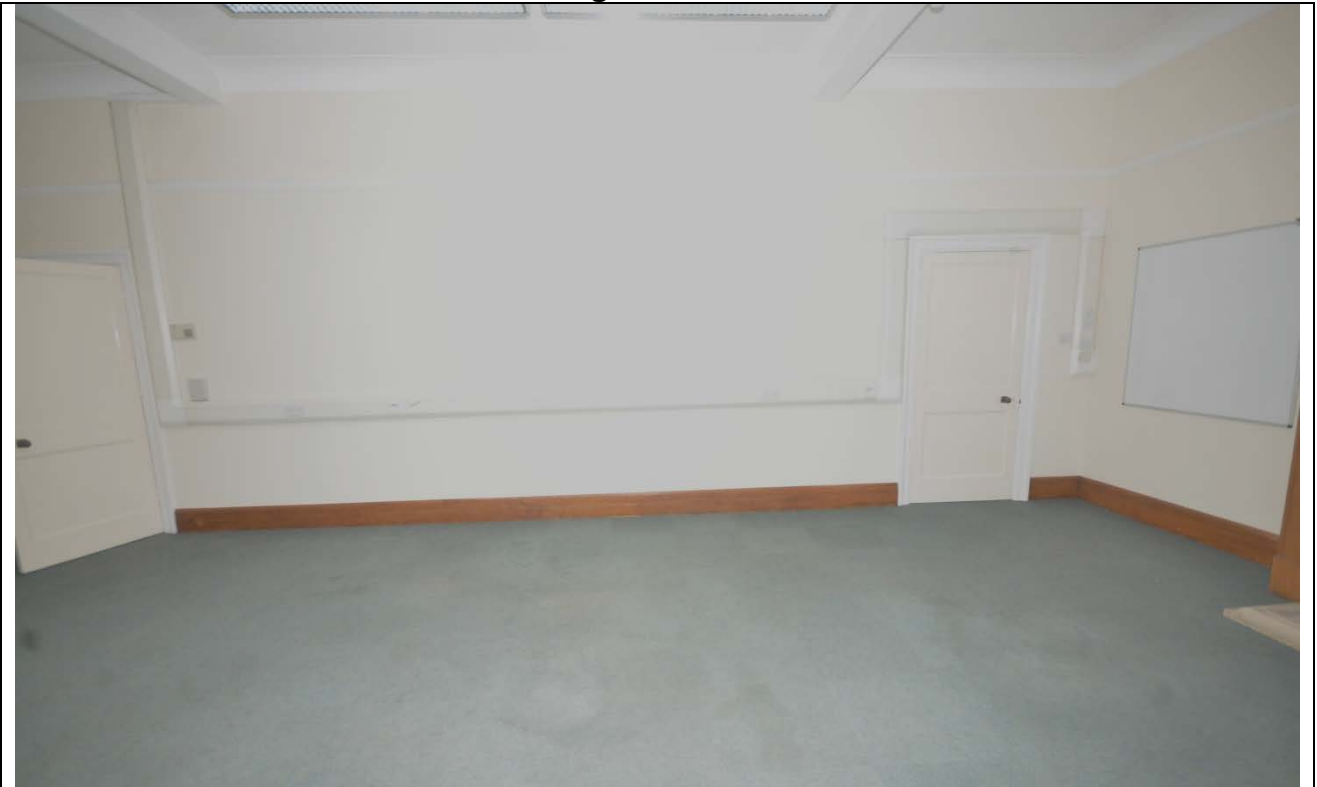
Plate 132: First Floor Room 13 Looking Northwest
