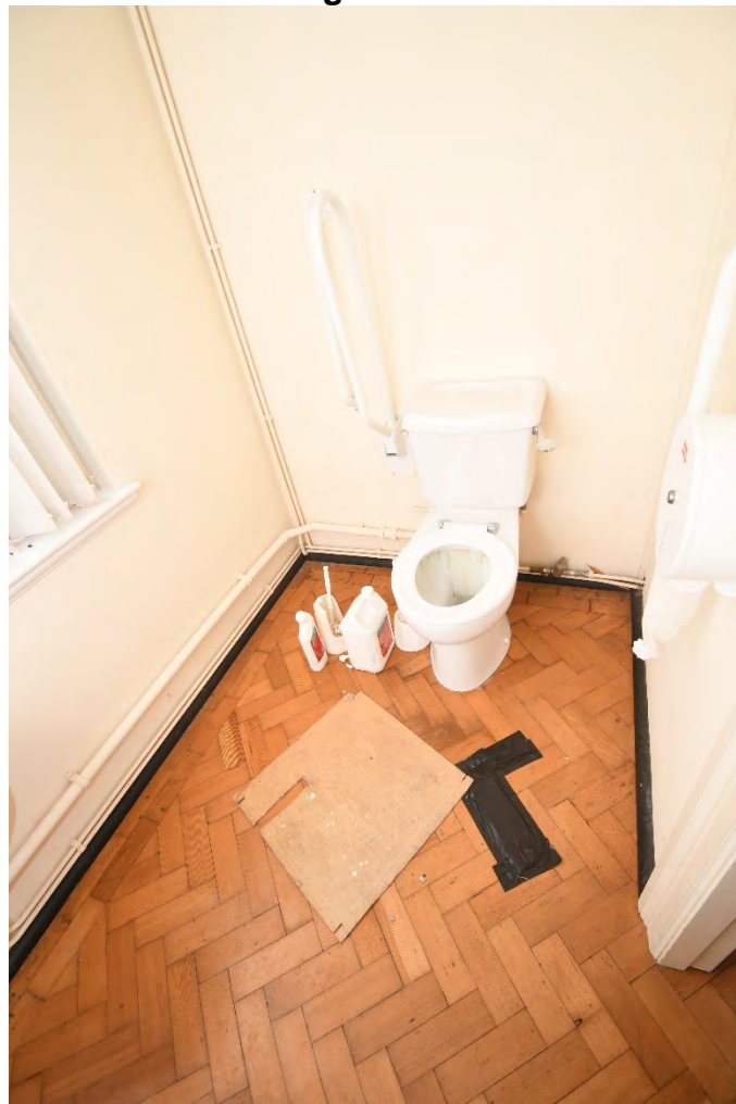
Plate 66: Ground Floor Room 10 looking Southwest
