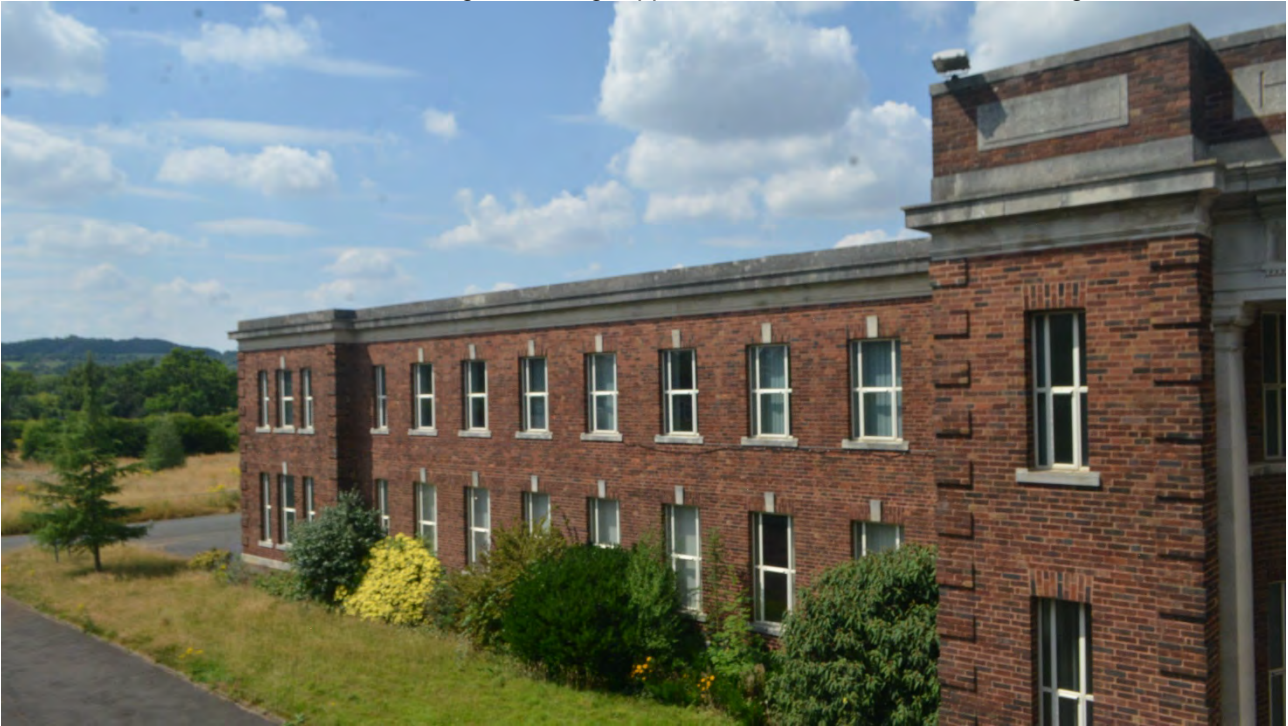
Plate 20: Elevated view, façade, southwest wing
