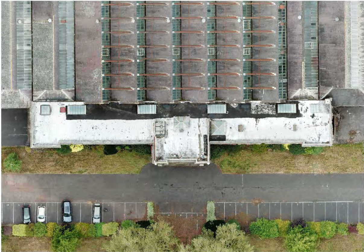
Plate 32: Aerial image of the administration building (commissioned for this exercise, September 2022)
