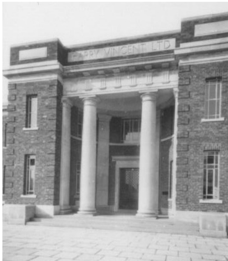
Figure 13: The entrance after completion (Romsley & Hunnington His Soc)
