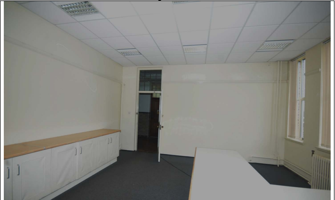
Plate 85: Ground Floor Room 15 Looking Northwest
