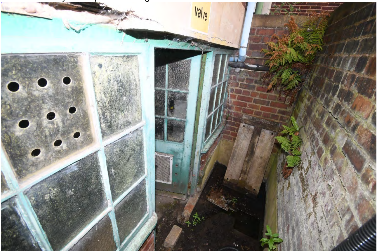
Plate 29: Exterior of plant room / basement
