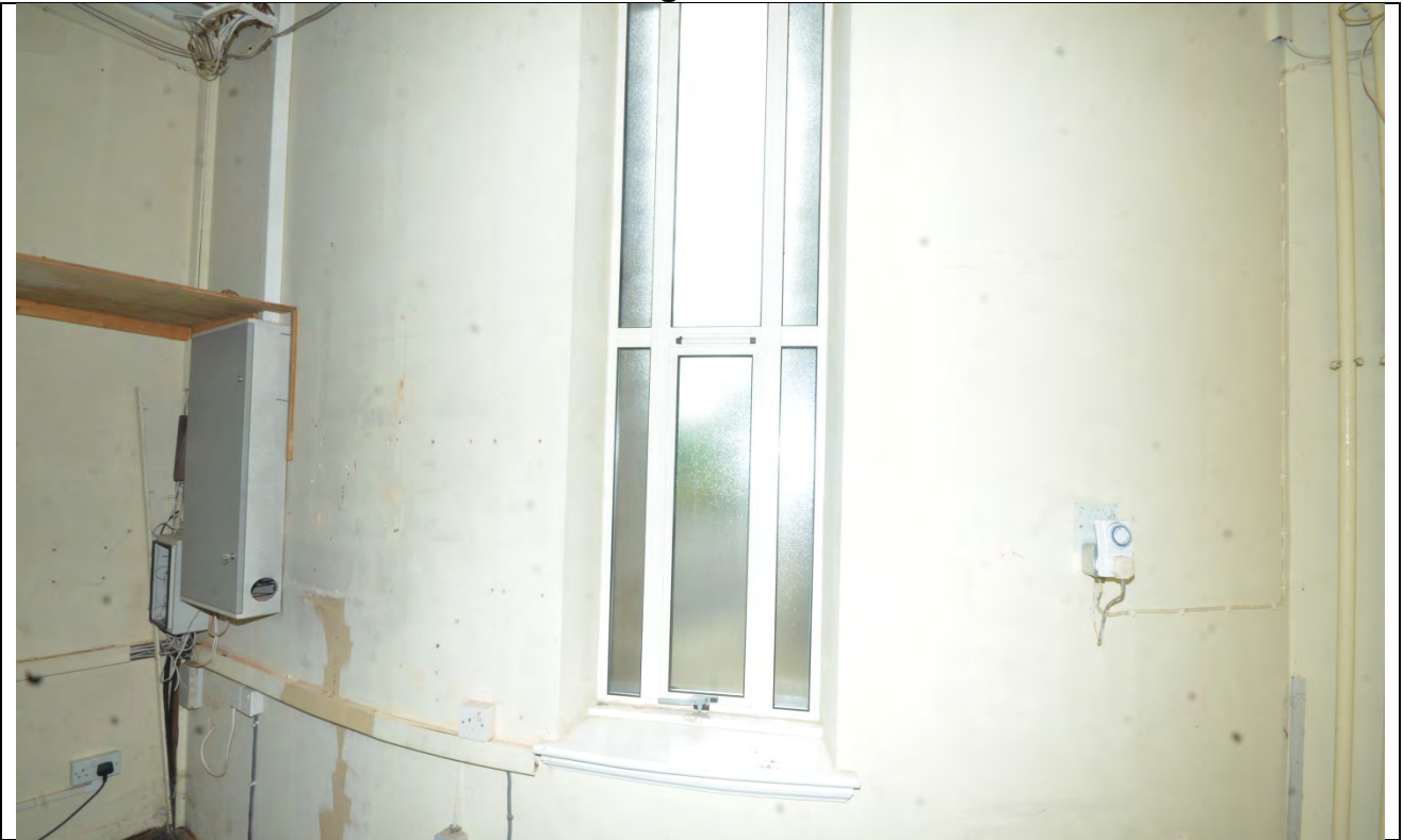
Plate 69: Ground Floor Room 11 Looking Southwest
