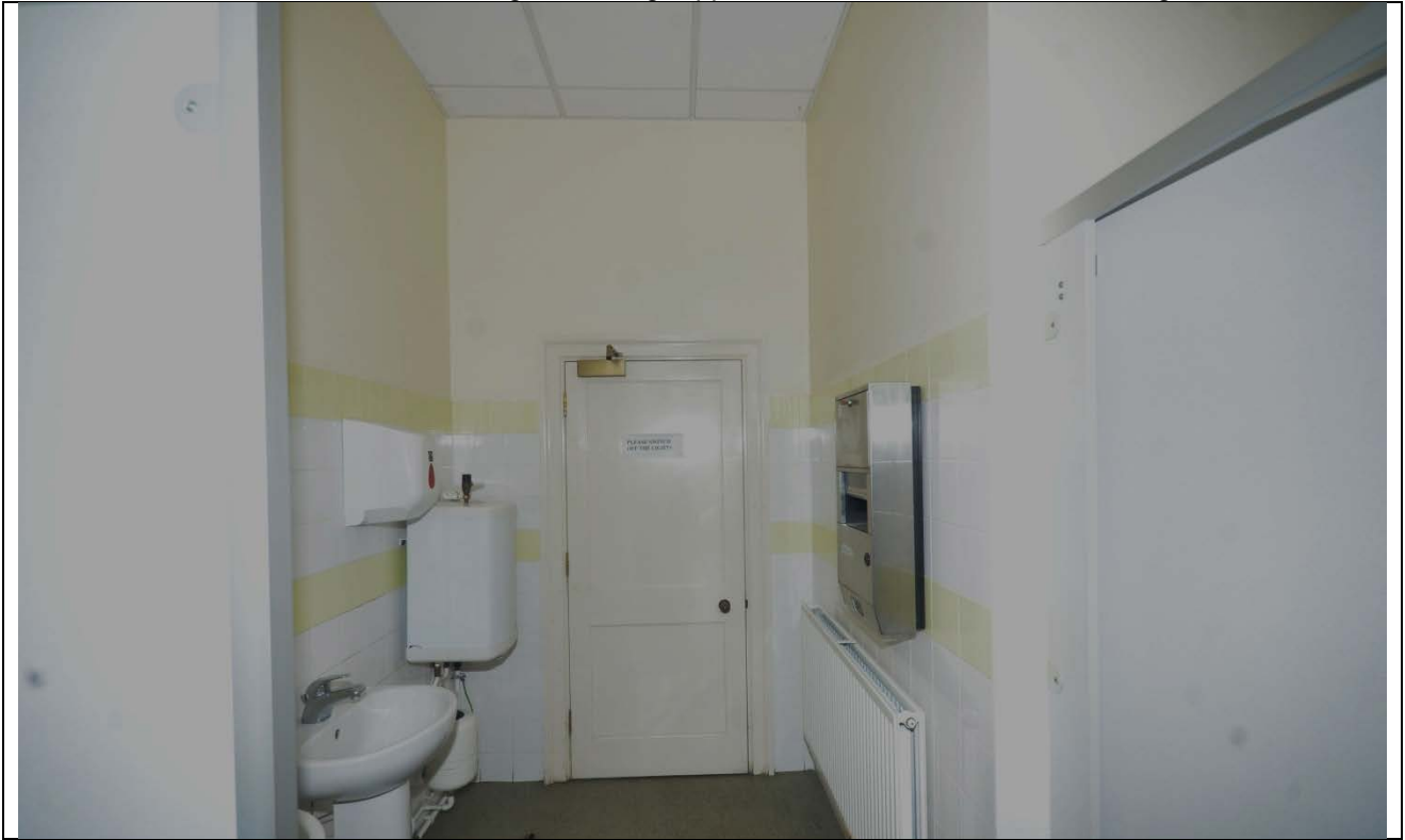
Plate 49: Ground Floor Room 5 Looking Northwest
