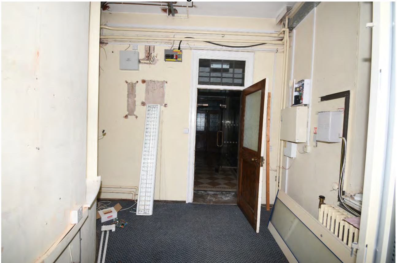
Plate 70: Ground Floor Room 11 Looking Northwest
