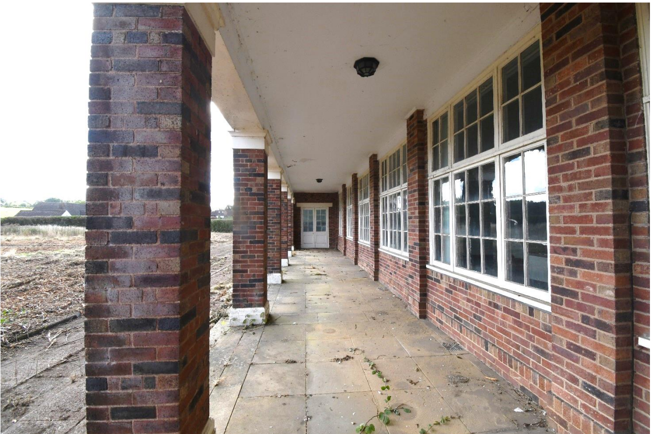
Plate 16: View to southwest along northeast veranda
