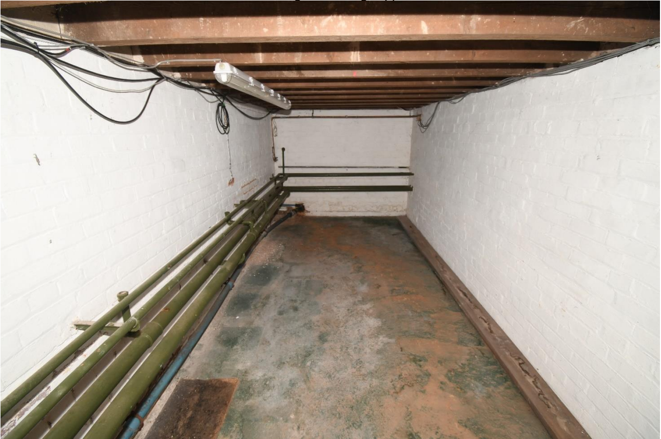
Plate 141: Bay 1 looking northeast
