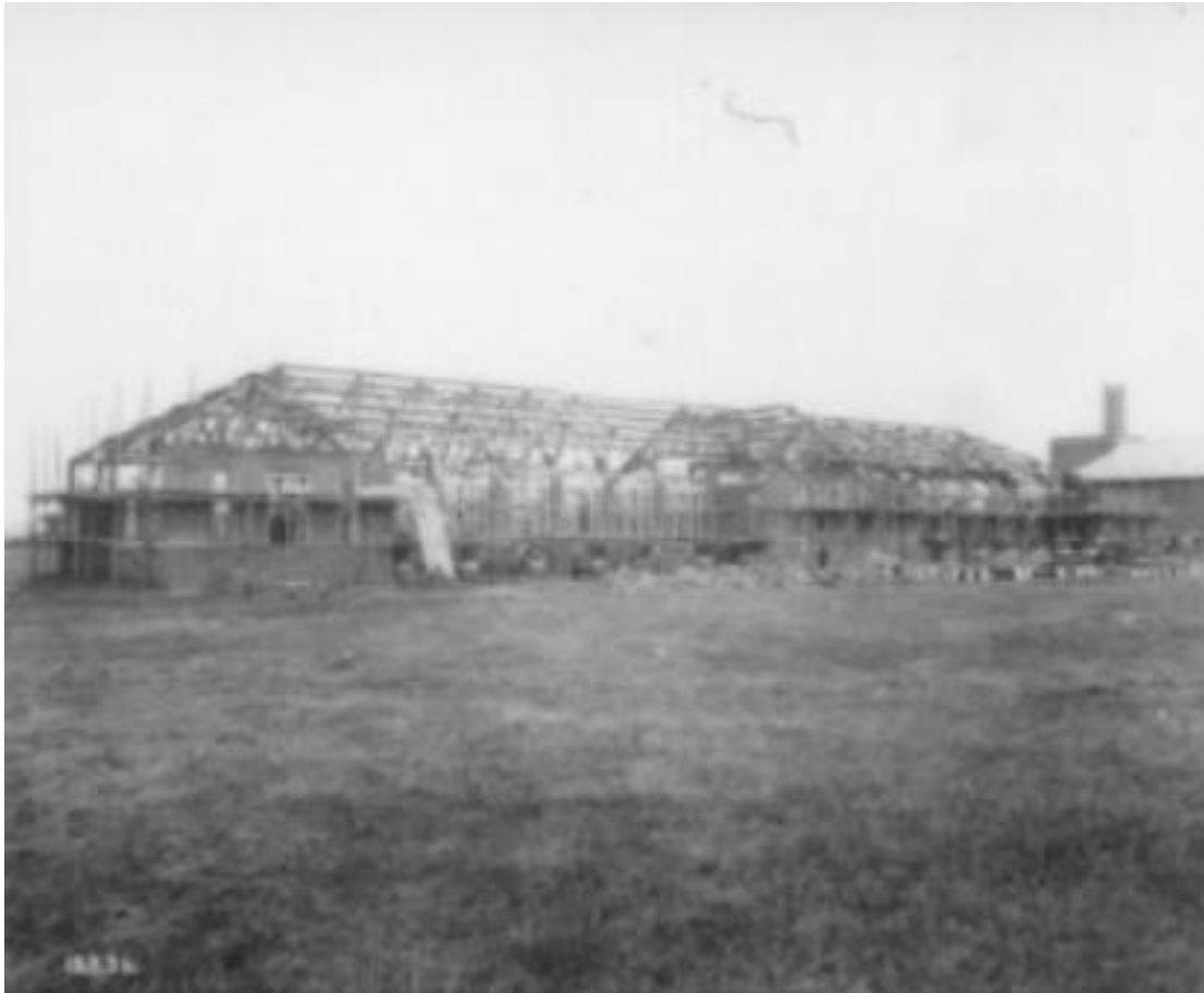
Plate 6: The canteen under construction (Blue Bird Album, Romsley & Hunnington History Society)
