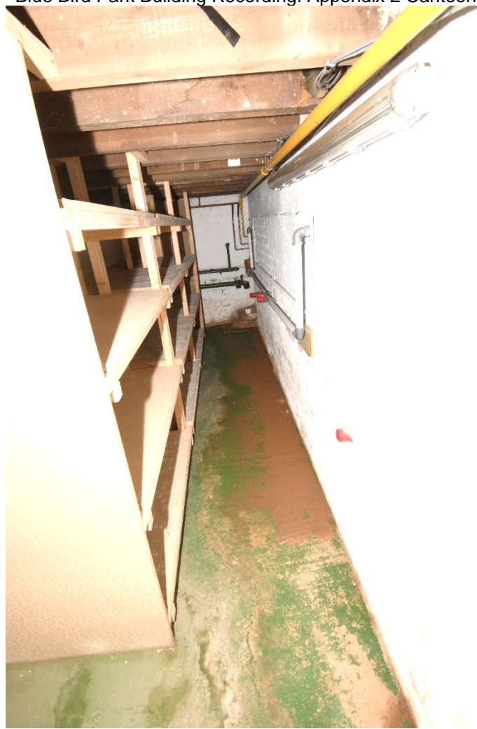
Plate 145: Bay 5 looking northeast
