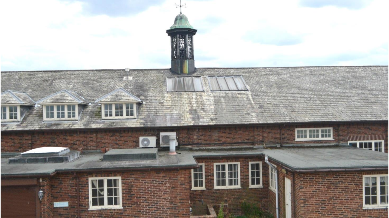
Plate 23: Elevated view of rear elevation
