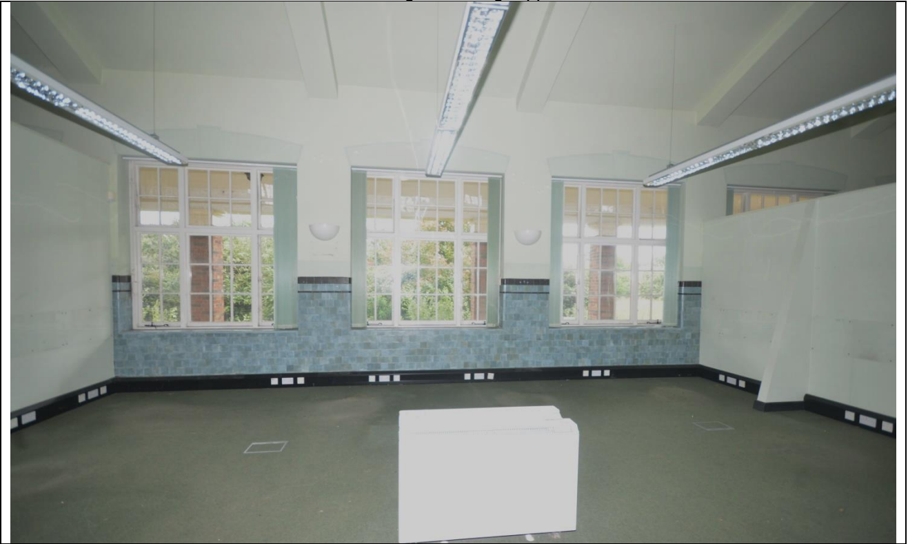
Plate 114: Room 27 Looking Southeast (central part)
