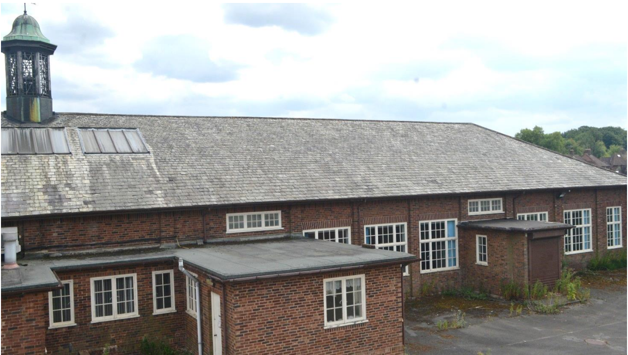
Plate 24: Elevated view of rear elevation
