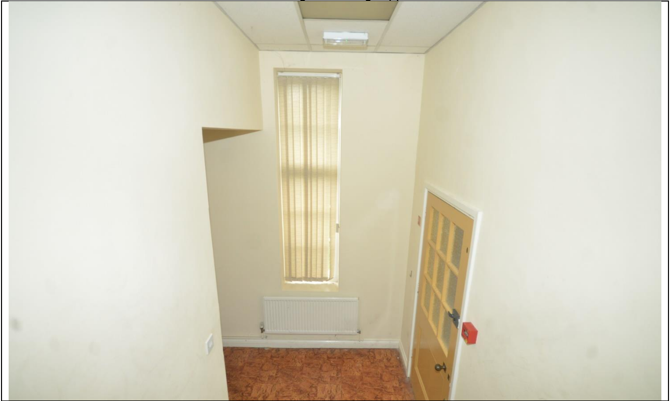
Plate 138: Room 34 Looking Southeast
