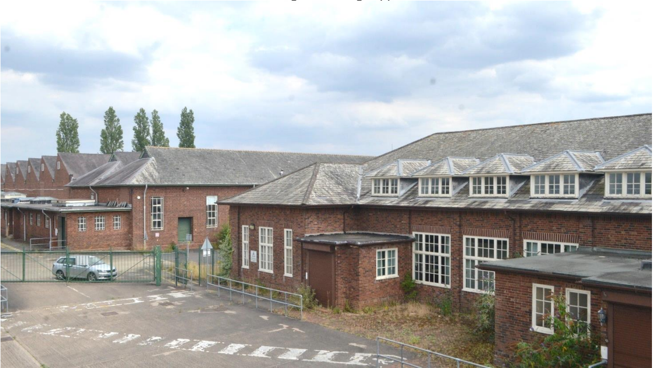
Plate 21: Elevated view of rear elevation
