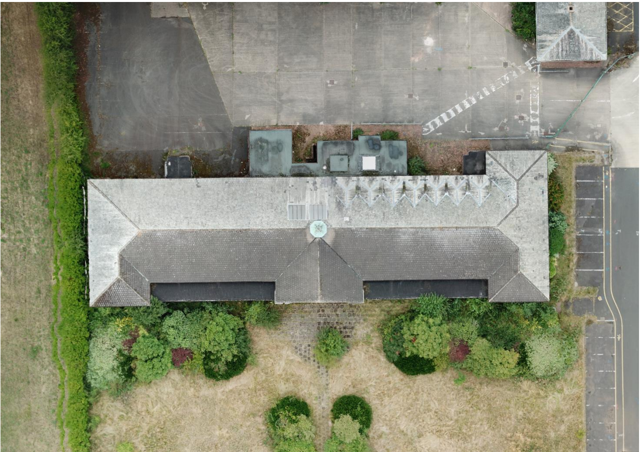
Plate 26: Aerial image of the canteen building
