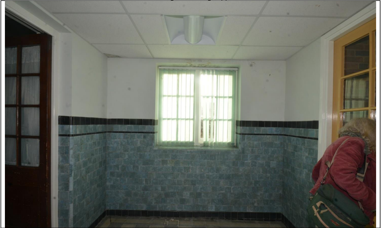
Plate 123: Room 28 Looking Southwest
