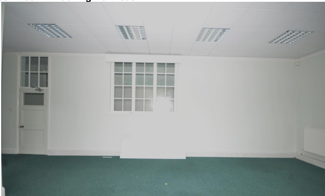
Plate 37: Room 4 Looking Southeast
