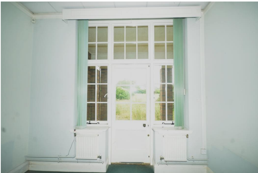
Plate 76: Room 16 Looking Southeast
