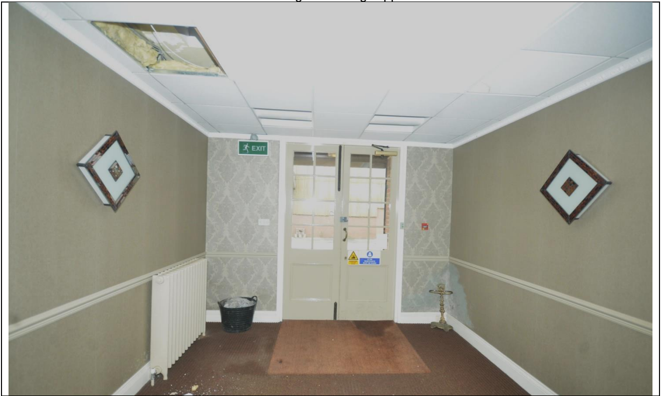
Plate 30: Room 1 Looking Northwest
