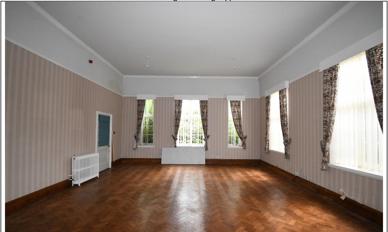
Plate 54: Room 8 Looking Southeast
