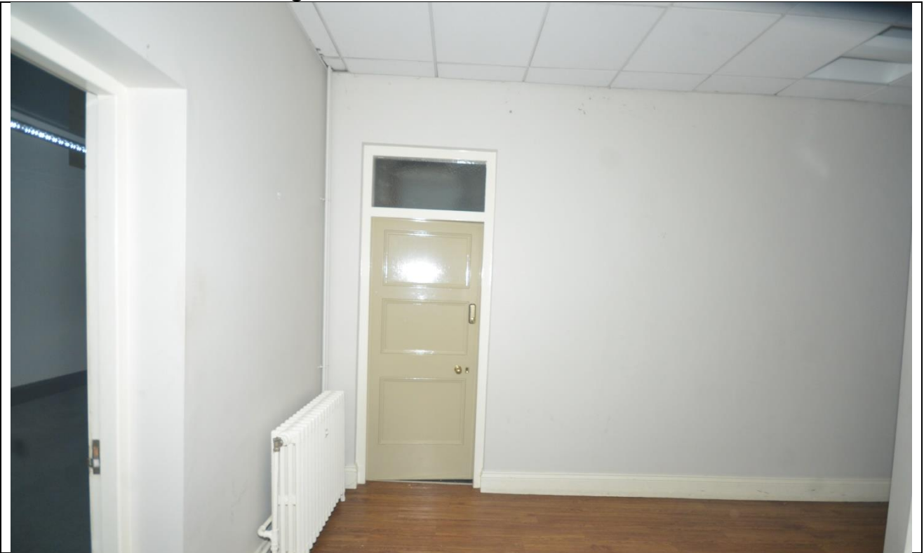
Plate 82: Room 17 Looking Northwest
