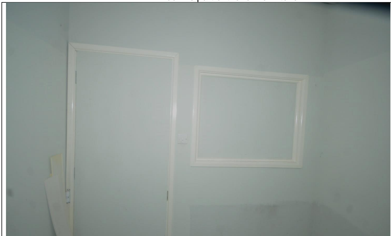
Plate 92: Room 20 Looking Southeast, showing blocked door and window
