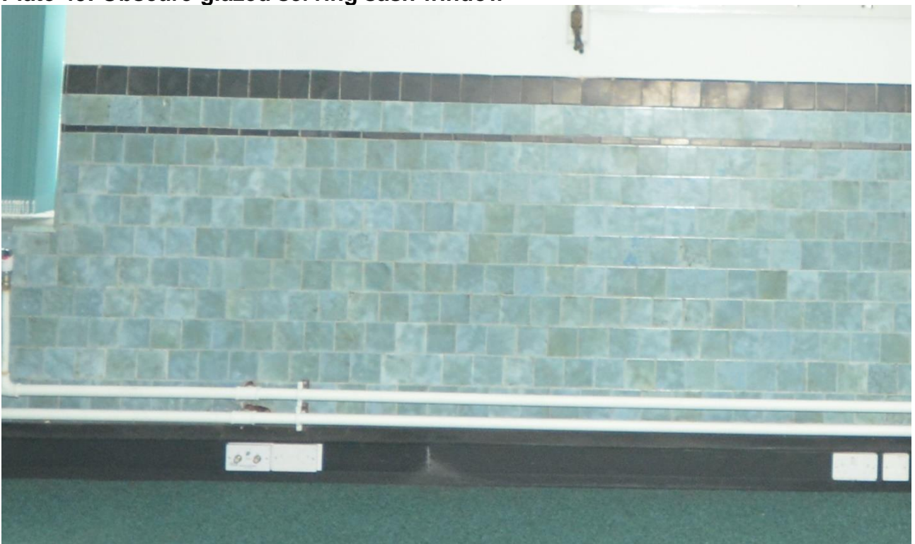
Plate 46: Detail of tiles
