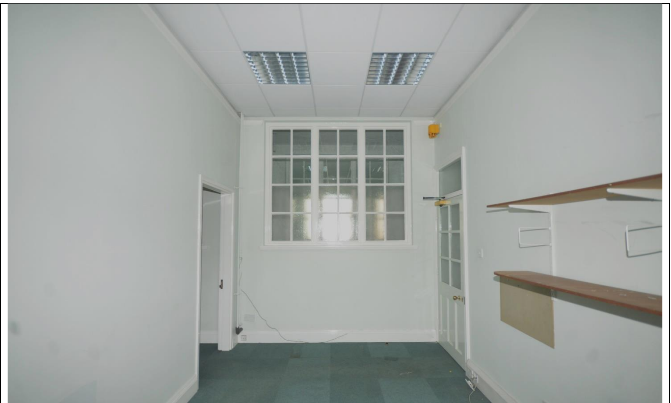
Plate 71: Room 13 Looking Northwest
