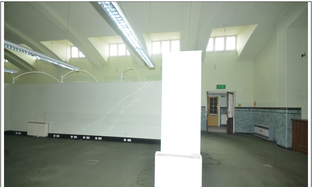
Plate 119: Room 27 Looking Northwest
