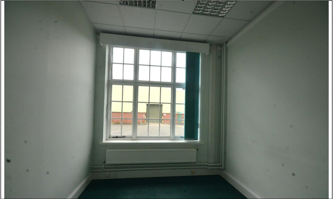
Plate 35: Room 3 Looking Northwest
