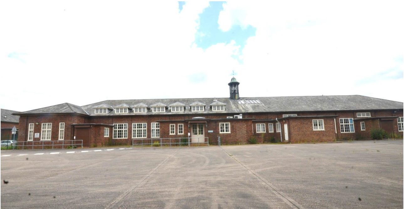
Plate 7: The rear of the building
