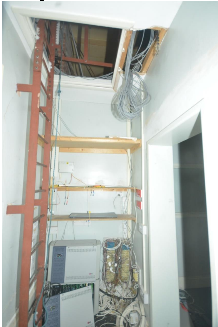
Plate 96: Ladder to roof space
