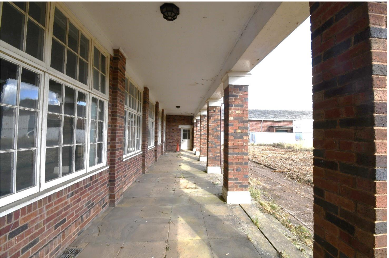
Plate 17: View to southwest along southwest veranda
