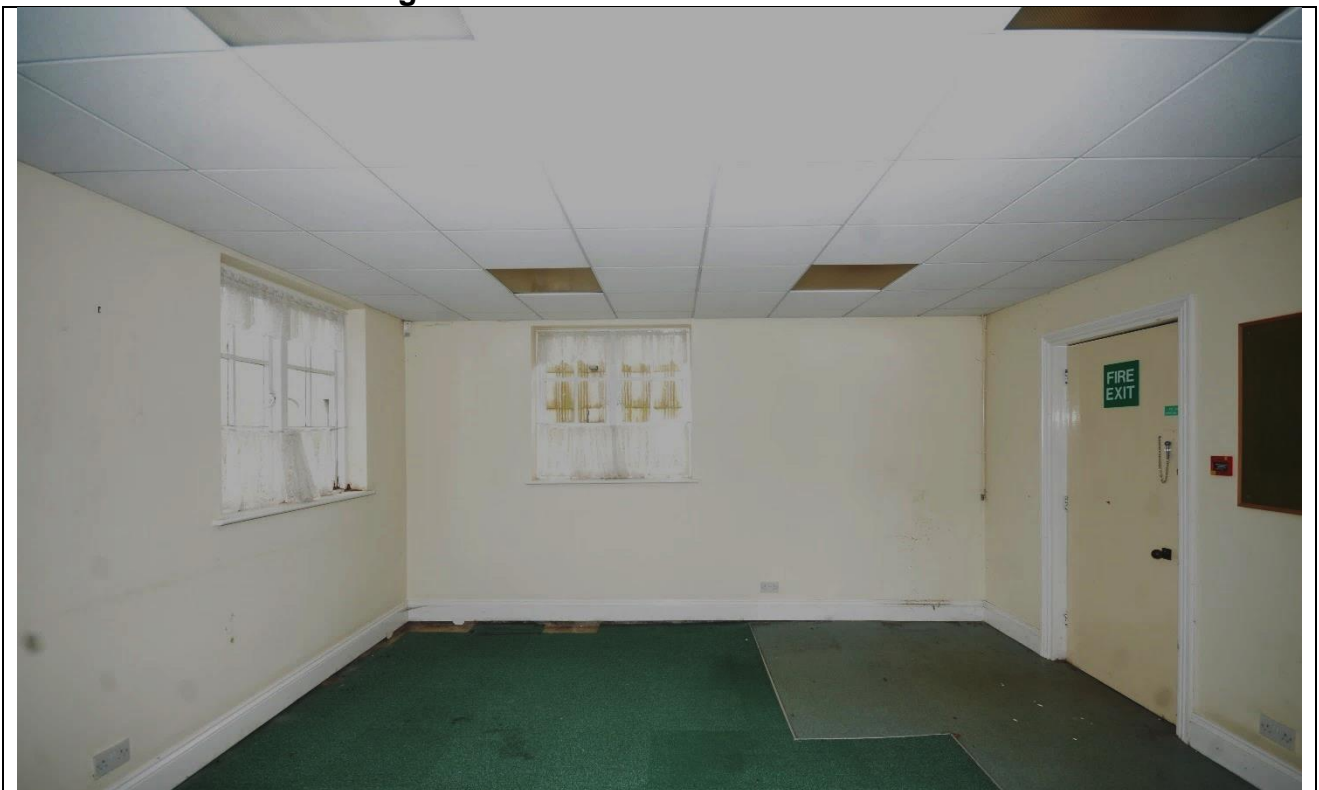
Plate 50: Room 6 Looking Northwest
