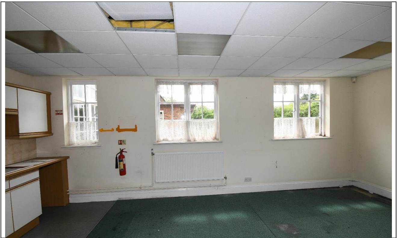
Plate 49: Room 6 Looking Southwest
