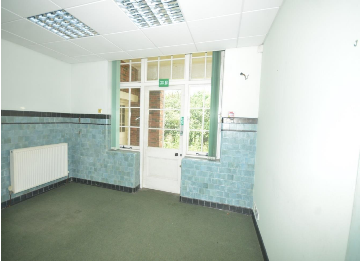
Plate 120: Small partitioned entrance lobby, eastern corner of room 27
