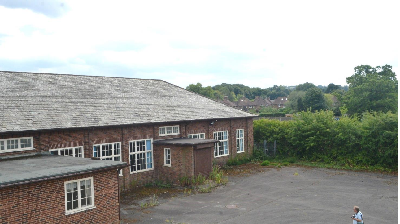
Plate 25: Elevated view of rear elevation
