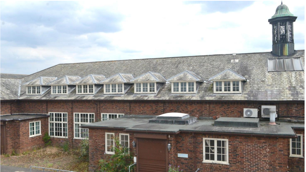
Plate 22: Elevated view of rear elevation
