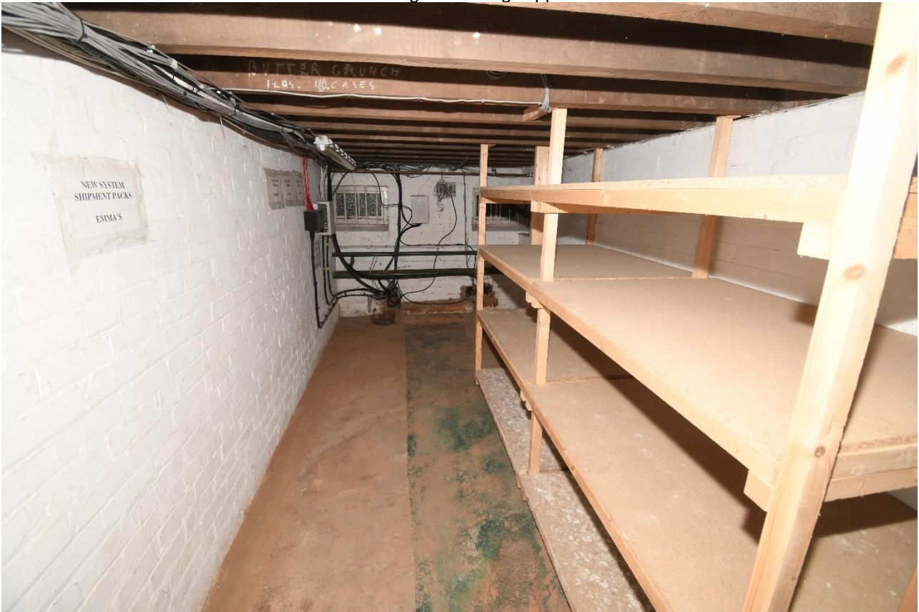
Plate 143: Bay 3 looking northeast
