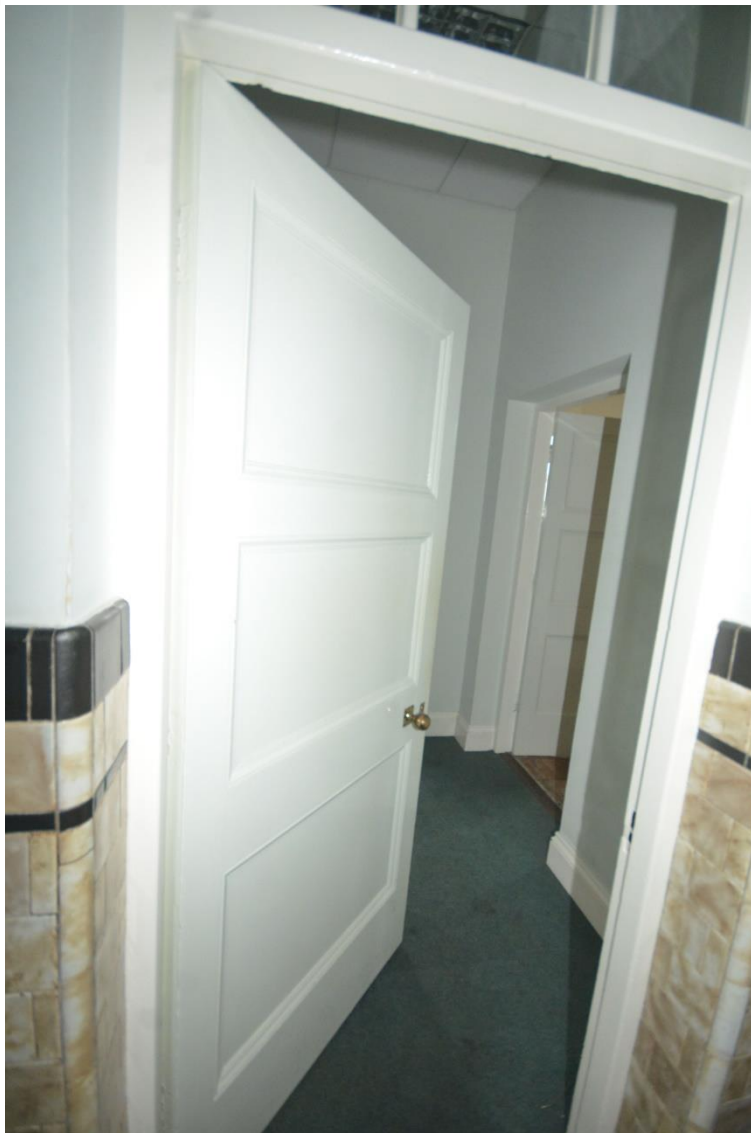
Plate 59: Room 9 Looking Southeast
