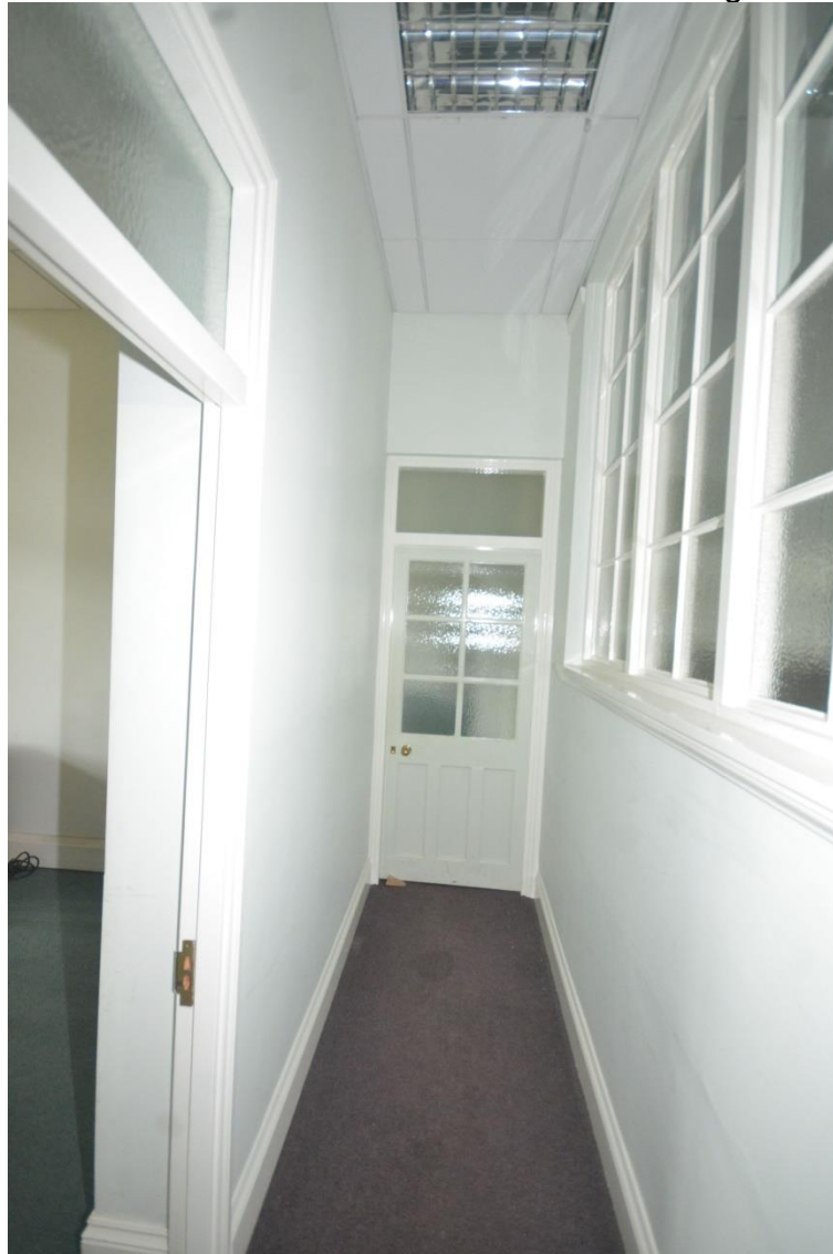
Plate 72: Room 14 Looking Southwest
