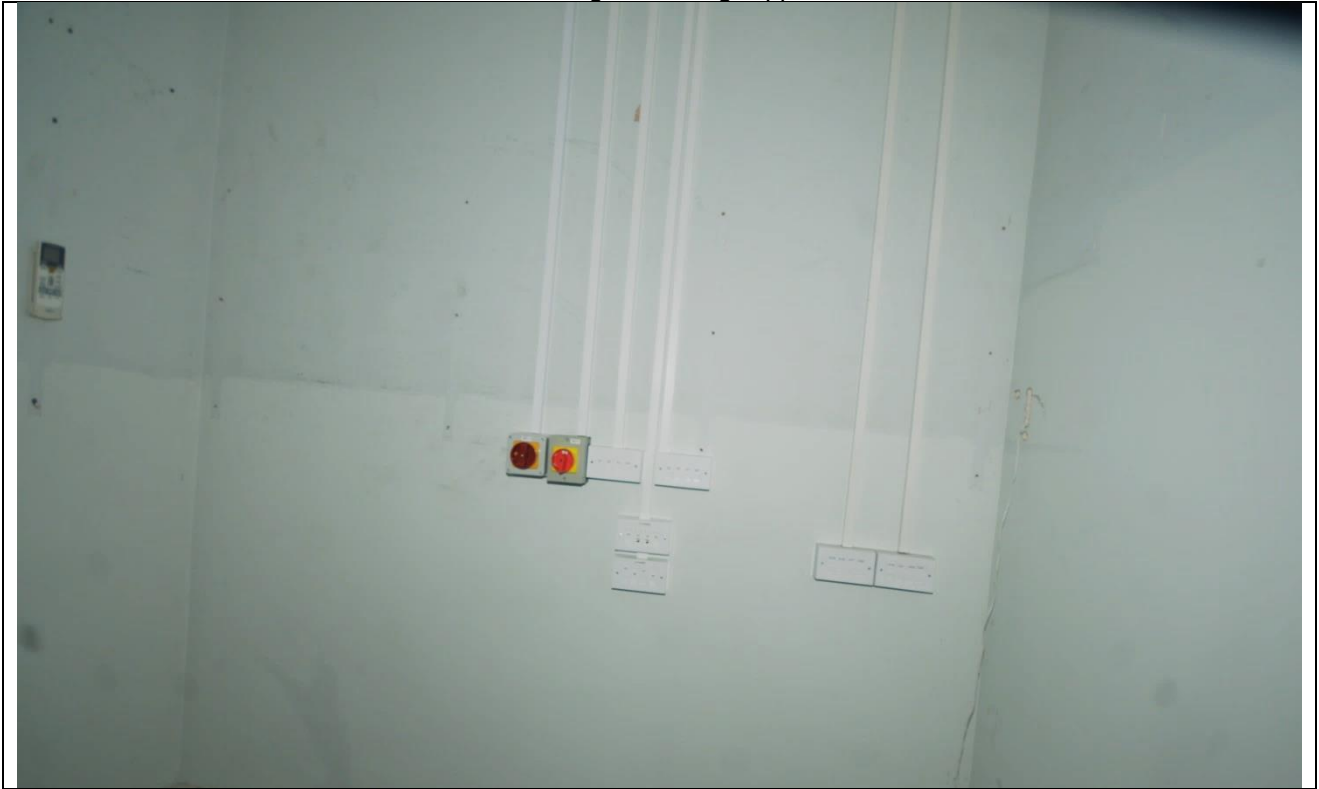
Plate 93: Room 20 Looking Northwest
