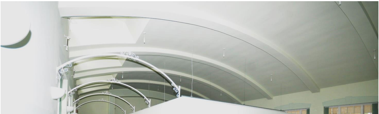
Plate 152: Detail of straight concrete arched beams over main auditorium
