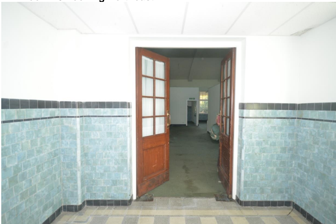
Plate 122: Room 28 Looking Southeast
