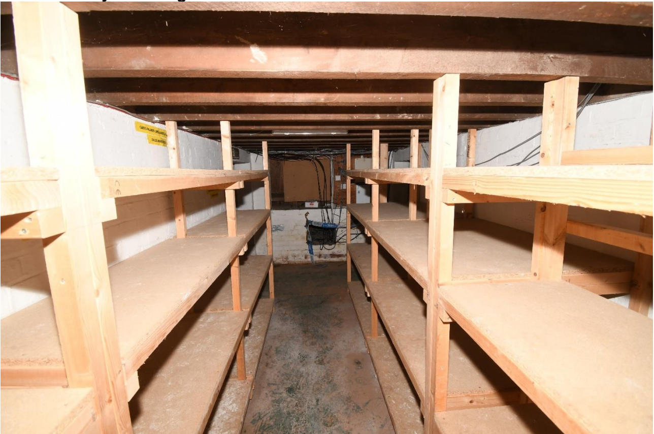
Plate 142: Bay 2 looking northeast
