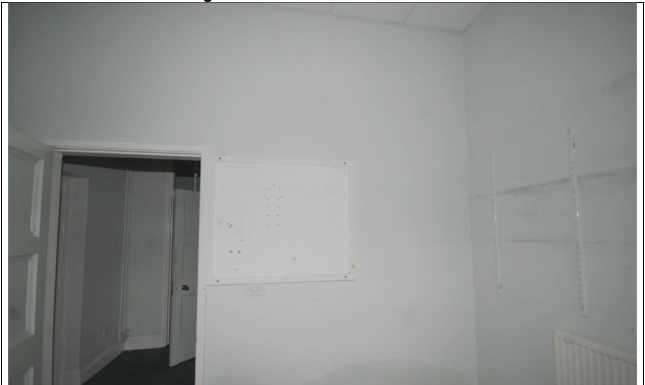
Plate 64: Room 11 Looking Northwest
