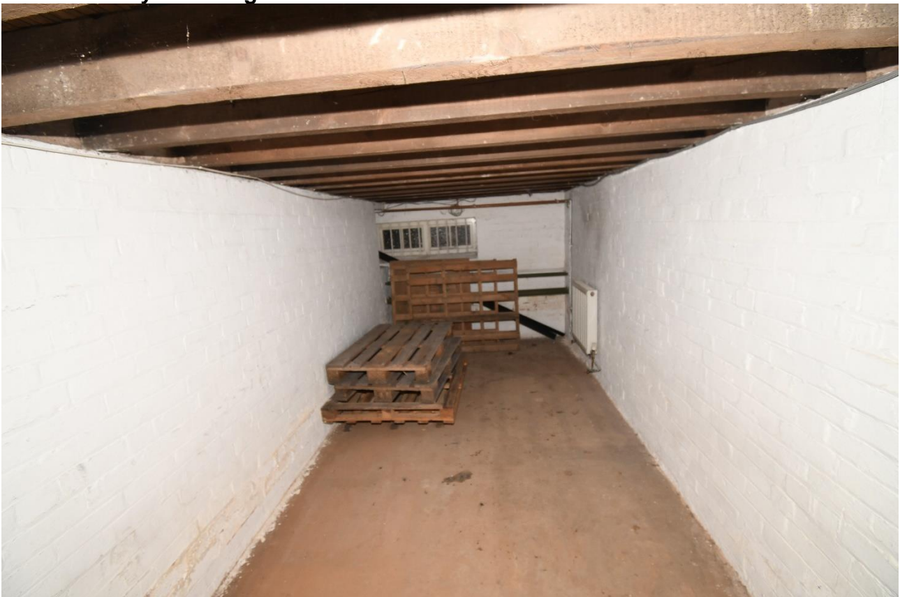
Plate 144: Bay 4 looking northeast
