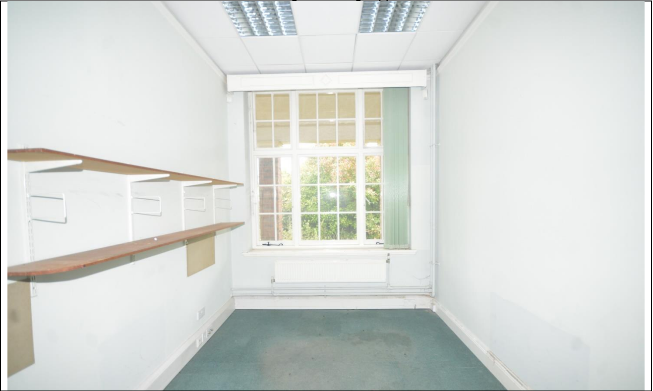
Plate 70: Room 13 Looking Southeast
