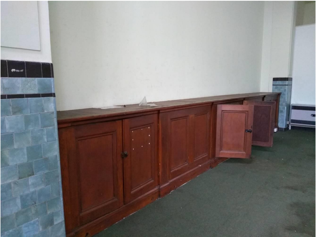
Plate 140: Entrance from room 27
