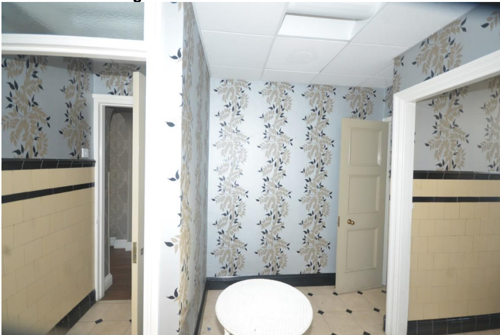
Plate 89: Room 19 Looking Southeast
