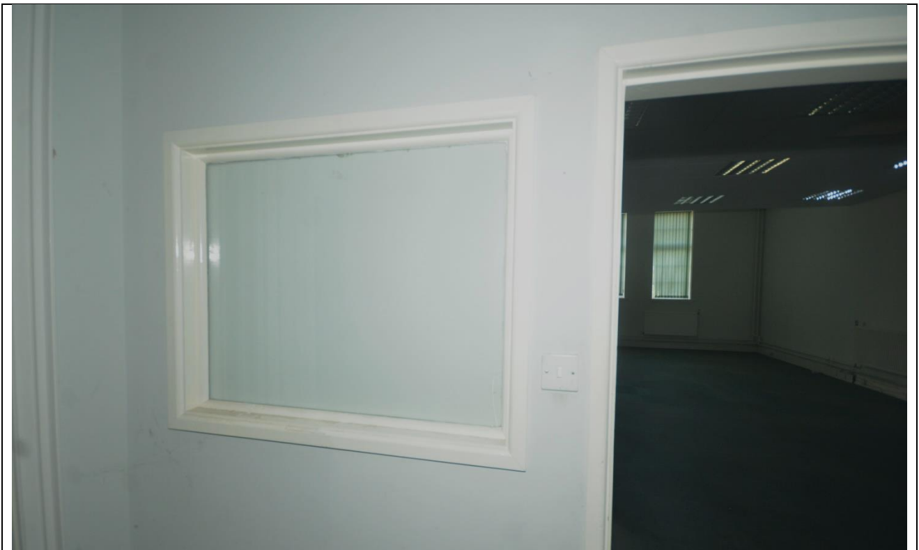
Plate 94: Room 21 Looking Southeast
