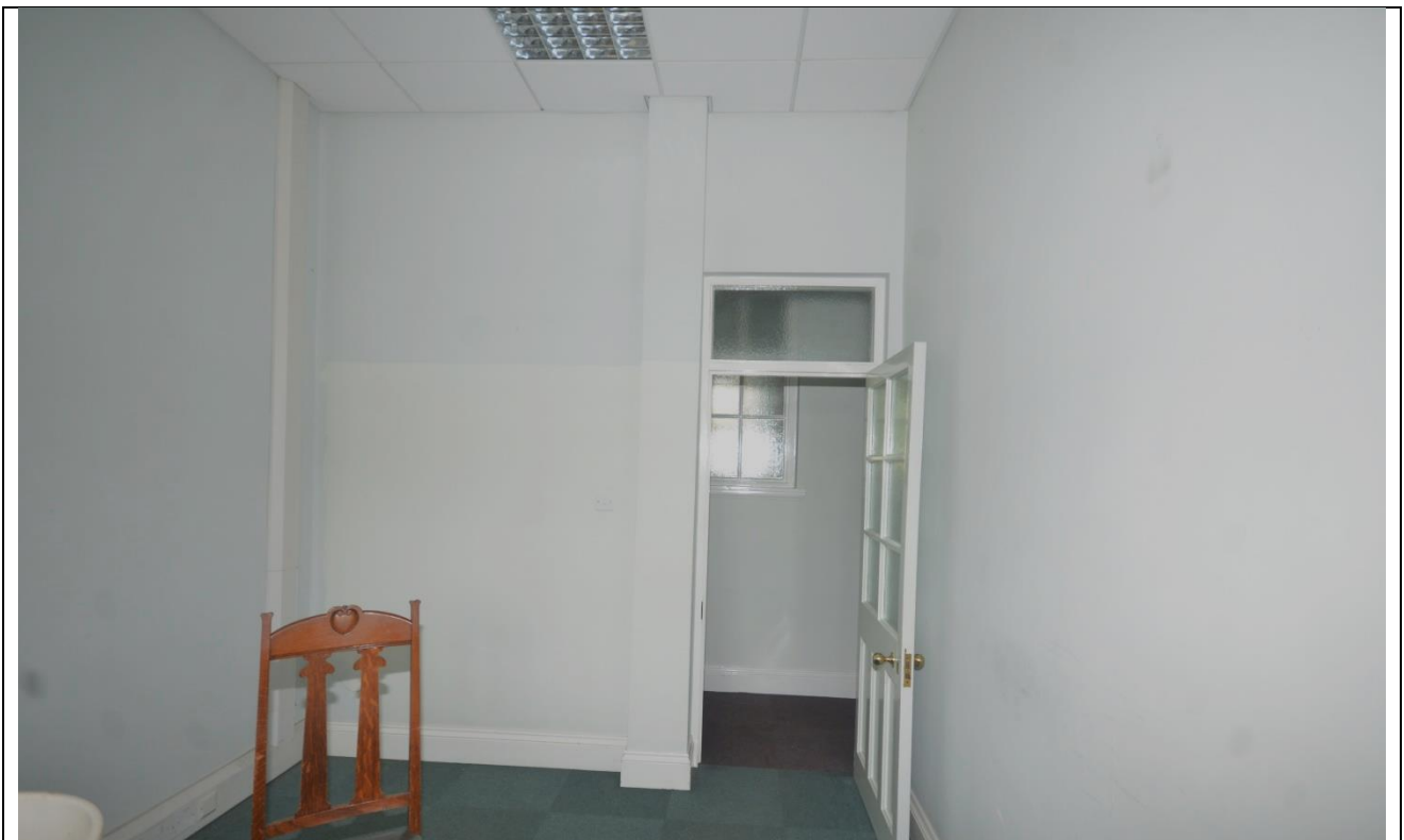
Plate 75: Room 15 Looking Northwest
