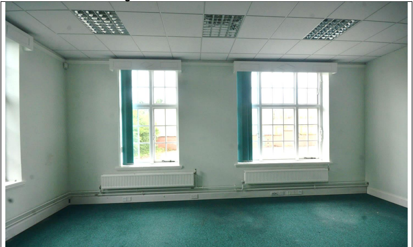
Plate 39: Room 4 Looking Northwest
