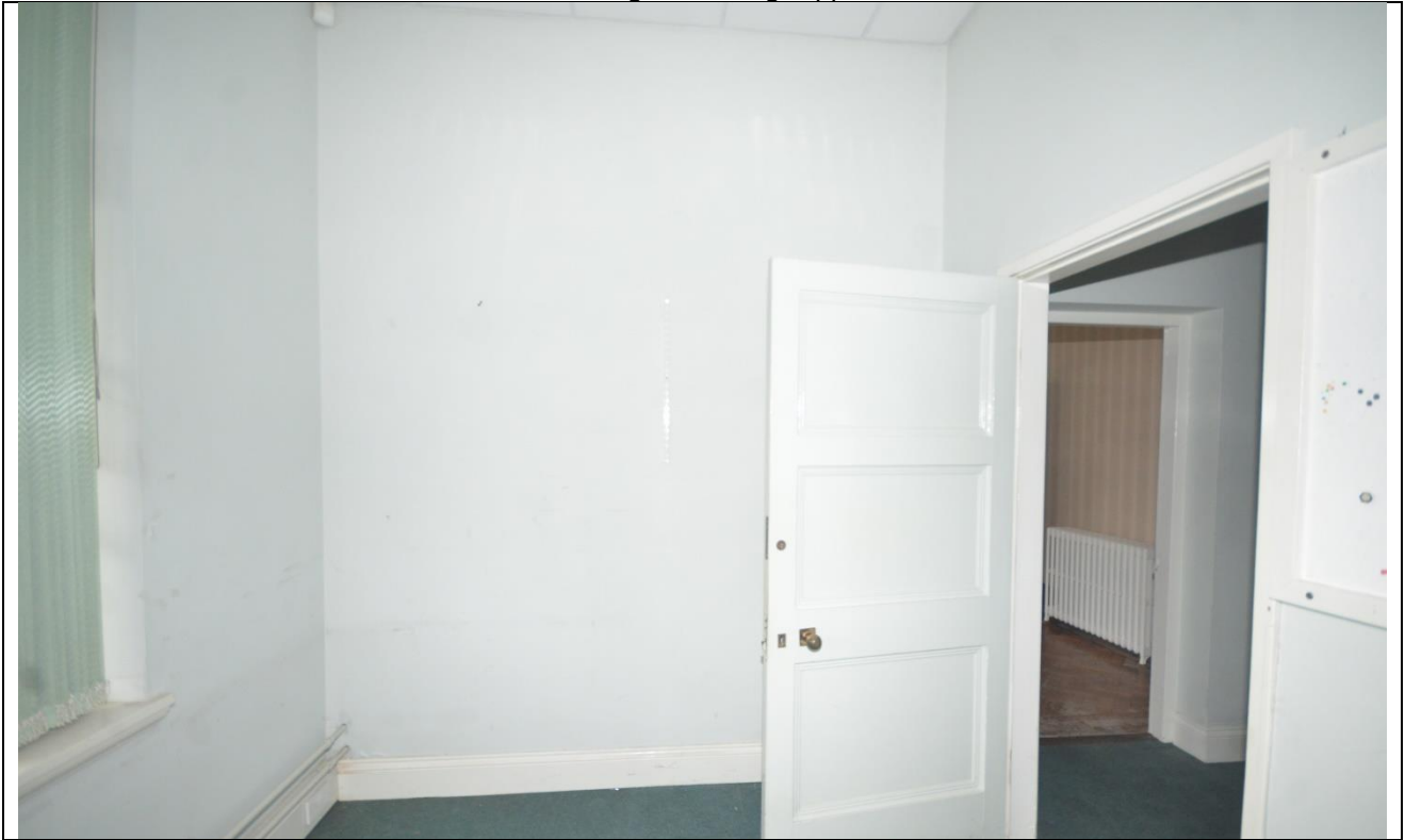
Plate 63: Room 11 Looking Southwest
