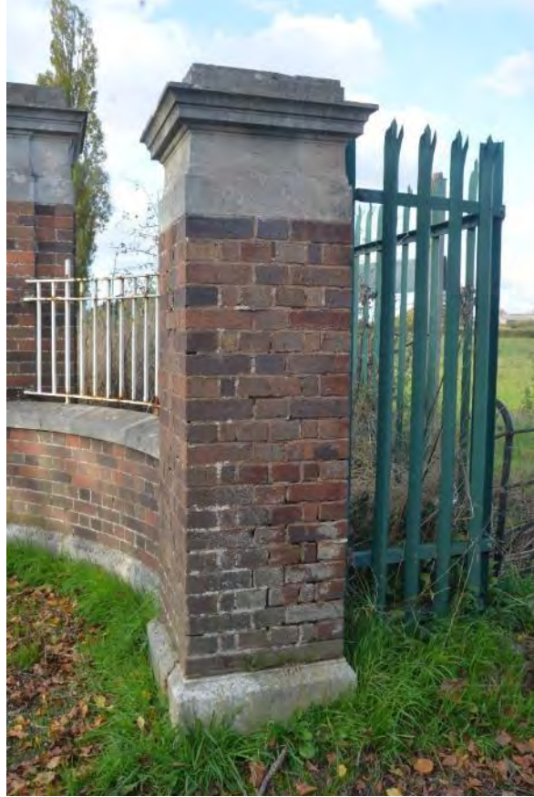
Plate 28: Detail of brick pier adjacent to northeast gate
