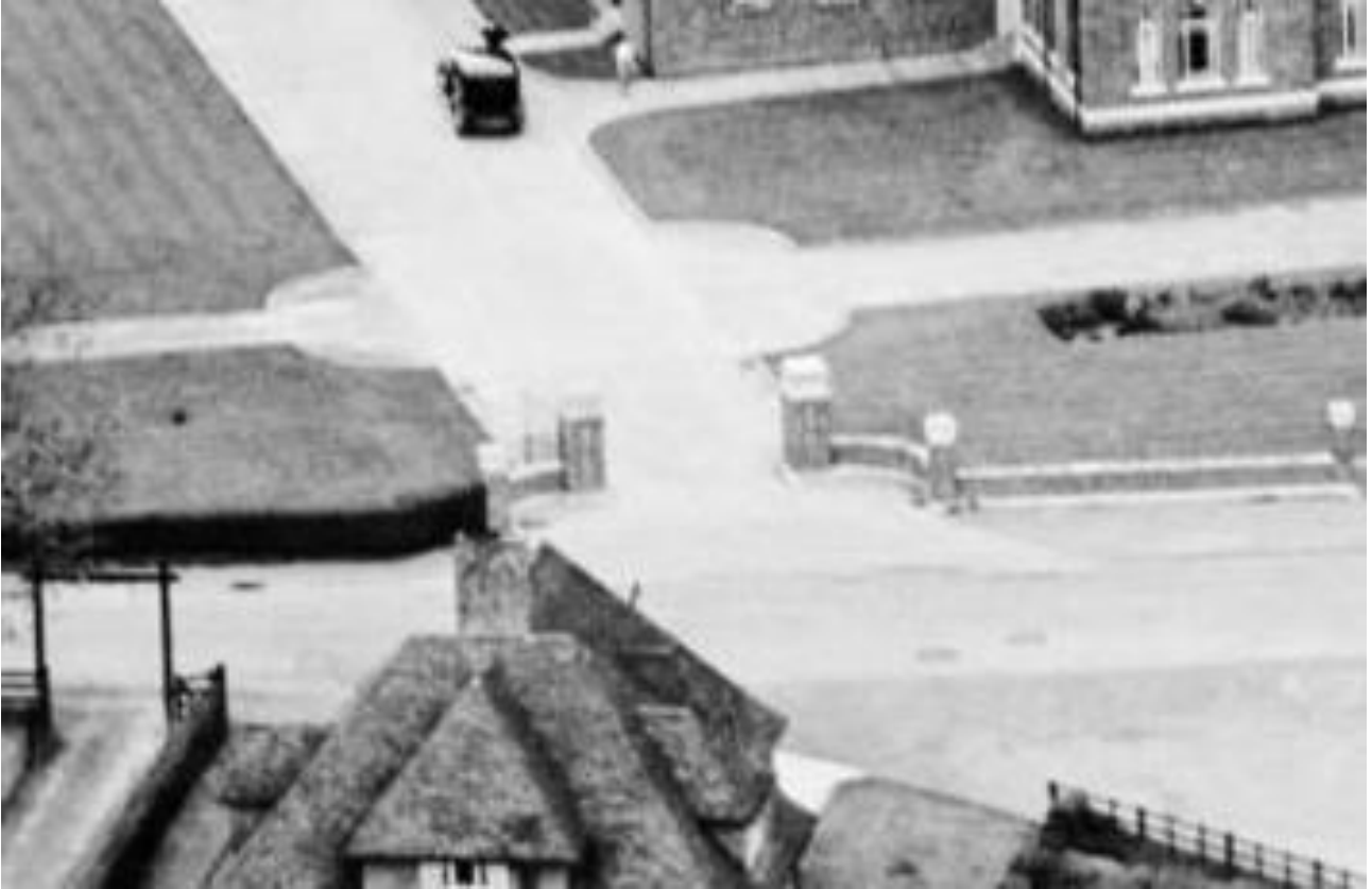
Plate 11: View of southwest entrance in 1936 showing original layout
