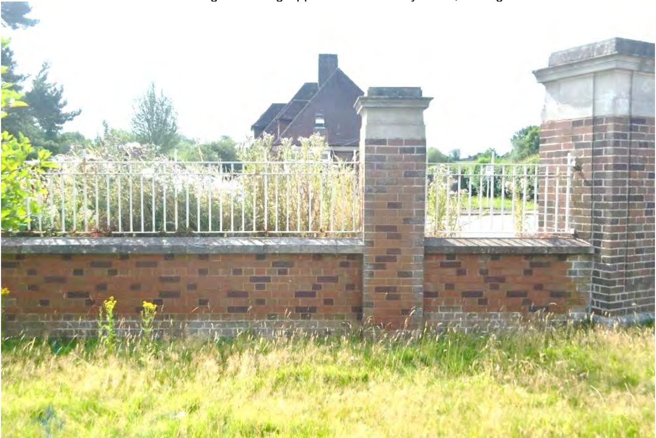
Plate 40: Boundary wall, internal
