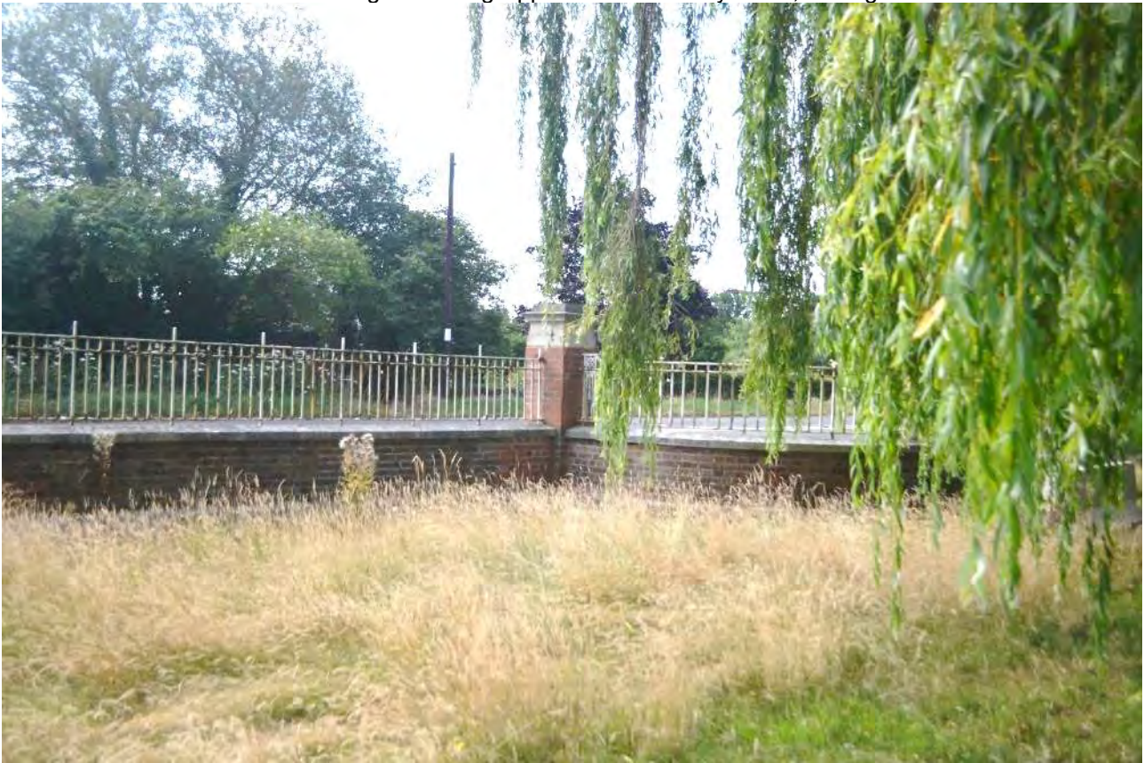
Plate 38: Boundary wall, internal
