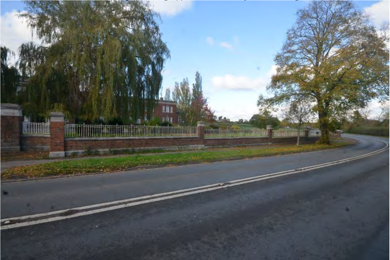
Plate 34: Boundary wall, external
