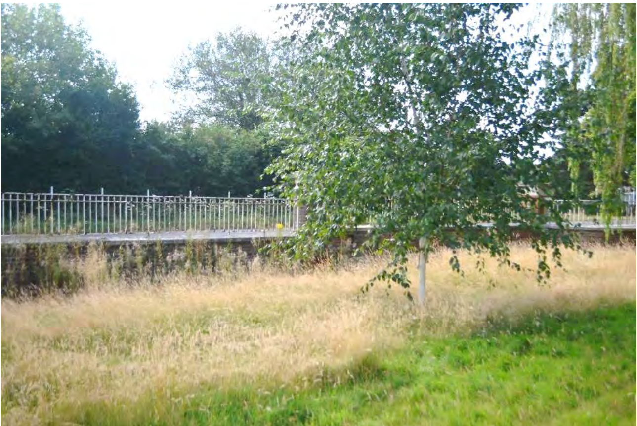
Plate 37: Boundary wall, internal
