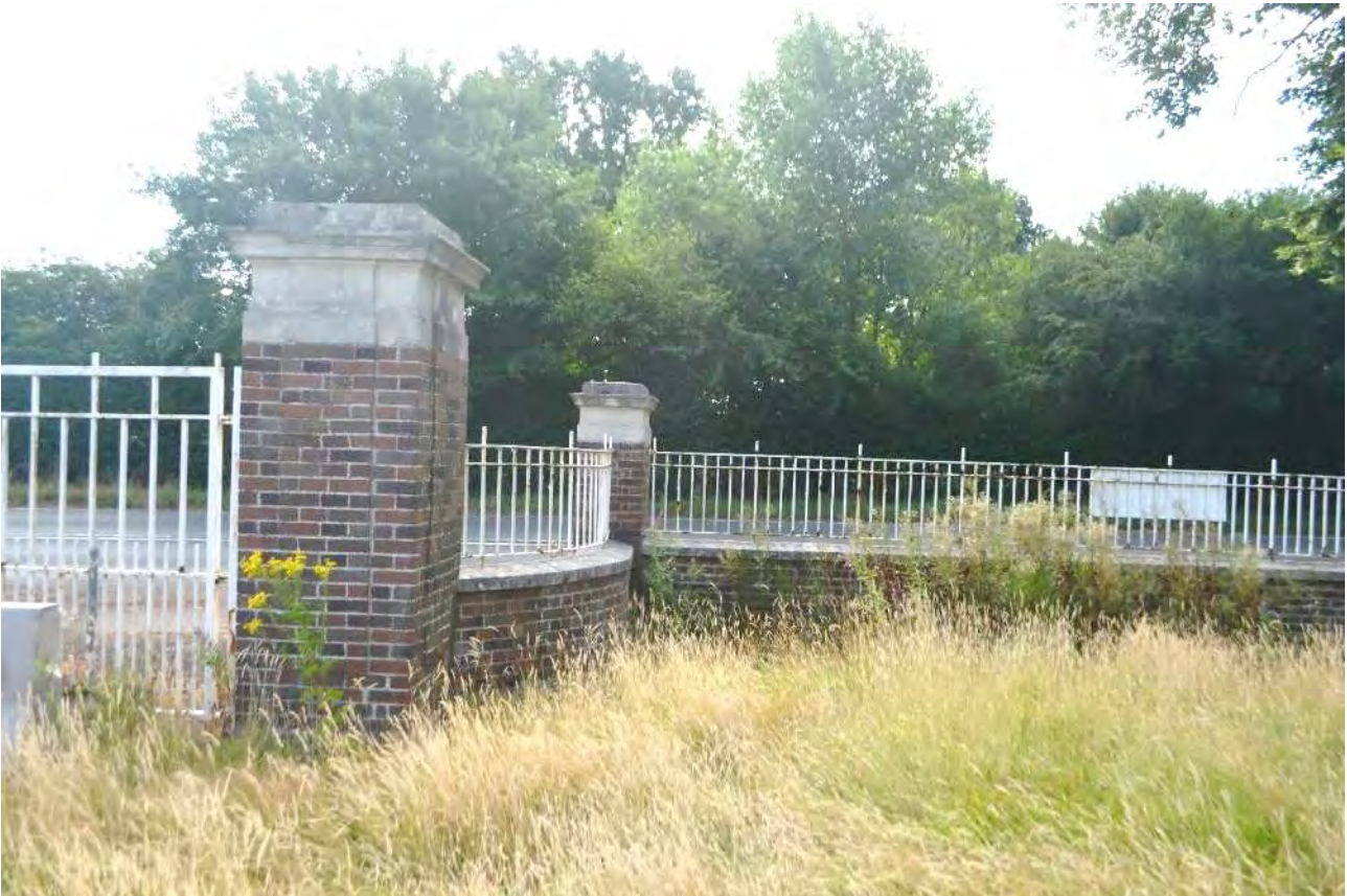
Plate 35: Boundary wall, internal
