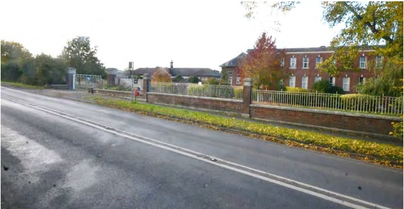
Plate 30: Boundary wall, external
