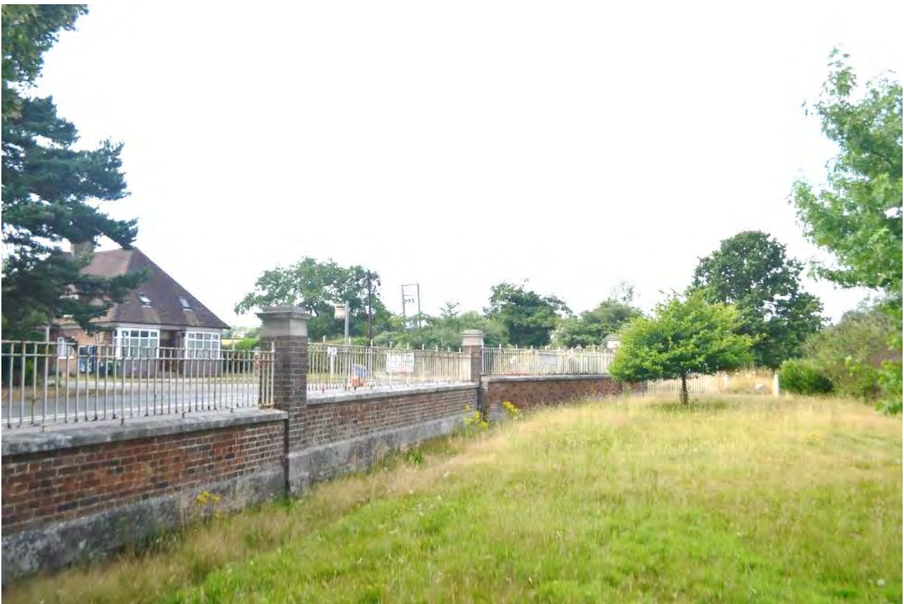
Plate 39: Boundary wall, internal
