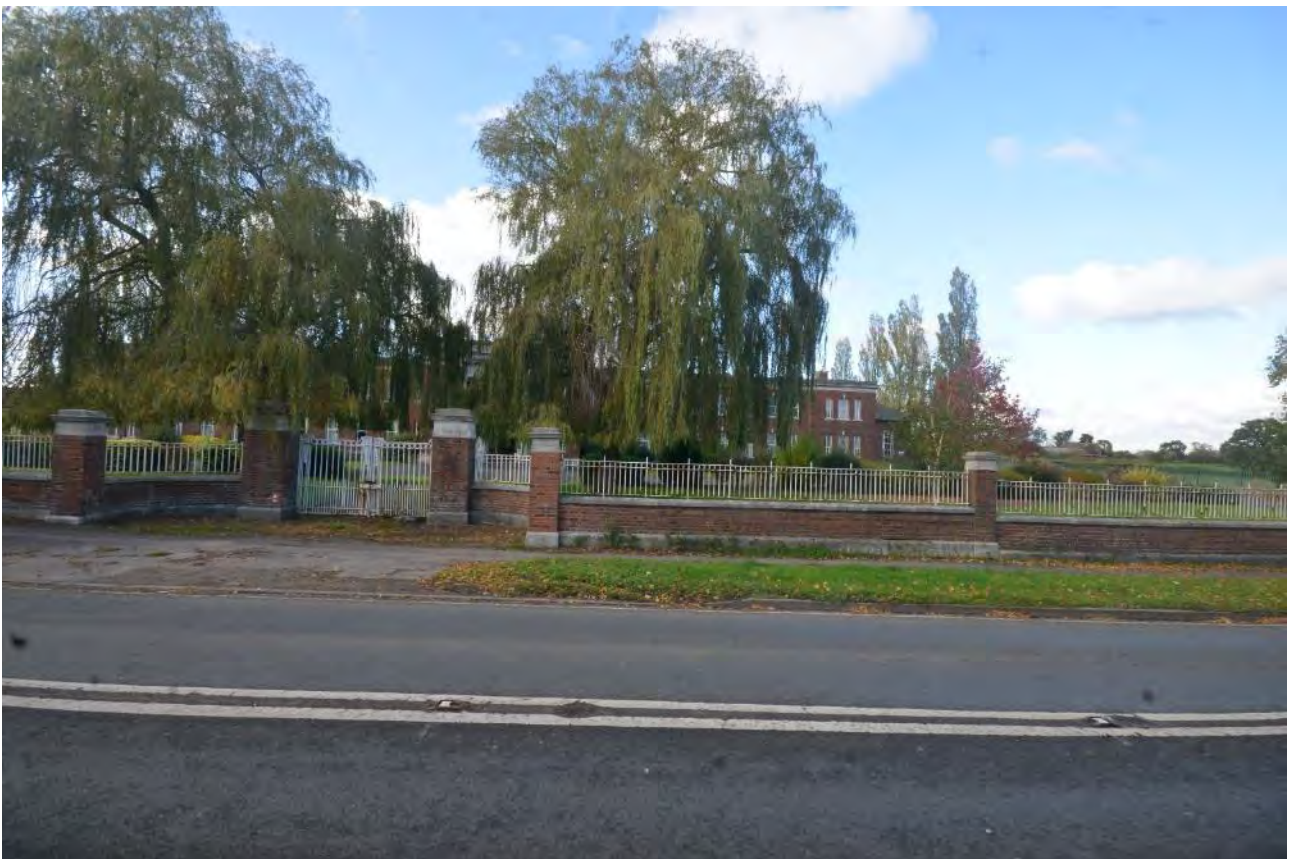
Plate 33: Boundary wall, external
