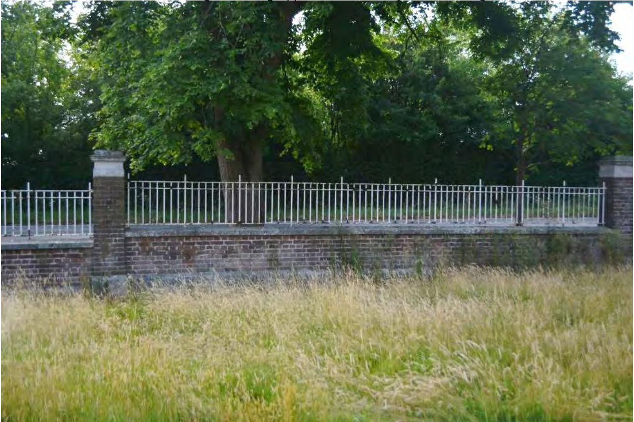
Plate 36: Boundary wall, internal
