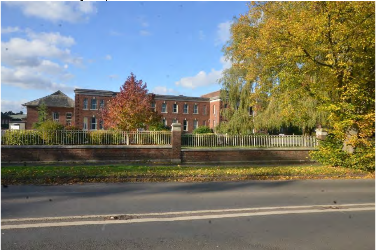
Plate 31: Boundary wall, external
