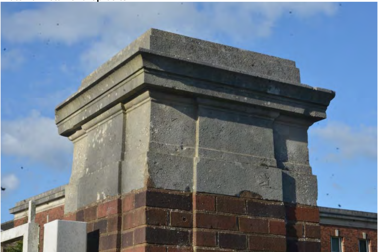
Plate 21: Detail of head of gate pier
