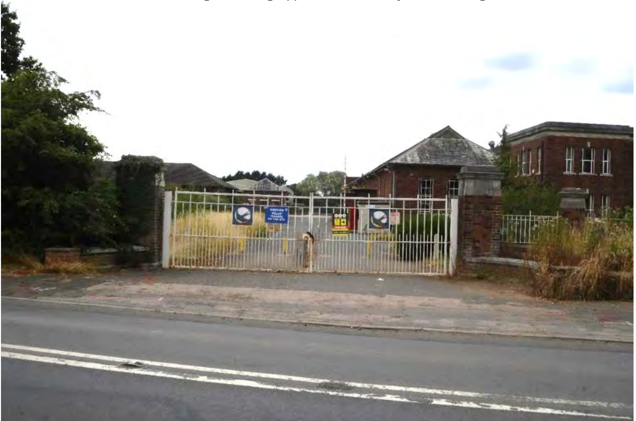
Plate 14: Southwest gates (vehicle), closed, viewed from outside
