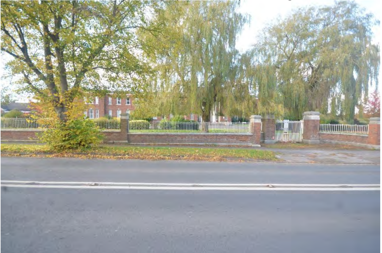
Plate 32: Boundary wall, external
