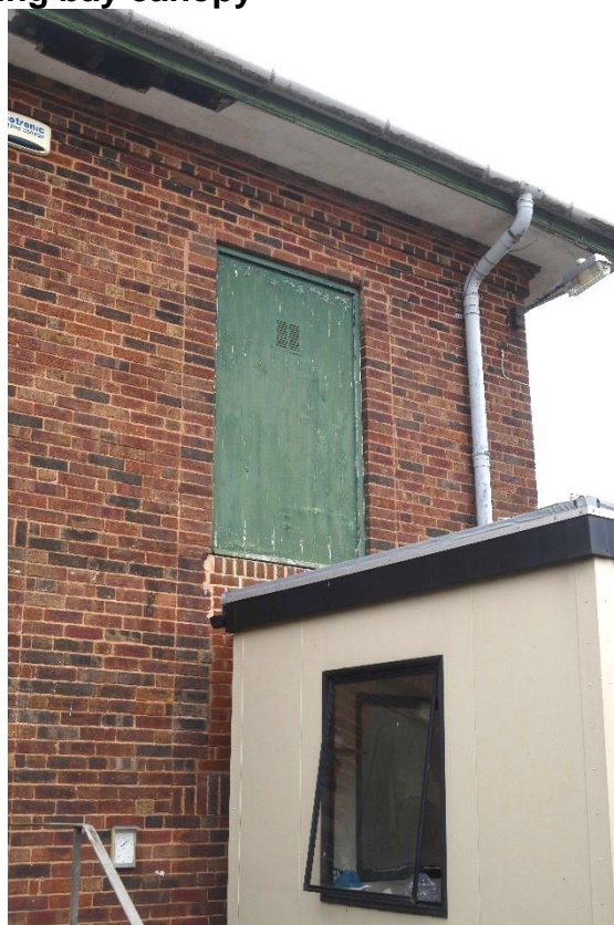
Plate 34: Detail of former first floor fire exit
