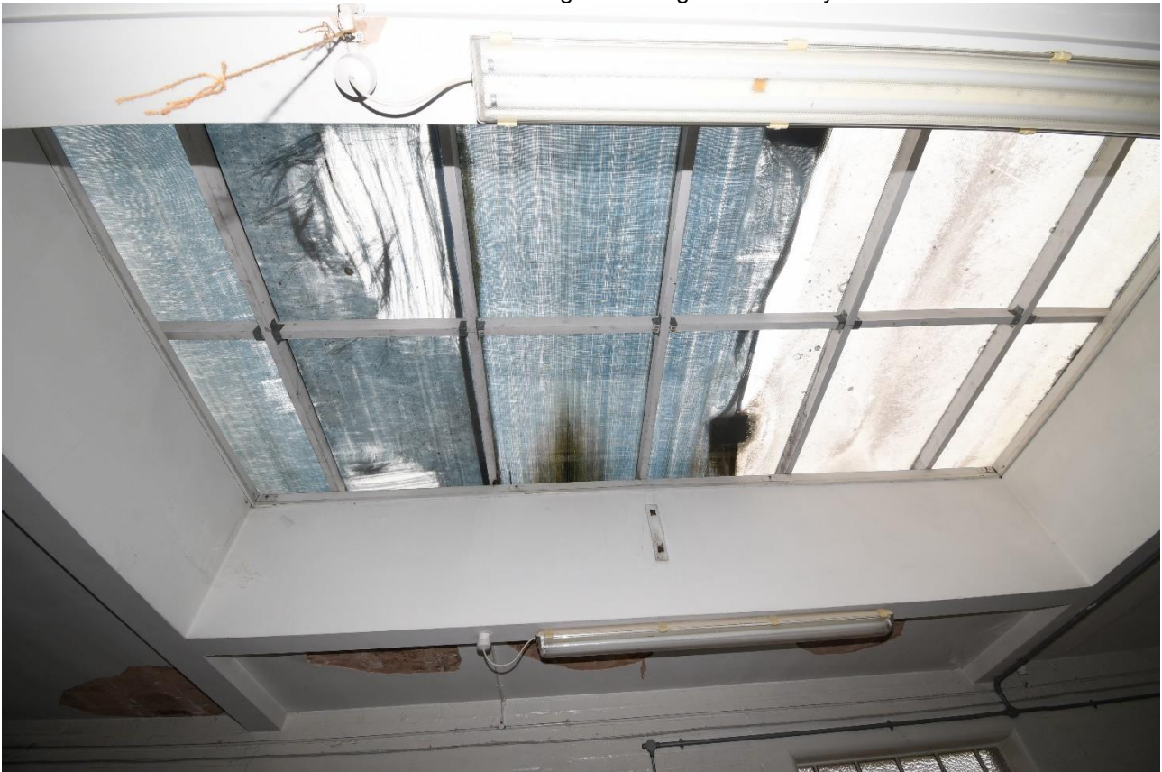
Plate 104: Detail of flat lantern over room 9
