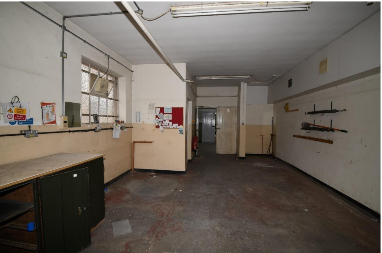
Plate 91: Northeast aspect, Room 7
