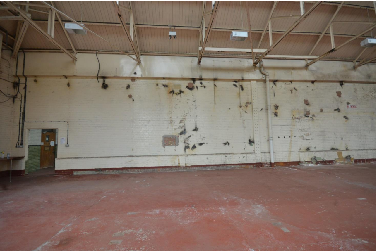
Plate 87: Southwest aspect, room 6
