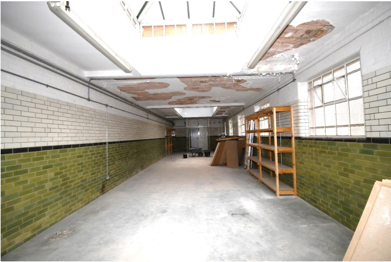
Plate 102: Southwest aspect, room 9
