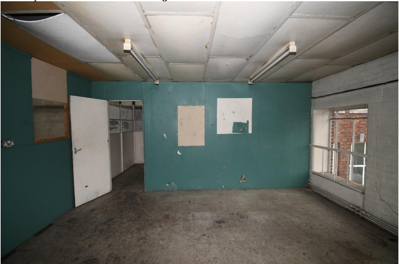
Plate 128: Northeast aspect, mezzanine room 2
