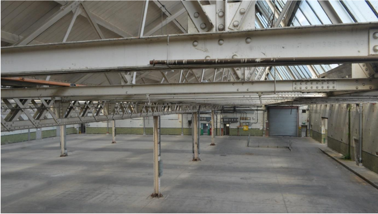
Plate 76: Detail of roof structure
