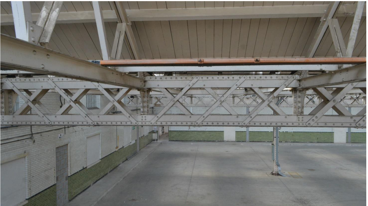
Plate 75: Detail of roof structure
