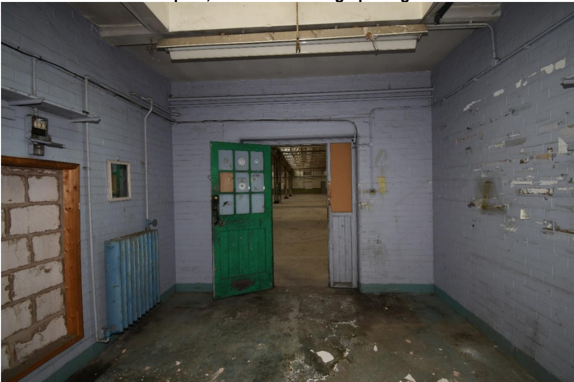
Plate 107: Southeast aspect, room 10 showing opening
