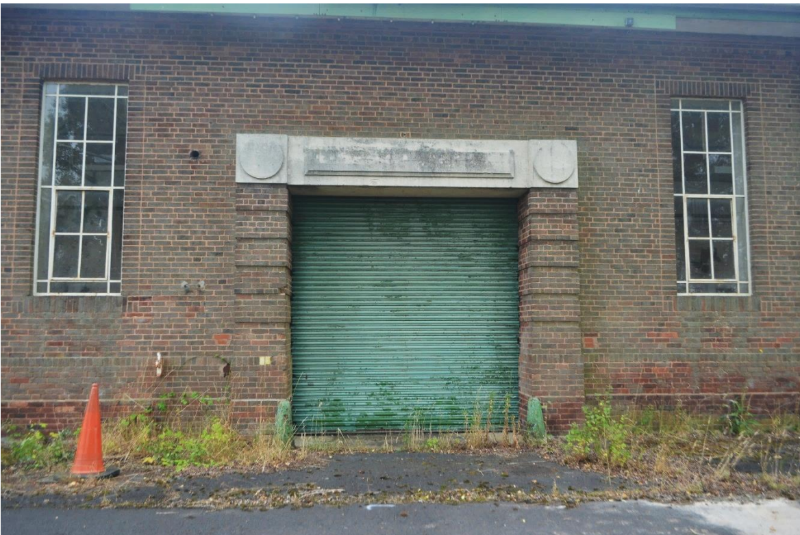
Plate 38: Detail of loading bay, northeast wall
