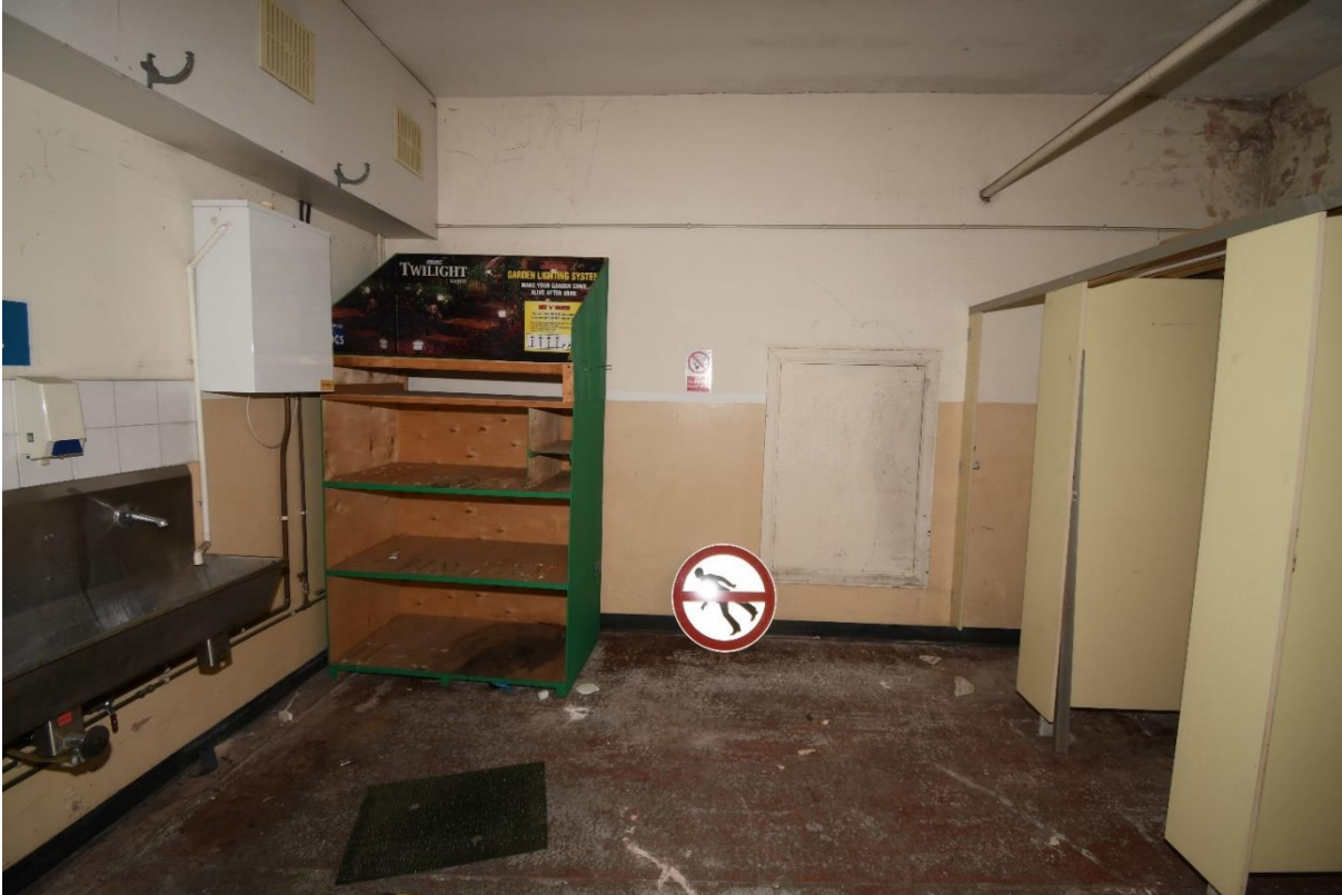
Plate 94: Southwest aspect, room 7a
