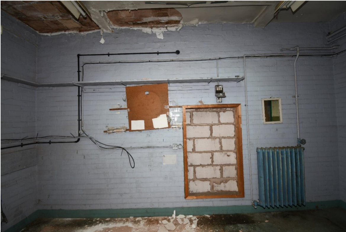
Plate 106: Northeast aspect, room 10 showing opening
