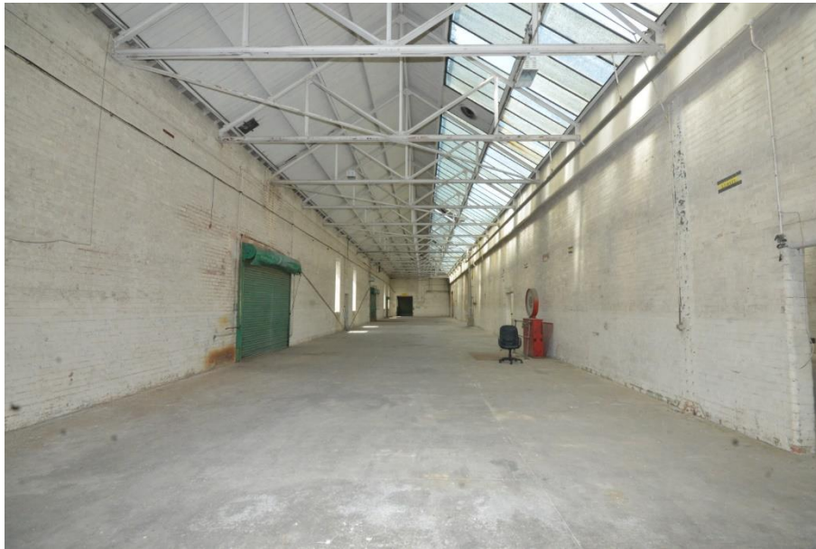
Plate 52: Room 1, northwest aspect
