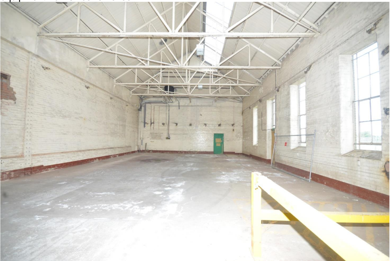
Plate 88: Northwest aspect, room 6
