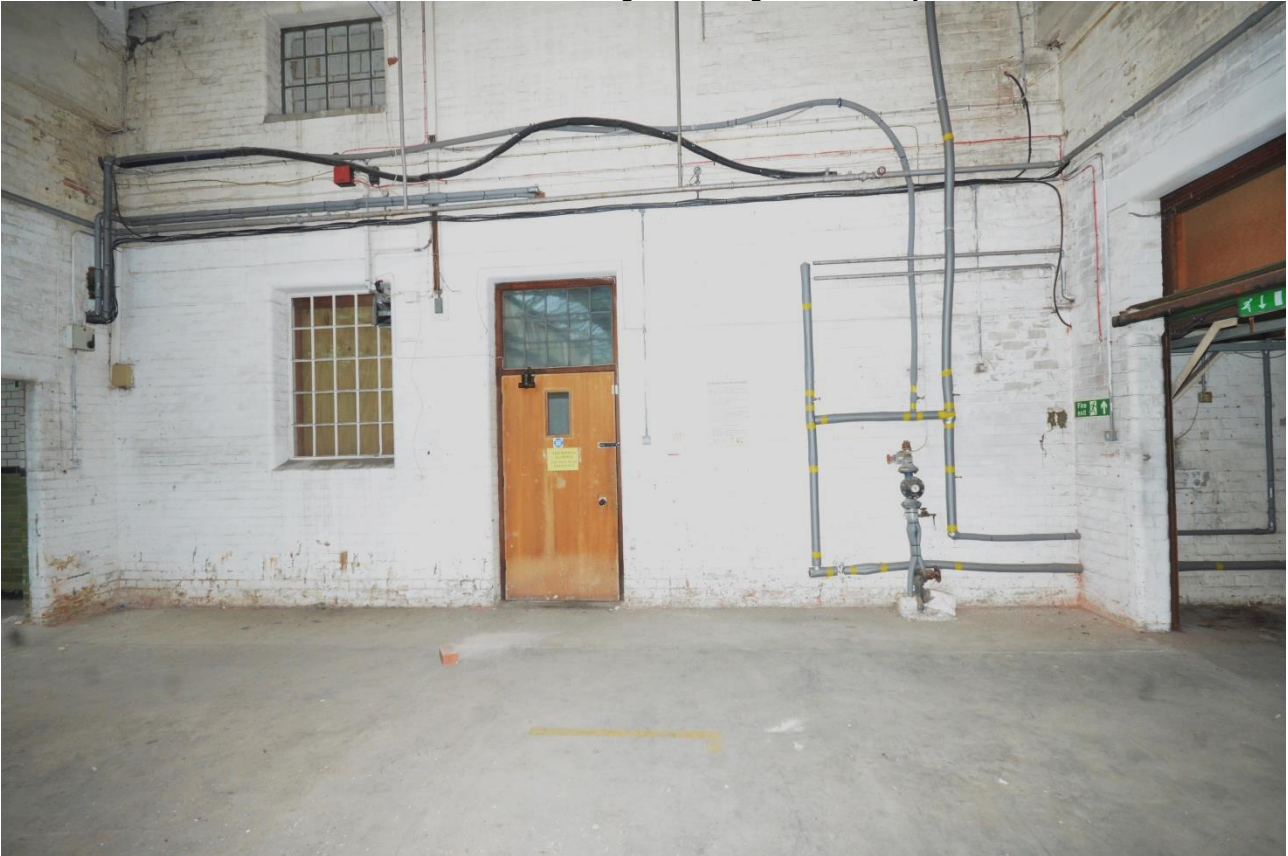
Plate 121: Door and windows to administration building in southeast wall of room 3
