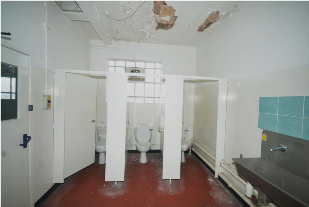
Plate 116: Northwest aspect, room 14
