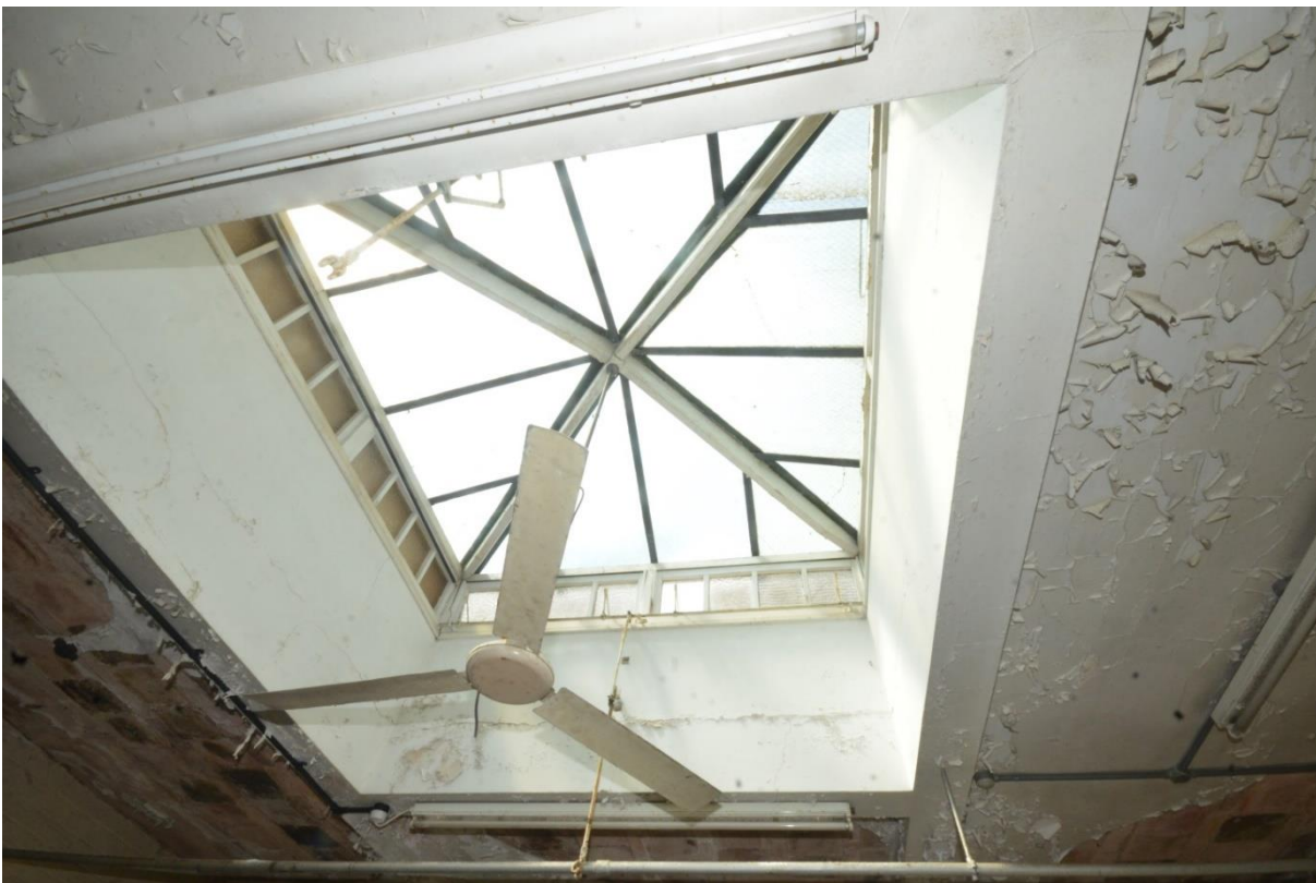
Plate 113: Lantern above room 12
