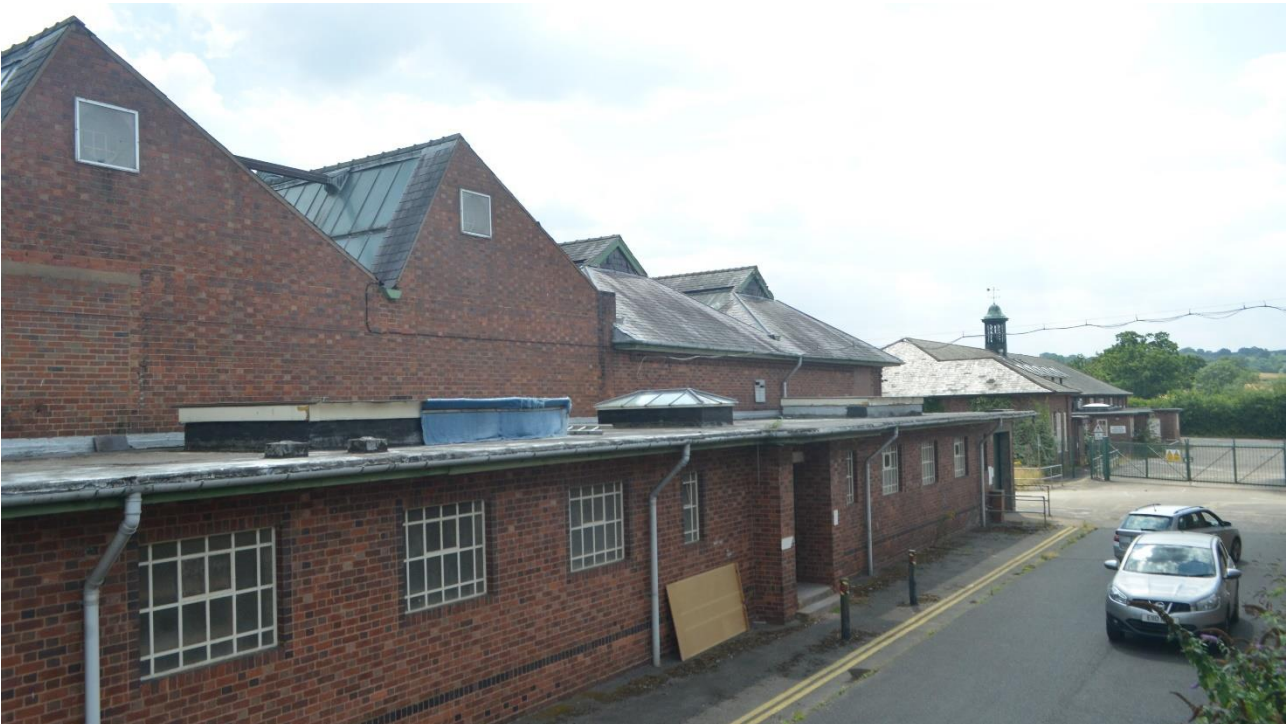
Plate 48: Detail of lanterns over rooms 7, 8 and 9
