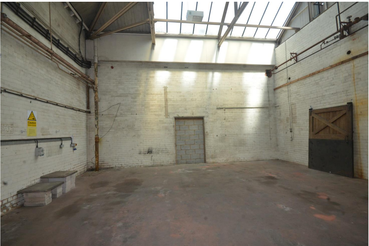
Plate 59: Northeast aspect, room 2
