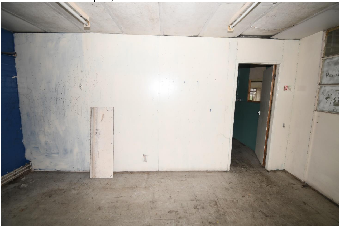
Plate 126: Southwest aspect, mezzanine room 1
