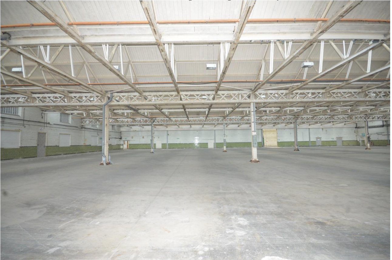
Plate 70: Southwest aspect, room 4
