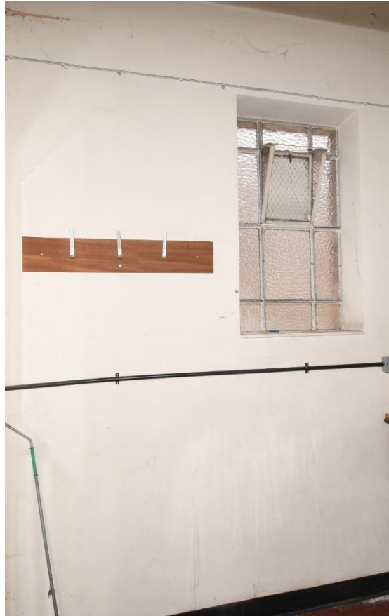
Plate 98: Northwest aspect, room 7b
