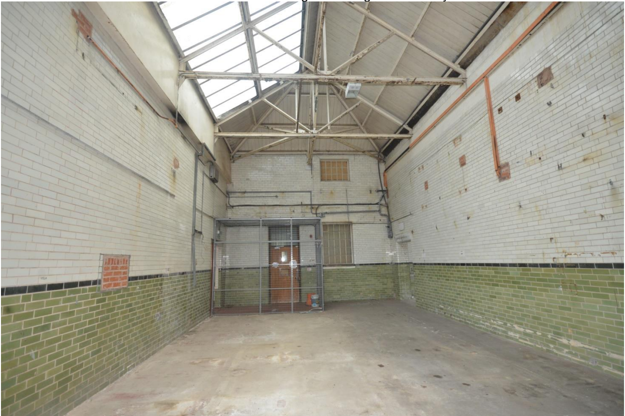
Plate 81: Detail of southeast wall, with mesh partition
