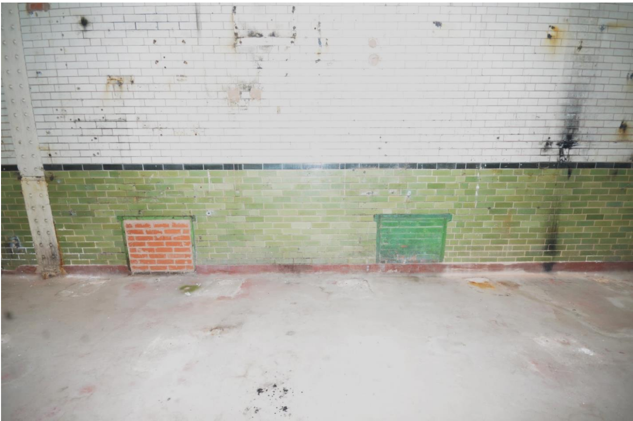
Plate 82: Detail of blocked openings in northeast wall
