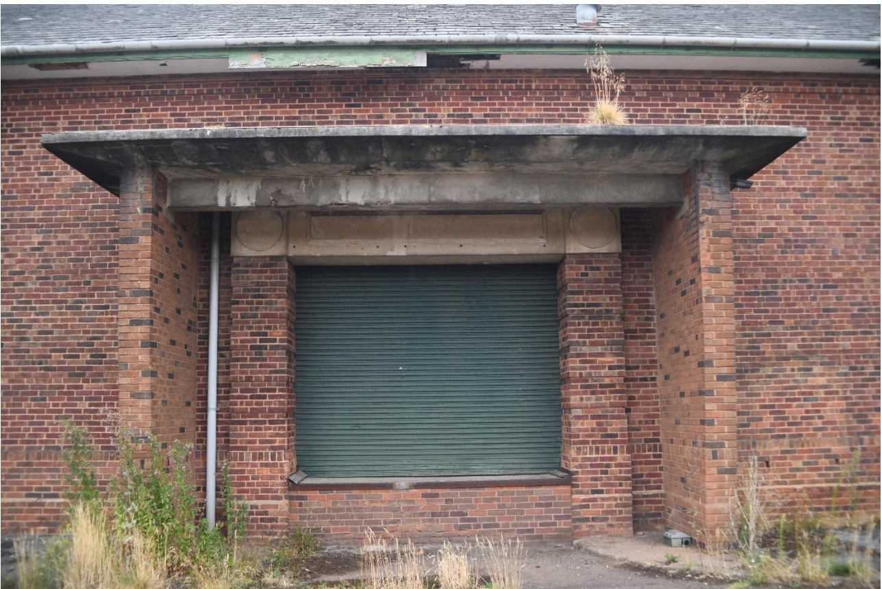
Plate 32: Detail of loading bay
