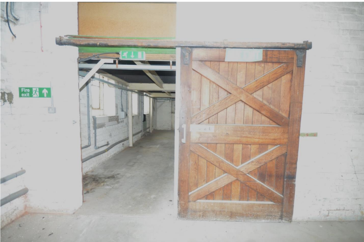
Plate 57: Detail of sliding door, room 1
