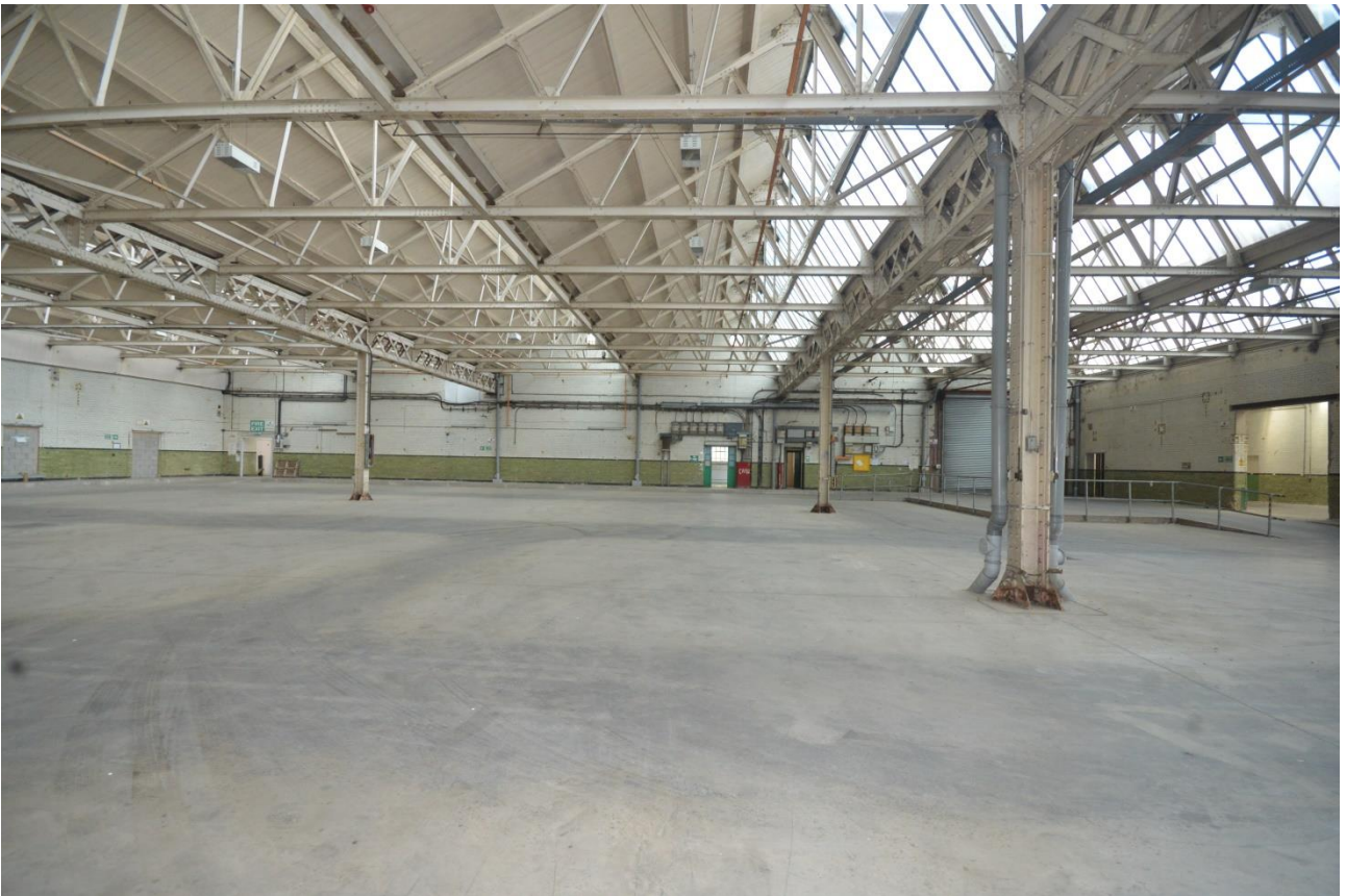
Plate 71: Northwest aspect, room 4
