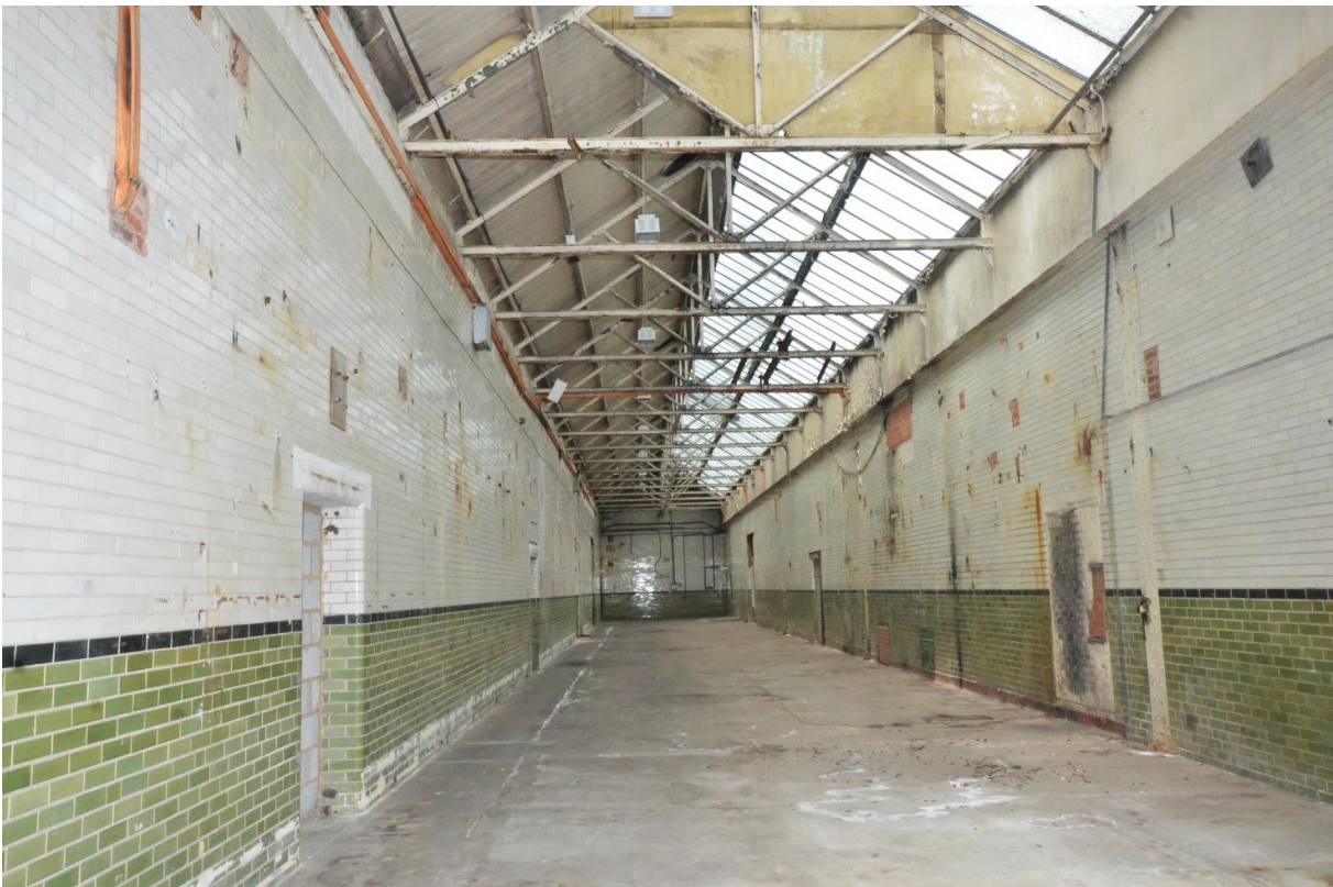
Plate 77: Northwest aspect, room 5
