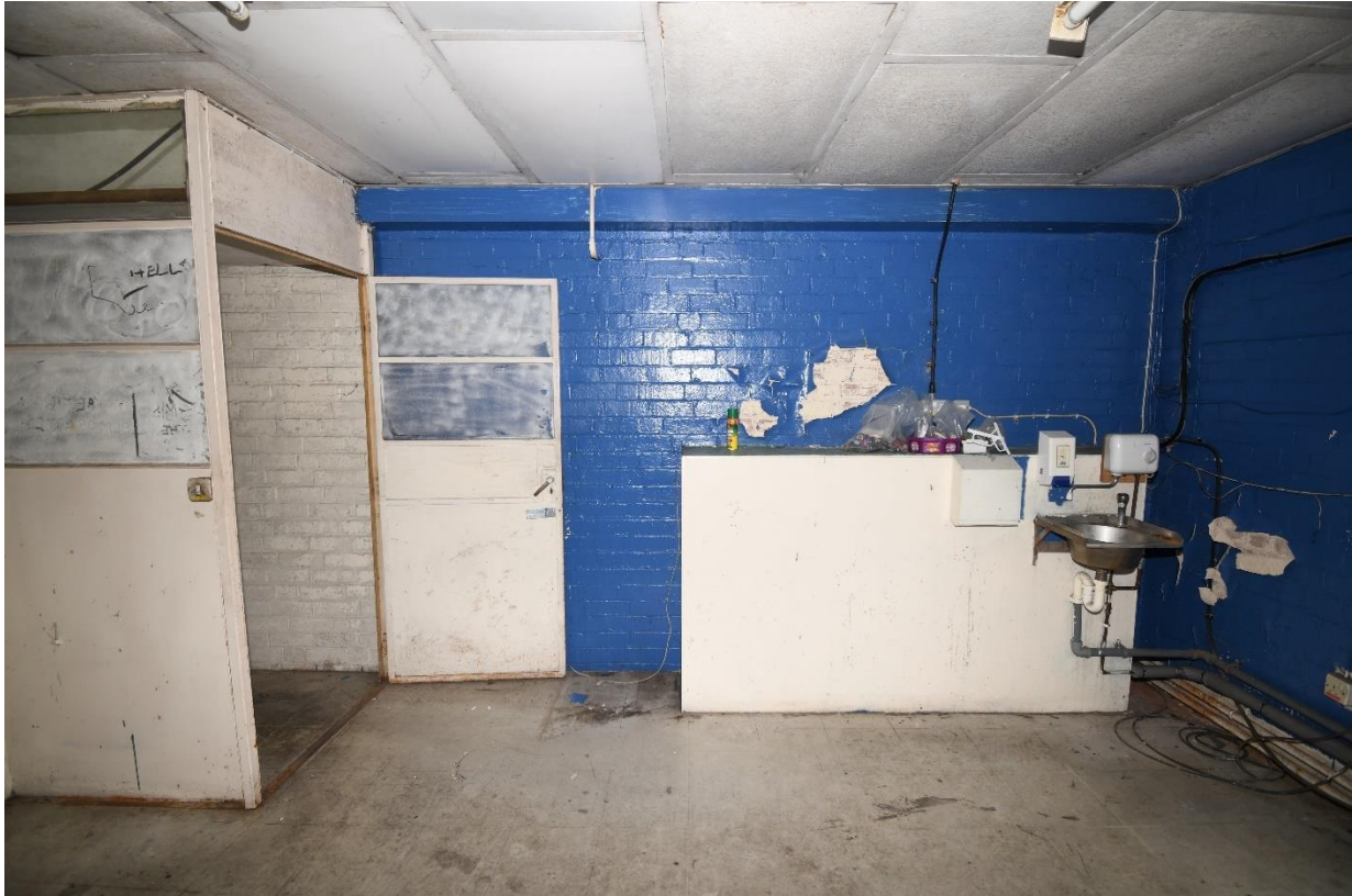
Plate 125: Northeast aspect, mezzanine room 1
