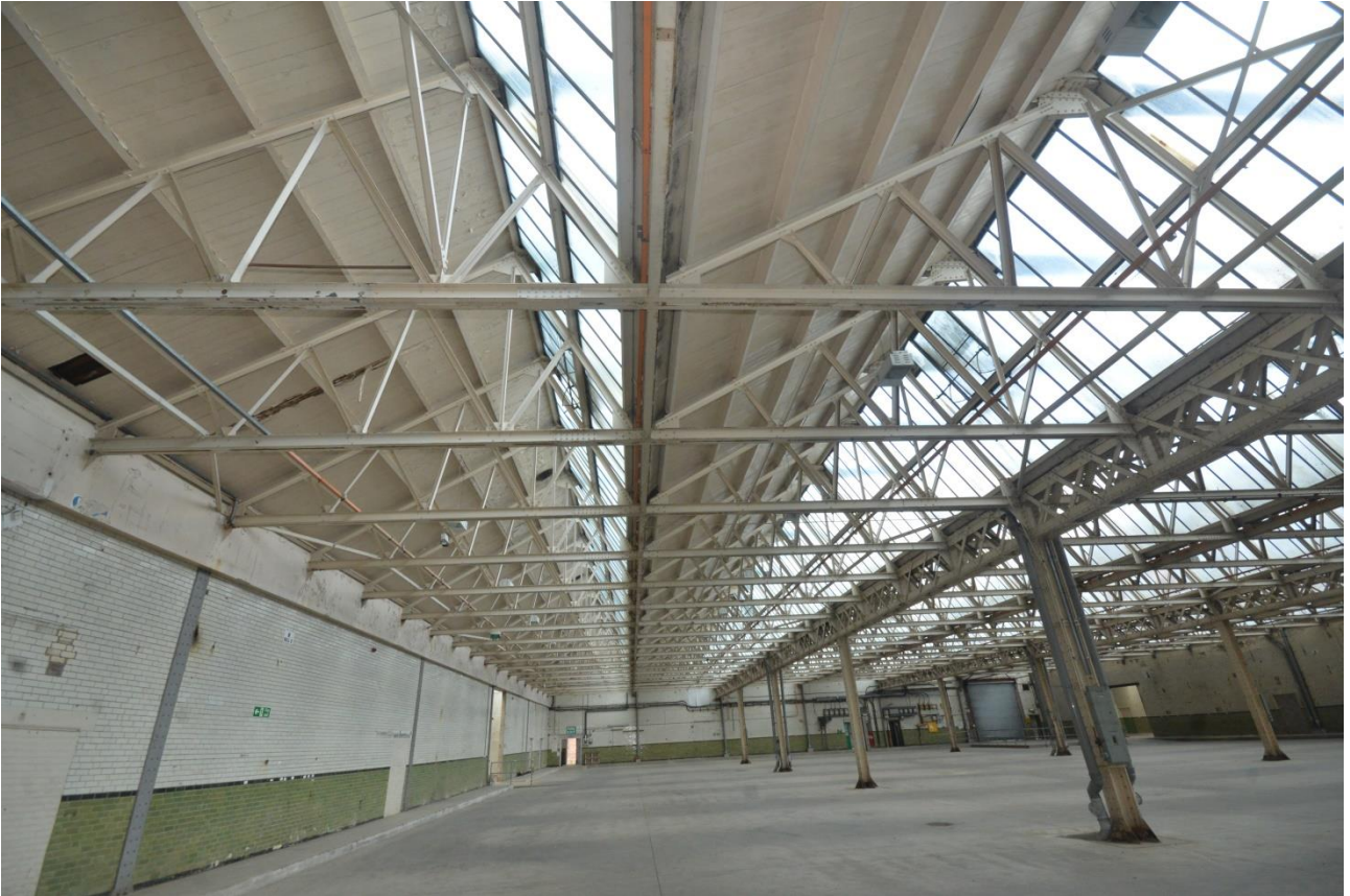
Plate 74: Detail of roof structure, viewed from southeast
