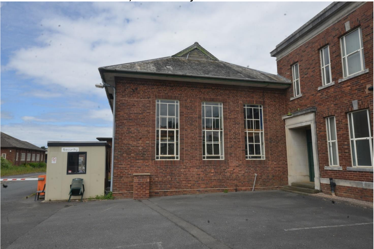
Plate 50: Southeast elevation, southwest bay
