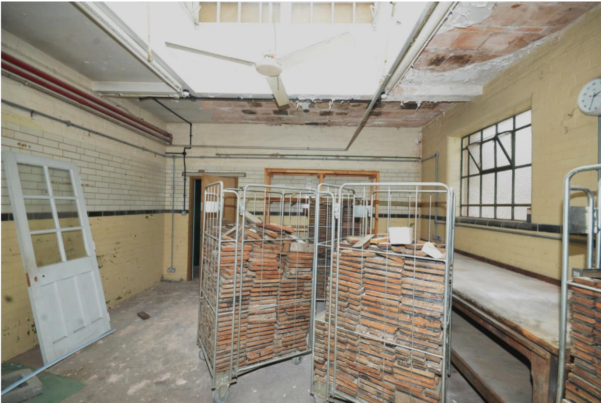
Plate 112: Southwest aspect, room 12
