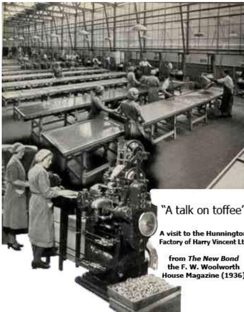
Plate 7: Internal view, 1936 (The New Bond, F. W. Woolworth House Magazine)
