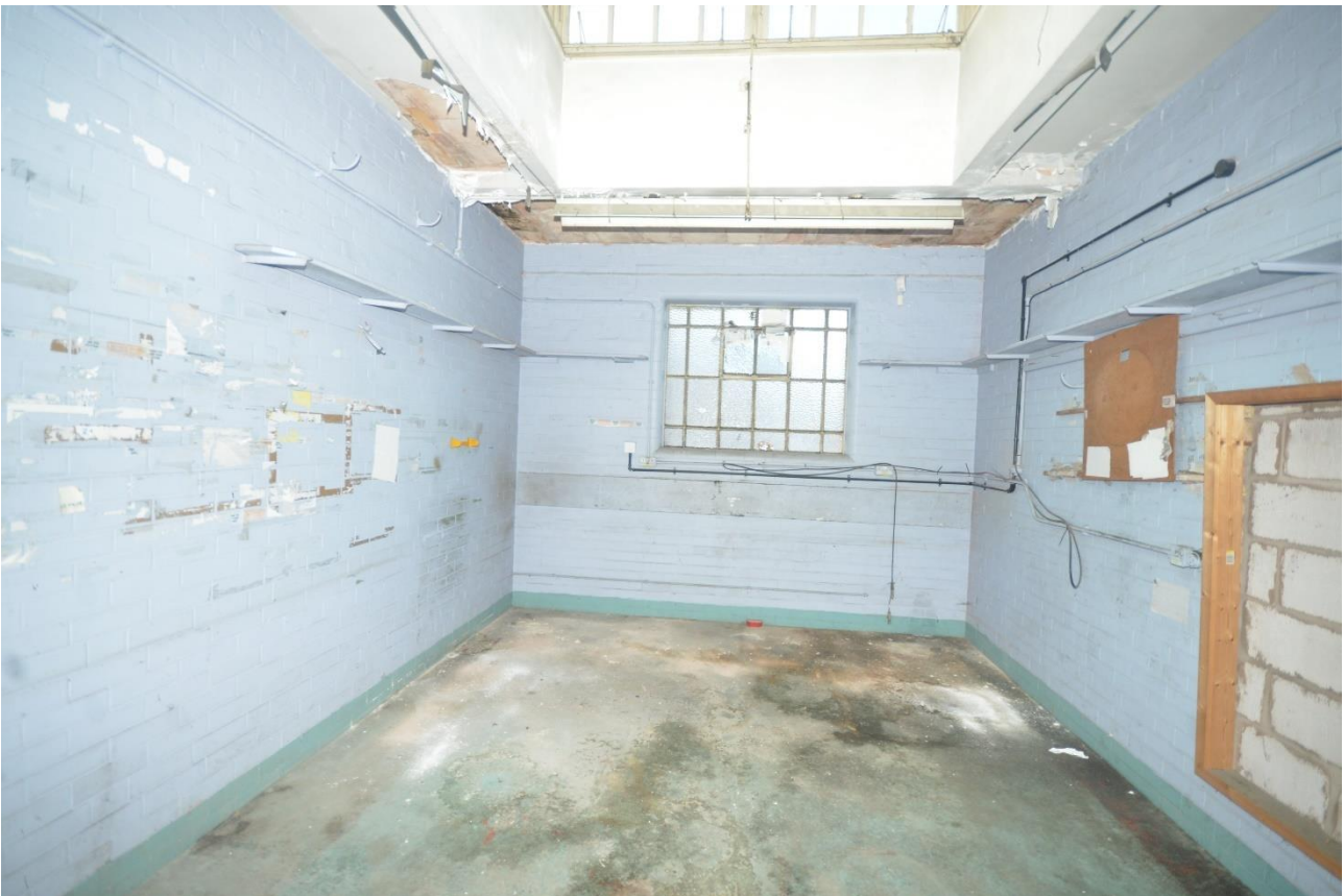
Plate 108: Northwest aspect, room 10
