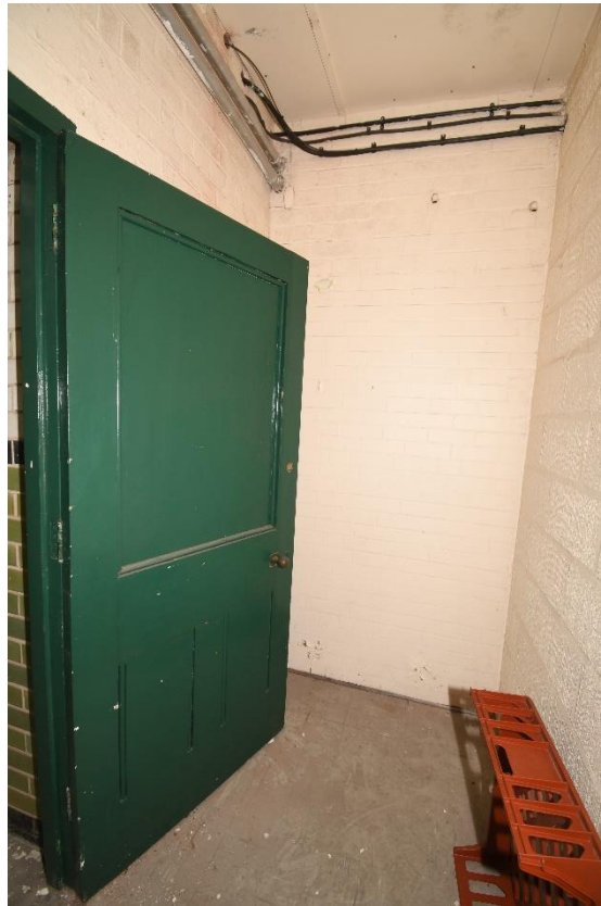
Plate 110: Southwest aspect, room 11a
