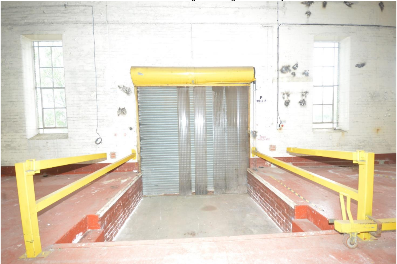
Plate 89: Detail of loading bay, room 6
