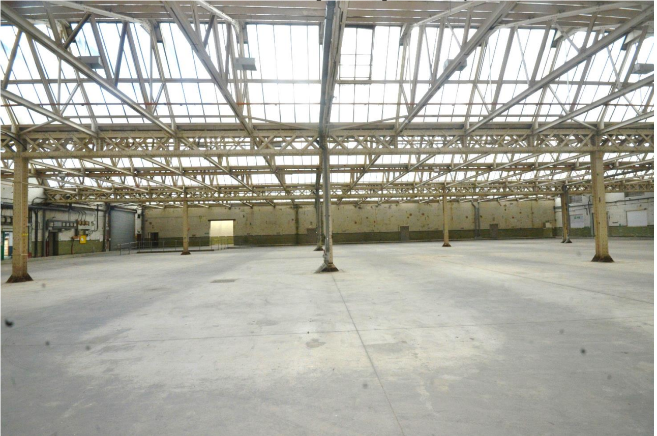
Plate 64: Northeast aspect, room 4
