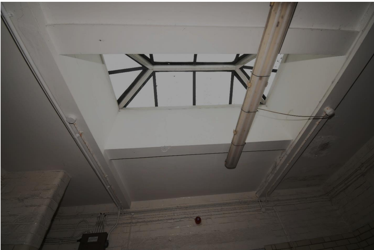
Plate 103: Detail of lantern over room 9
