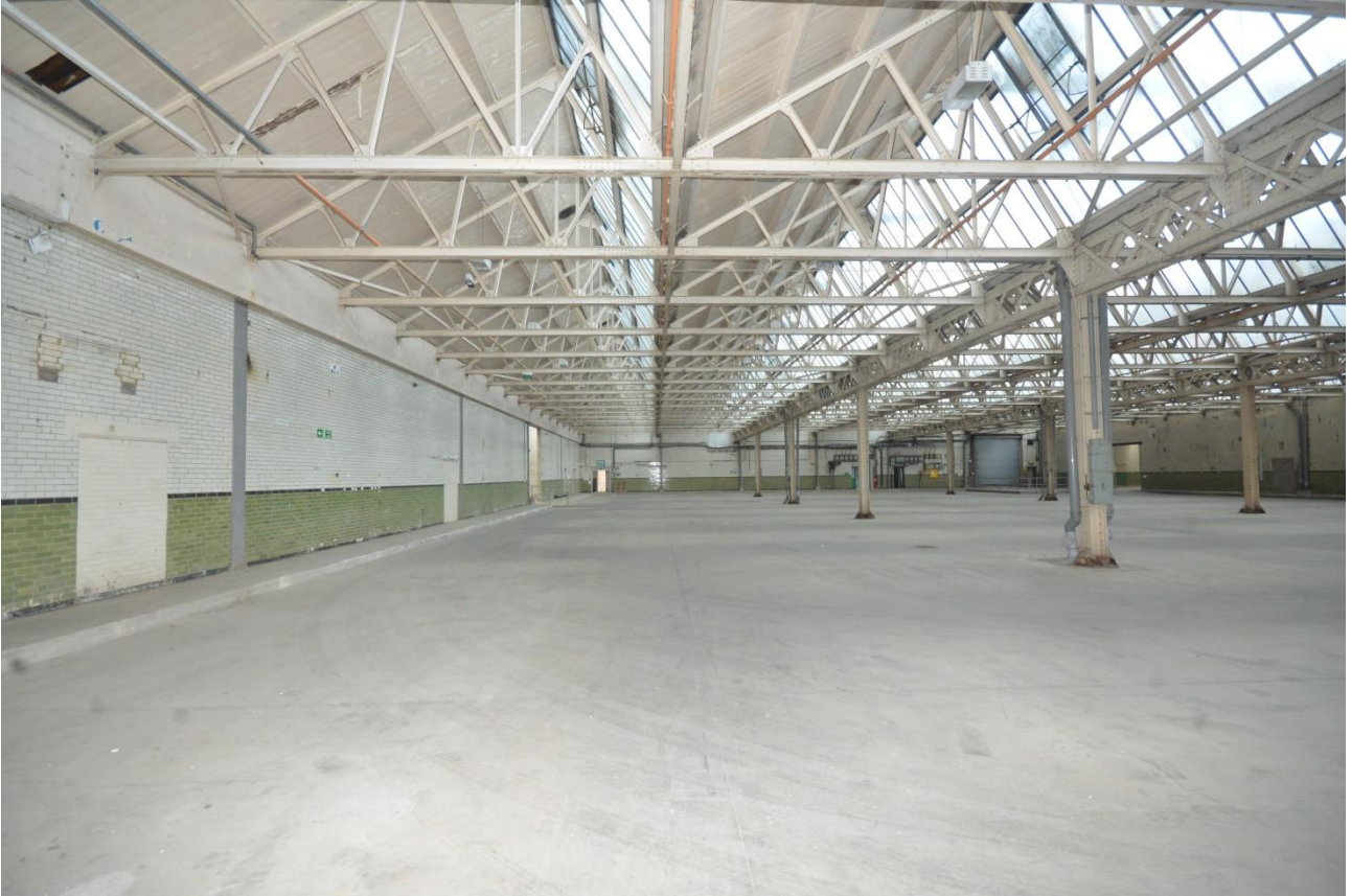
Plate 63: Northwest aspect, room 4
