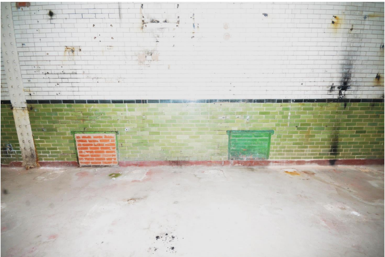
Plate 80:Detail of blocked openings in northeast wall
