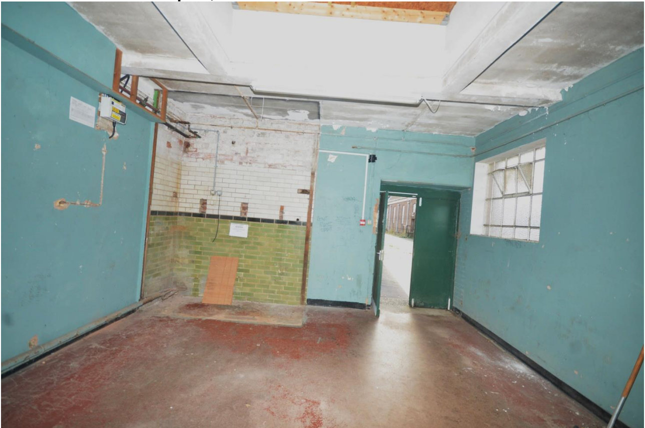
Plate 115: Southwest aspect, room 13
