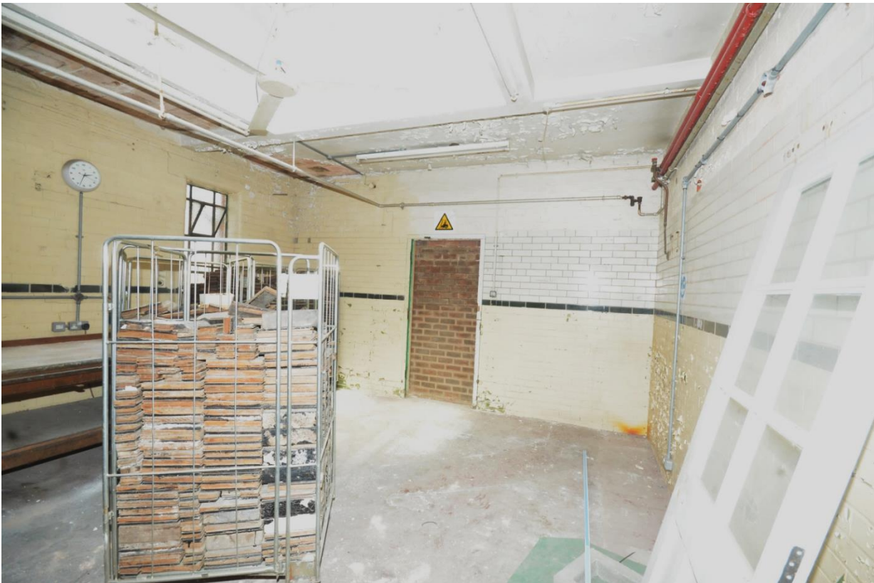
Plate 111: Northeast aspect, room 12
