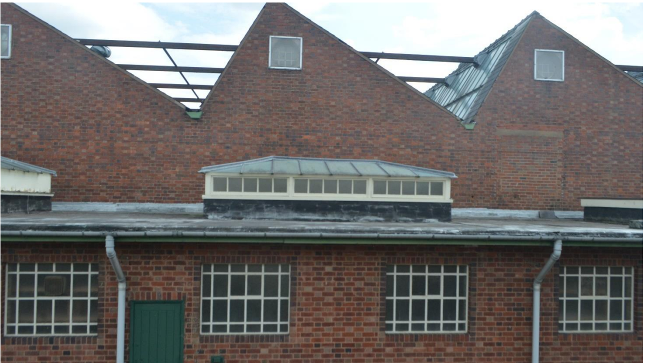
Plate 46: Detail of lantern over room 9
