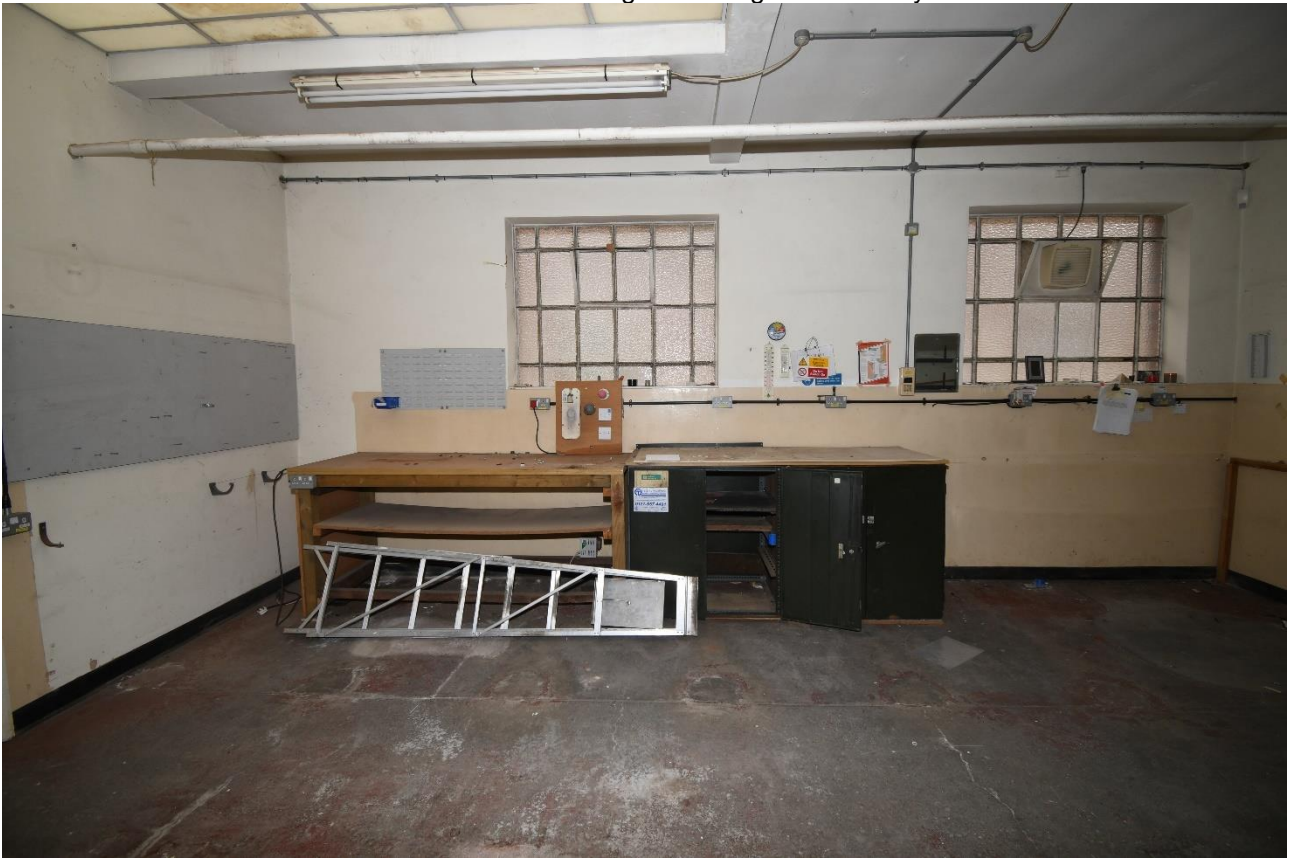
Plate 93: Northwest aspect, room 7
