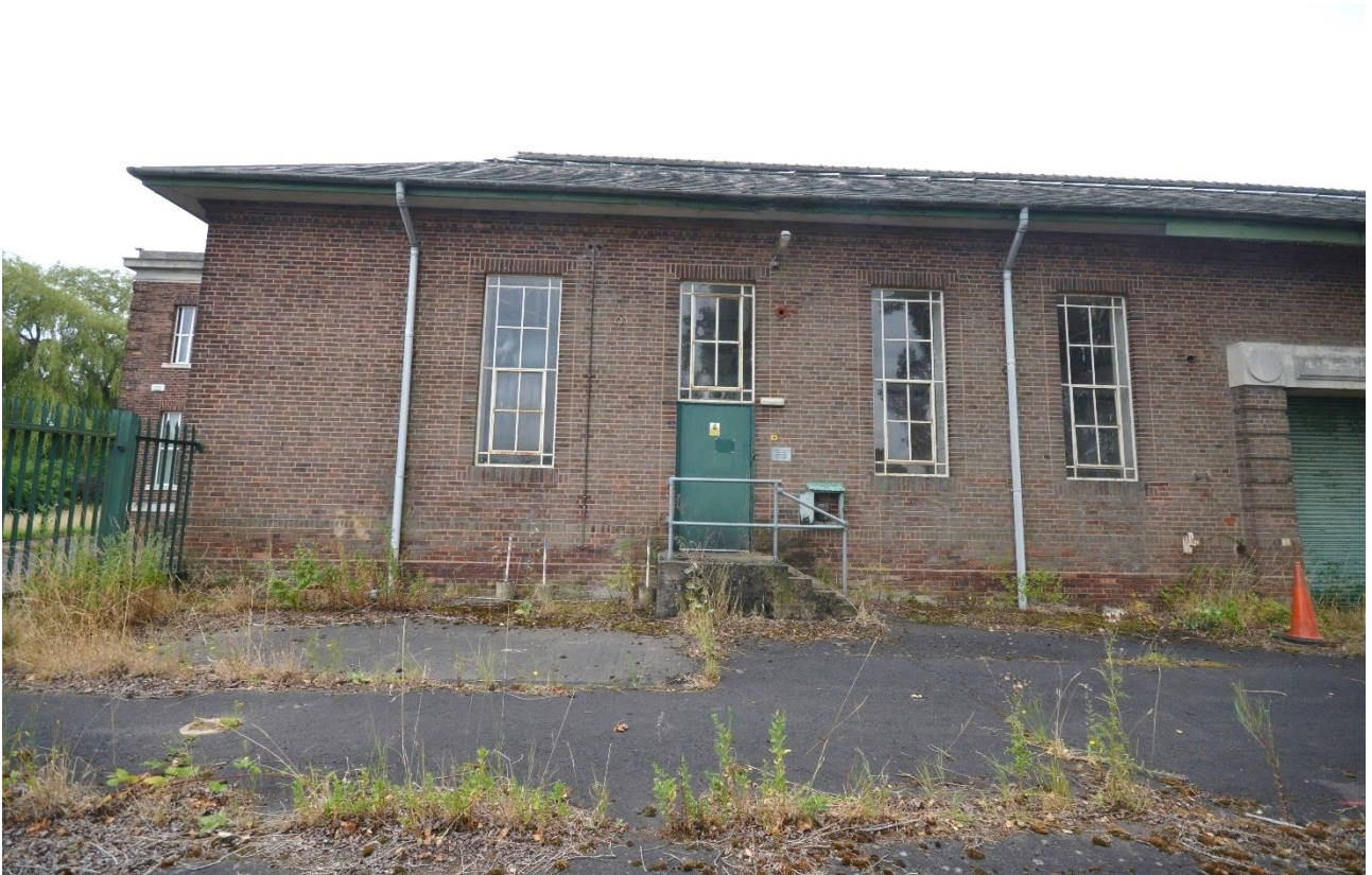
Plate 36: Southeast part, northeast elevation
