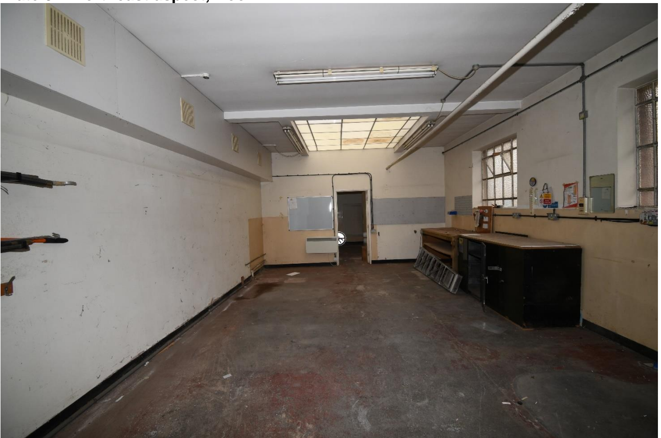
Plate 92: Southwest aspect, room 7
