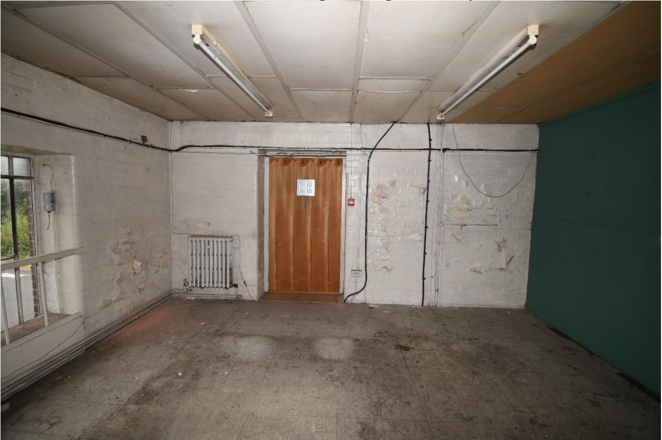
Plate 129: Southwest aspect, mezzanine room 2
