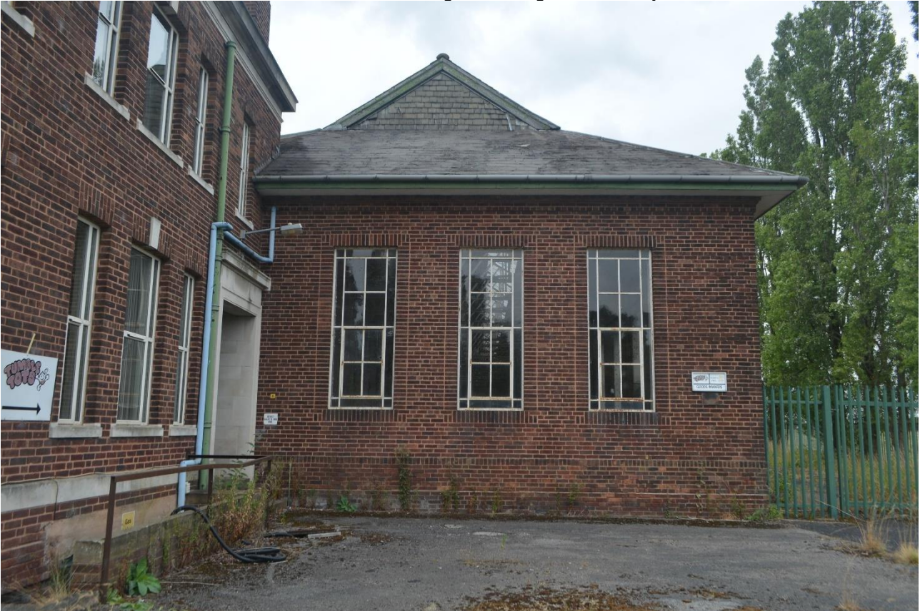
Plate 49: Southeast elevation, northeast bay
