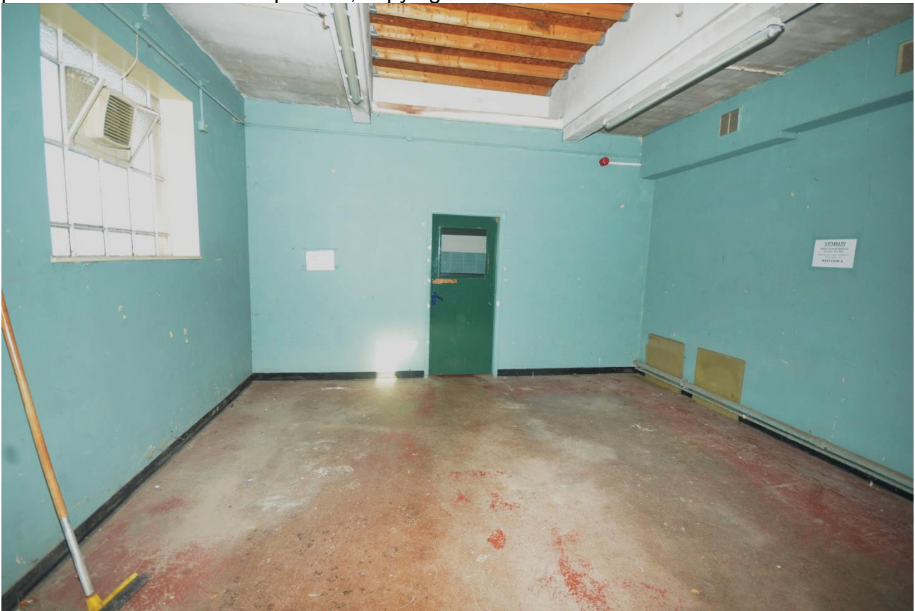
Plate 114: Northeast aspect, room 13
