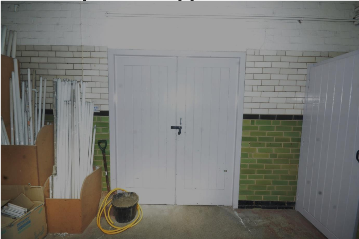
Plate 100: Northeast aspect, room 8
