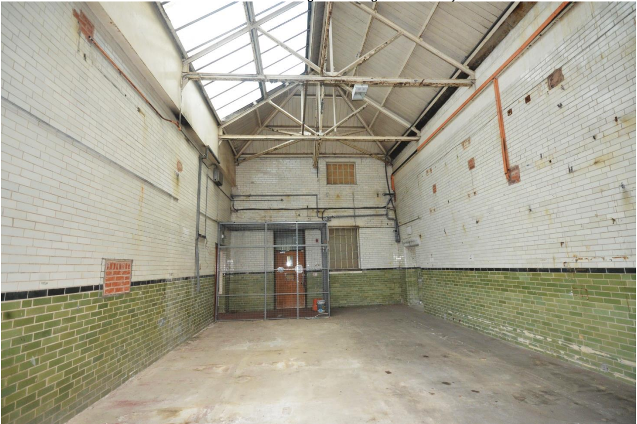
Plate 123: Door and windows to administration building in southeast wall of room 5
