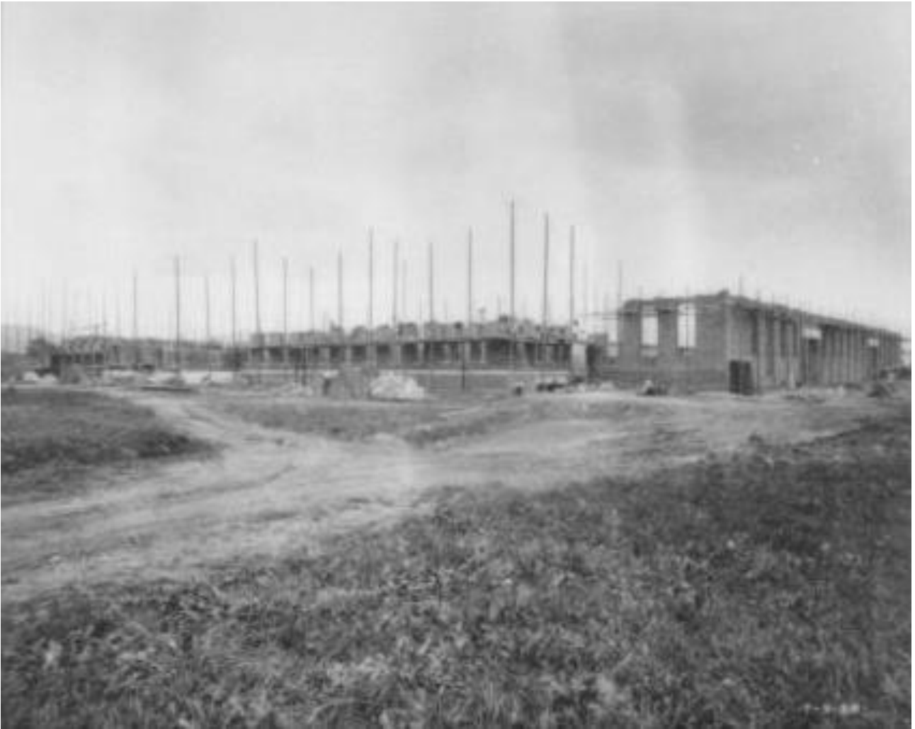
Plate 1: The manufactory under construction, 1927 (Blue Bird Album, Romsley & Hunnington His Society)
