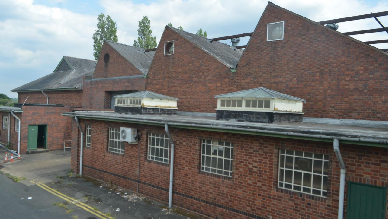
Plate 47: Detail of lanterns over rooms 10 and 12
