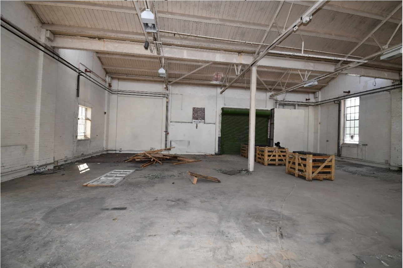
Plate 29: Southwest aspect following removal of southern partition stud walls
