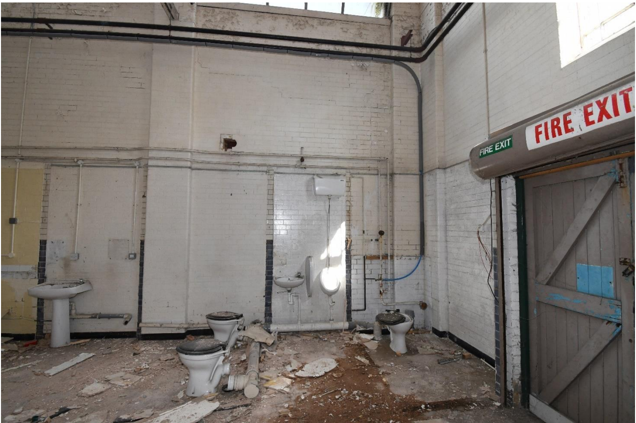
Plate 28: Area of lavatories following removal of stud walls
