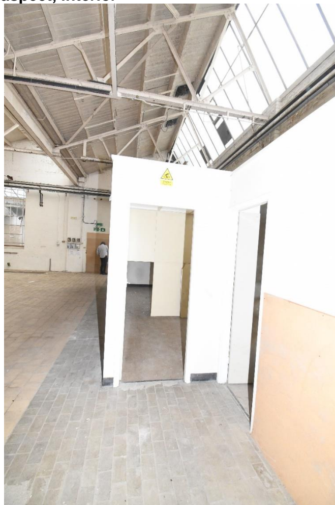
Plate 22: View into partitioned rooms, northwest end of building
