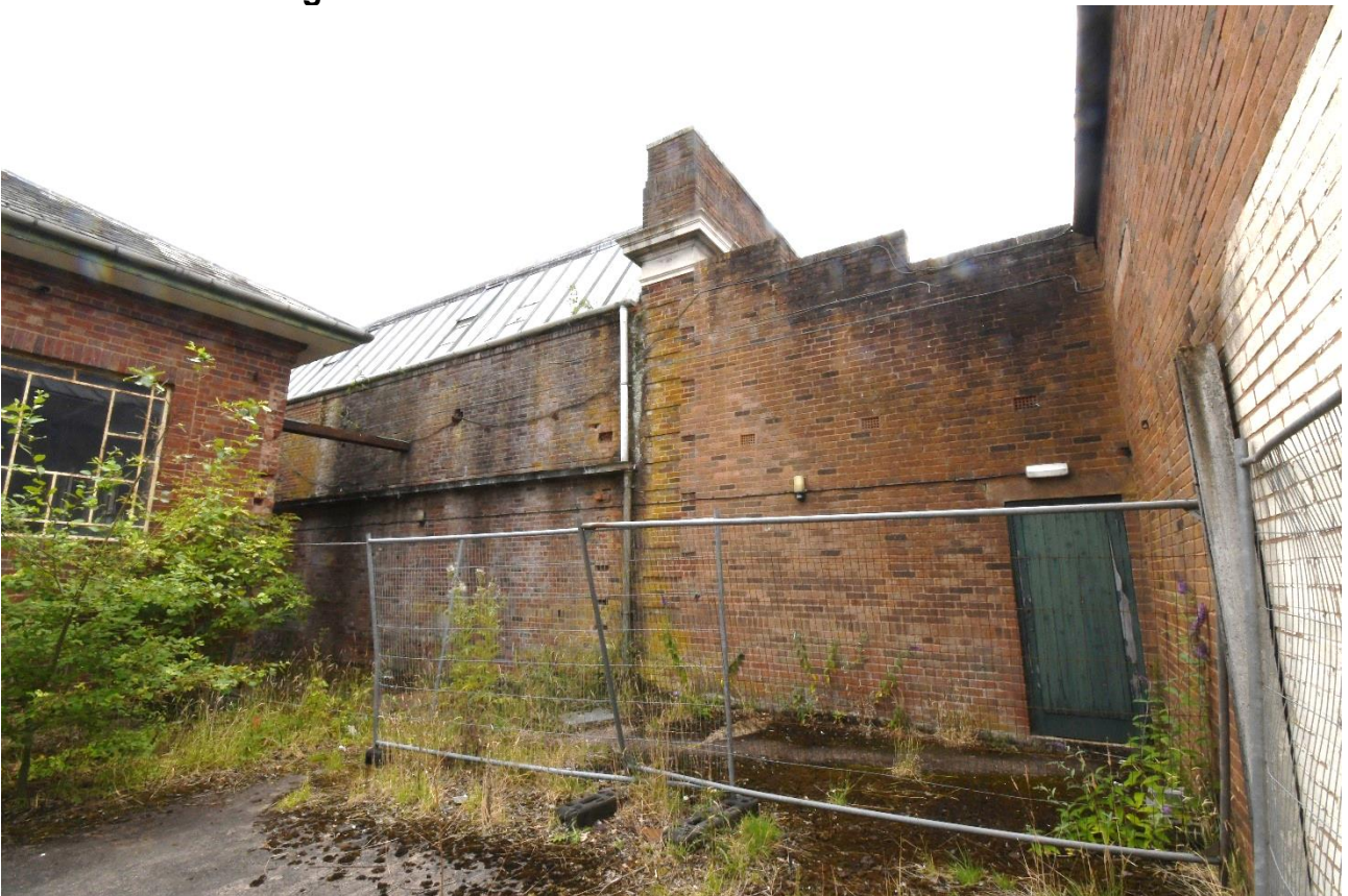
Plate 15: Northwest part, northeast wall
