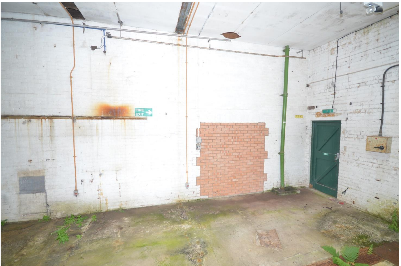
Plate 26: Northeast end of extension
