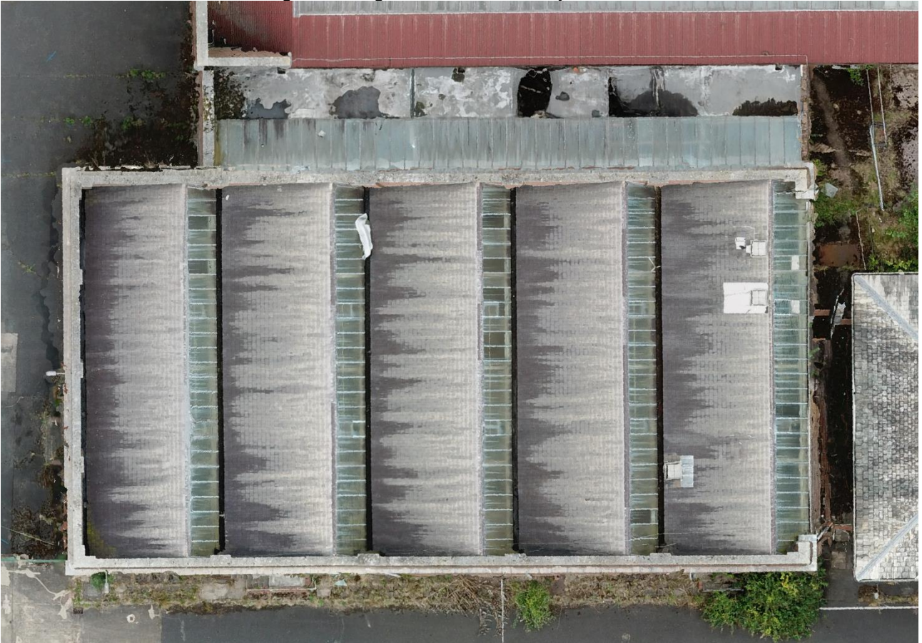
Plate 16: Detail of roof from 2022 survey
