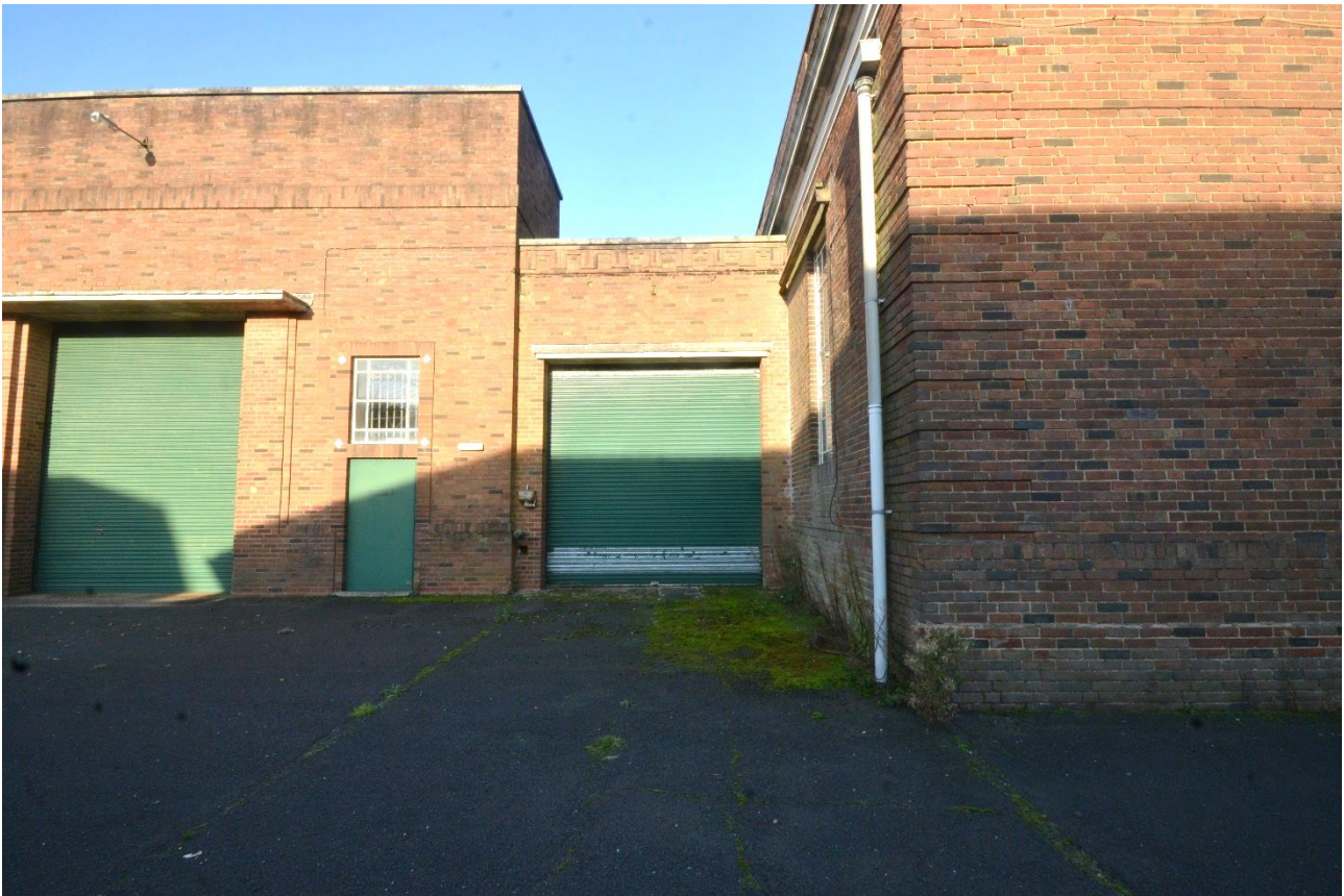
Plate 9: Southwest elevation, northwest extension
