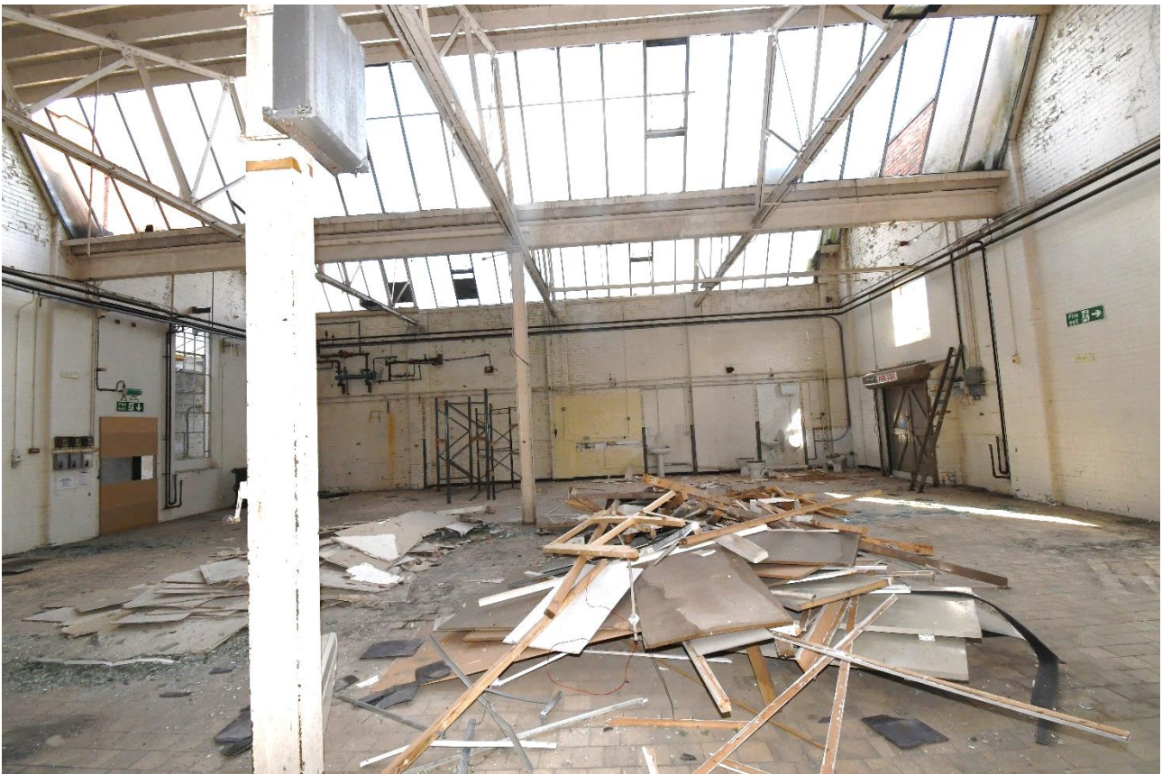
Plate 27: Area of northeast partition rooms following removal of recent stud walls
