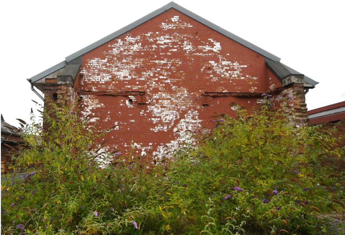
Plate 26: Interior of southwest wall (northeast wall of power house)
