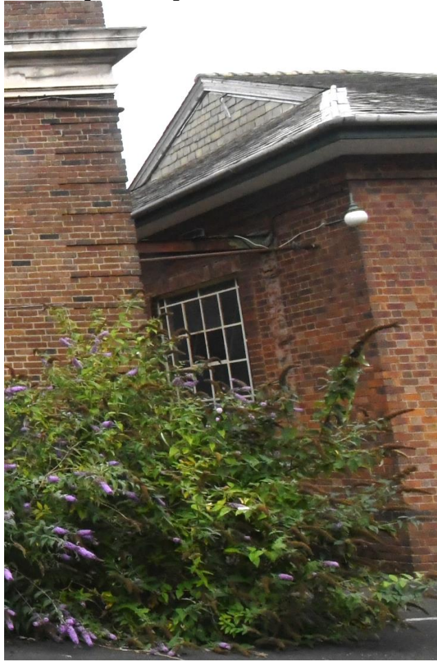
Plate 8: View of window in southwest wall
