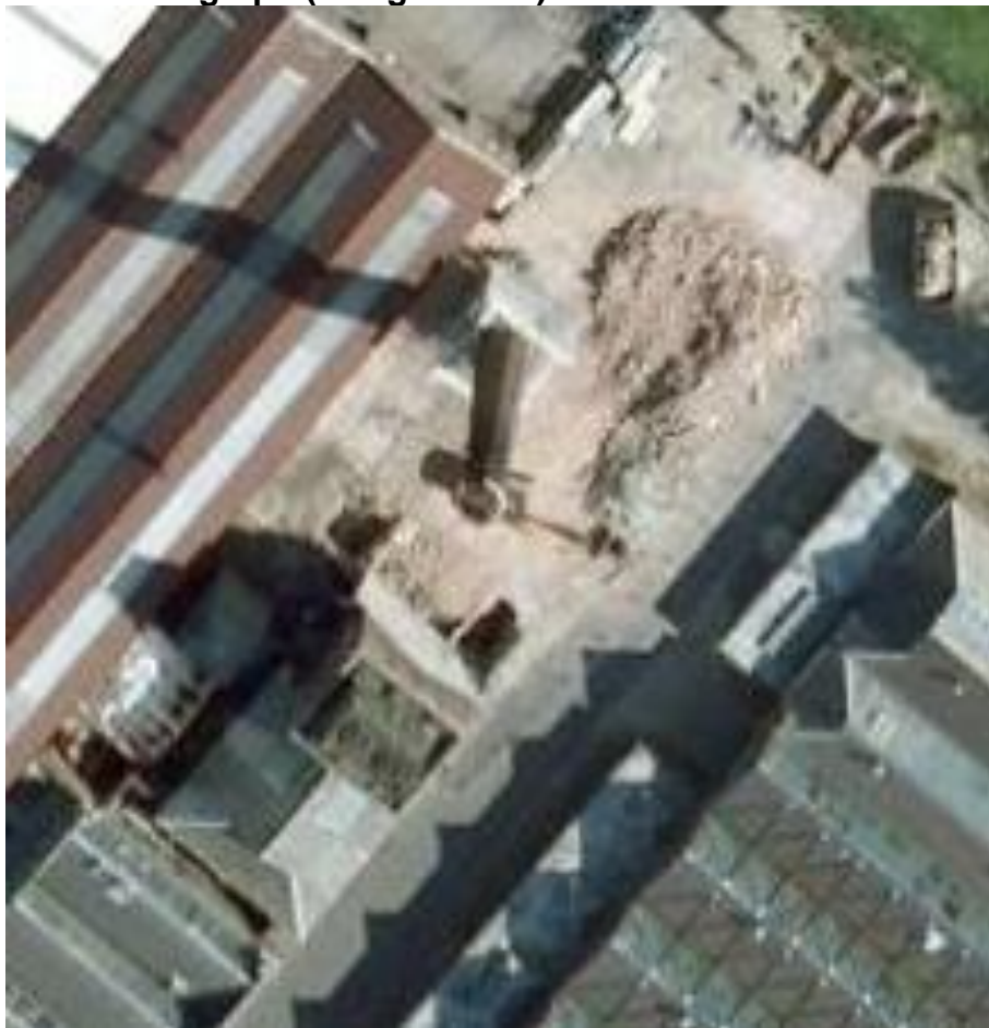
Plate 13: 2007 Air Photograph, partway through demolition of boiler house (Google Earth)
