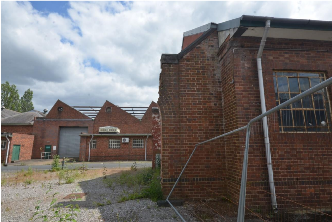
Plate 24: Stub of northwest wall of boiler house, showing start of arch
