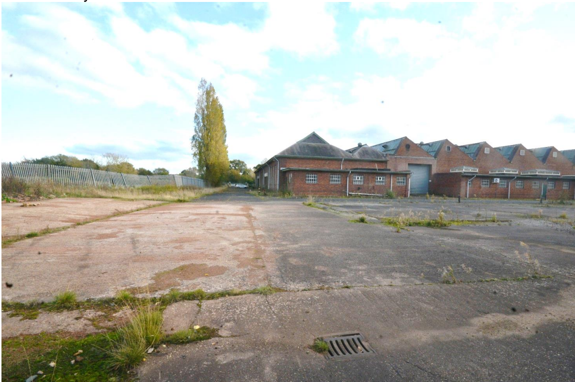
Plate 27: Concrete slab viewed from the northeast, looking towards the manufactory
