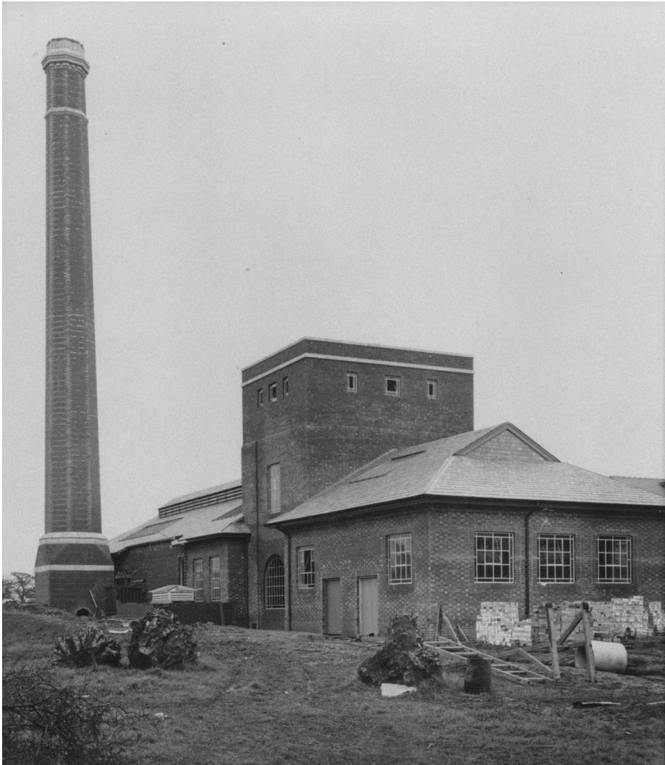
Plate 29: Rear of power house and boiler house viewed from the west, December 1926 (Romsley & Hunnington History Society)
