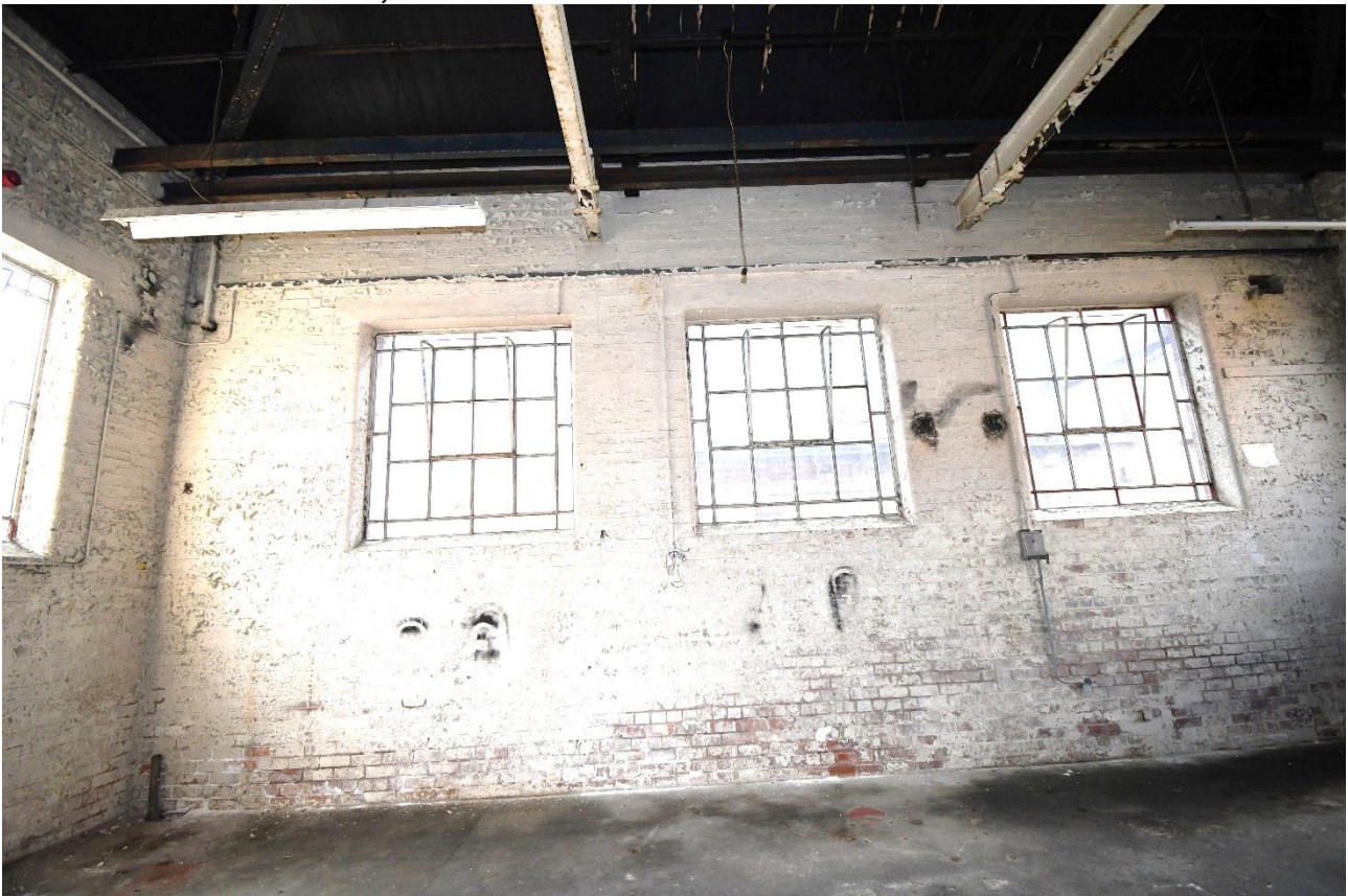
Plate 18: Southwest elevation, southwest room
