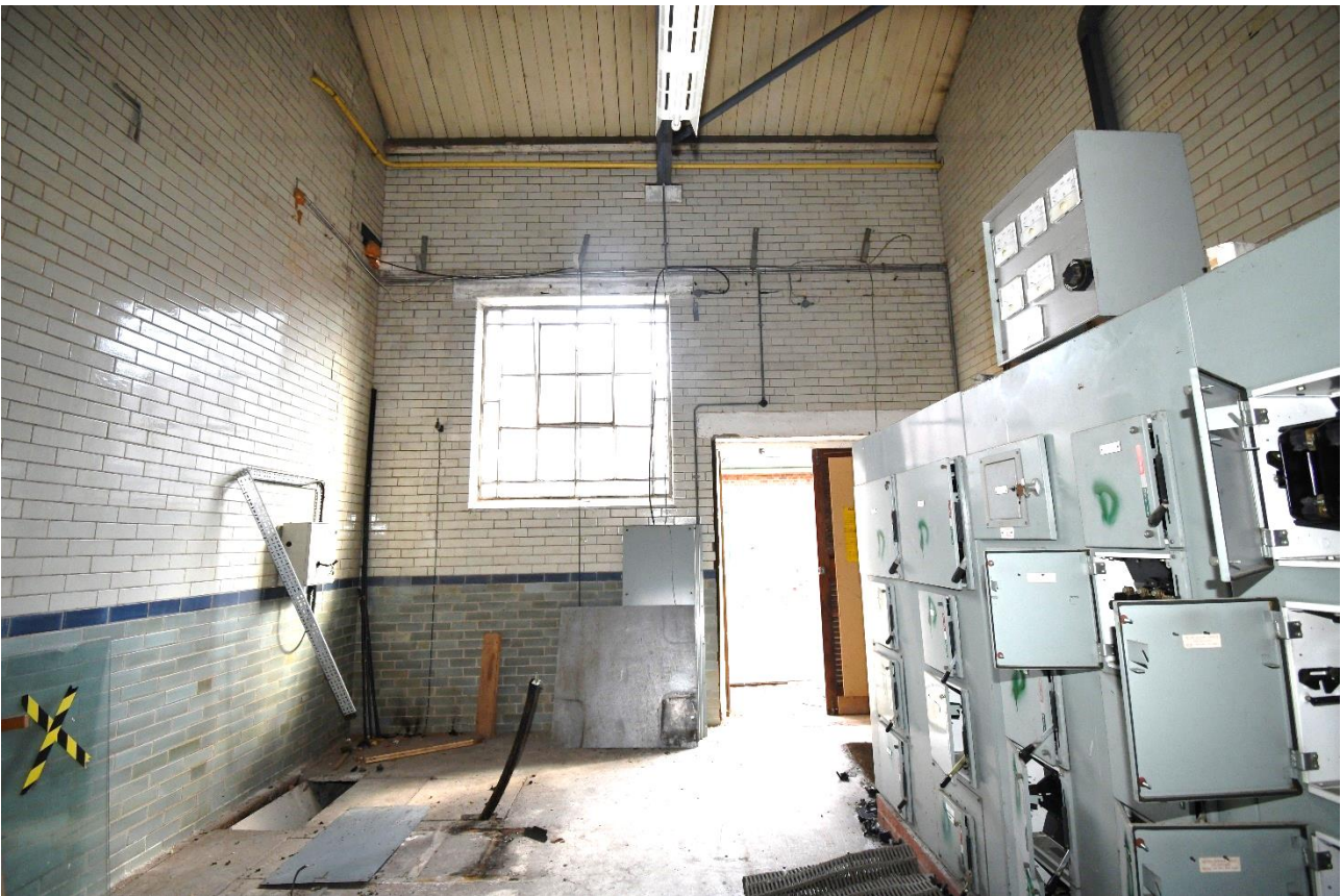
Plate 23: Southeast aspect, northeast room
