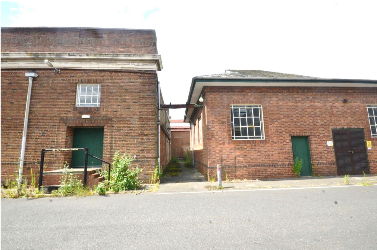
Plate 7: View between laboratory and power house
