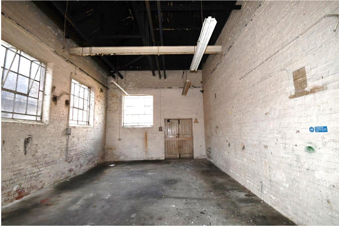
Plate 15: Northwest aspect, southwest room
