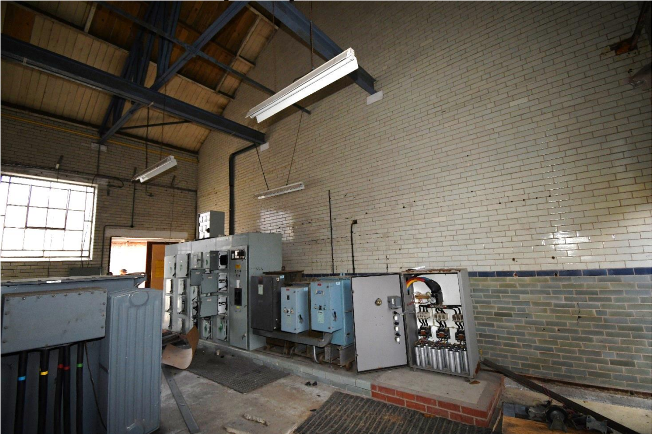
Plate 21: Southern corner, northeast room
