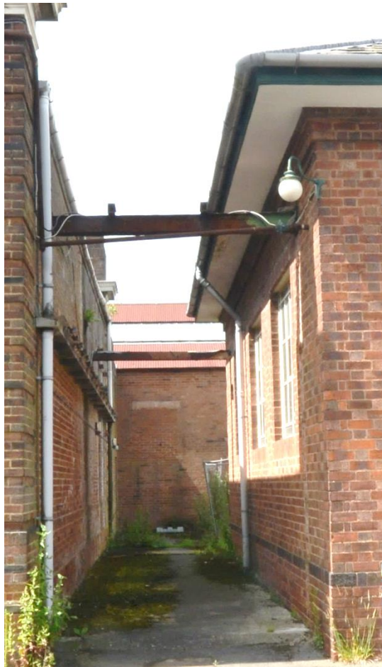
Plate 9: View from the southeast along southwest wall
