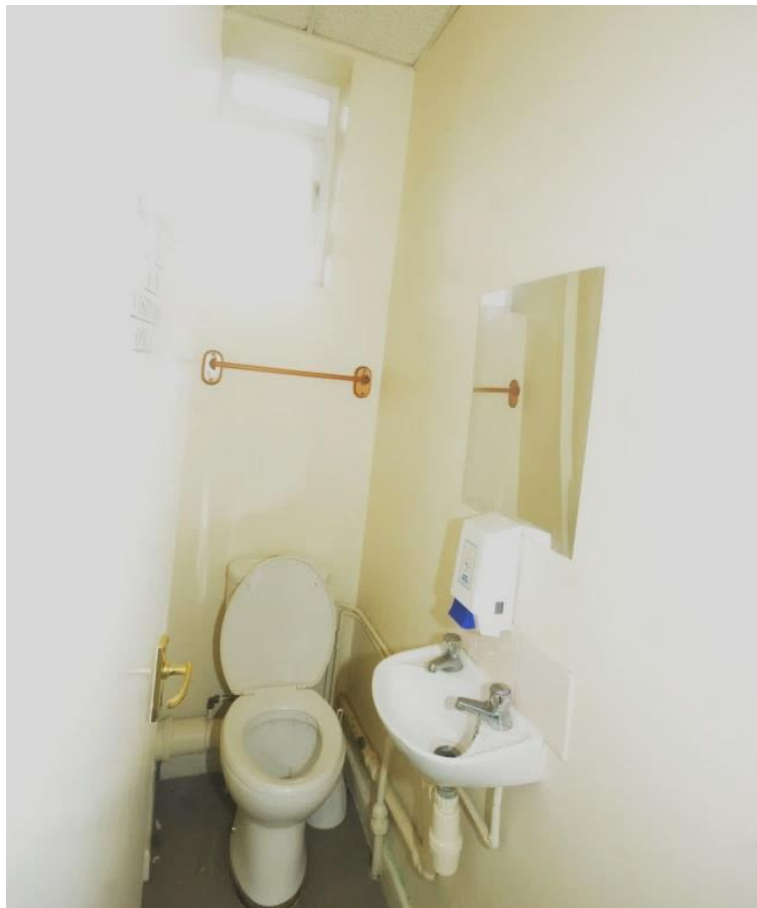
Plate 34: SW aspect, lavatory
