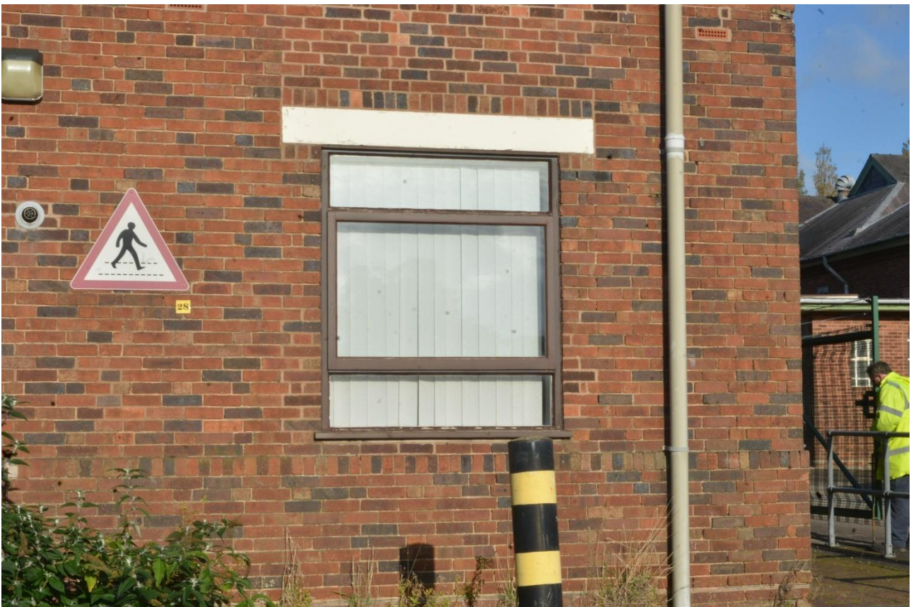
Plate 22: Detail of window, southwest elevation
