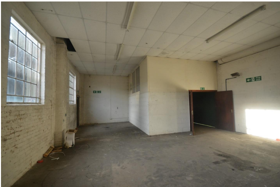
Plate 44: Northwest aspect, room 9
