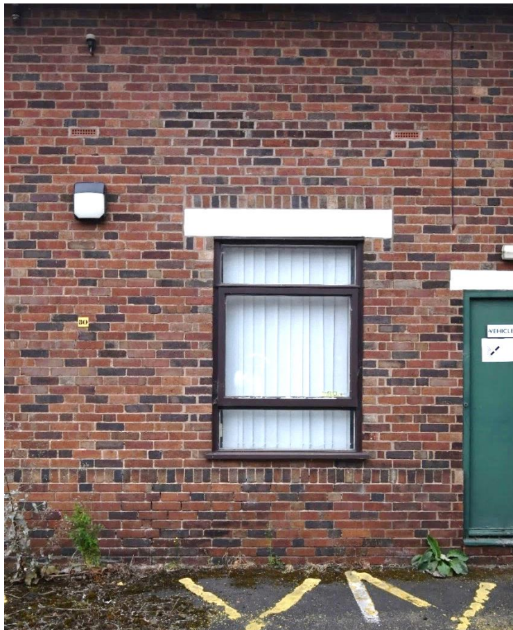
Plate 12: Detail of window, northeast elevation
