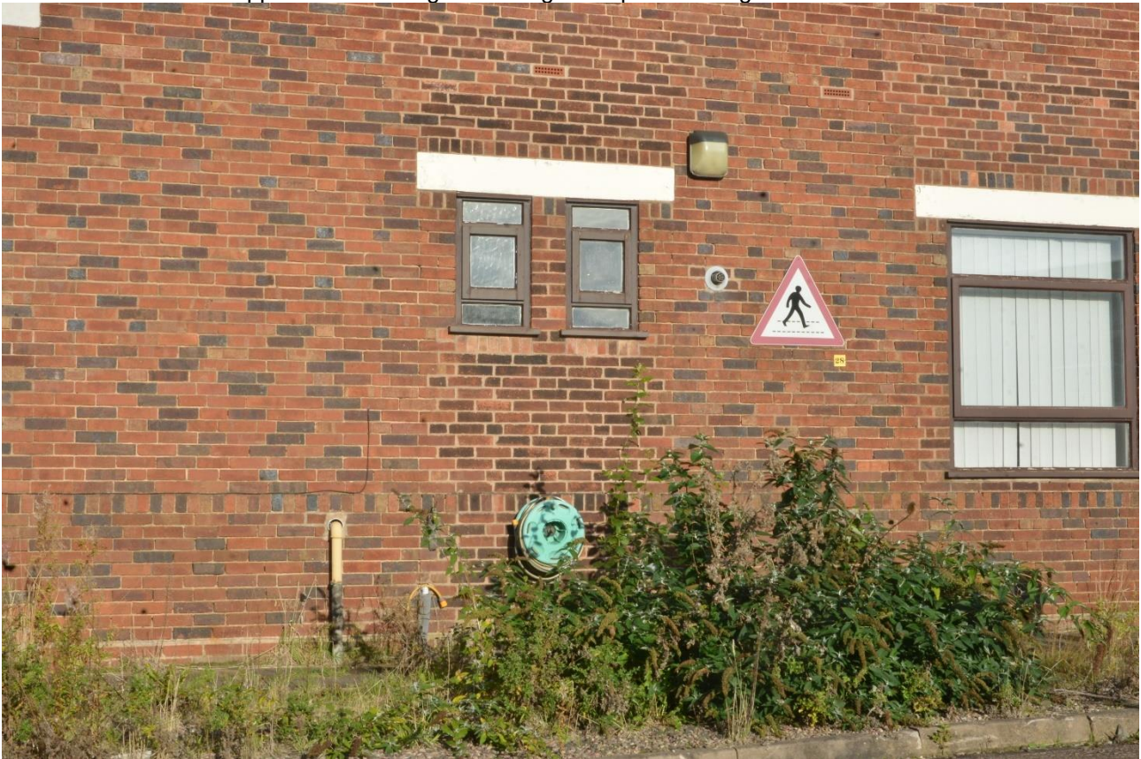
Plate 21: Detail of windows, southwest elevation
