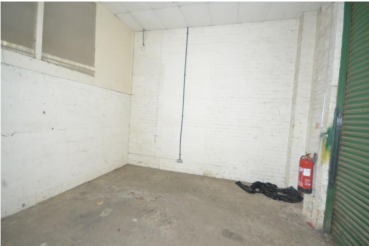
Plate 48: Northwest aspect, room 10
