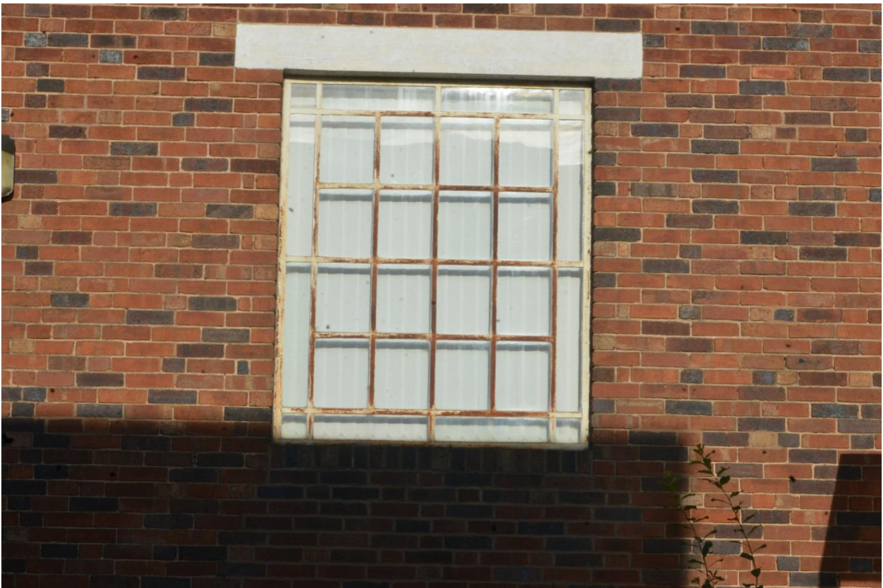
Plate 20: Detail of window, southwest elevation
