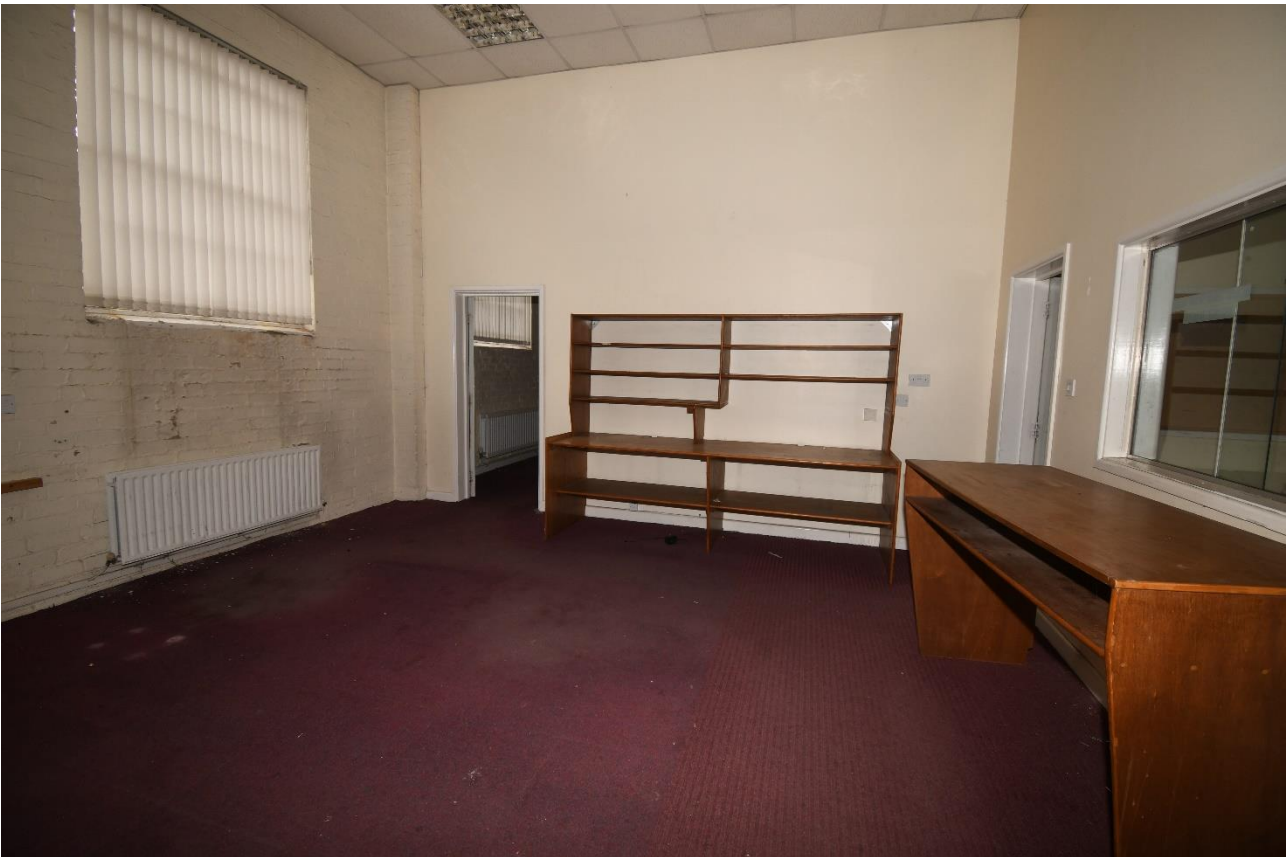
Plate 35: Northwest aspect, room 6
