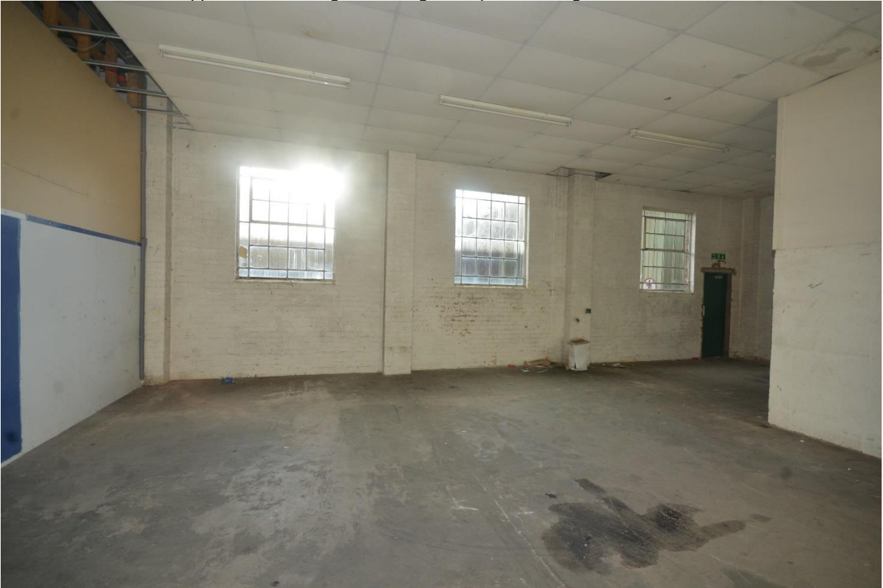
Plate 47: Southwest aspect, room 9
