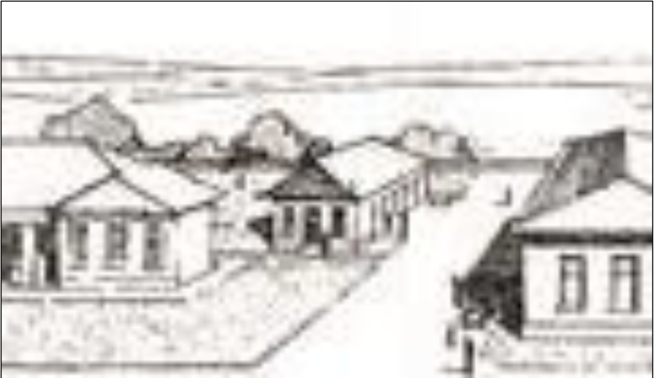
Figure 3: Detail of transport building from 1927 Midlander article
