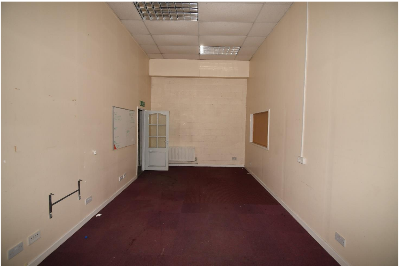
Plate 43: Northeast aspect, room 8
