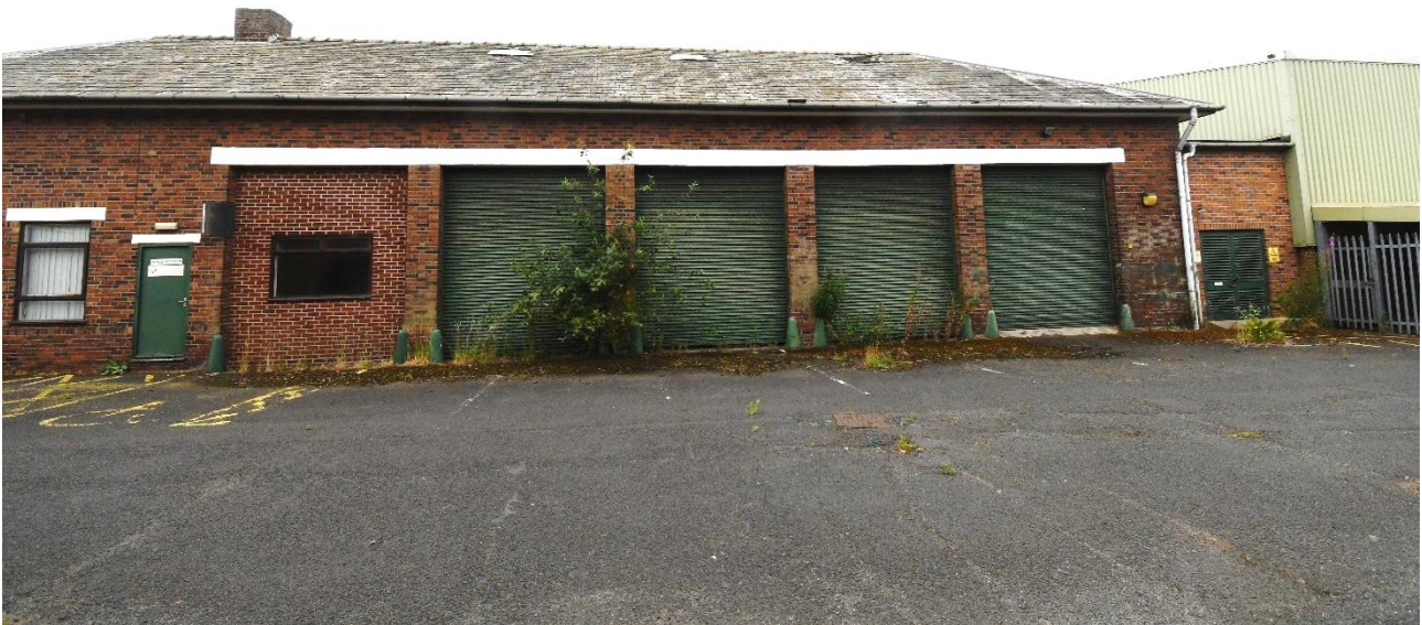
Plate 10: Northwest part of northeast elevation
