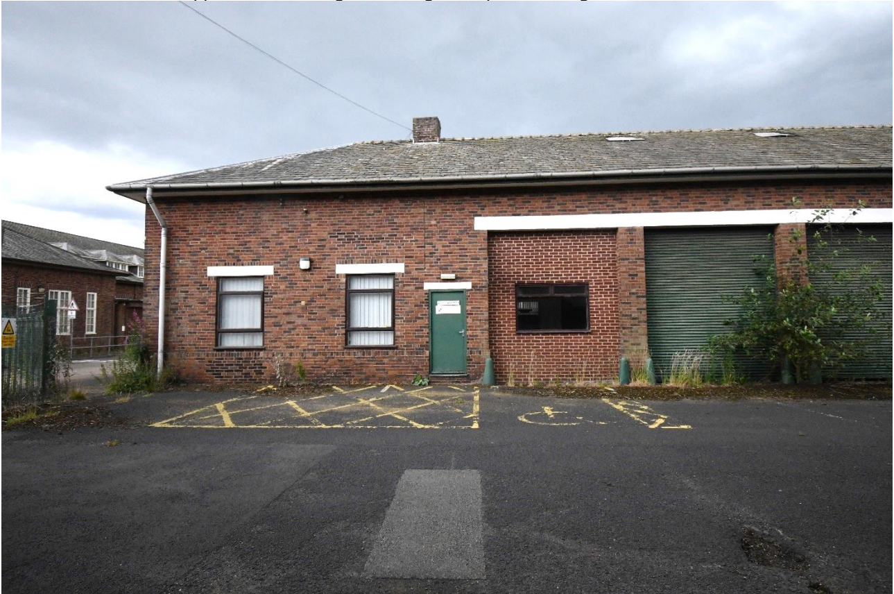
Plate 9: Southeast part of northeast elevation
