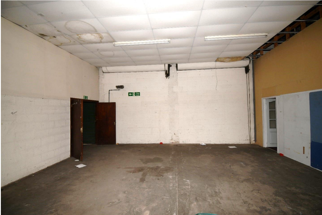
Plate 45: Southwest aspect, room 9
