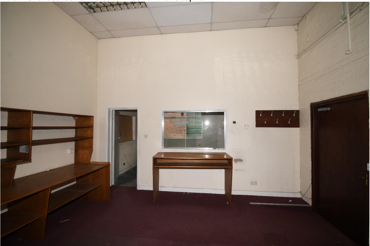
Plate 36: Northeast aspect, room 6
