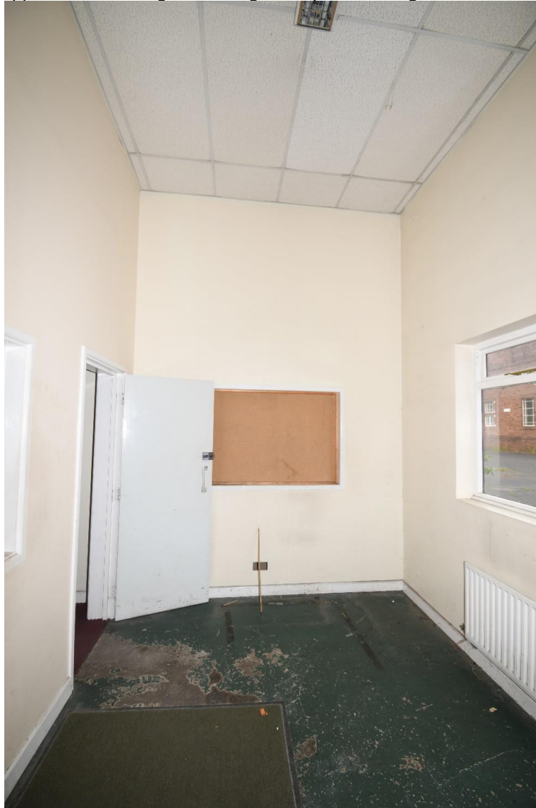
Plate 41: Northwest aspect, room 7
