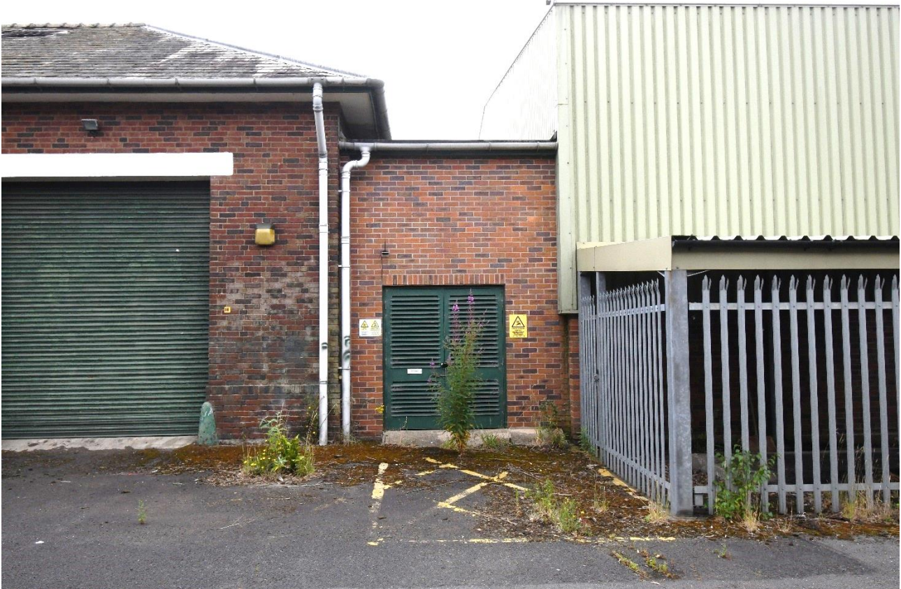
Plate 11: Link between transport building and building 11
