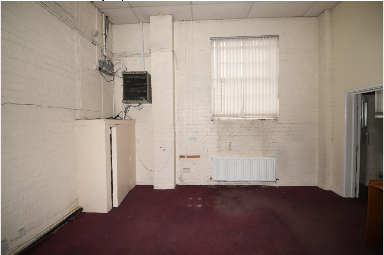
Plate 38: Southwest aspect, room 6
