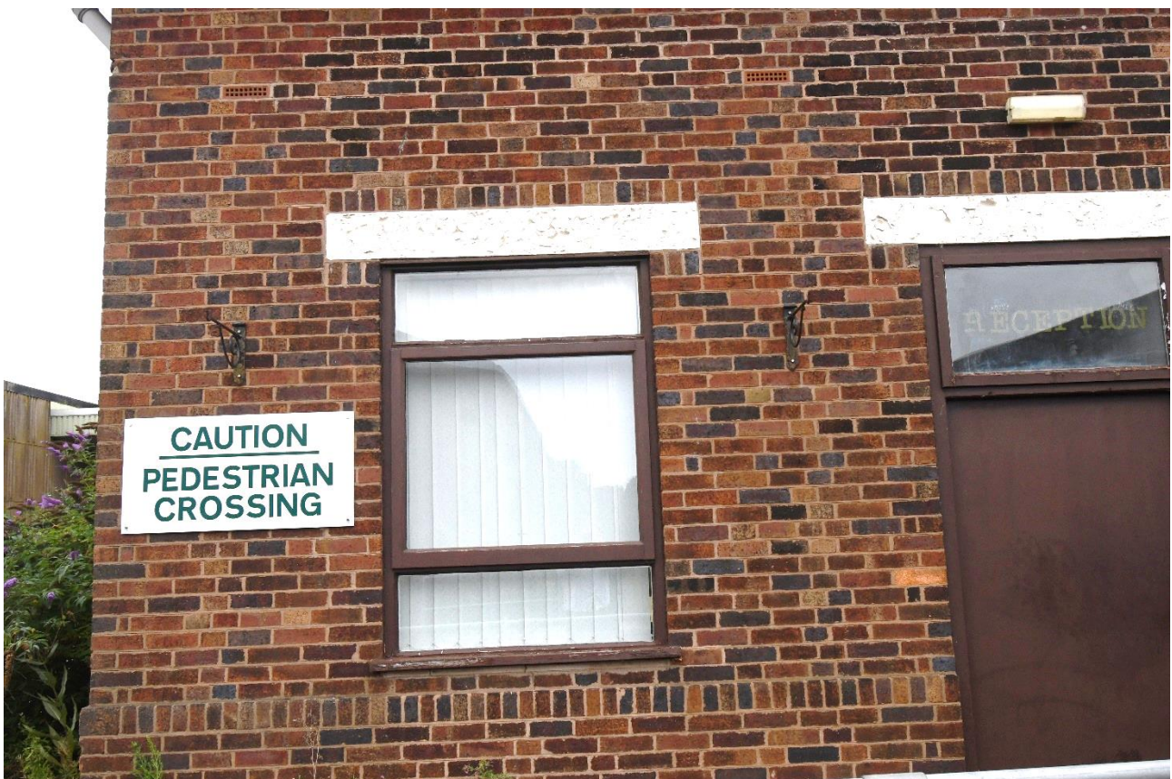
Plate 16: Detail of southeast window
