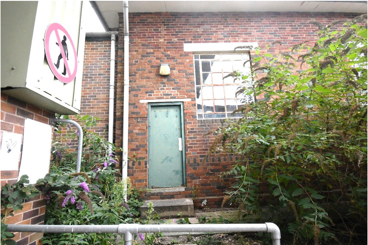
Plate 19: Detail of door and window, northwest end of southwest elevation
