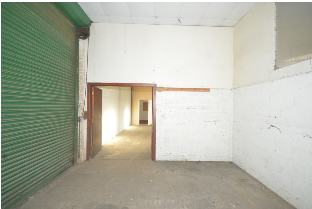
Plate 49: Southwest aspect, room 10
