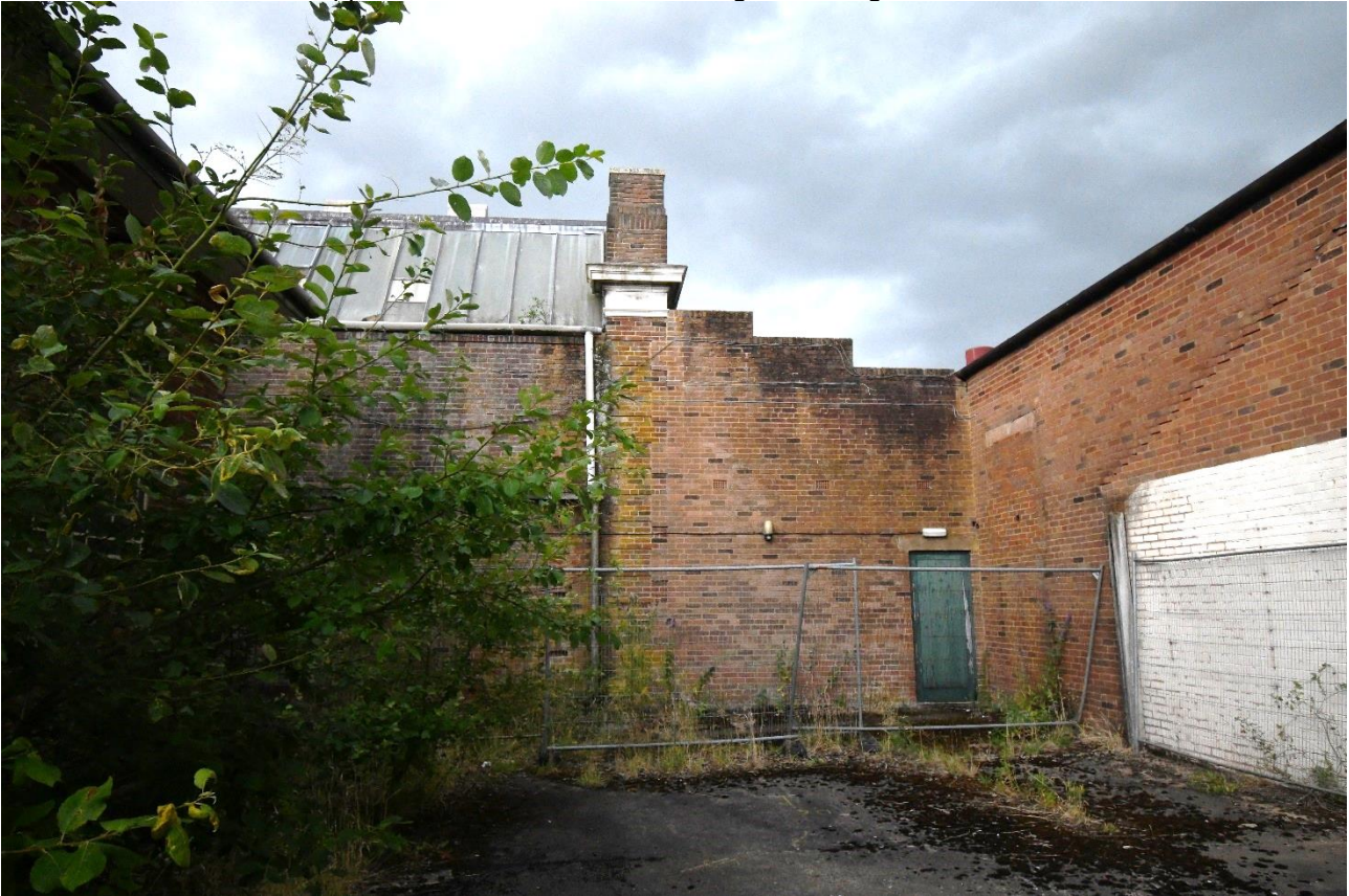
Plate 13: Join between warehouse (right) and laboratory (left)
