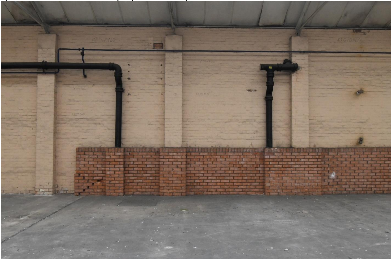
Plate 22: Detail of service pipes, southeast wall
