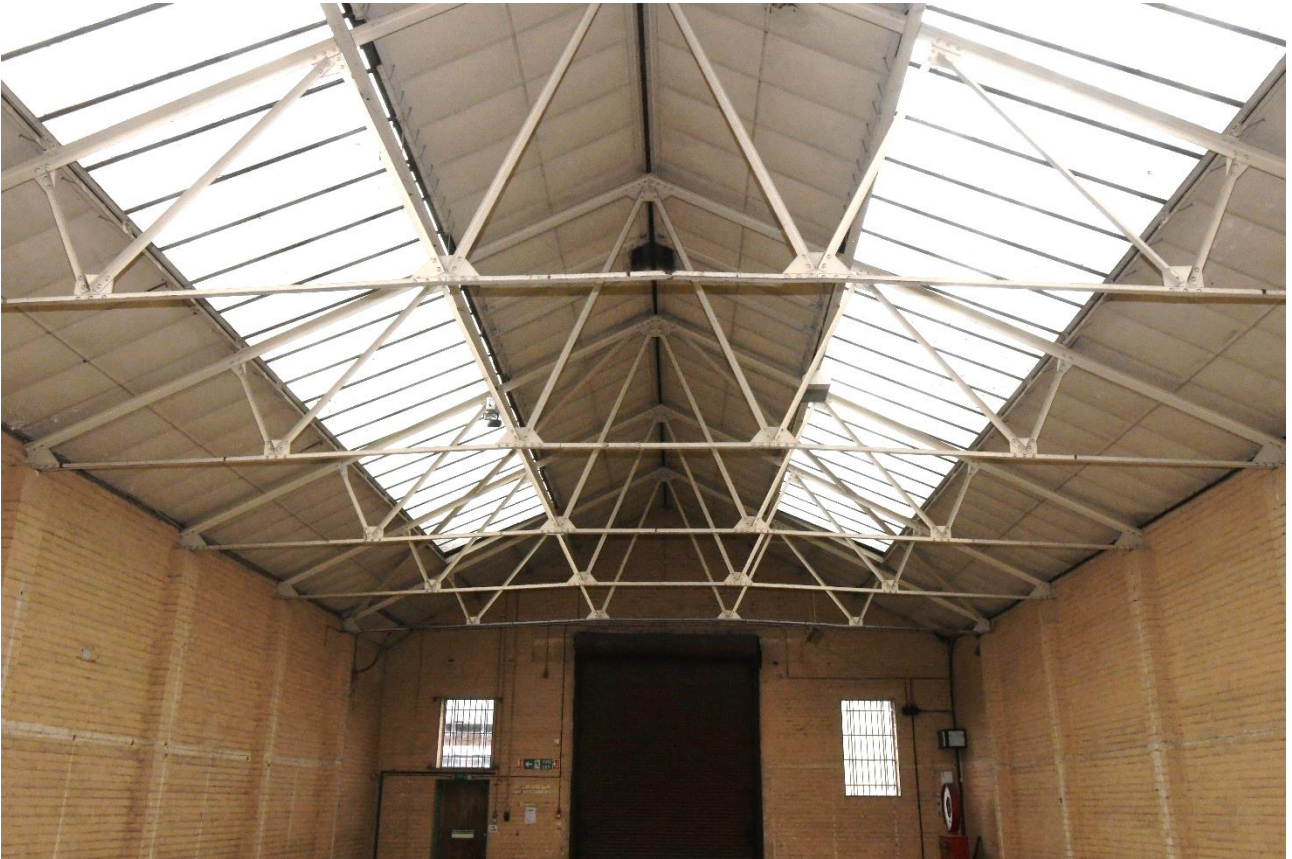
Plate 33: Detail of double fink roof structure
