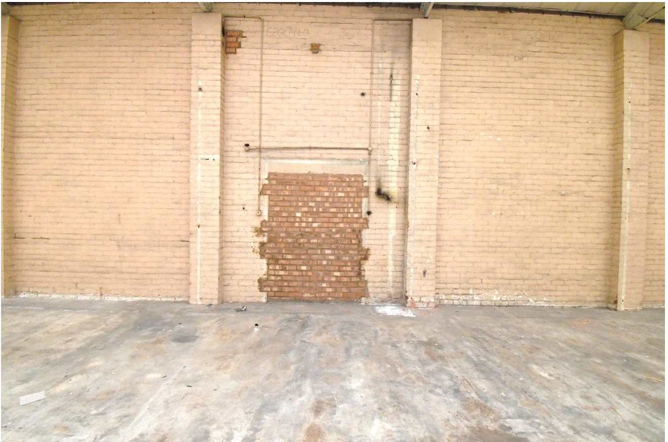
Plate 32: Detail of blocked opening in southeast wall to former boiler house
