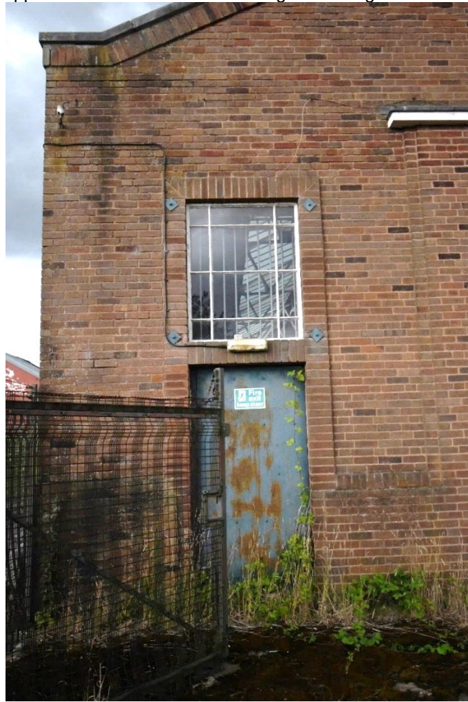
Plate 9: Detail of door and window, northeast elevation
