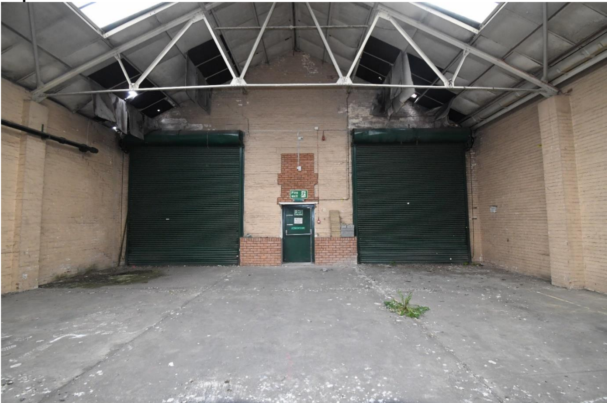
Plate 18: Detail of northeast wall
