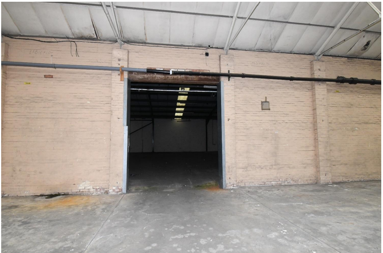
Plate 20: Opening into building 10
