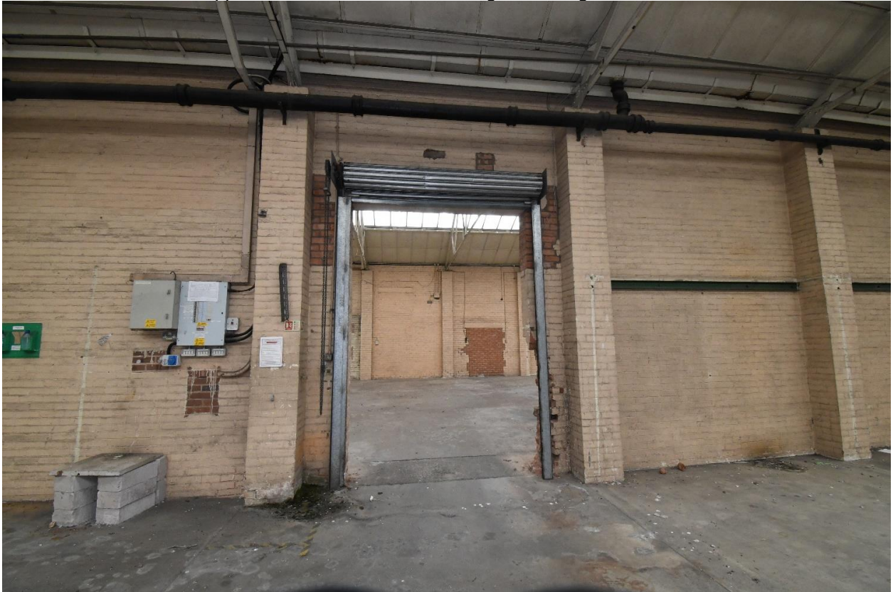
Plate 21: Opening into southeast bay, with roller shutter
