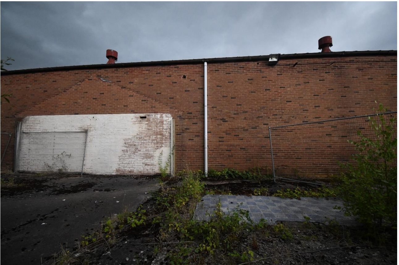
Plate 12: Central part of southeast elevation showing scar from previous building
