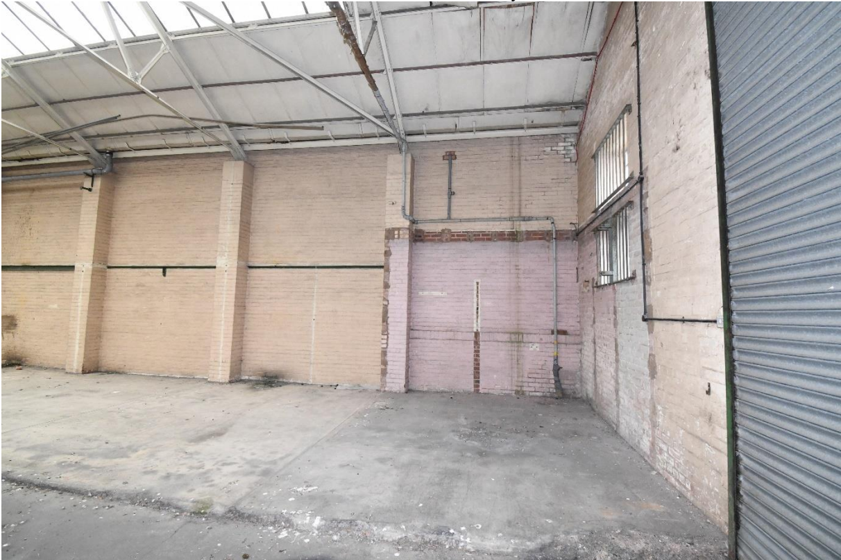
Plate 17: Detail of southwest end of southeast wall, showing barred window and scar from previous structure
