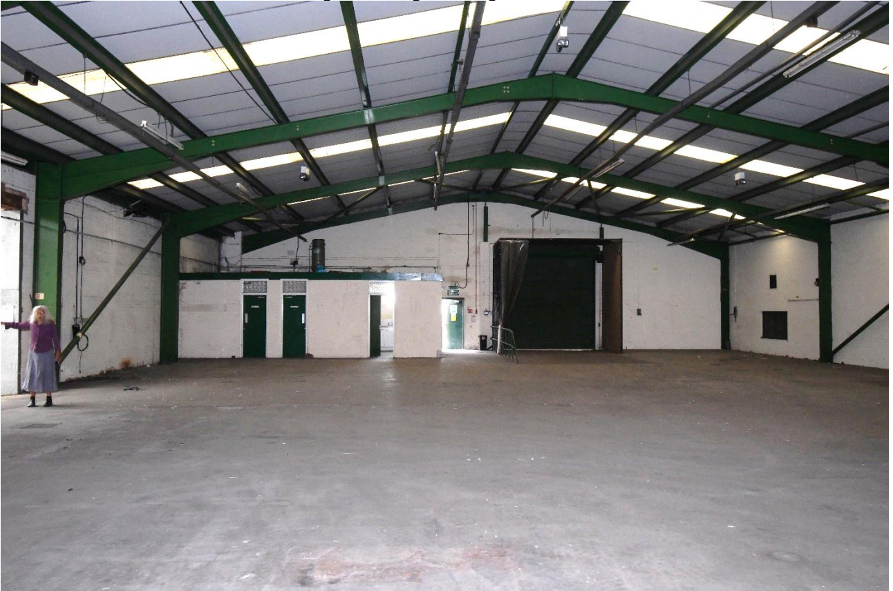
Plate 11: Southwest aspect, building 10 interior
