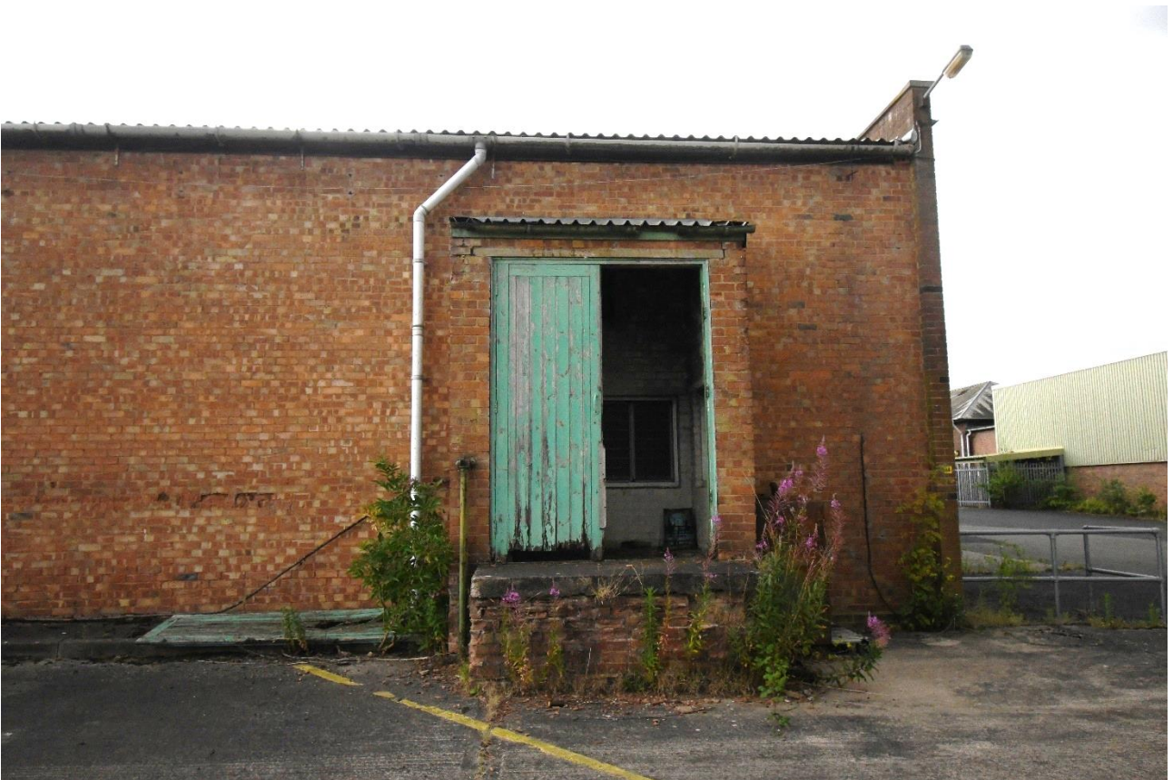
Plate 6: Detail of door, northwest elevation
