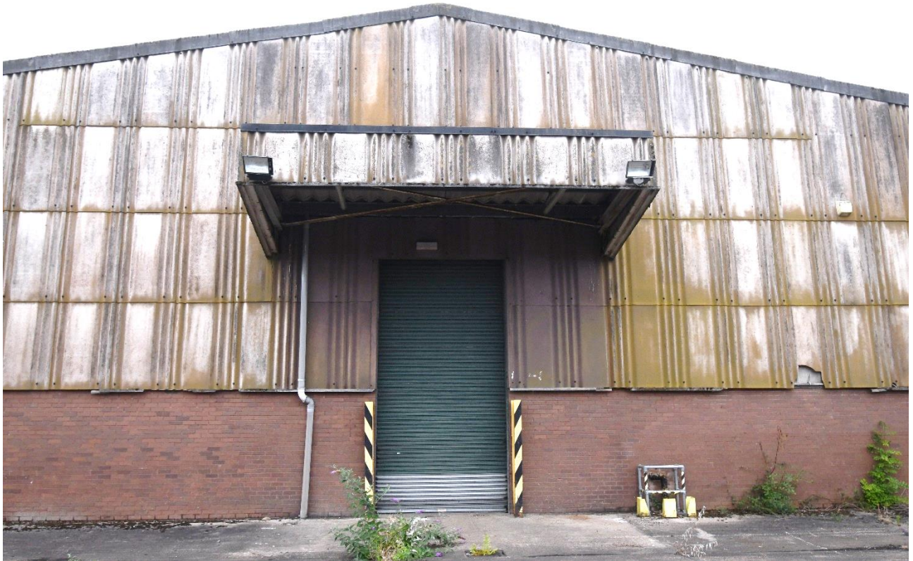
Plate 23: Central door, southeast elevation
