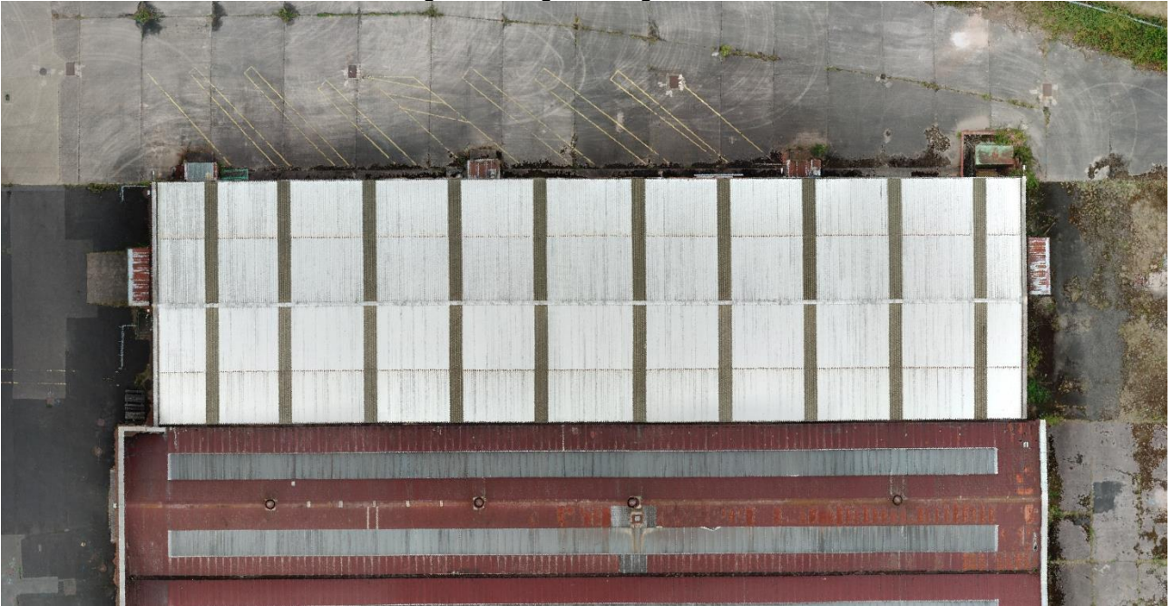
Plate 1: Aerial view, Building 10, September 2022
