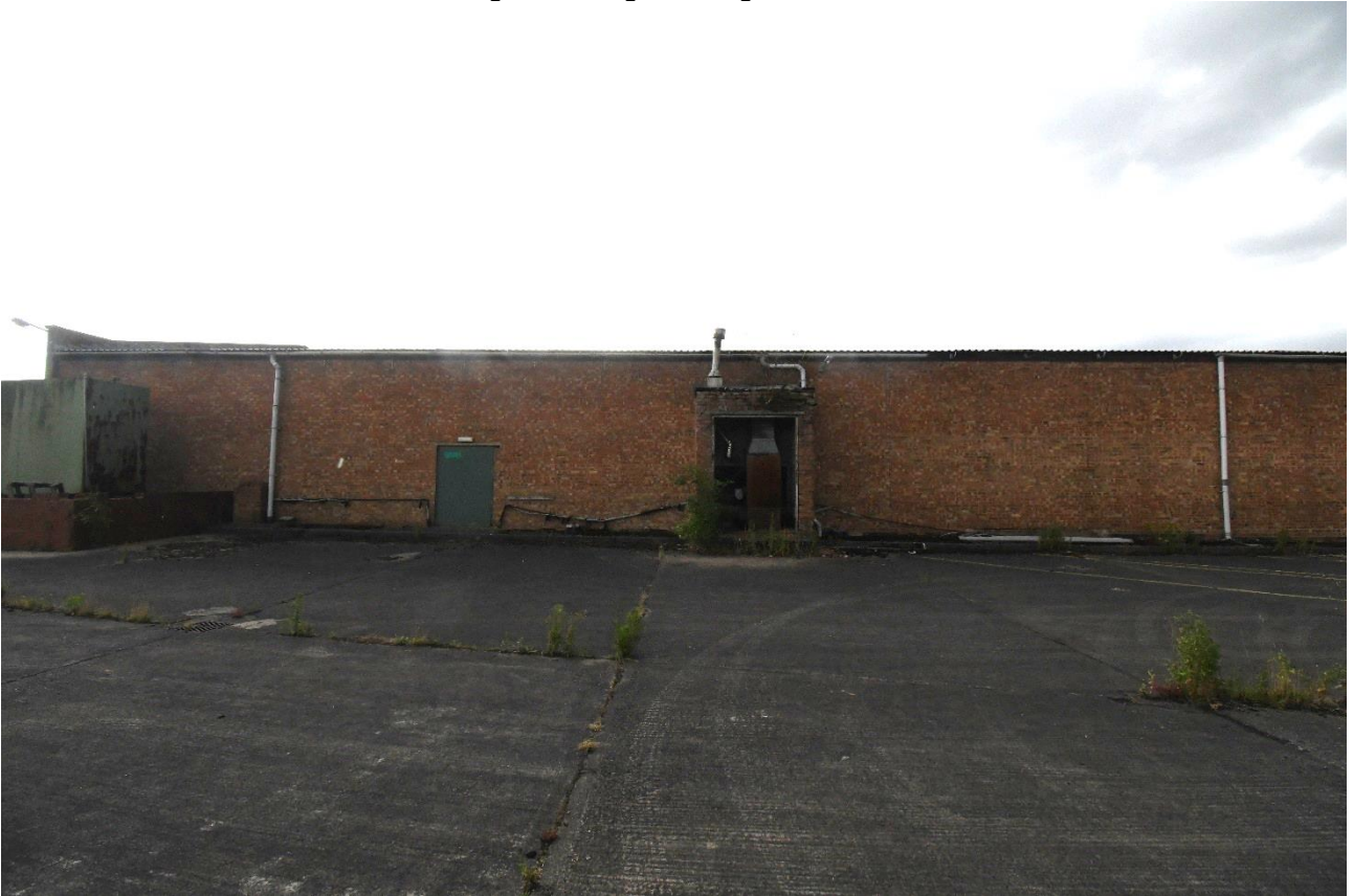
Plate 5: Northeast part, northwest elevation
