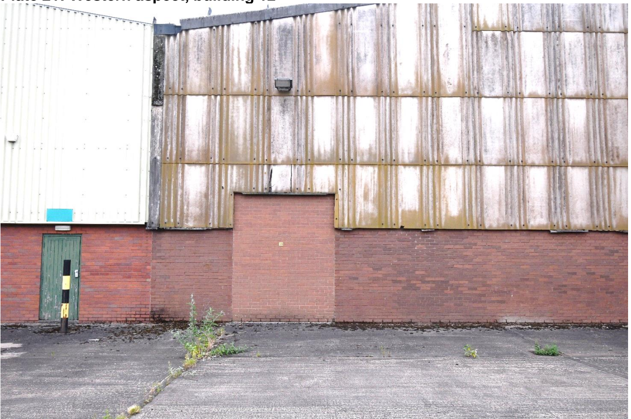
Plate 22: Blocked southwest door, southeast elevation
