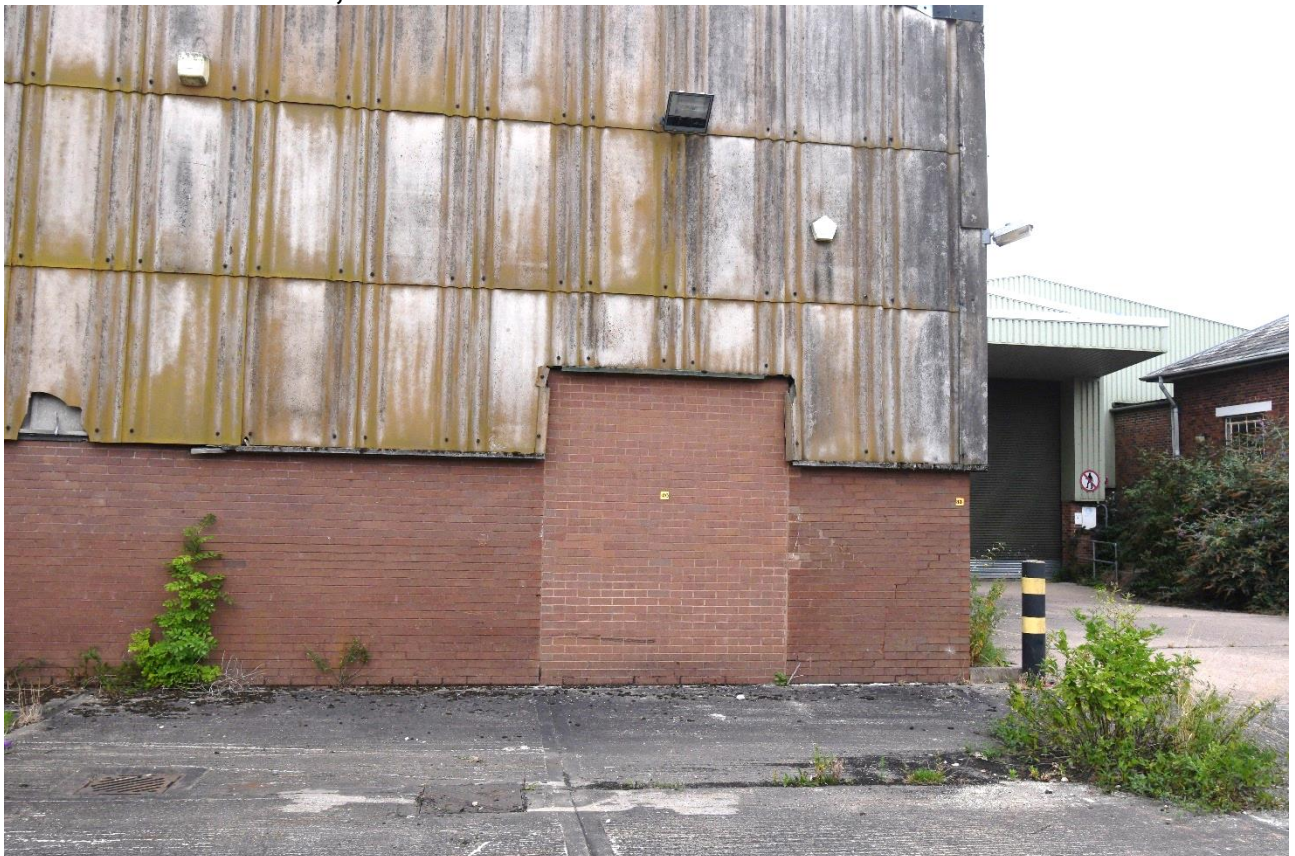
Plate 24: Blocked northeast door, southeast elevation
