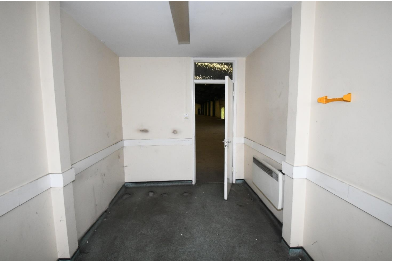
Plate 12: Mess room in partitioned part of building 10
