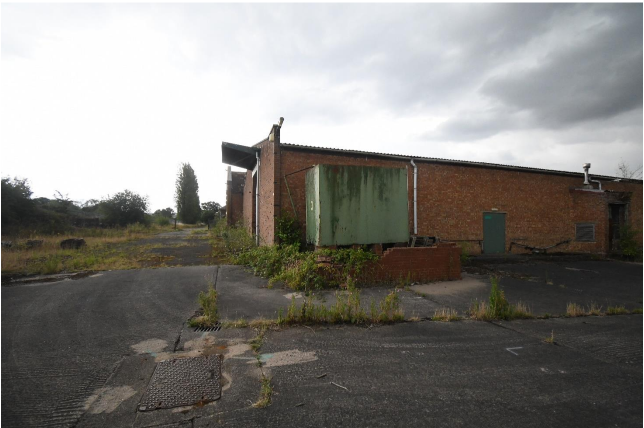
Plate 8: Detail of tank, northeast end of building 10
