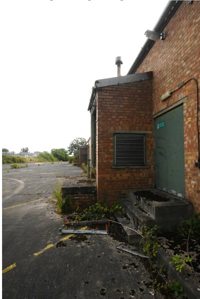
Plate 7: Detail of doors, northwest elevation
