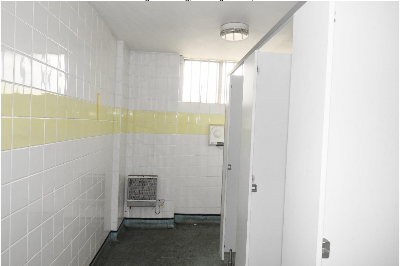
Plate 13: Lavatory in partitioned part of building 10
