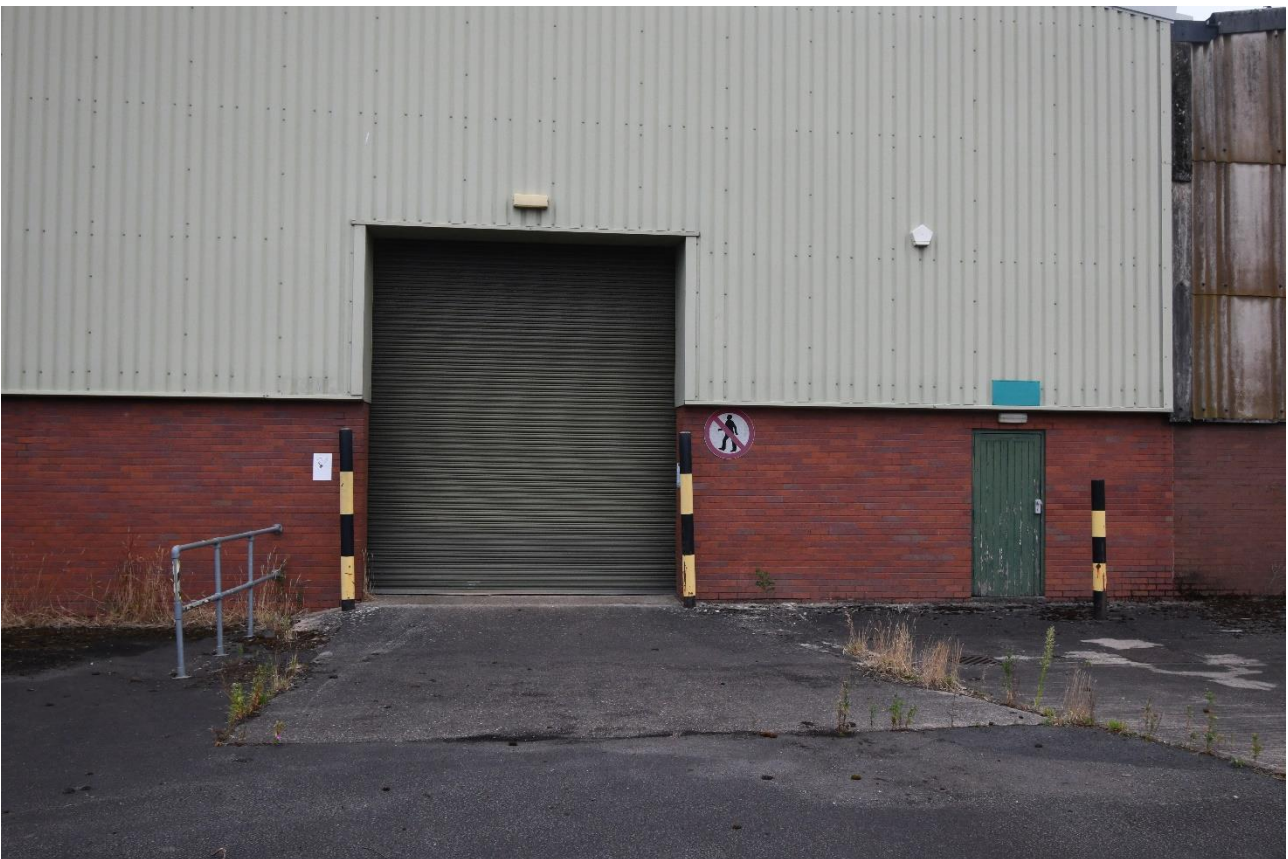
Plate 32: Detail of doors, southeast aspect
