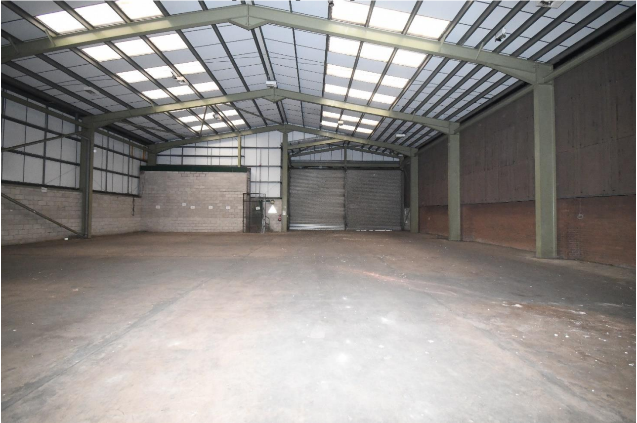
Plate 20: Southeast aspect, building 11
